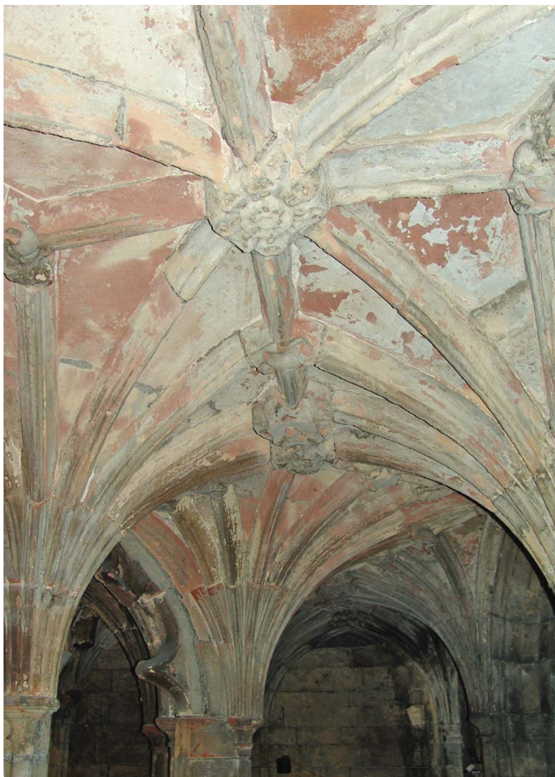
Plate 14 (above). Surface erosion of the stone boss and past overlying paint layers can be noted here.
