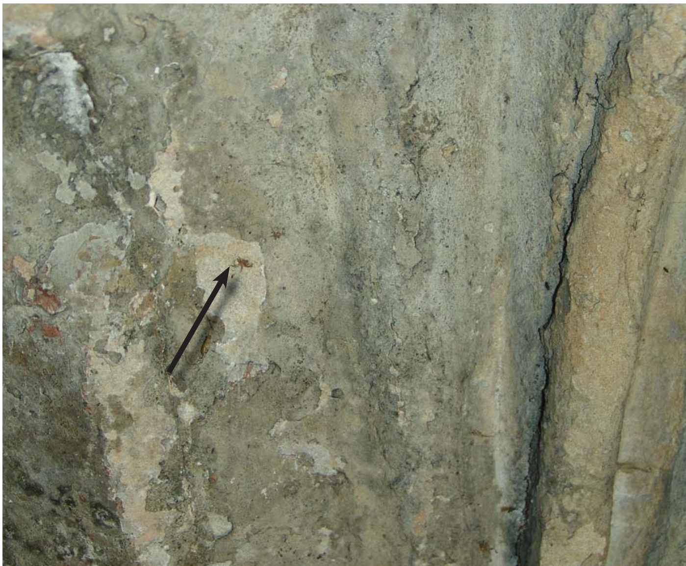
Figure 3. Sample site 2. Area of south wall of upper choir showing typical distribution of fragmentary limewash layers interleaved between dirt layers.
