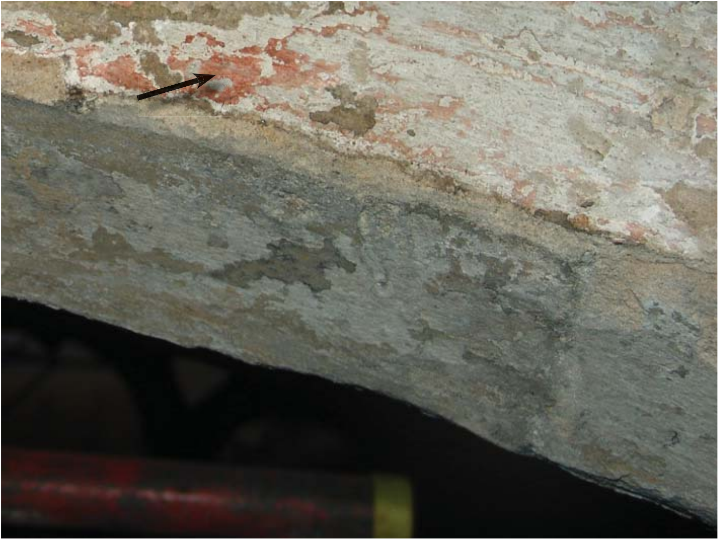
Plate 10 (above). Red pigment was found in small isolated areas across the vault, although as the cross-section analysis proves this has been applied over a number of white layers, suggesting it is of a later date.
