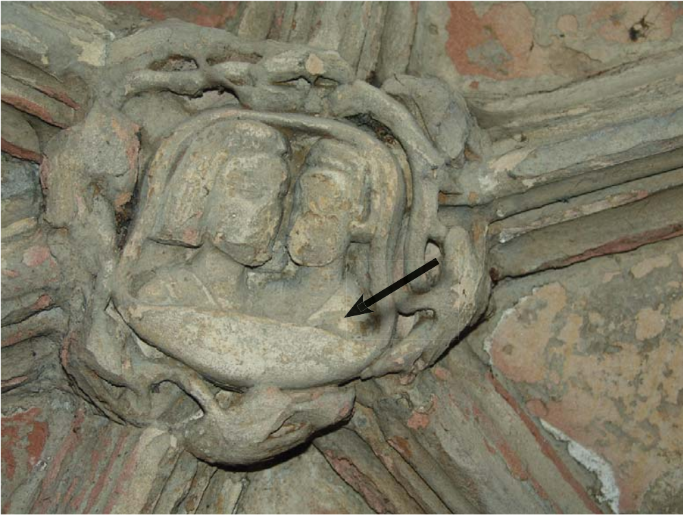
Plate 8 (above). Evidence for a green pigment was noted across a number of different areas of the vault - here within boss 63 CB N.
