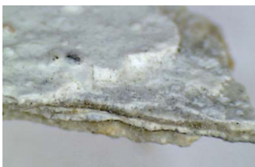
Figure 4. Sample 2. Overlying limewash layers of varying thickness, interleaved between dirt layers. (x 200 magnification)
