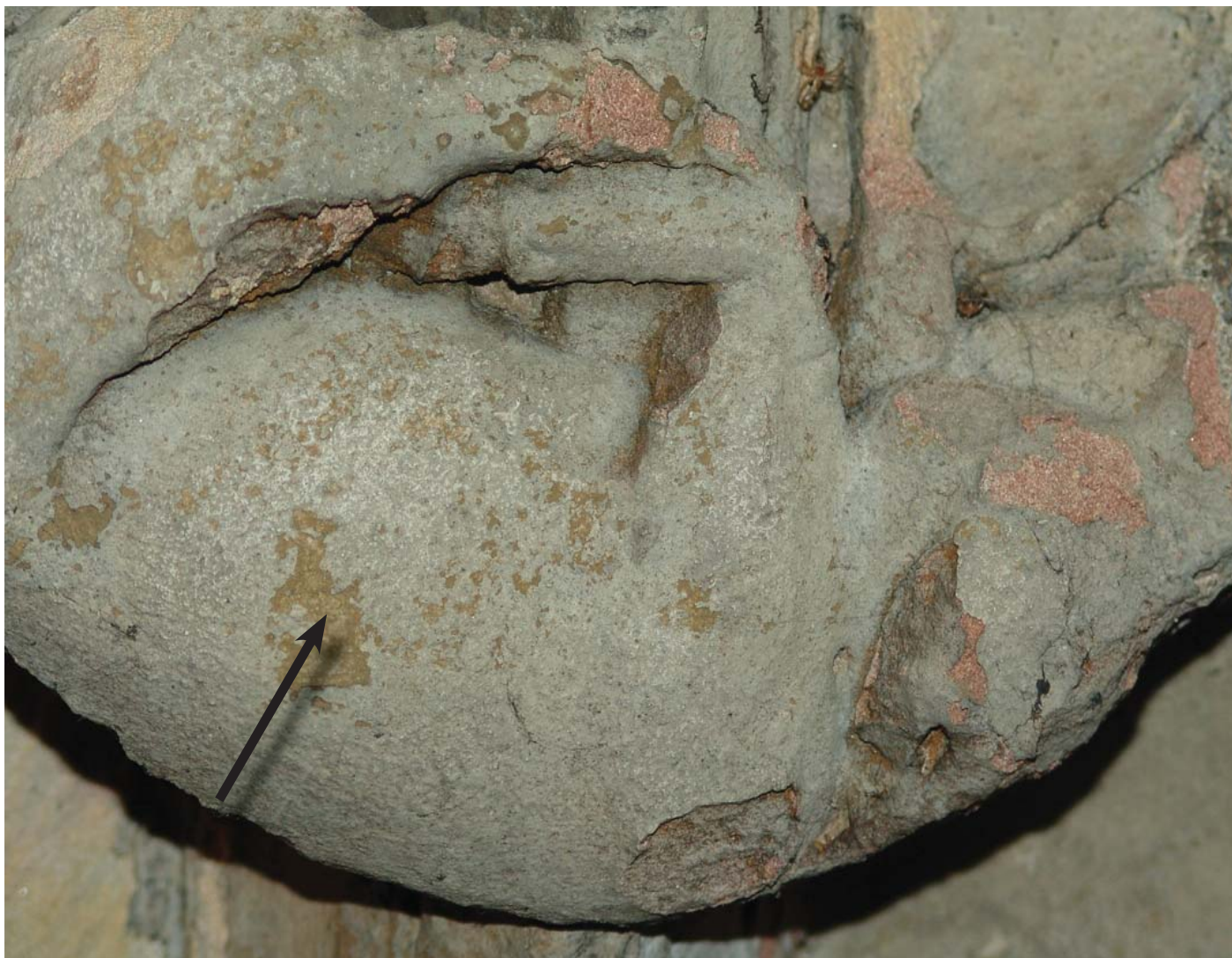
Figure 10. Sample site 5. Boss 64 SB. Here evidence for the underlying green pigment can be noted, as well as general levels of deposited dirt and other debris.
