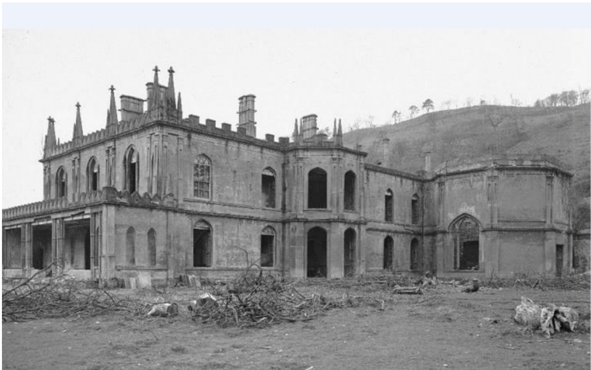
Figure 44: Pre-demolition 1951, note tree sections.
