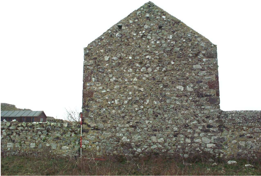
Skomer Island Farm outbuilding range: west wall exterior, from west
