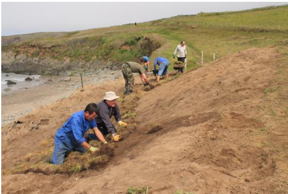
Photograph 12. Re-turfing the site.
