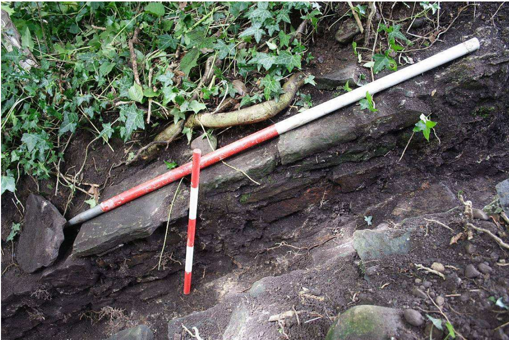
Photo 18: NW facing of the inner face of the side wall of the same channel. 1 x 1m & 1 x 0.5m scale.
