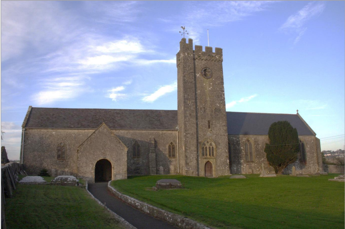
Photograph showing the nave and tower of Monkton Priory Church. Looking north.
