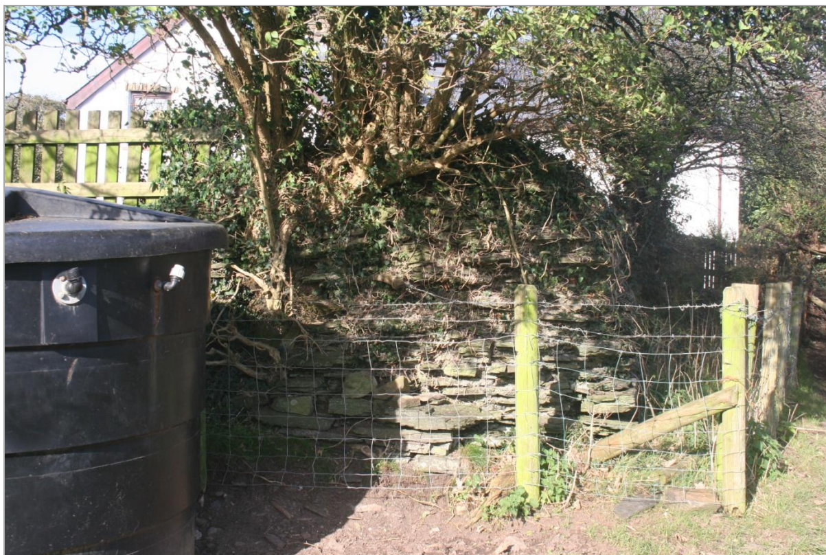
All that remains today of the medieval hospice of St Mary's is a short length of ruined wall that now lies at the end of a modern garden.
