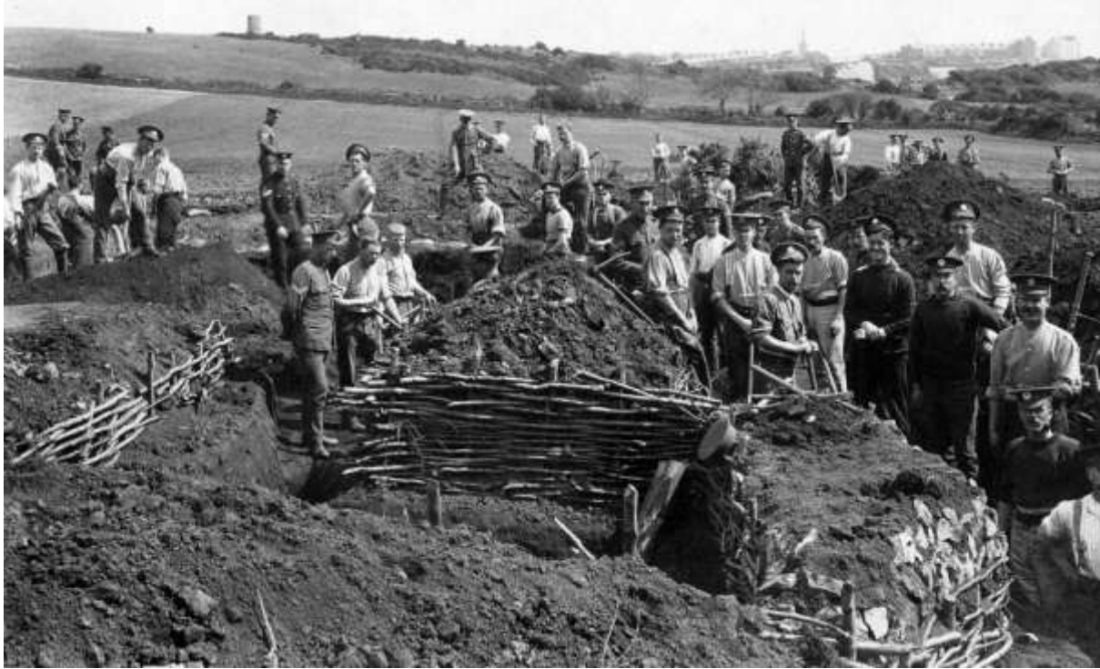
Penally practice trenches under construction, image courtesy of Roger JC Thomas
