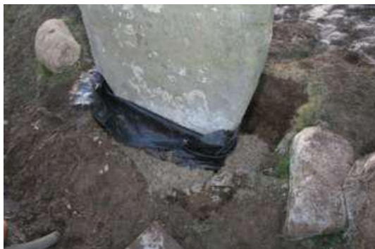
Photograph 16. General view of the stone replaced in the socket with geotextile acting as a separation layer between limecrete and the stone. The limecrete ring was the third of five overall layers, securing the stone firmly in position. Excess geotextile was removed before the turf was re-laid. Photographs: Elliot Ryder Conservation.
