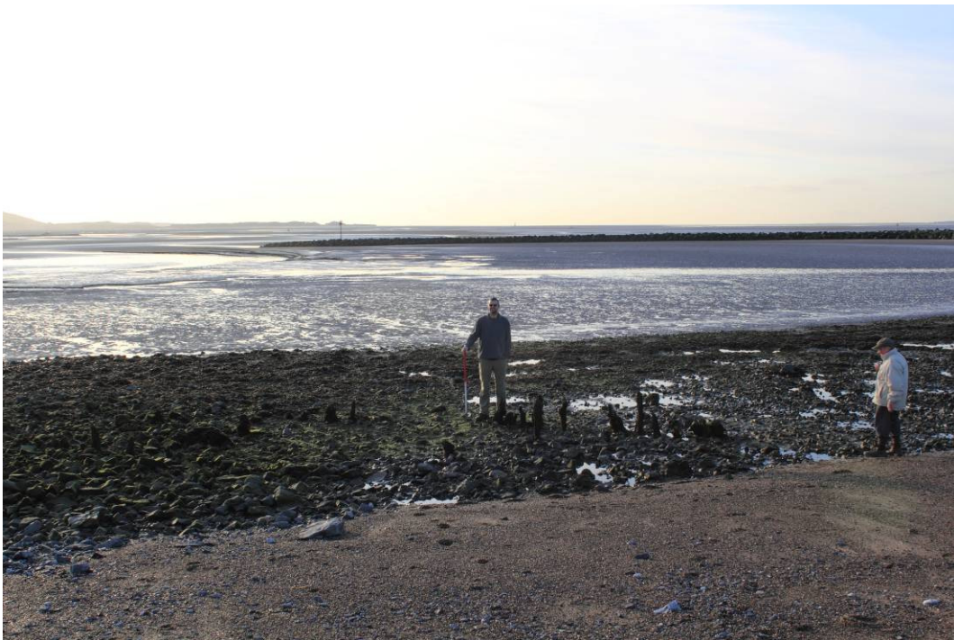
Photo 2: Upright timber posts exposed on the foreshore at Llanelli
