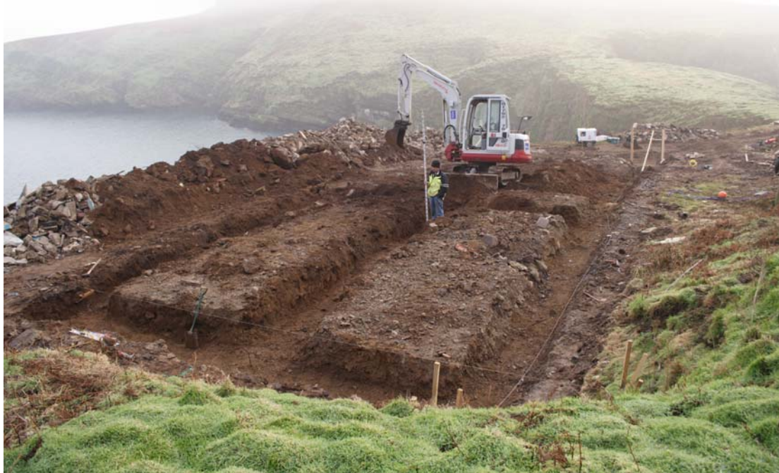
Photo 1: Trenches excavated previously. View east
