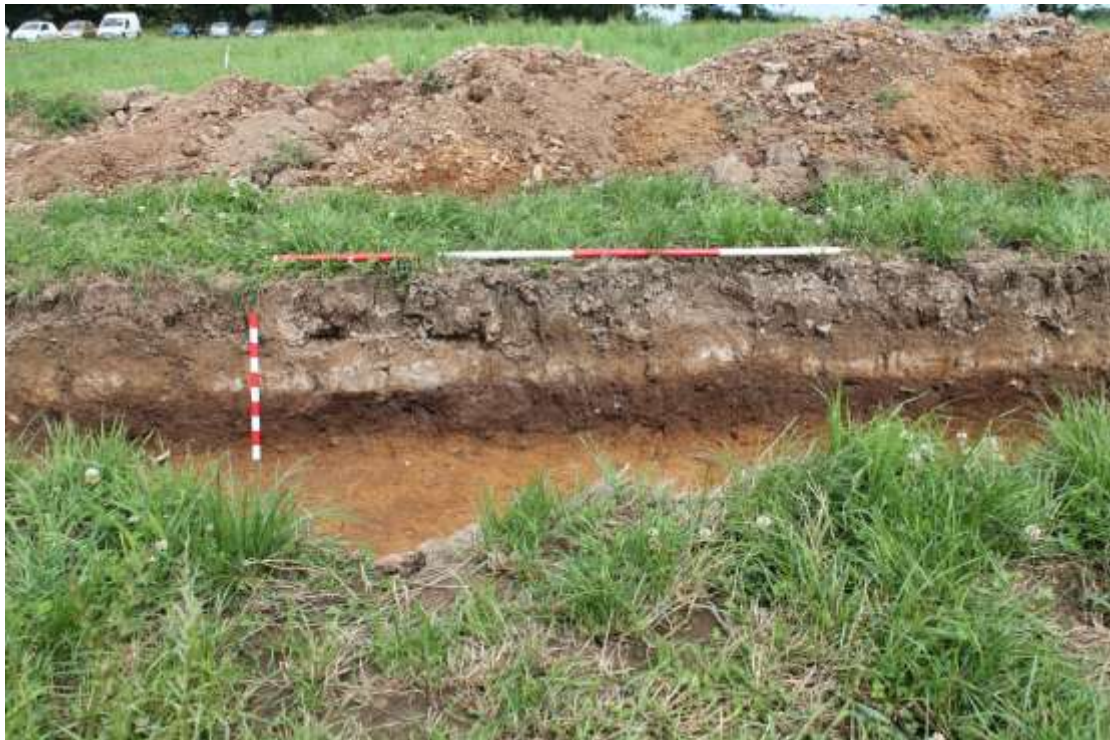
Photo 15: Representative photo of section of Trench 3B showing the clear distinctions between the light grey clay layer and buried darker soil below
