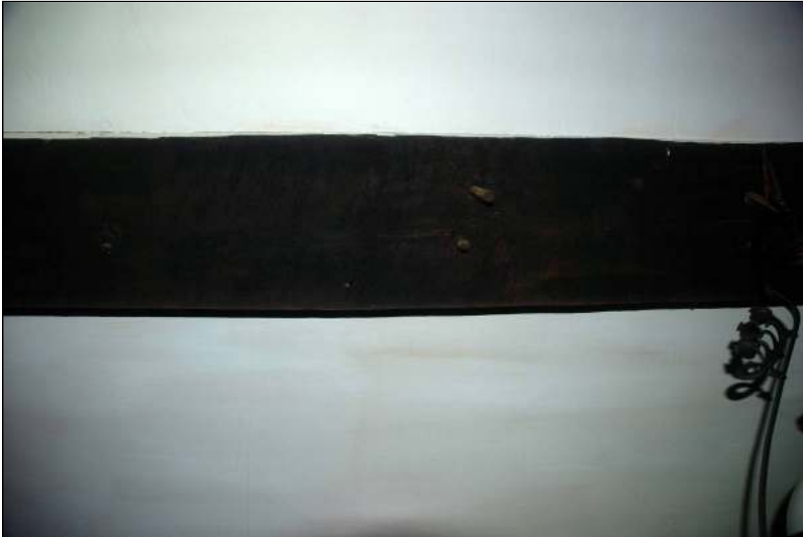
Plate 9: Pegs showing the positions of the common rafters attached to the lower front purlin
