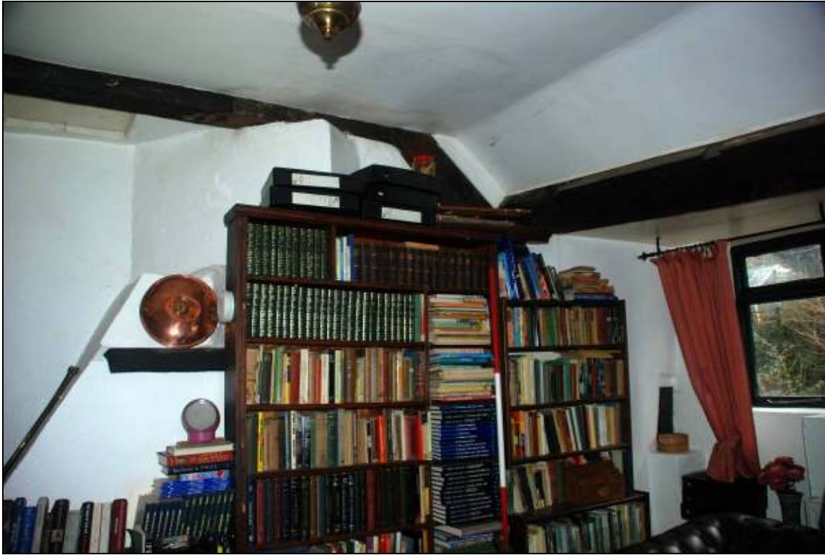
Plate 7: Truss 1, looking east
