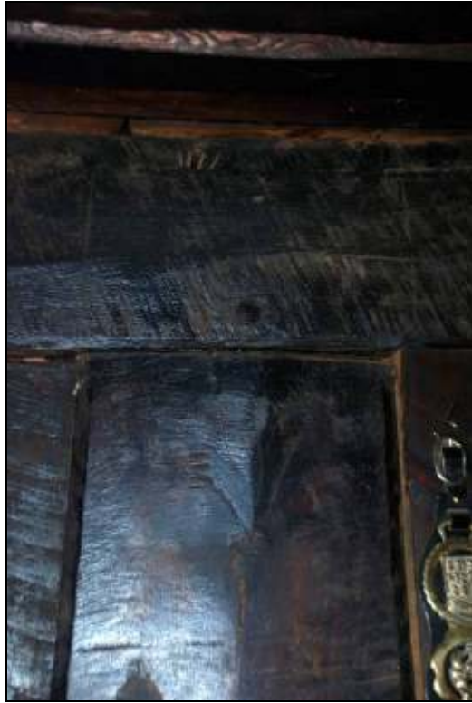
Plate 18: Carpenter's mark of "IIII" on partition rail and post
