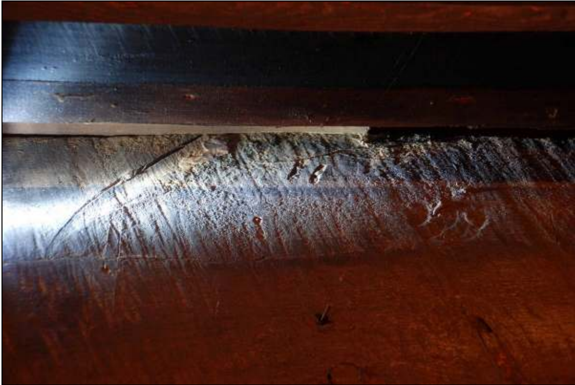
Plate 16: Carpenter's mark of "II" on partition
