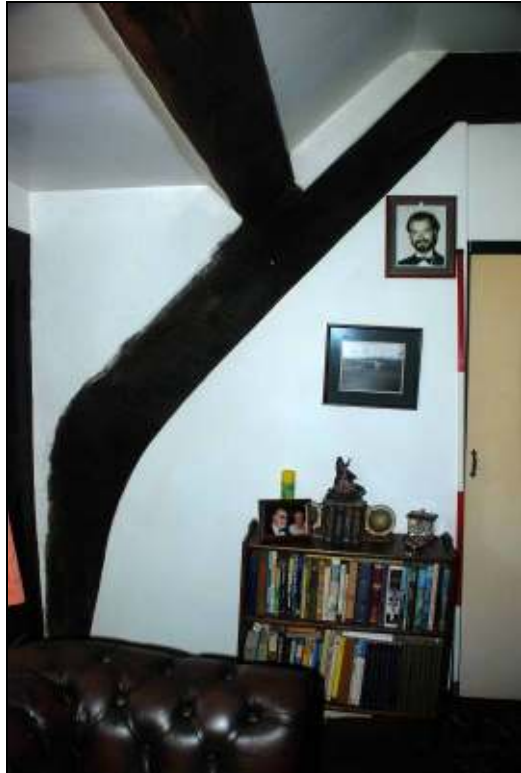
Plate 12: Truss 2, south east cruck, looking north
