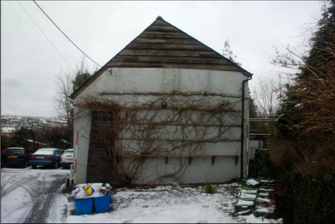
Plate 3: South west gable end
