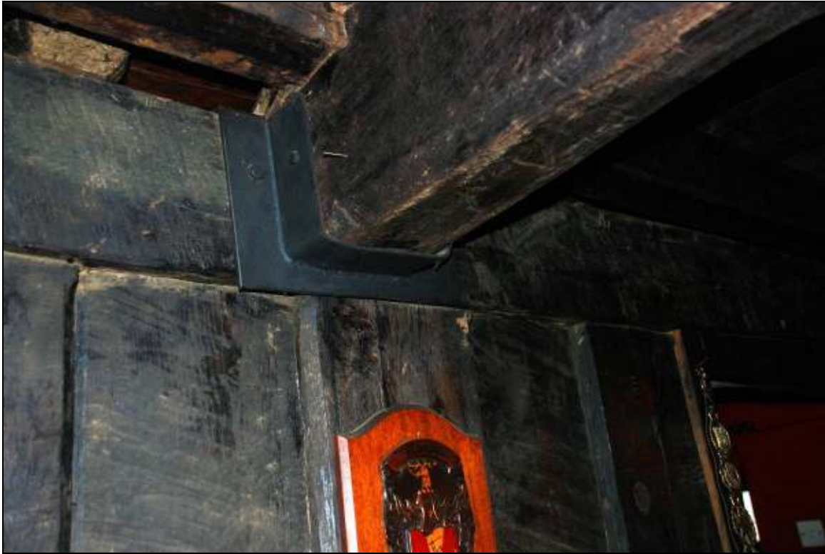
Plate 21: Transverse beam in lower NE room, looking west
