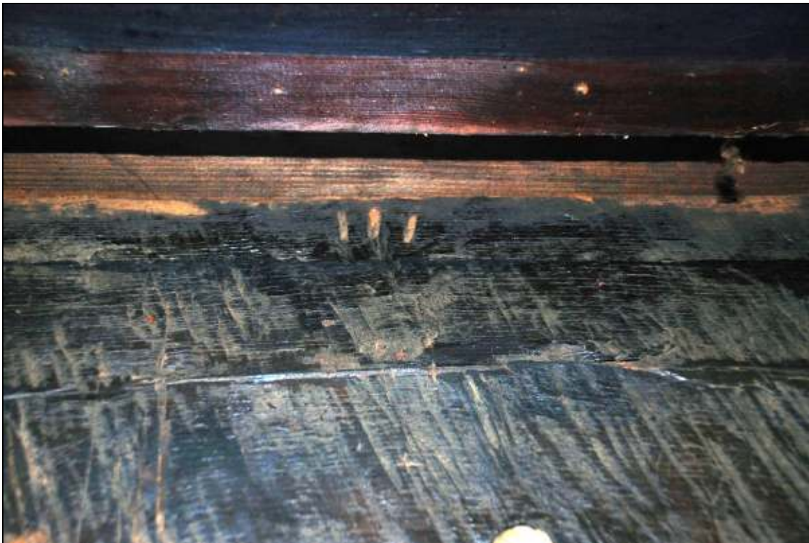
Plate 16: Carpenter's mark of "II" on partition
