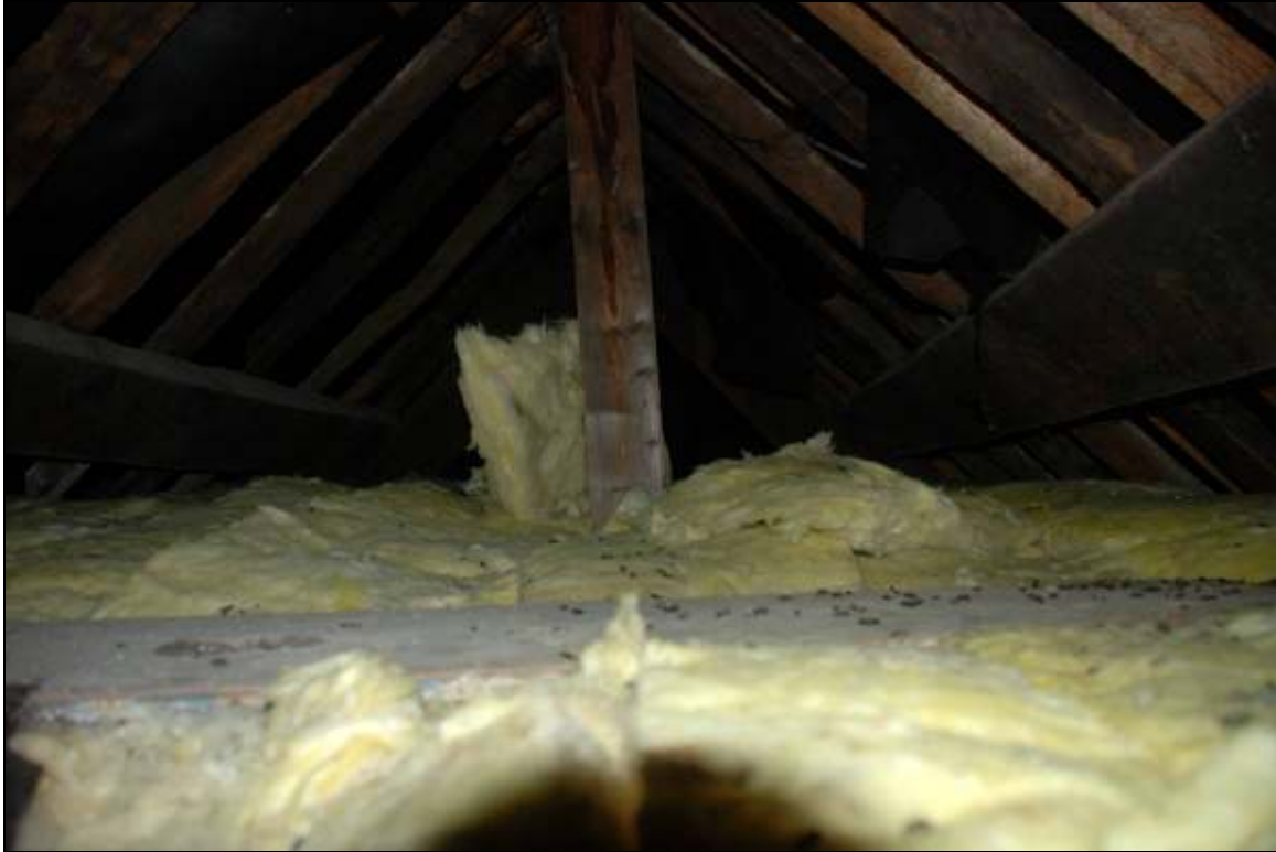
Plate 10: The roof space looking south west
