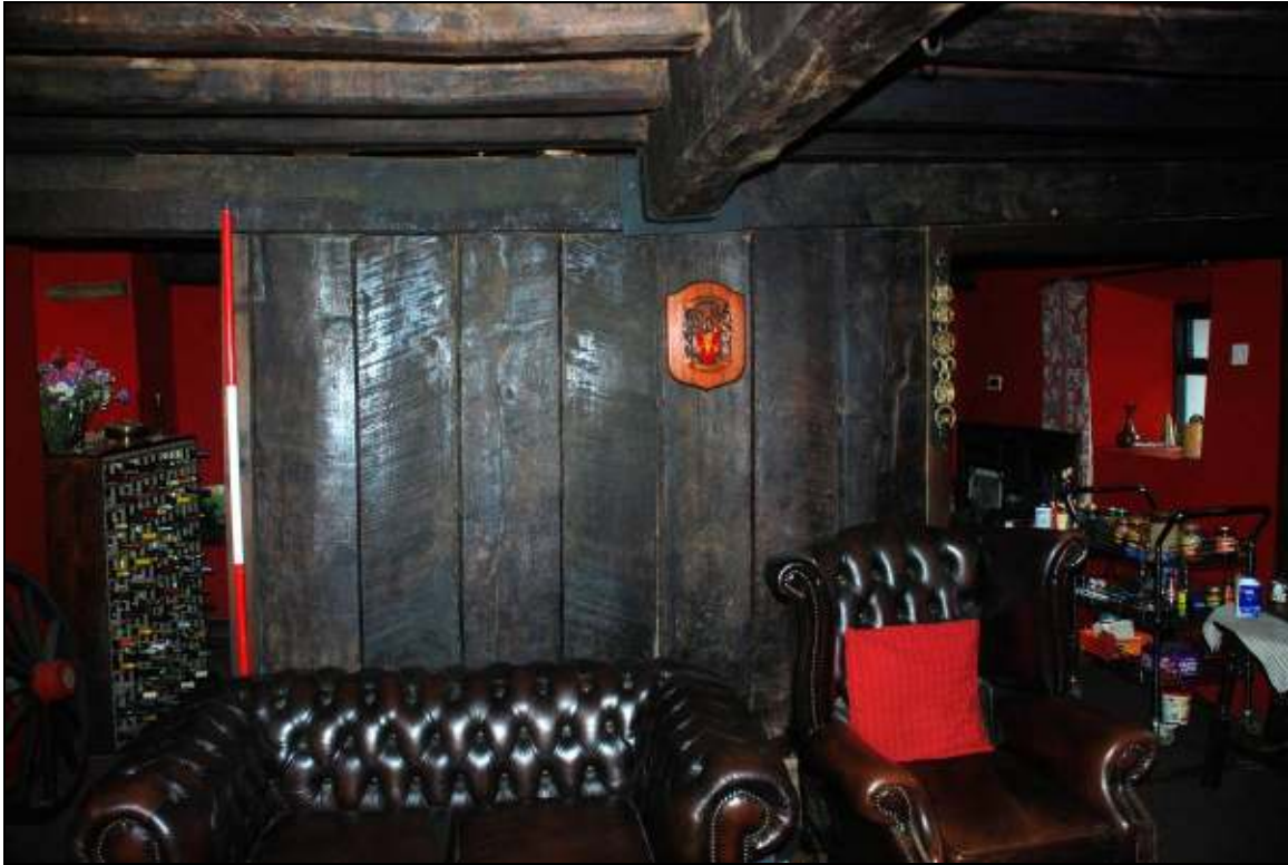
Plate 15: Post and Plank Partition looking south west
