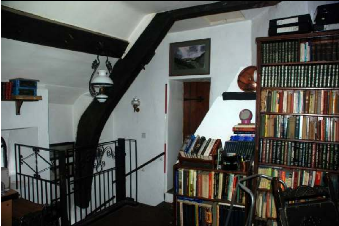
Plate 6: Truss 1, looking north
