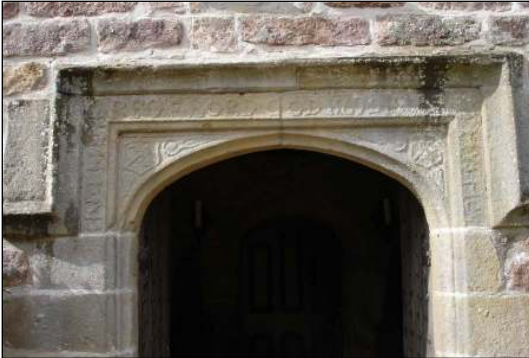
Figure 1: Photograph of inscription over main porch door, bearing the date 1569
