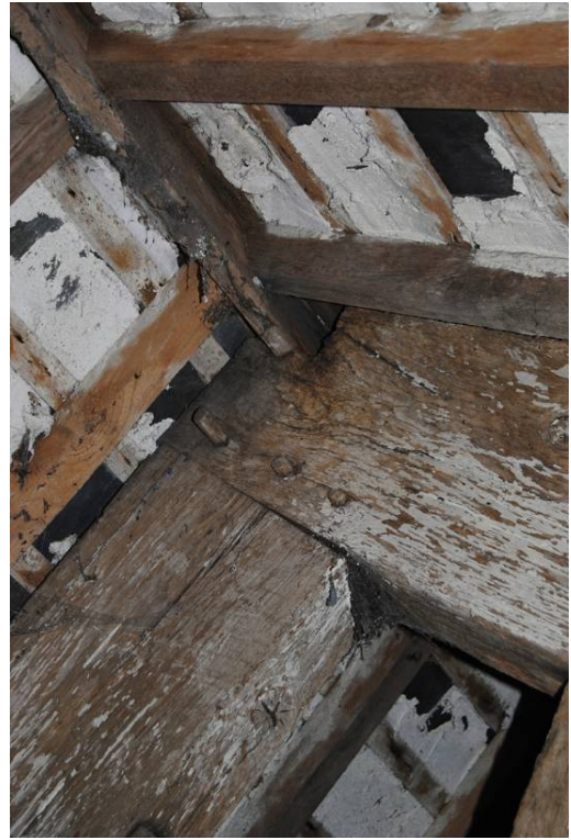
Figure 17: Collar beam truss; apex detail.
