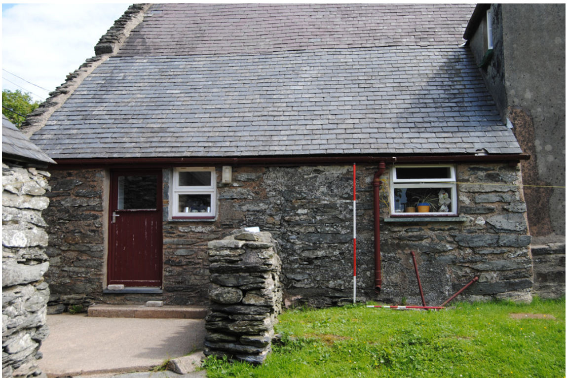
Plate 10: Undated, pent-roofed extension to north-west corner (note straight joint to right of boundary wall).
