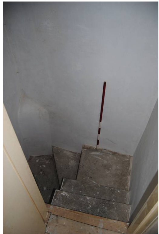
Plate 24: Winder stair from [1F05].
