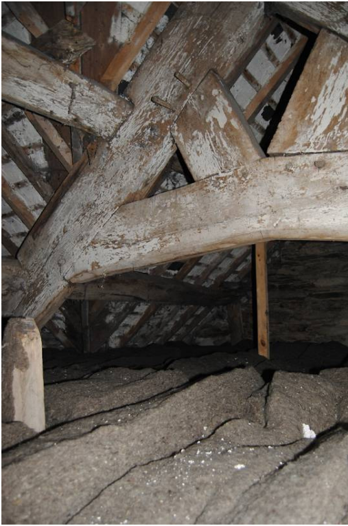
Plate 16: Primary collar beam truss at Bay 1/2.
