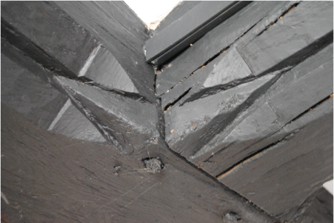
Plate 13: Detail of moulding at intersection of transverse (left) and longitudinal (right) floor beams [GF01].
