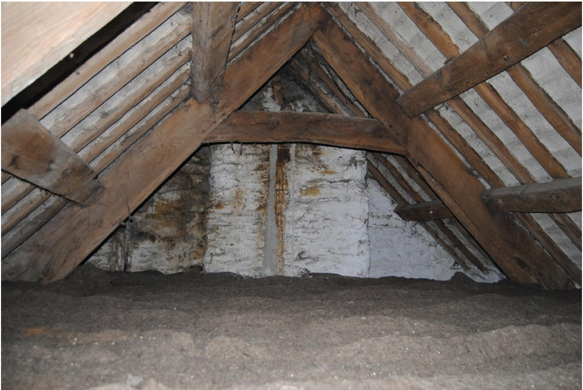
Plate 27: Northern extension; roof structure.
