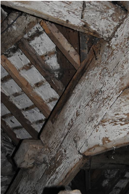
Plate 18: Collar beam truss, socket for former wind bracing (upper purlin, north).
