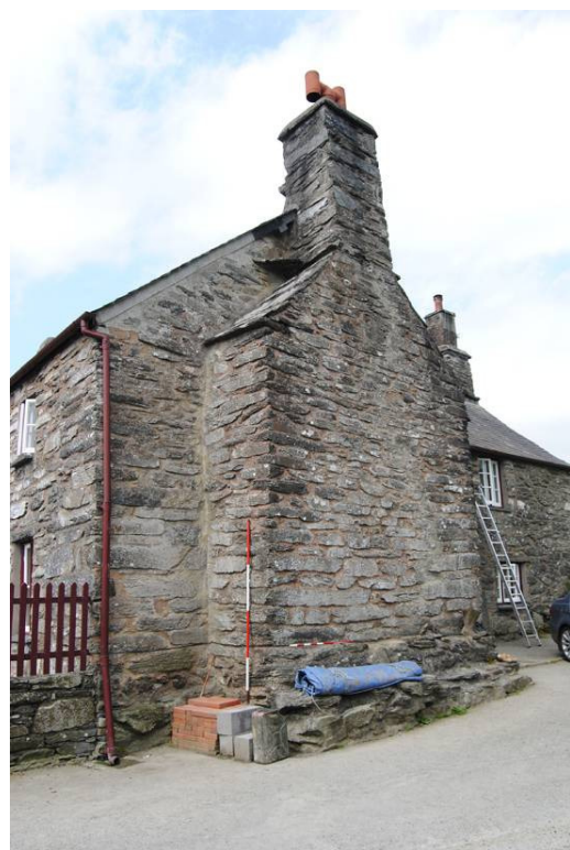
Plate 5: Projecting shouldered stack to east.
