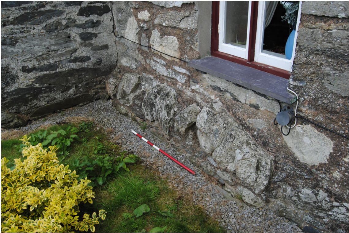
Plate 6: Offset rough stone plinth at base of primary range, south elevation.
