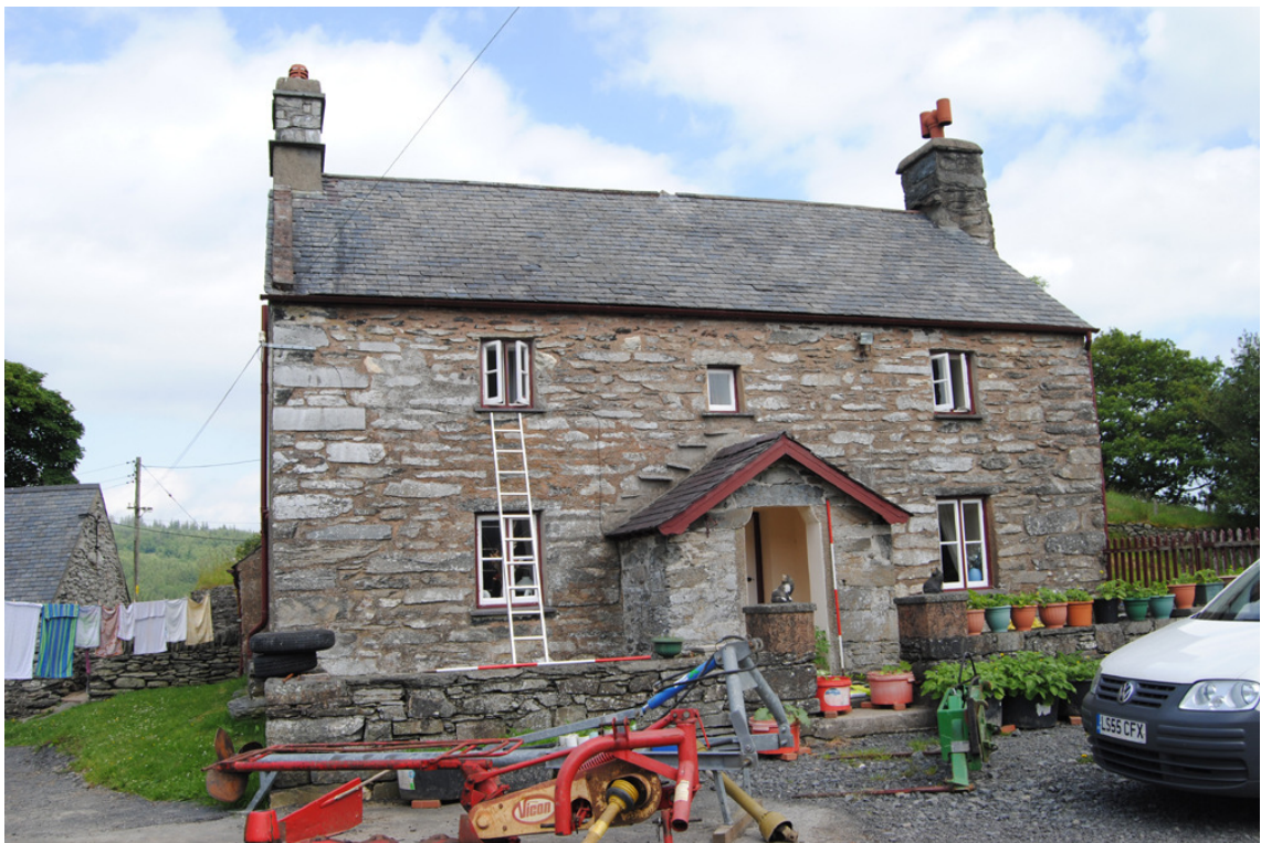
Plate 2: South range, principal (south) elevation.
