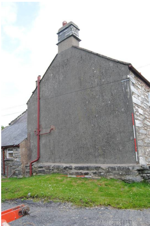
Plate 4: Cement rendered west elevation with ridge stack.
