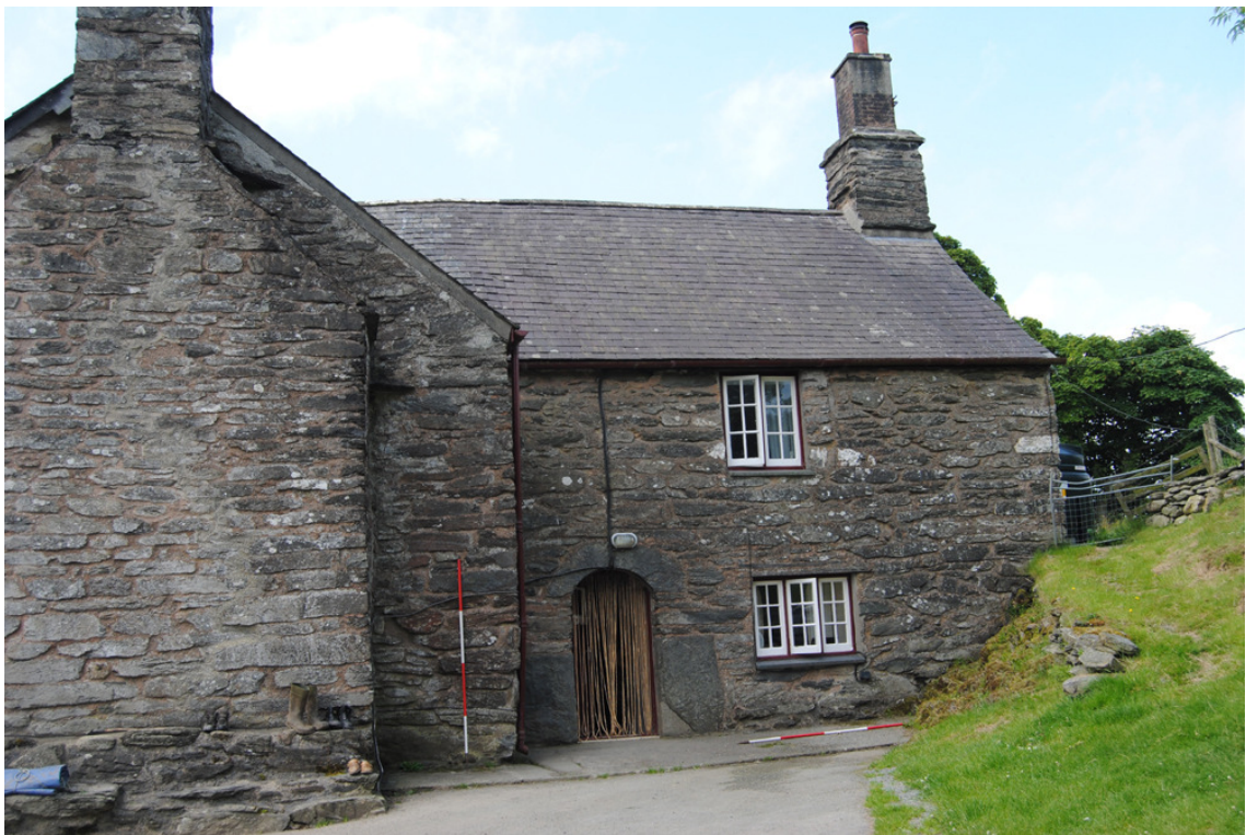
Plate 7: South range, east gable (left) and secondary north range; east elevation (right).
