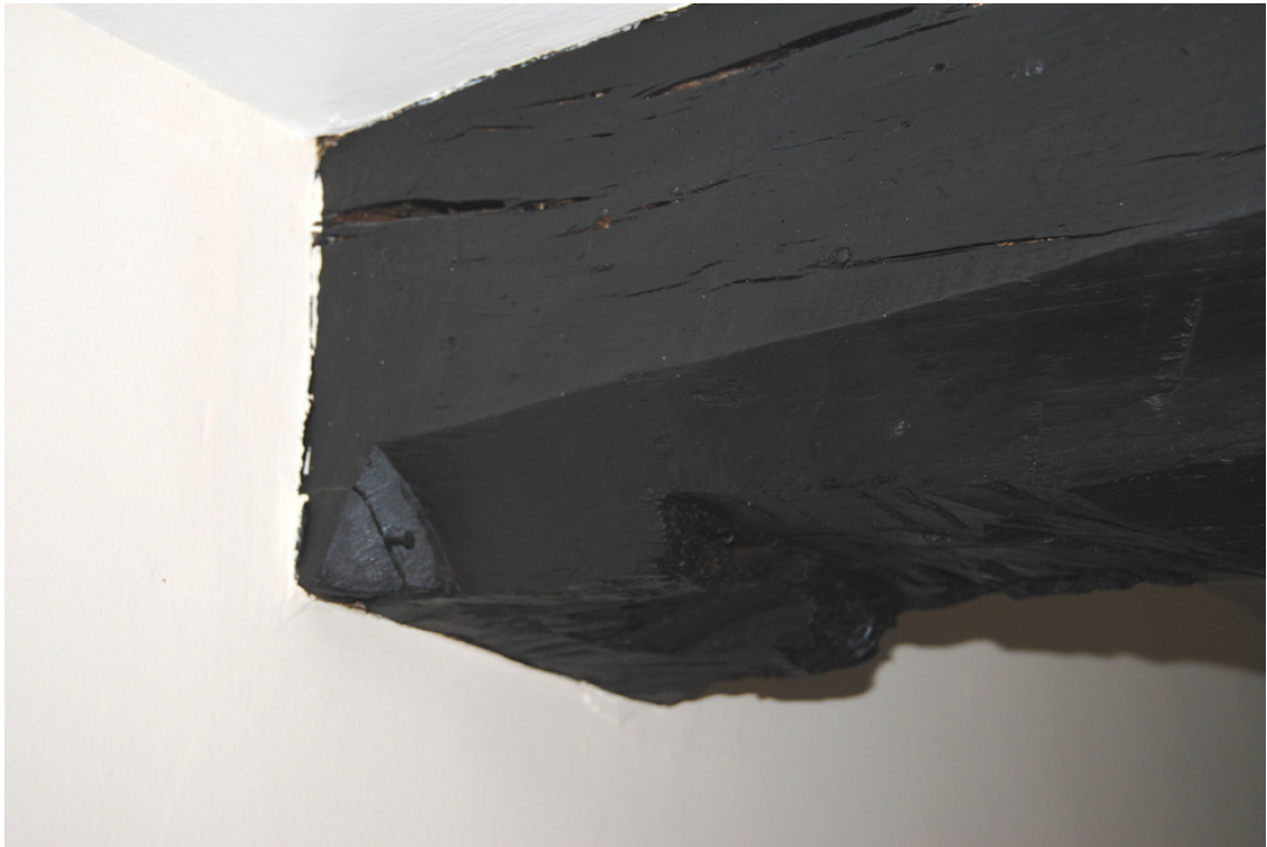
Plate 22: North extension, Room [GF05] detail of transverse beam.
