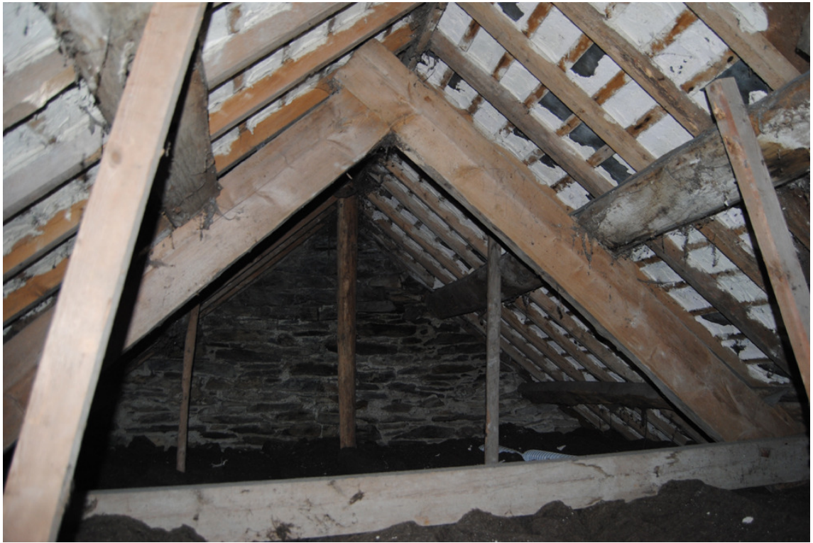
Plate 20: Renewed softwood truss at Bay 2/3.
