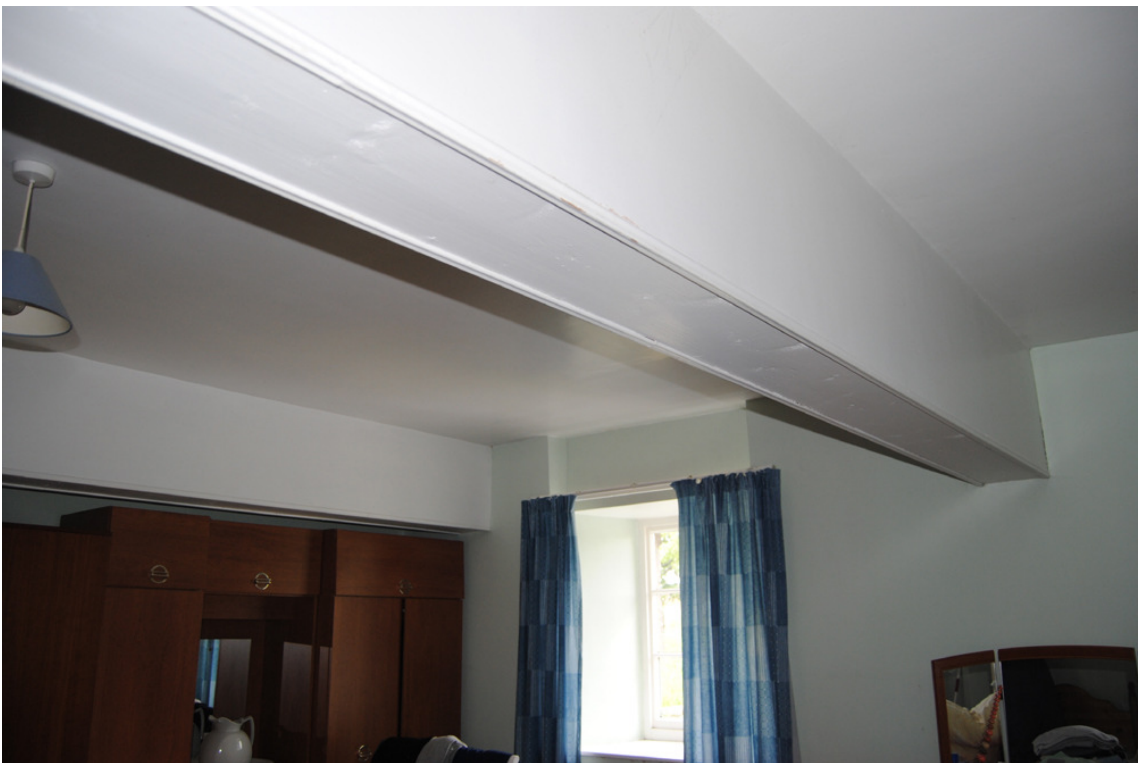
Plate 26: Boxed in transverse (?tie)beams within [1F05].
