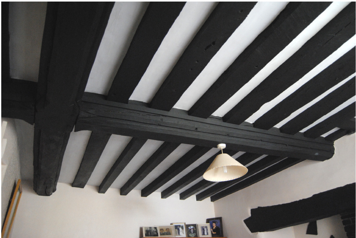
Plate 12: Room [GF01], moulded ceiling beams (dated to 1515/17) and primary joists.
