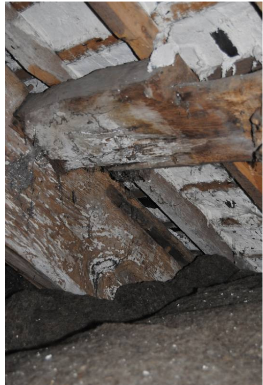
Plate 19: Collar beam truss, socket for former wind bracing (lower purlin, south).
