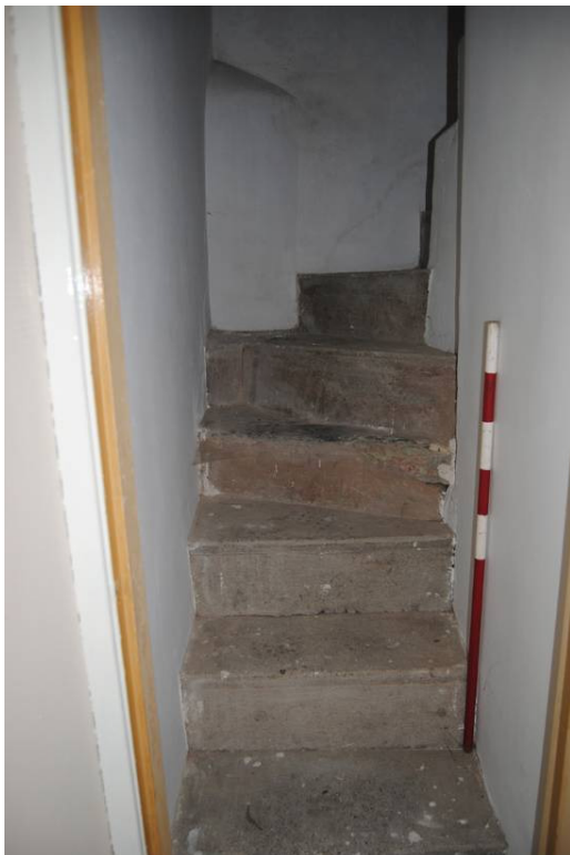
Plate 23: Winder stair from [GF04].
