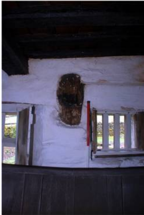
Plate 7: Base of possible cruck frame in main, ground floor room
