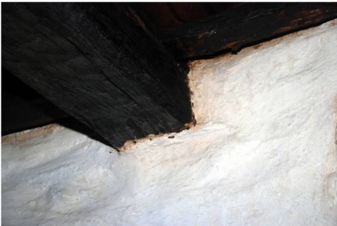
Plate 10: Chamfer and stop on ceiling beam
