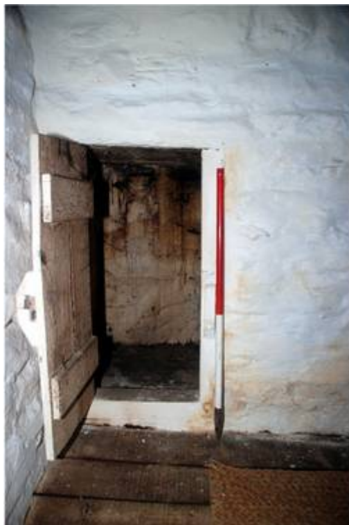
Plate 12: Cupboard in south east corner of the first floor
