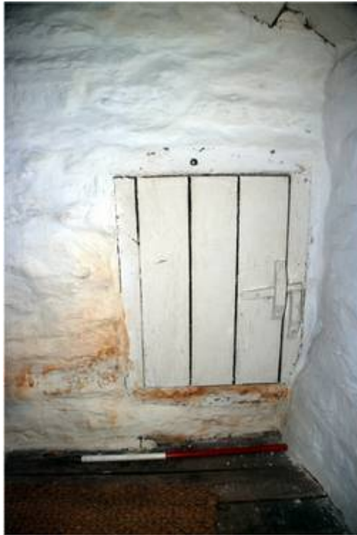
Plate 13: Cupboard in SW corner of first floor
