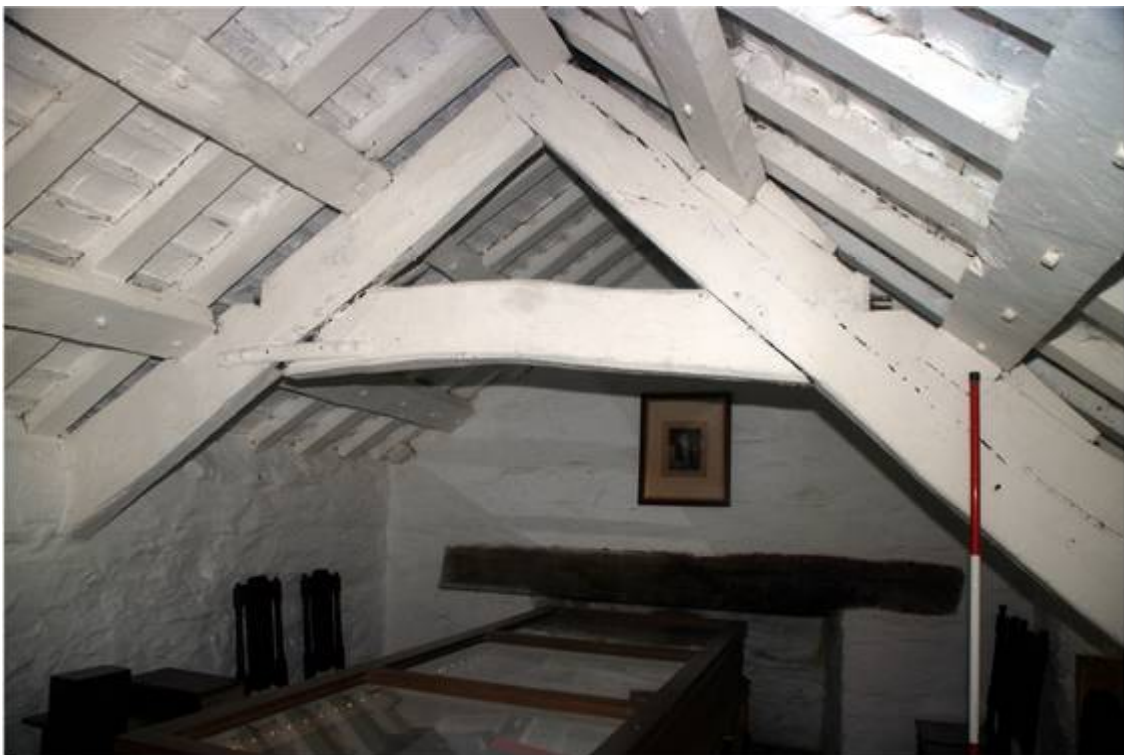
Plate 16: Truss 3, looking NNW
