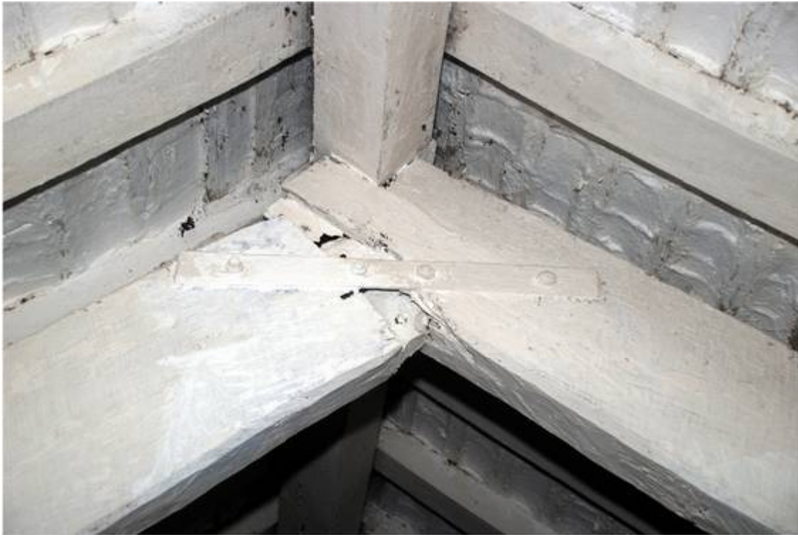
Plate 17: Iron Plate strengthening Truss 1
