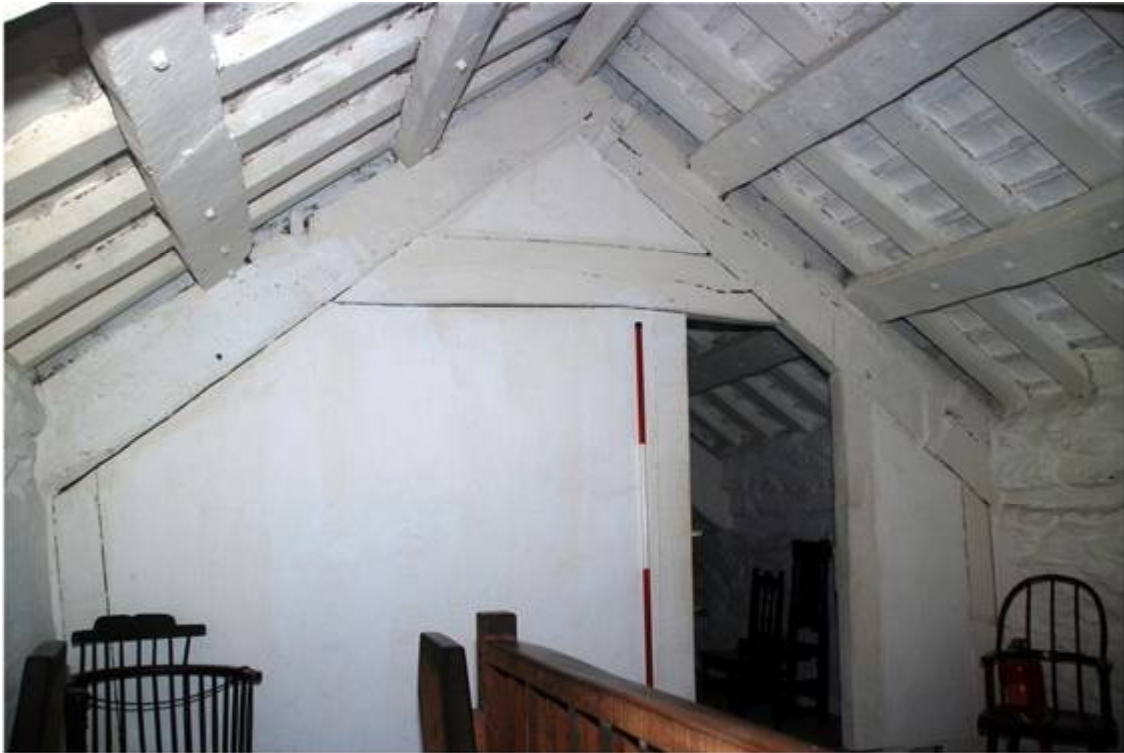
Plate 15: Truss 2, looking north
