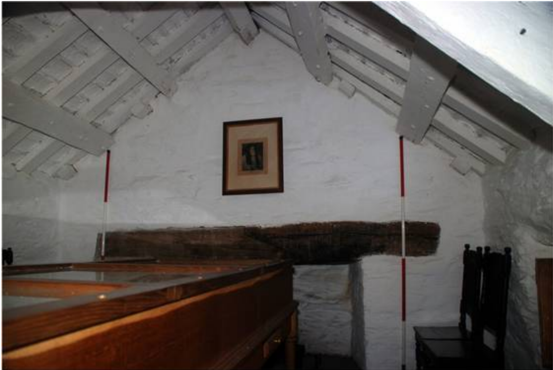
Plate 19: Chimney in the north gable wall
