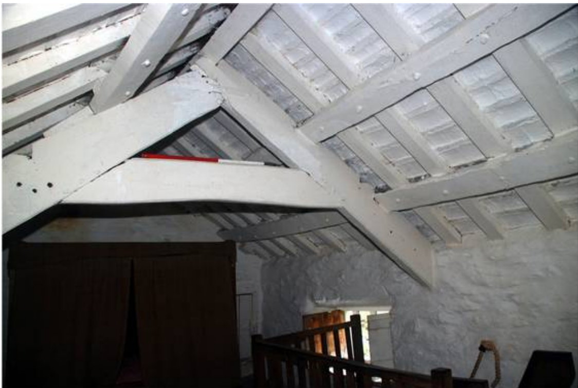
Plate 14: Truss 1, looking SSW
