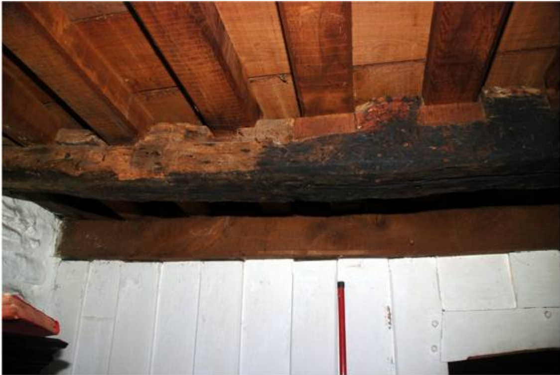
Plate 11: Replacement joists
