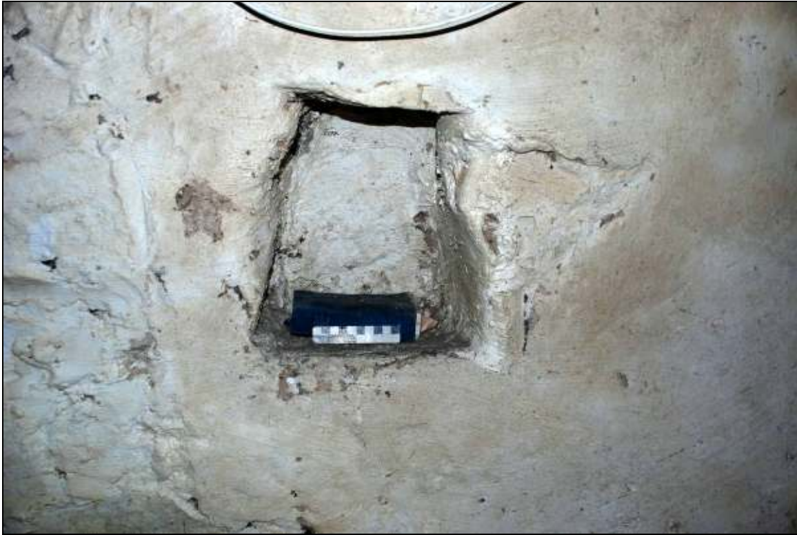
Plate 48: Niche in cellar wall
