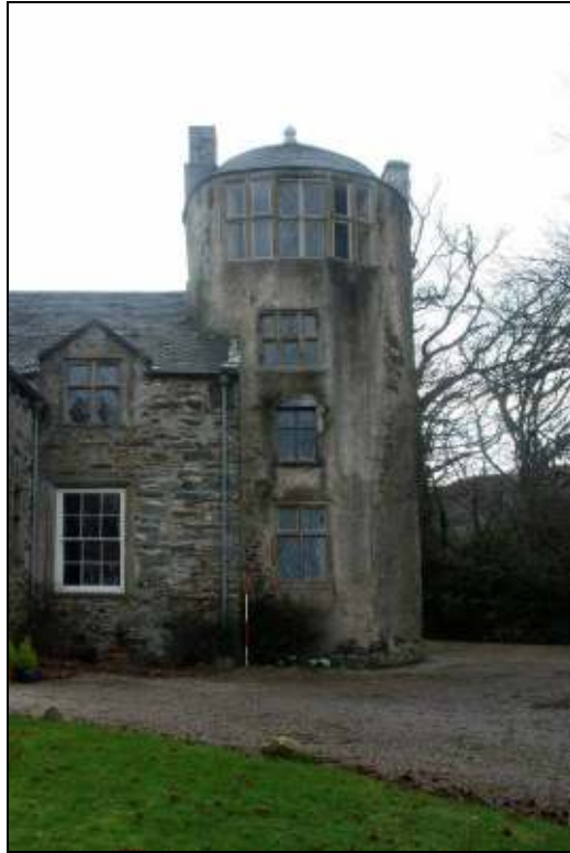
Plate 3: Front elevation of tower
