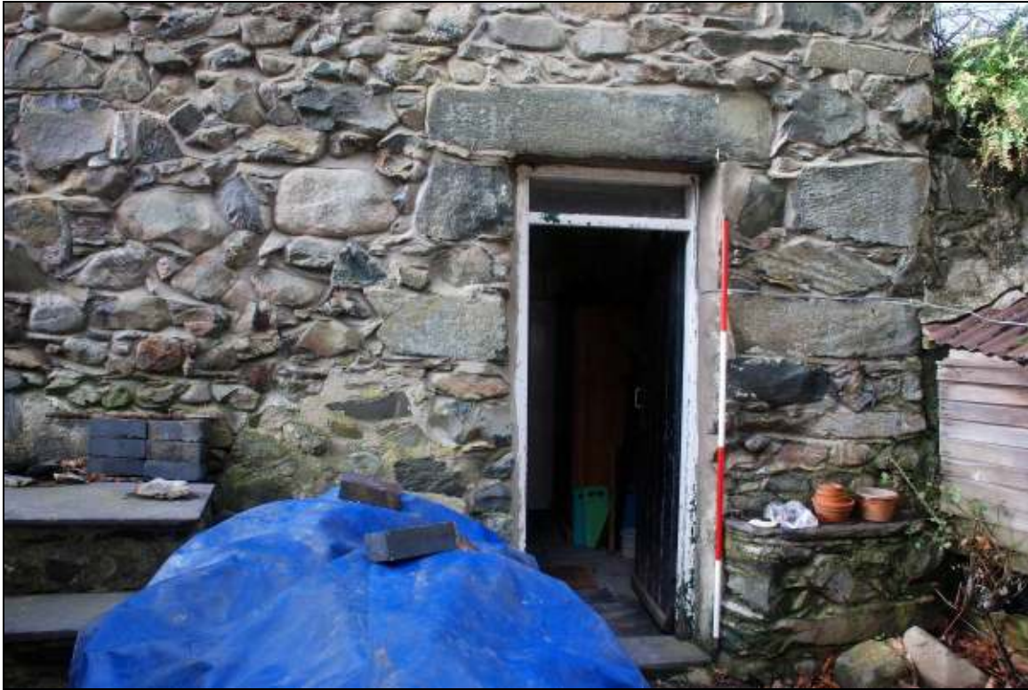
Plate 18: Door in gable end of north eastern range, looking SW
