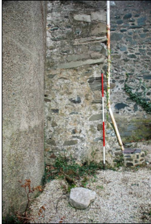
Plate 10: Possible blocked opening in SW corner of central range, looking NE
