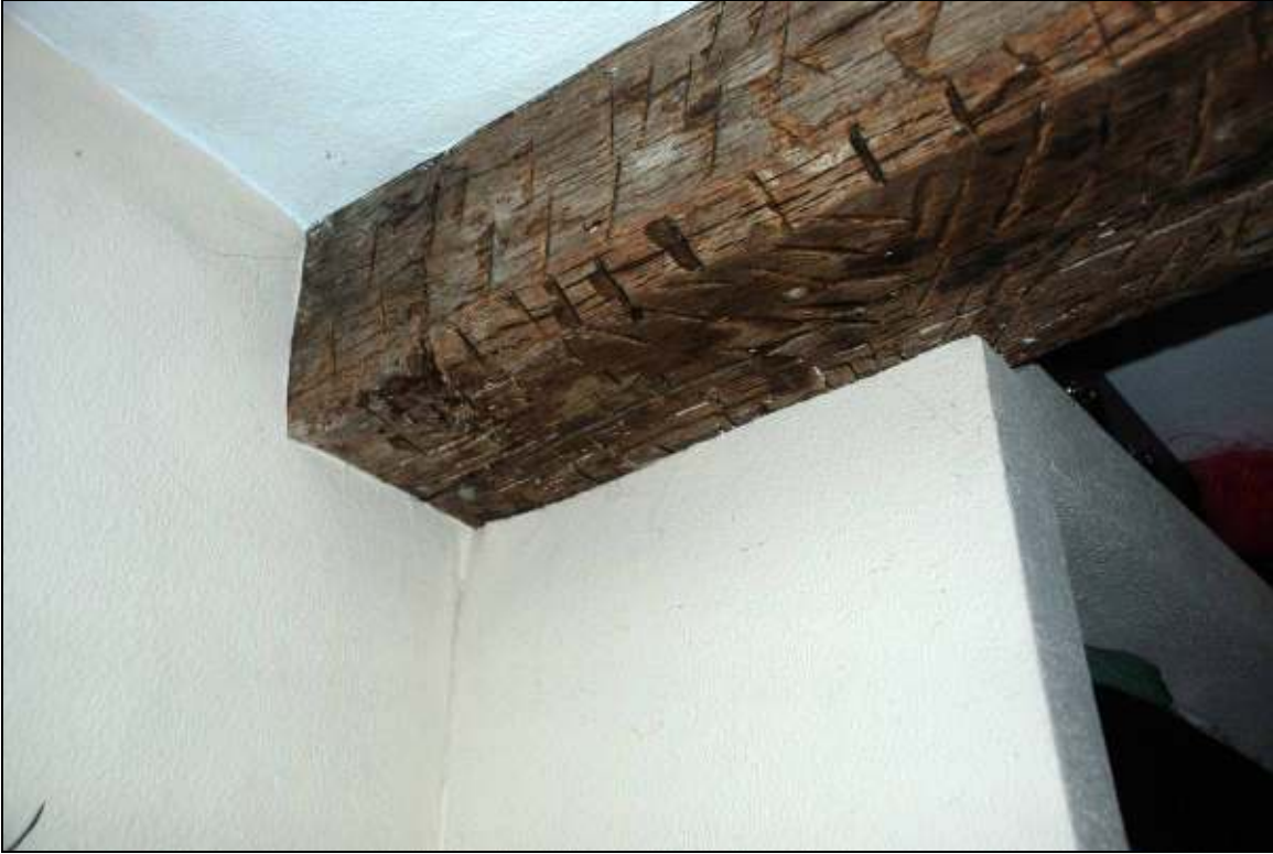
Plate 40: Tie beam on first floor of central range
