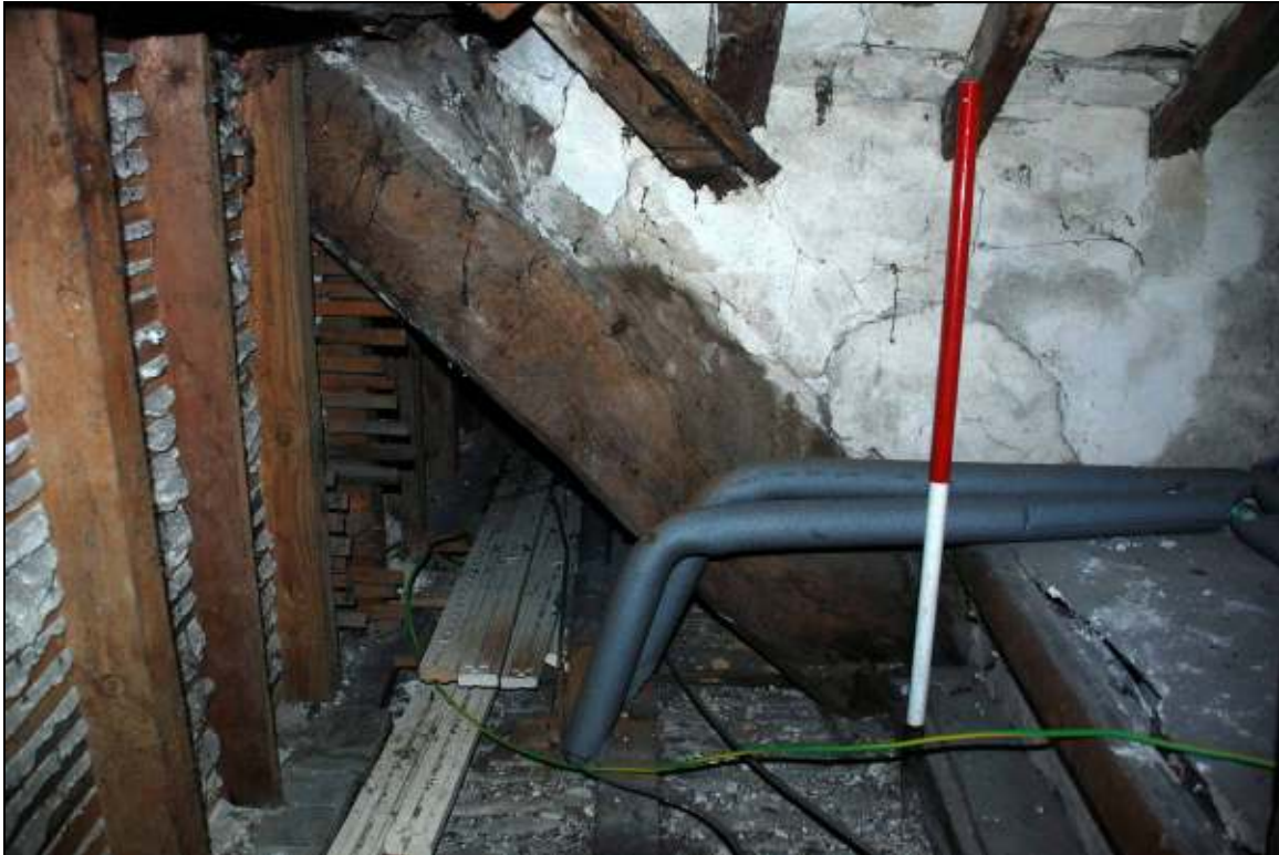
Plate 42: Foot of Truss 5, looking NE
