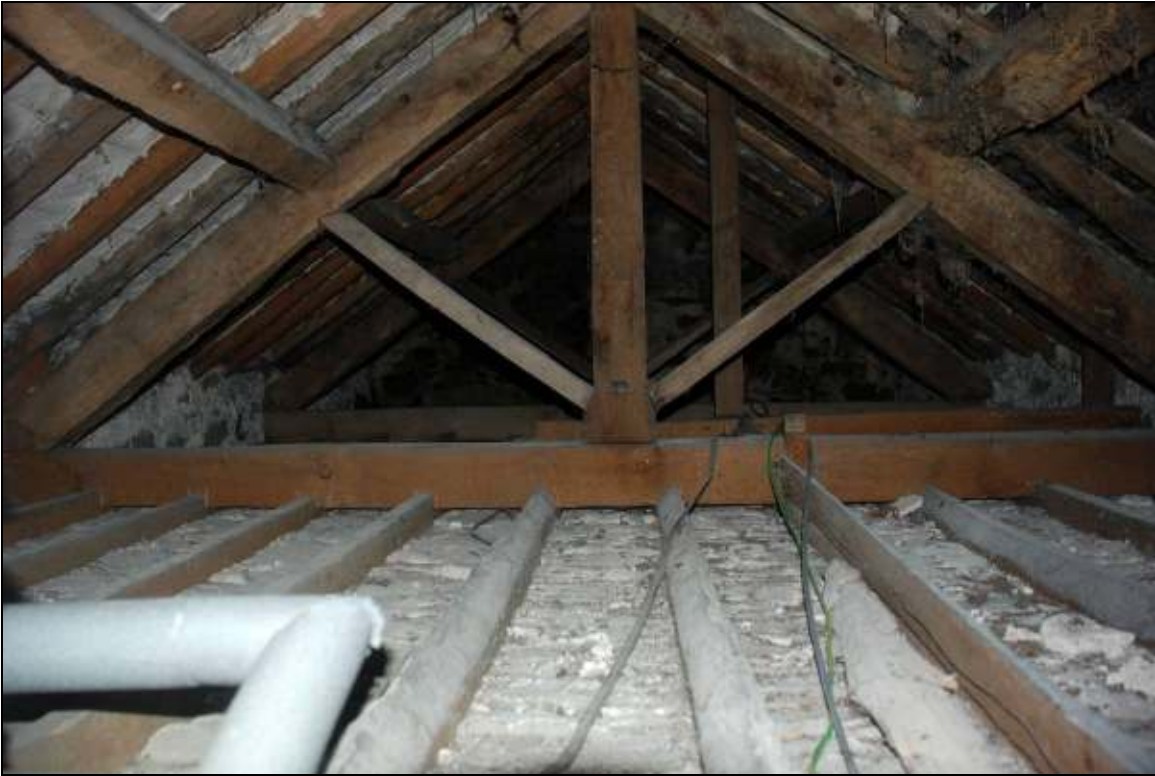
Plate 56: The roof structure for the south wing, looking SE
