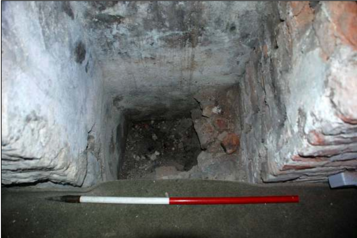
Plate 30: Stone lined recess on first floor of tower, looking down
