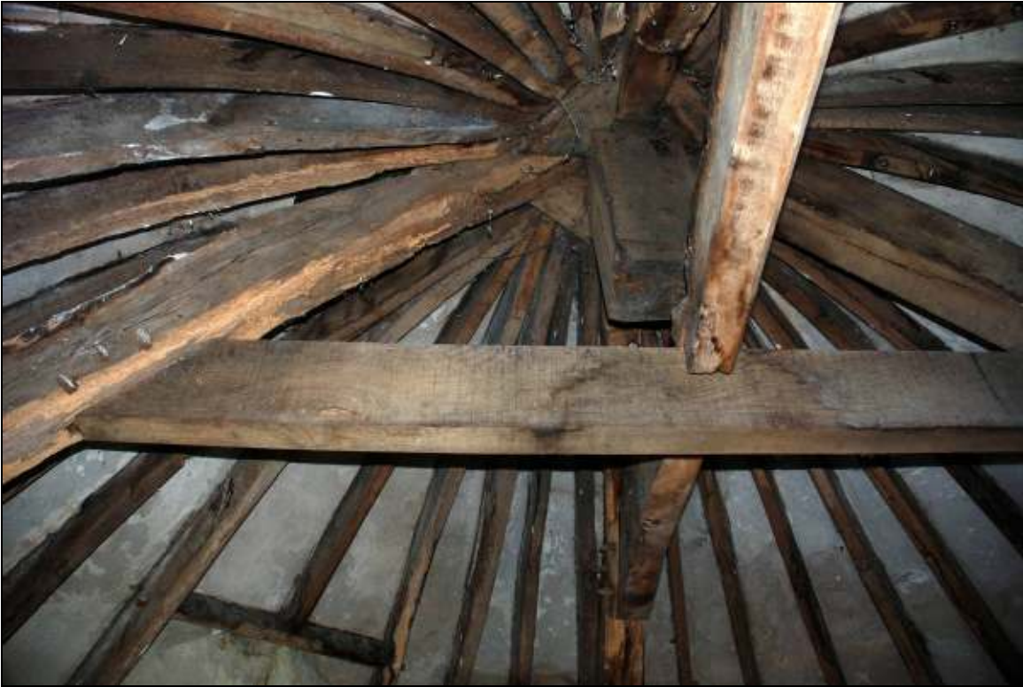
Plate 33: Tower roof structure
