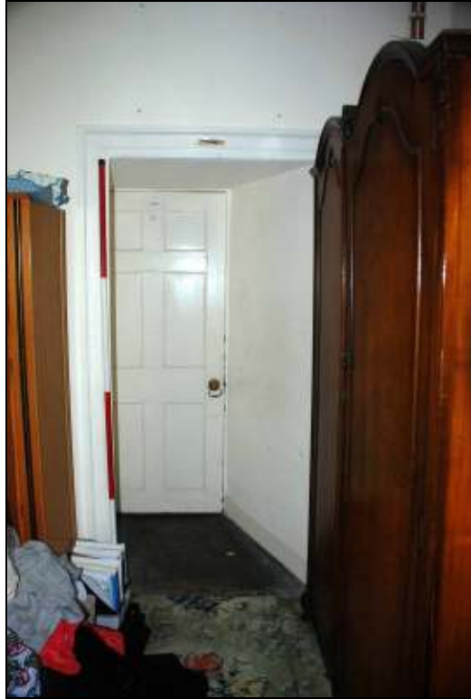
Plate 28: Angled passage between south wing and central range on first floor, looking NW
