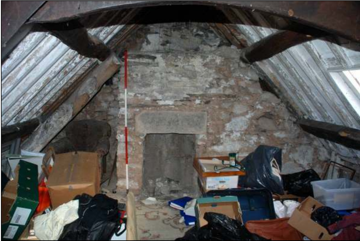
Plate 54: Truss 1, looking NE
