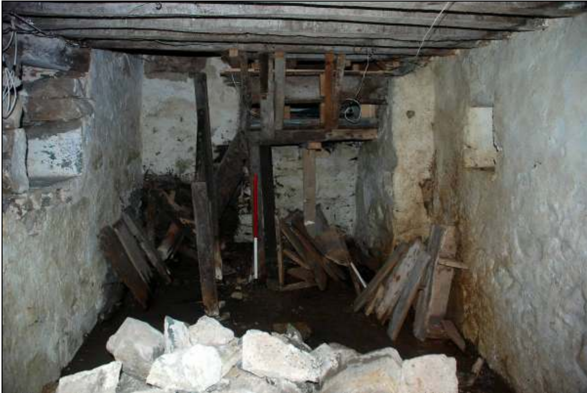
Plate 45: Remains of staircase in cellar, looking NE
