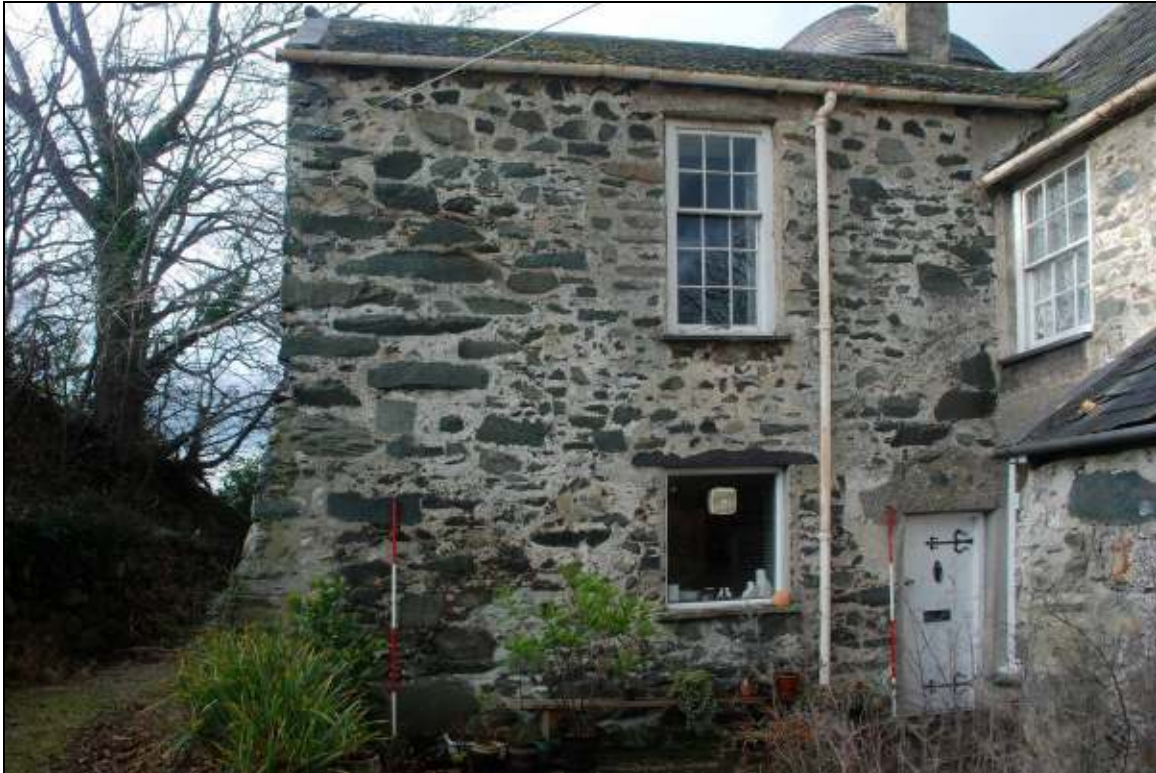
Plate 21: South wing looking SW
