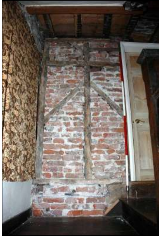
Plate 37: Brick and timber wall in staircase, between ground and first floors
