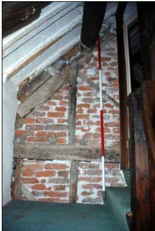
Plate 37: Brick and timber wall in staircase, between ground and first floors
