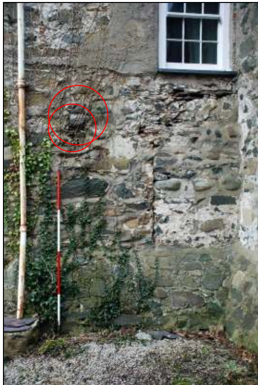
Plate 10: Possible blocked opening in SW corner of central range, looking NE
