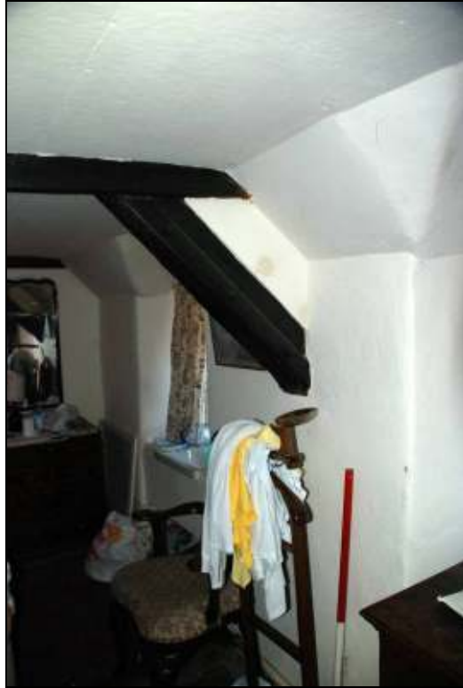
Plate 14: Base of Truss 3, looking north
