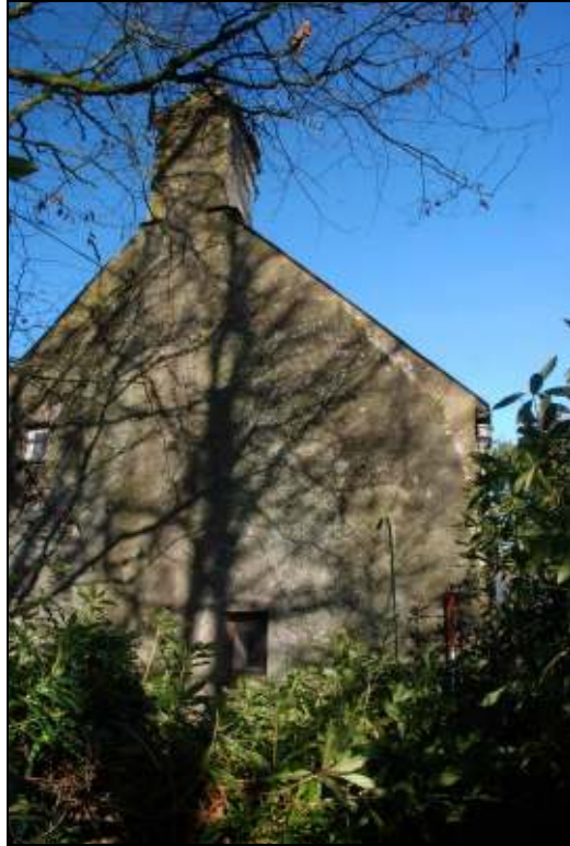
Plate 2: Gable end looking south
