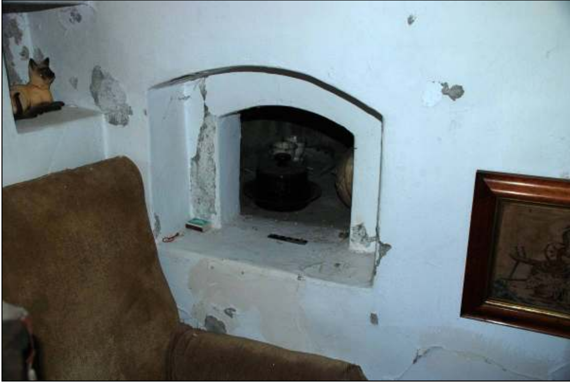
Plate 10: Bread oven, looking south west
