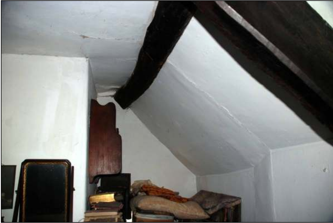
Plate 16: Lower rear purlin, looking south
