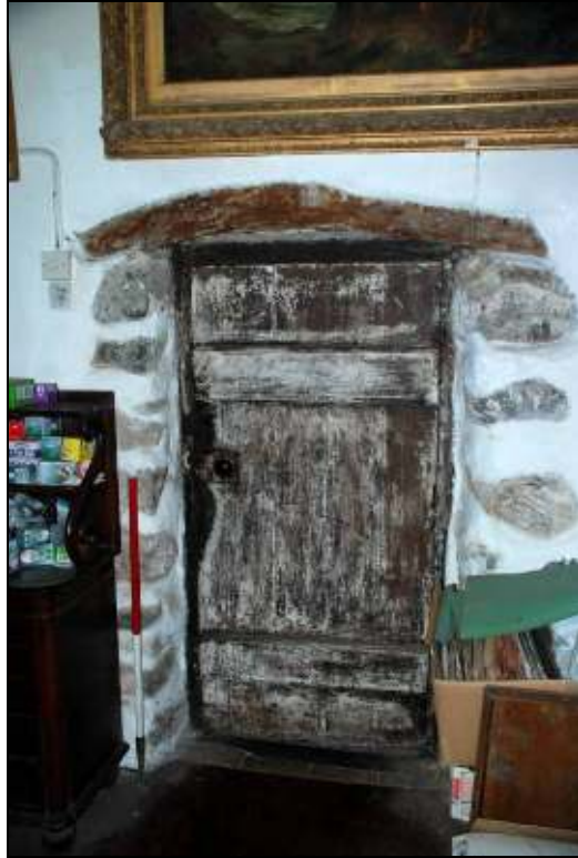
Plate 11: Western doorway, looking east
