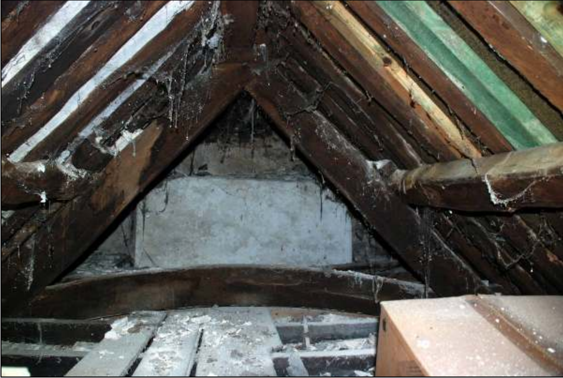
Plate 17: Truss 1, looking south
