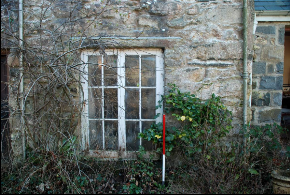
Plate 5: Southern ground floor window
