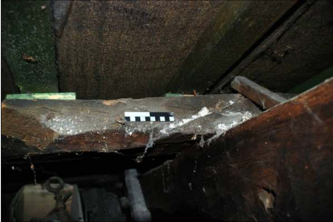
Plate 20: Splayed scarf joint on upper purlin, looking NW
