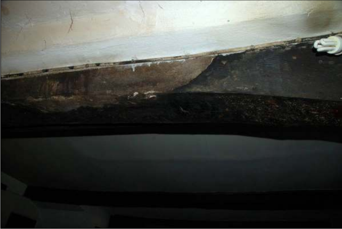
Plate 9: Cement repair to back of bressumer
