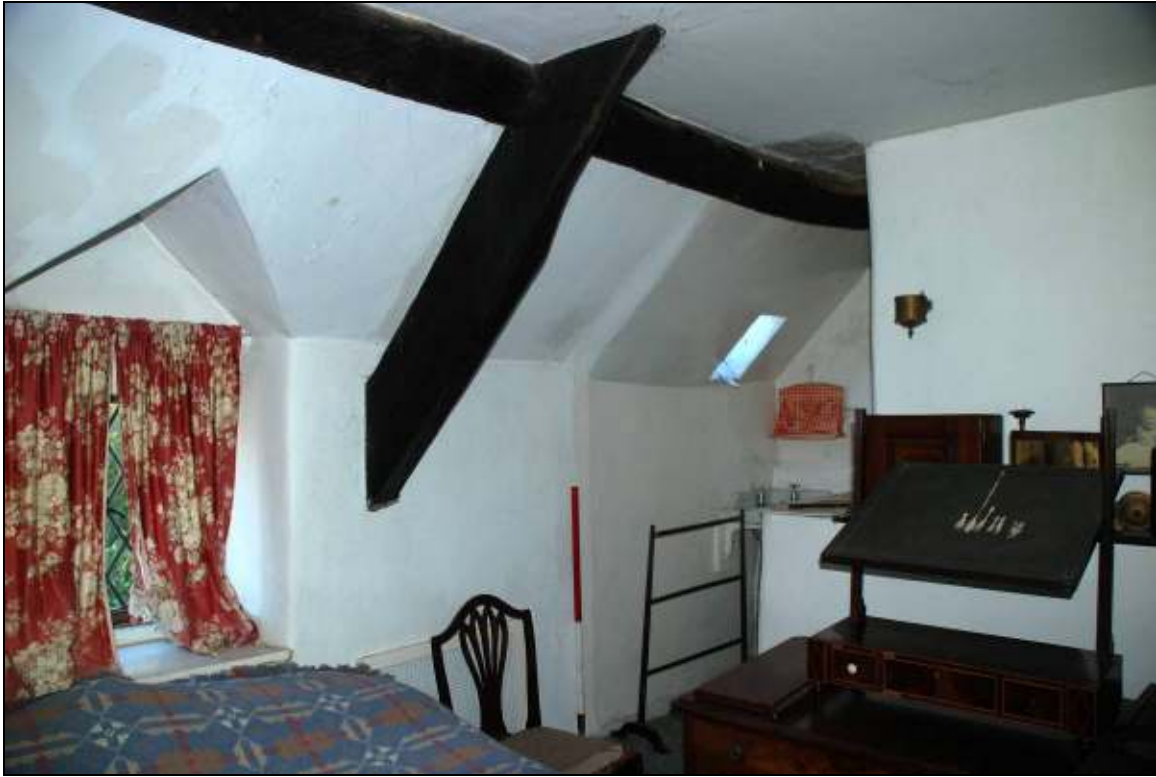
Plate 12: Base of Truss 1, looking SE
