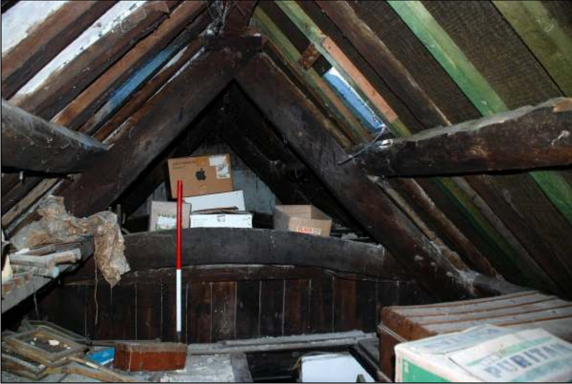
Plate 18: Truss 2, looking south
