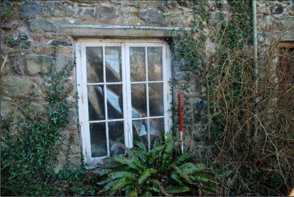
Plate 6: Northern ground floor window
