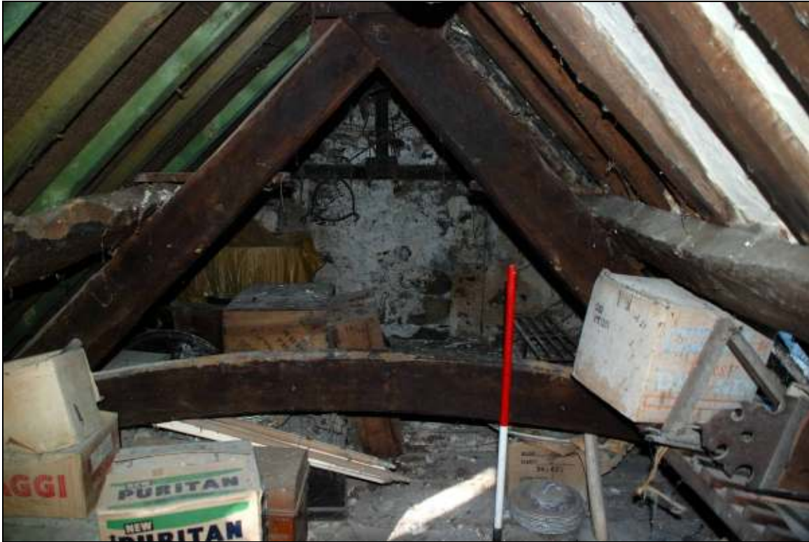
Plate 19: Truss 3, looking north
