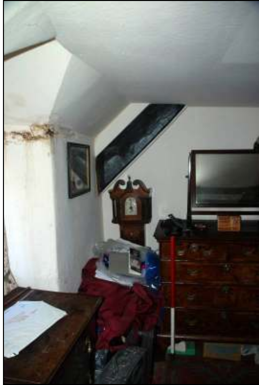
Plate 13: Base of Truss 2, looking south
