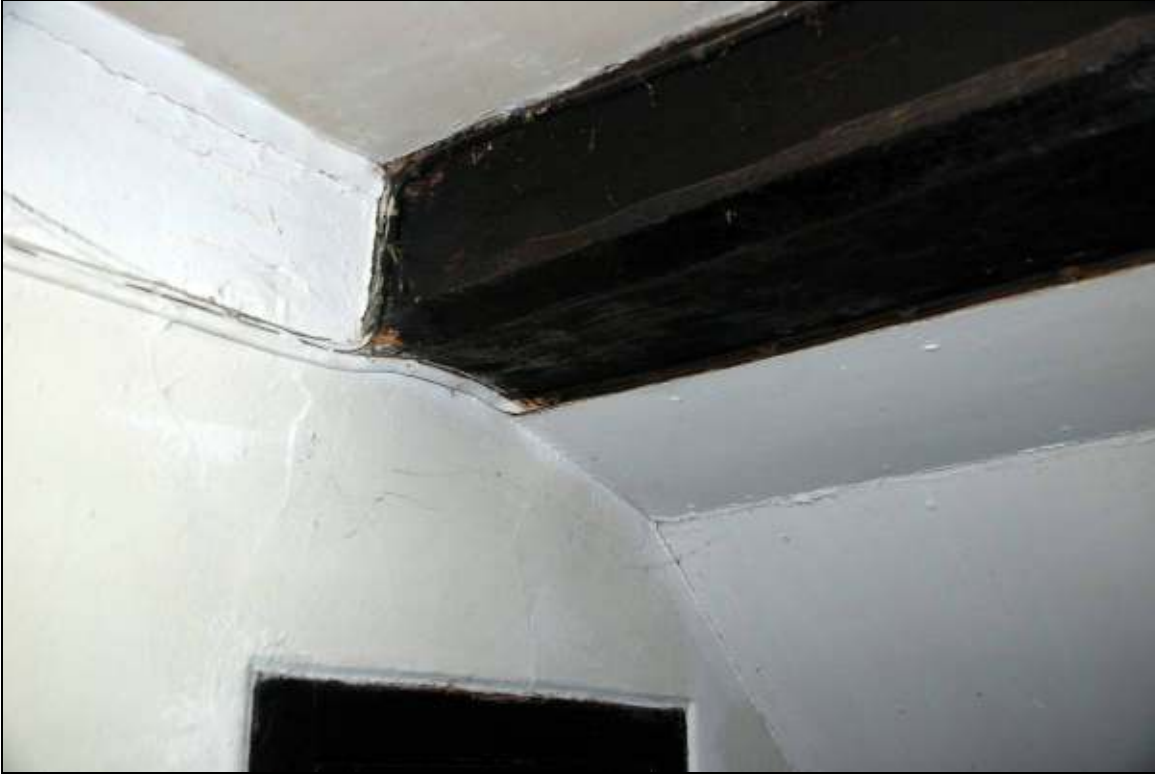
Plate 7: Tie beam, looking north west
