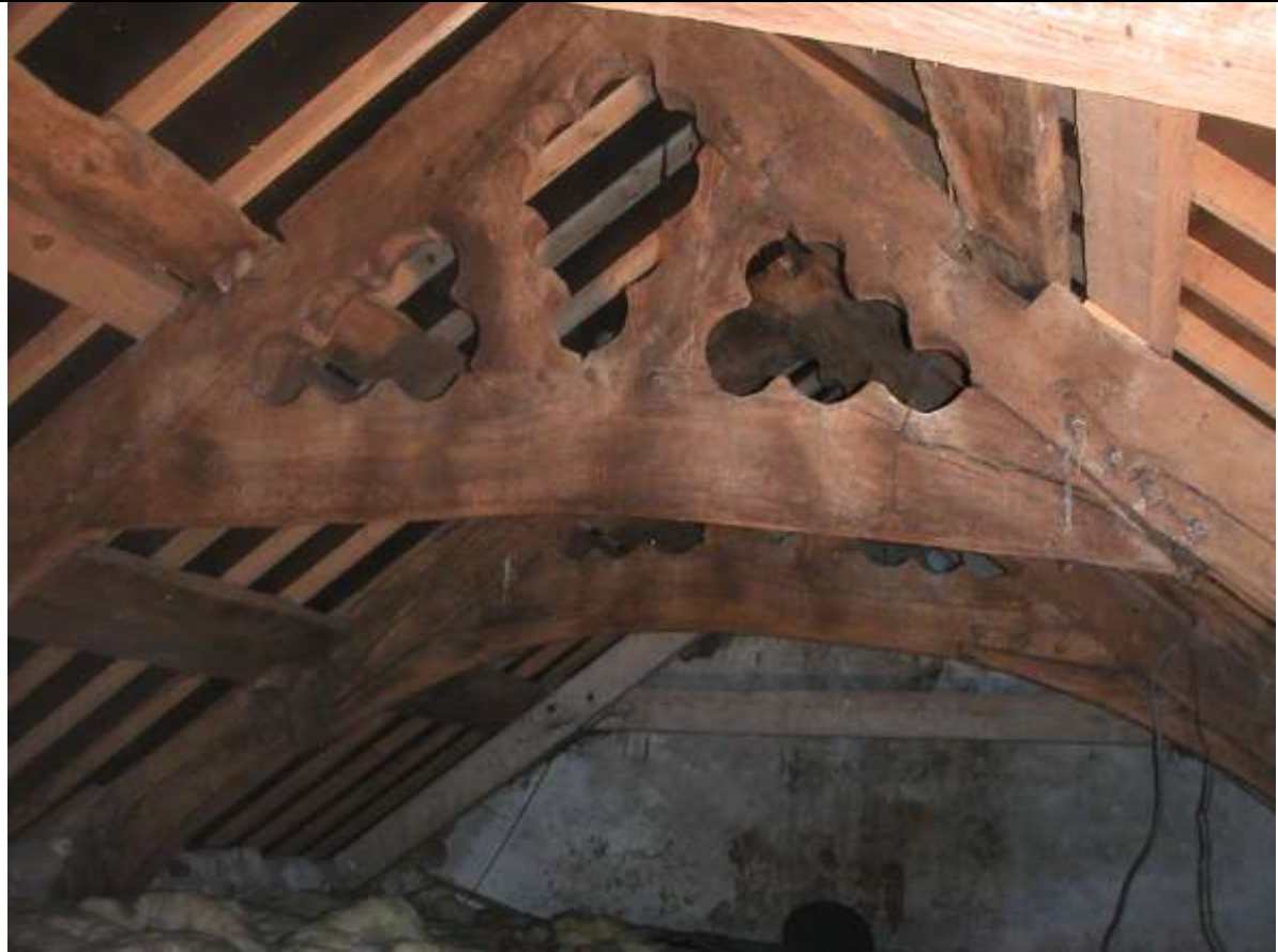
Plate 5 Trusses 2 & 3 (viewed from north - Truss 2 in foreground)
