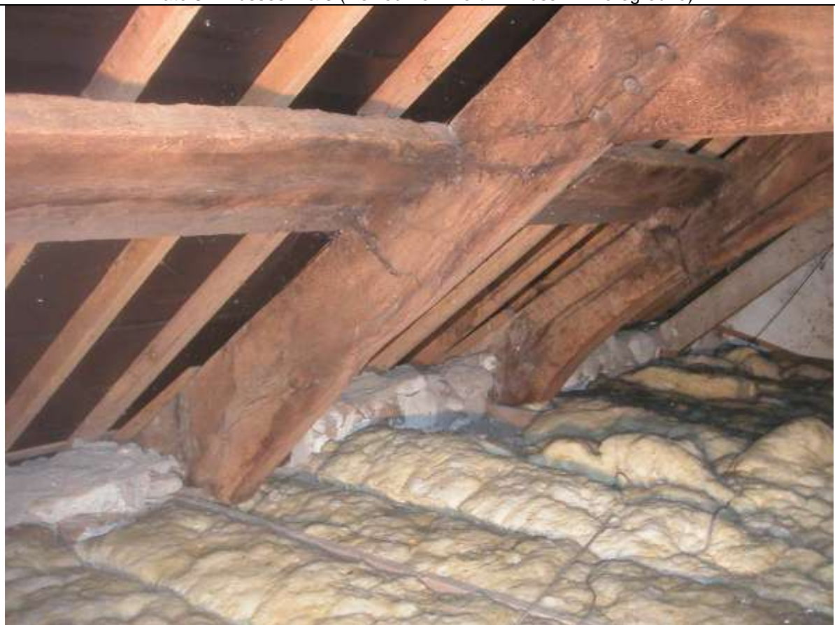
Plate 6 Trusses 2 & 3 (viewed from north - Truss 2 in foreground)
