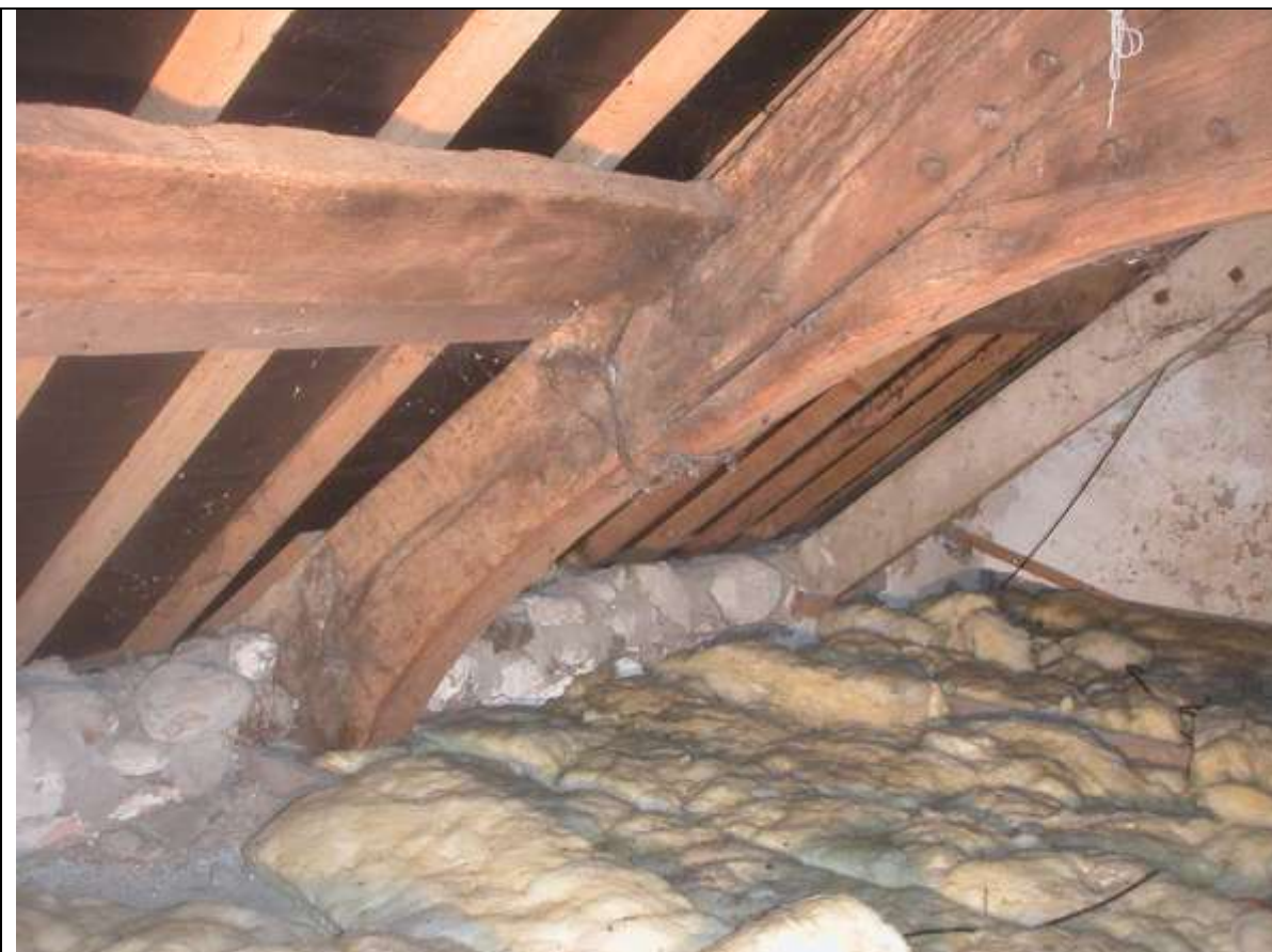
Plate 7 Truss 3 (viewed from north)
