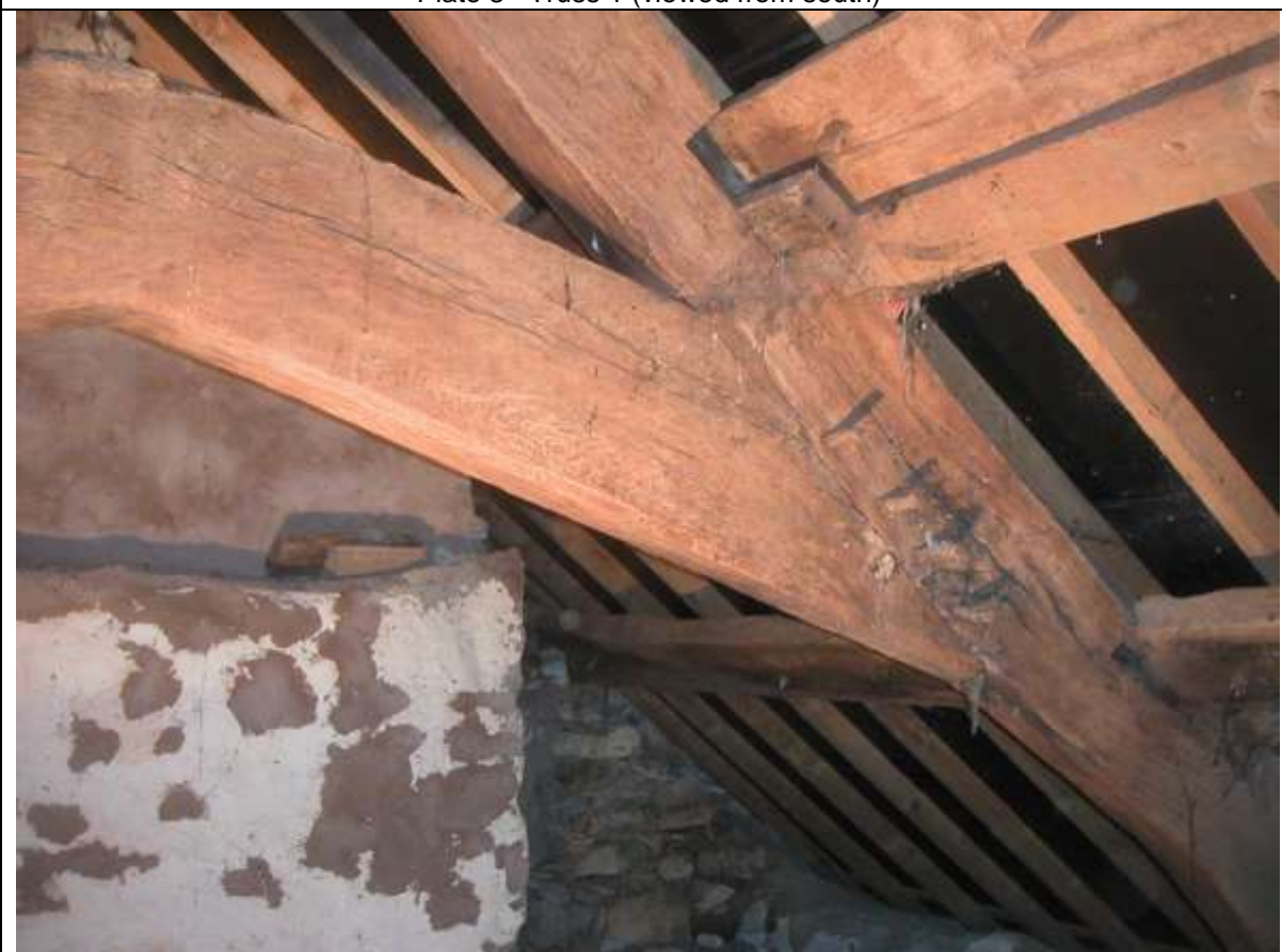
Plate 4 Truss 1 (viewed from south)
