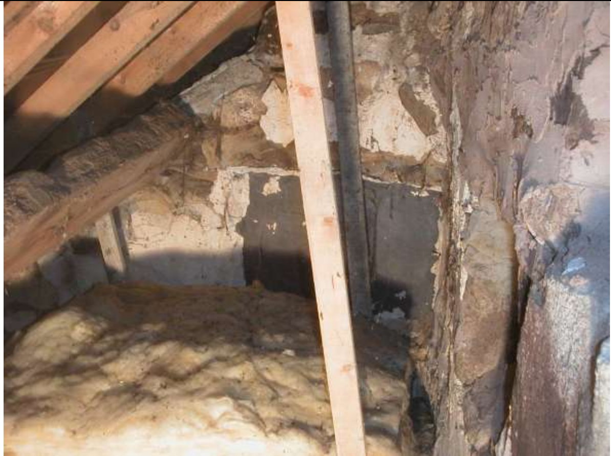
Plate 12 Possible blocked window in north gable
