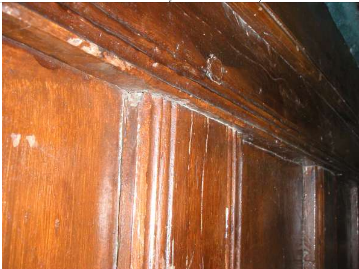
Plate 11 Partition (detail of post and head mouldings)
