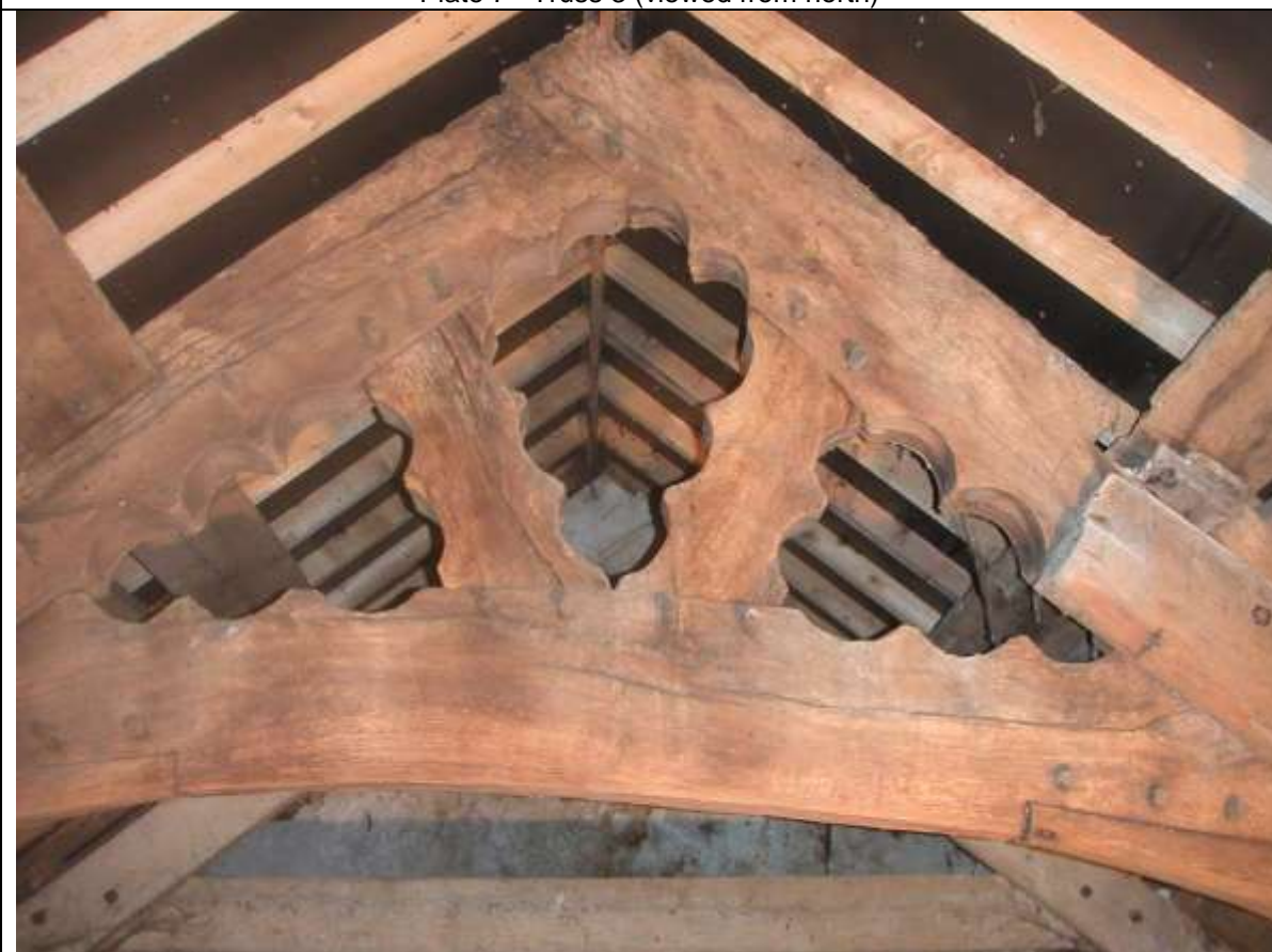
Plate 8 Truss 3 (viewed from north)
