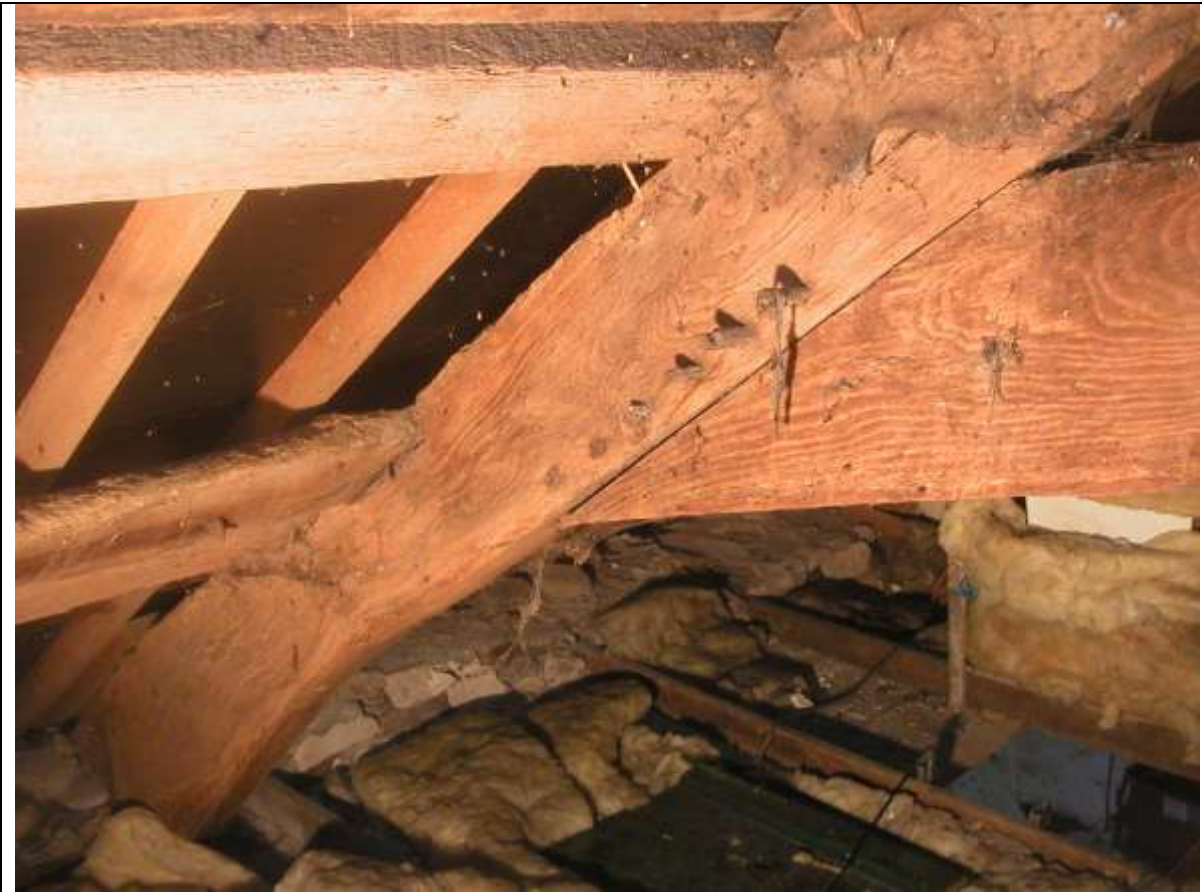
Plate 3 Truss 1 (viewed from south)
