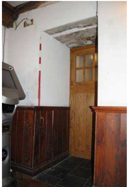
Plate 12: Primary opening (former window?), south-east angle ([GF01a]).
