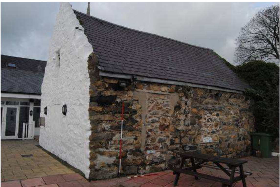
Plate 31: Outbuilding; south-west angle and south elevation.
