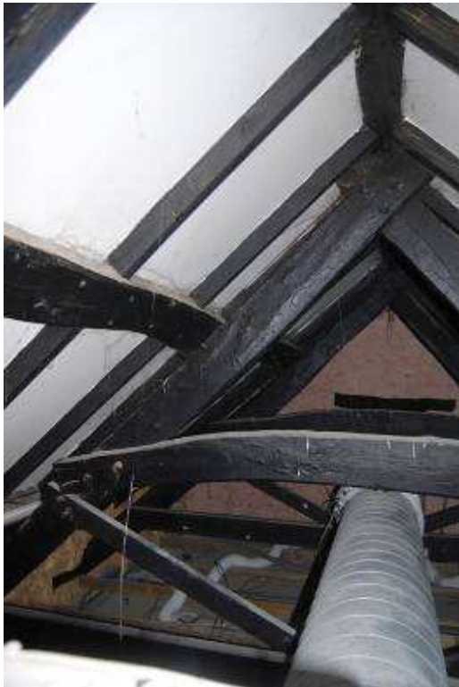
Plate 32: Outbuilding roof structure.
