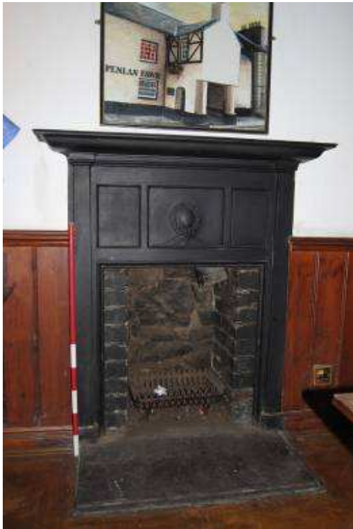
Plate 11: Inserted FP, east wall.
