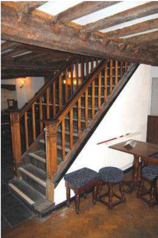
Plate 16: Inserted stair at Bay 2.
