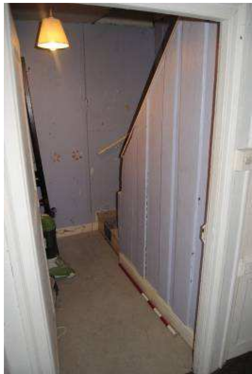
Plate 20: Stair to attic ([1F04]).
