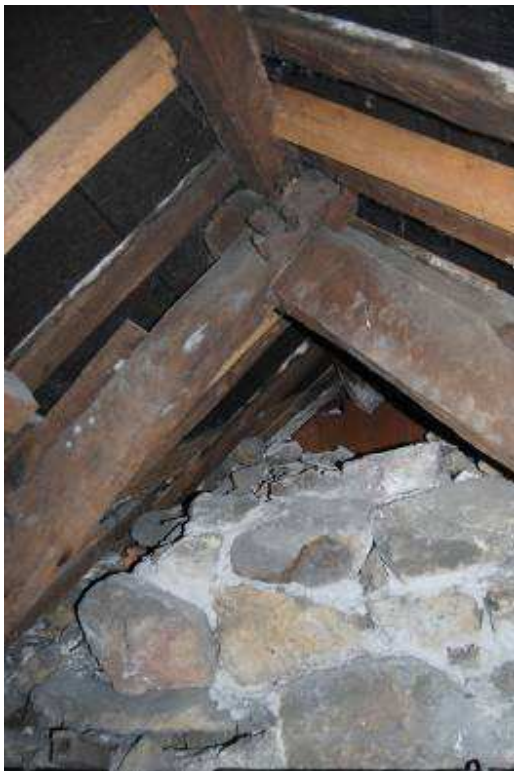
Plate 22: Roof structure over porch.
