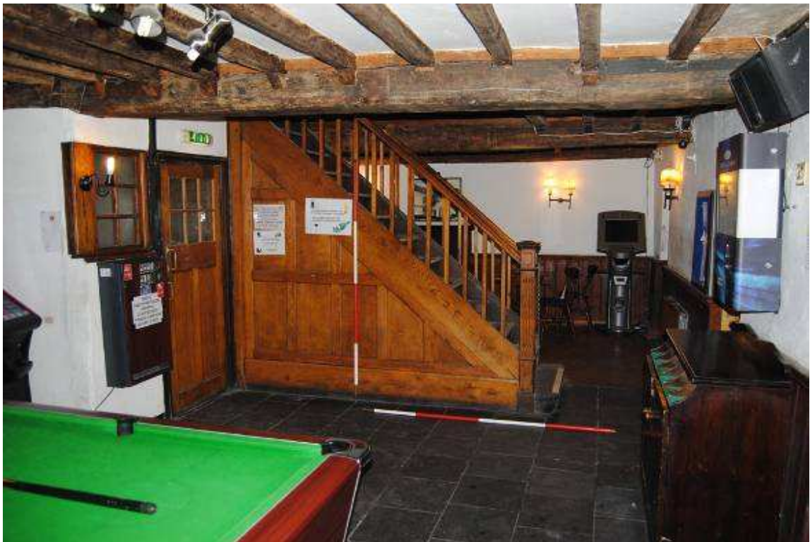
Plate 9: [GF01b] general view looking east.
