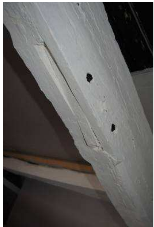
Plate 27: Truss T2; sawn off primary collar
