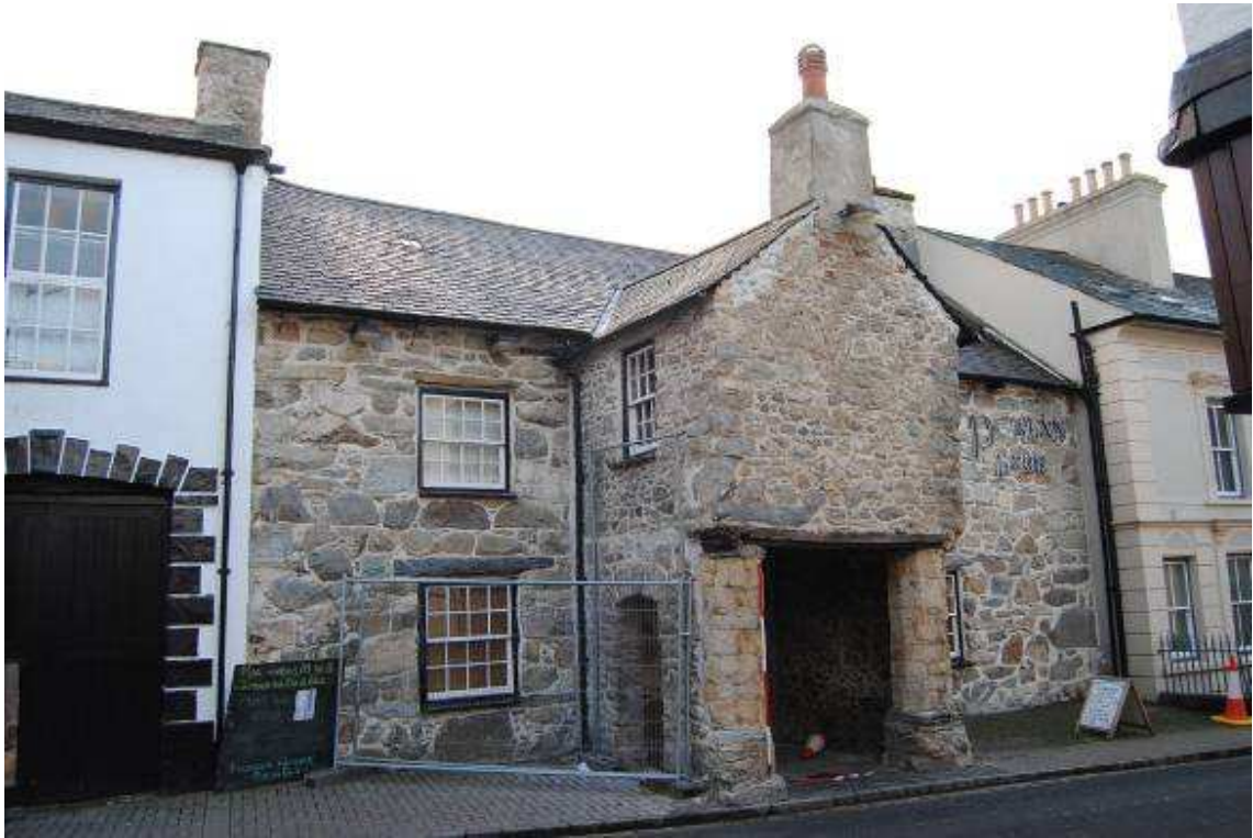
Plate 1: North (street) elevation looking south-west.
