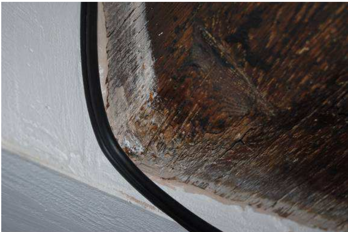
Plate 15: Ogee chamfer-stop of ceiling beam at Bay 2/3 (S); [GF01].
