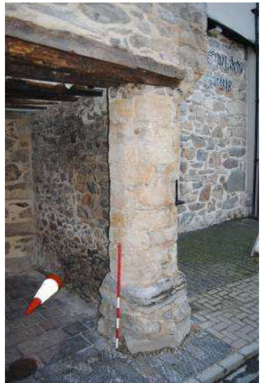
Plate 4: Western pillar of secondary porch.
