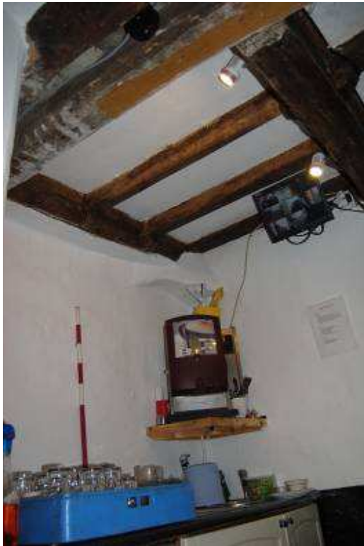
Plate 14: Site of primary stair to south of FP.
