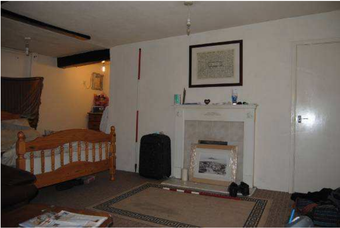
Plate 18: [1F01], looking south-west; note recess to south (left) of stack for ?primary stair.
