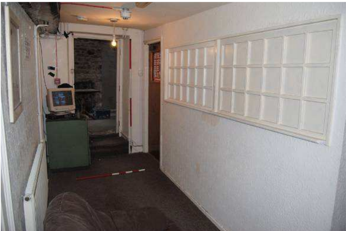
Plate 17: First floor landing [1F02], looking north towards porch.
