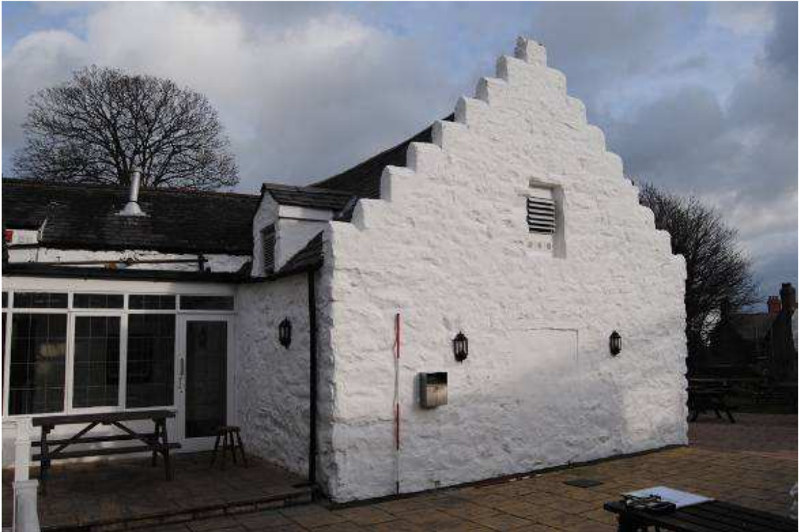
Plate 30: Outbuilding; western stepped-gable end, note dormer to north elevation.
