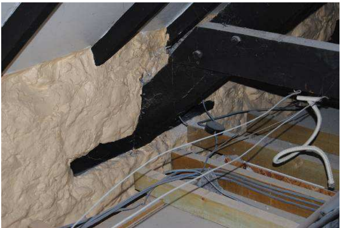
Plate 34: Outbuilding; principal rafter resting on timber pad set into stonework.
