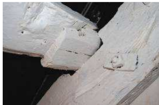
Plate 29: Detail of purlin scarf
