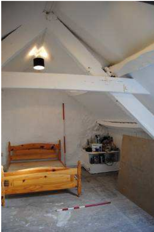
Plate 26: [2F02], truss T1.
