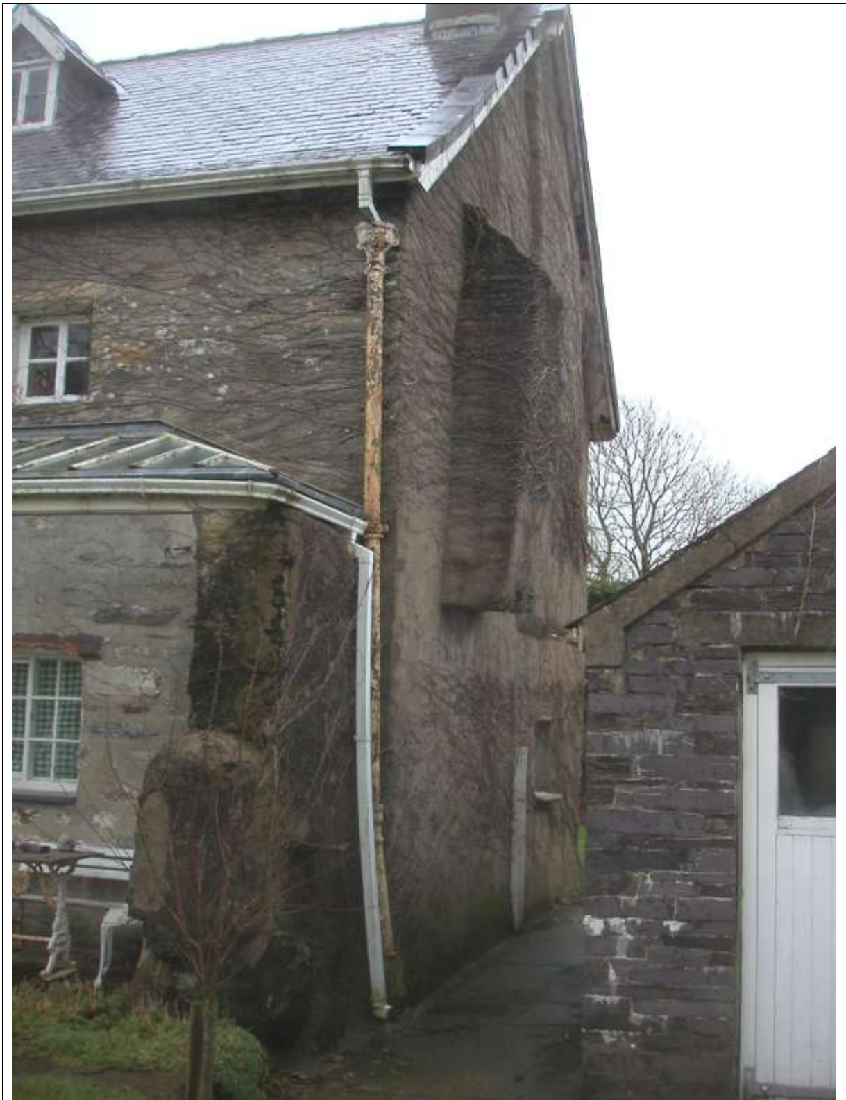
Plate 6 south gable, with projecting garderobe (?)
