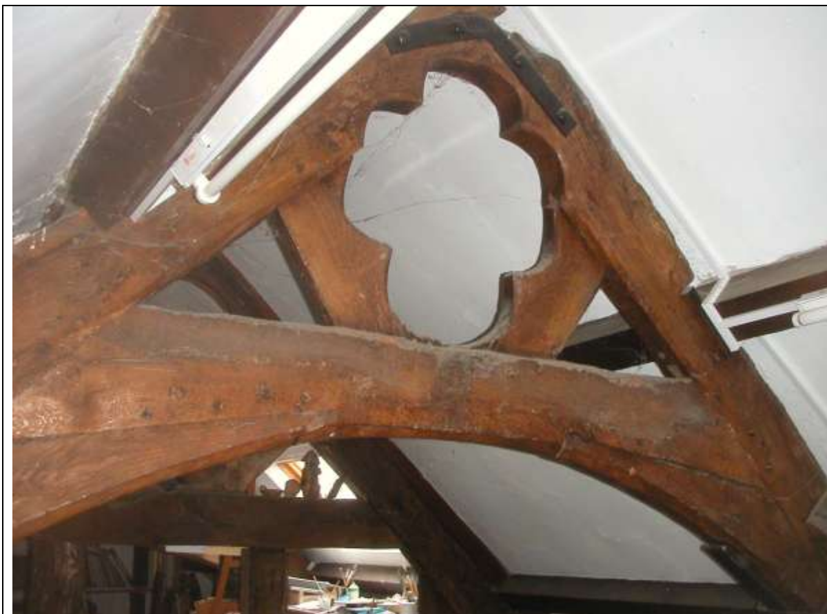
Plate 1 Truss 3, from south
