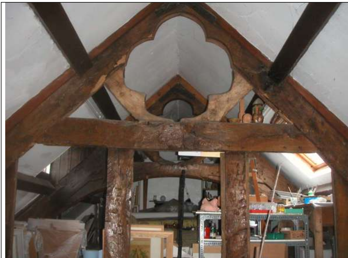
Plate 3 Truss 2, from south (truss 1 beyond)
