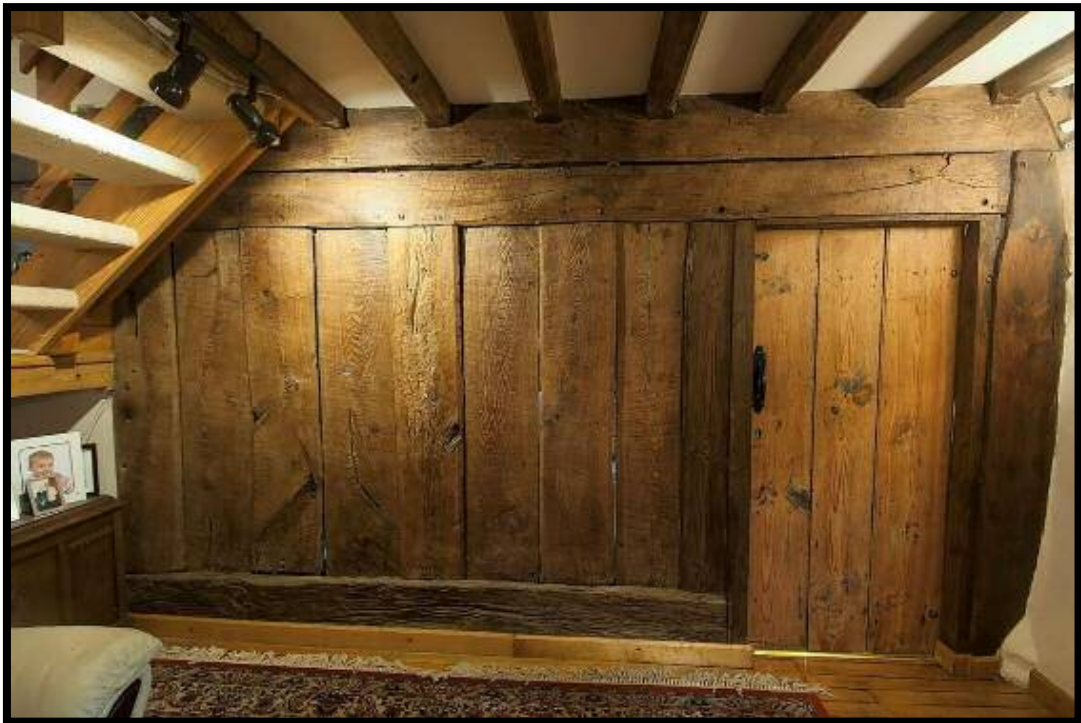
Figure 9: Plank and muntin screen at high end.
