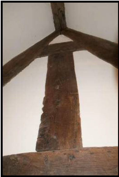
Figure 17: Truss 2. King strut sitting on collar.
