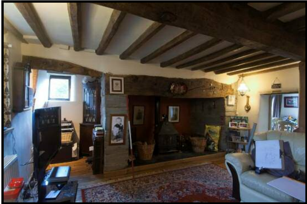
Figure 6: Former hall with inserted floor and fireplace.
