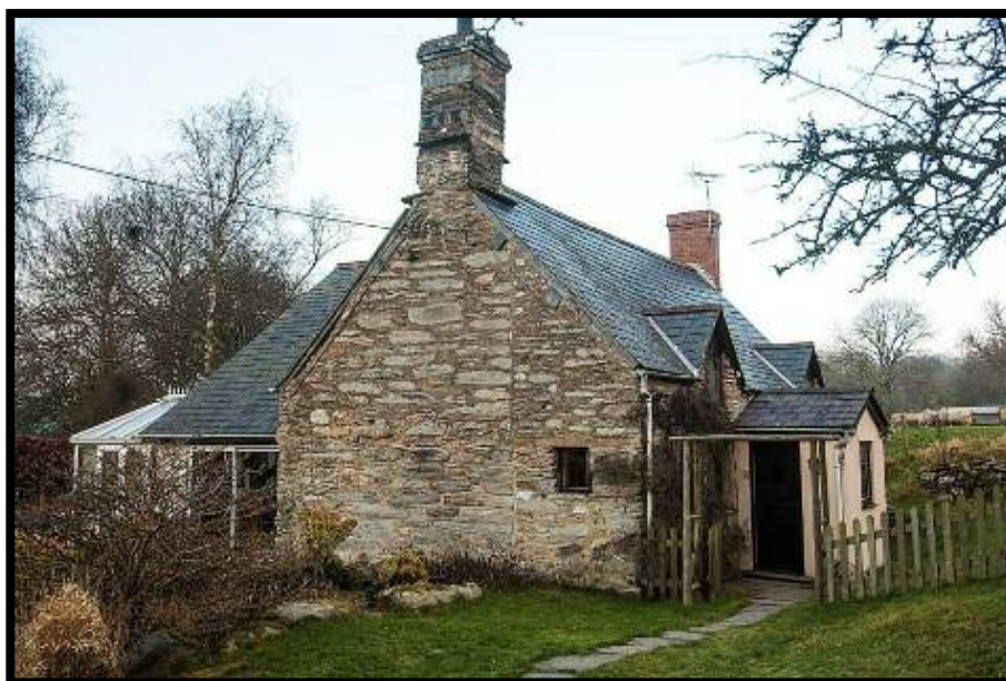
Figure 5: Llanerch from SW showing gable and vertical masonry joint.
