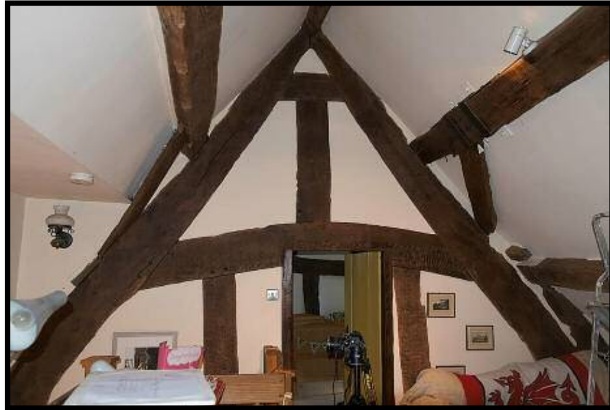
Figure 16: Truss 2, the central former closed partition. Note wind braces.
