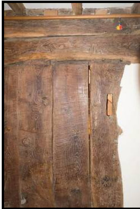
Figure 12: Inner room side of plank & muntin screen. Top of right hand post rebated for door head. Mortise for fixing bench to screen.
