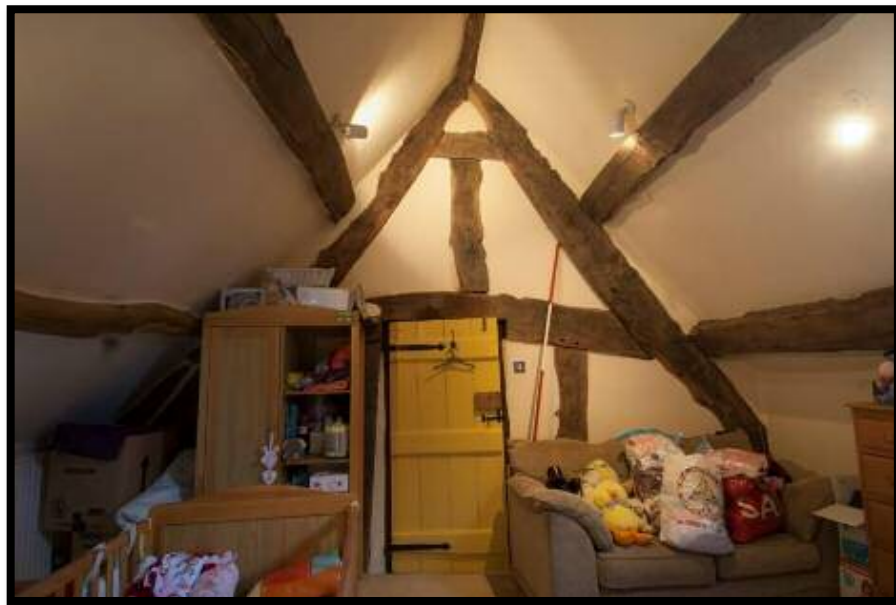
Figure 24: Reverse side of Truss 2 from FF2 upper inner room.
