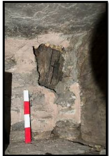
Figure 7: Right cruck blade with mortise and remnant of tie beam also mortised for partition.
