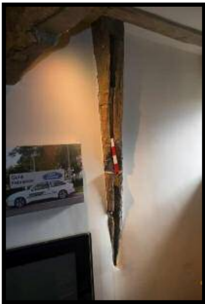
Figure 8: Left cruck blade of T1 with mortise and groove.
