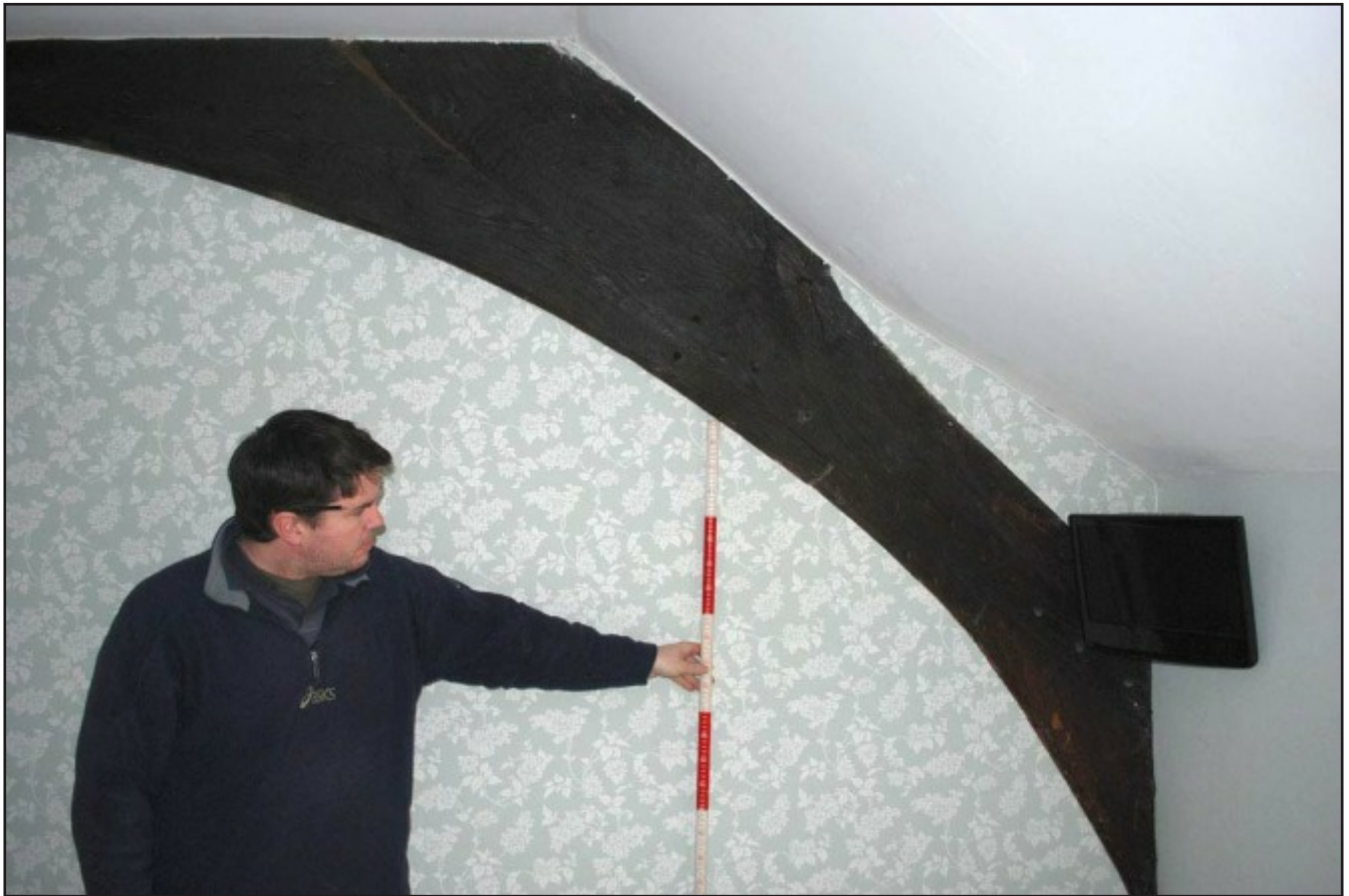
Plate 3: The eastern side of the southern face of the southern cruck which divides the hall; view from the south.
