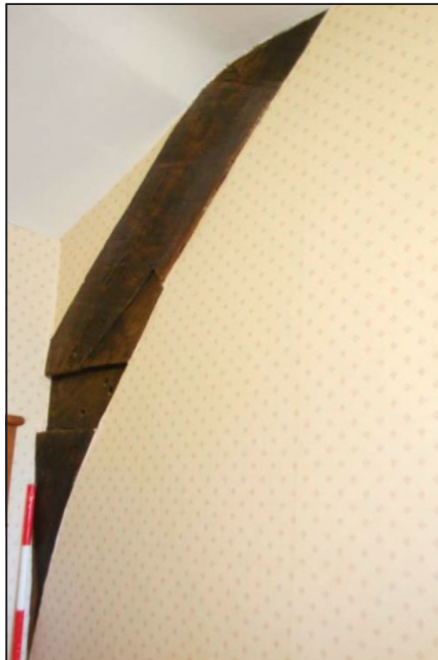
Plate 10: The eastern side of the southern face of the northern cruck which forms the southside of the screens passage
