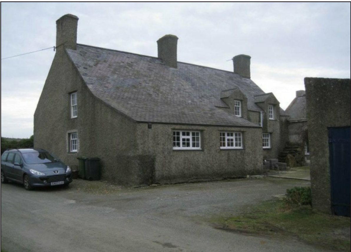
Plate 02: The western elevation of Trefadog; view from the northwest.
