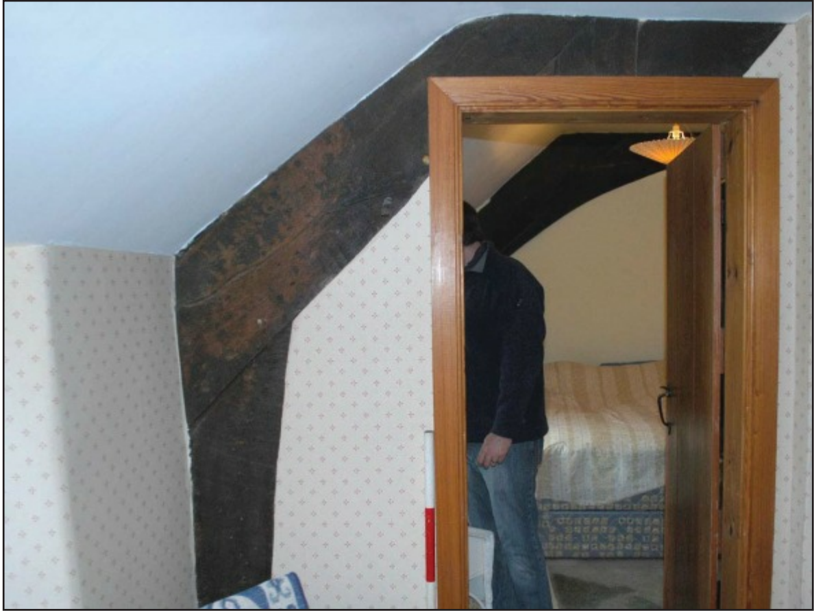
Plate 9: The eastern side of the northern face of the central cruck which forms the southside of the screens passage; view from the north.
