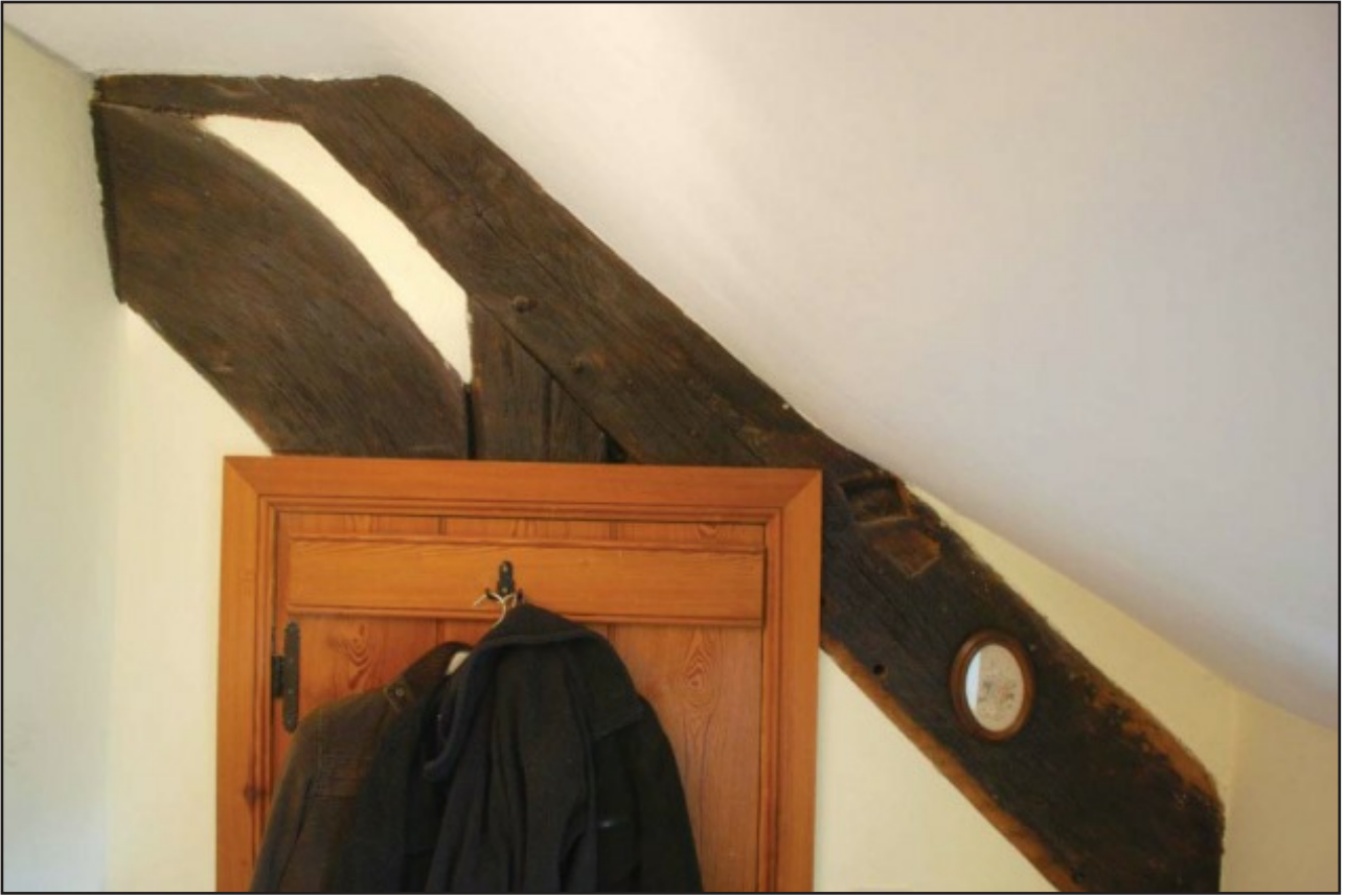
Plate 7: The eastern side of the southern face of the central cruck which forms the south side of the screens passage; view from the south.
