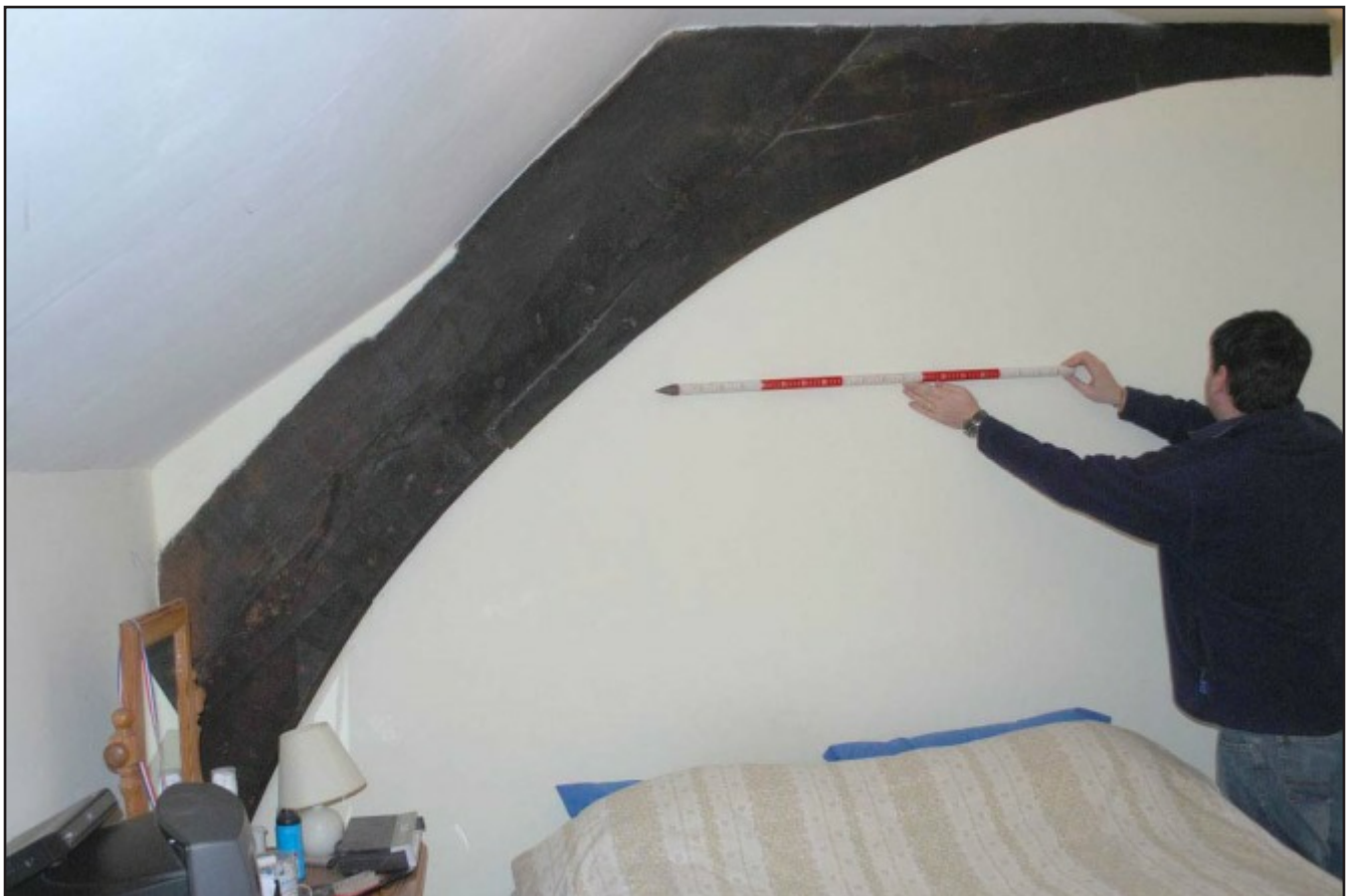
Plate 6: The eastern side of the northern face of the southern cruck which divides the hall; view from the north.
