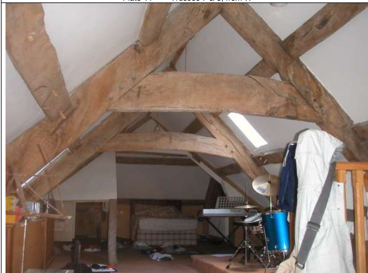
Plate 12 Trusses 10 & 11, from W
