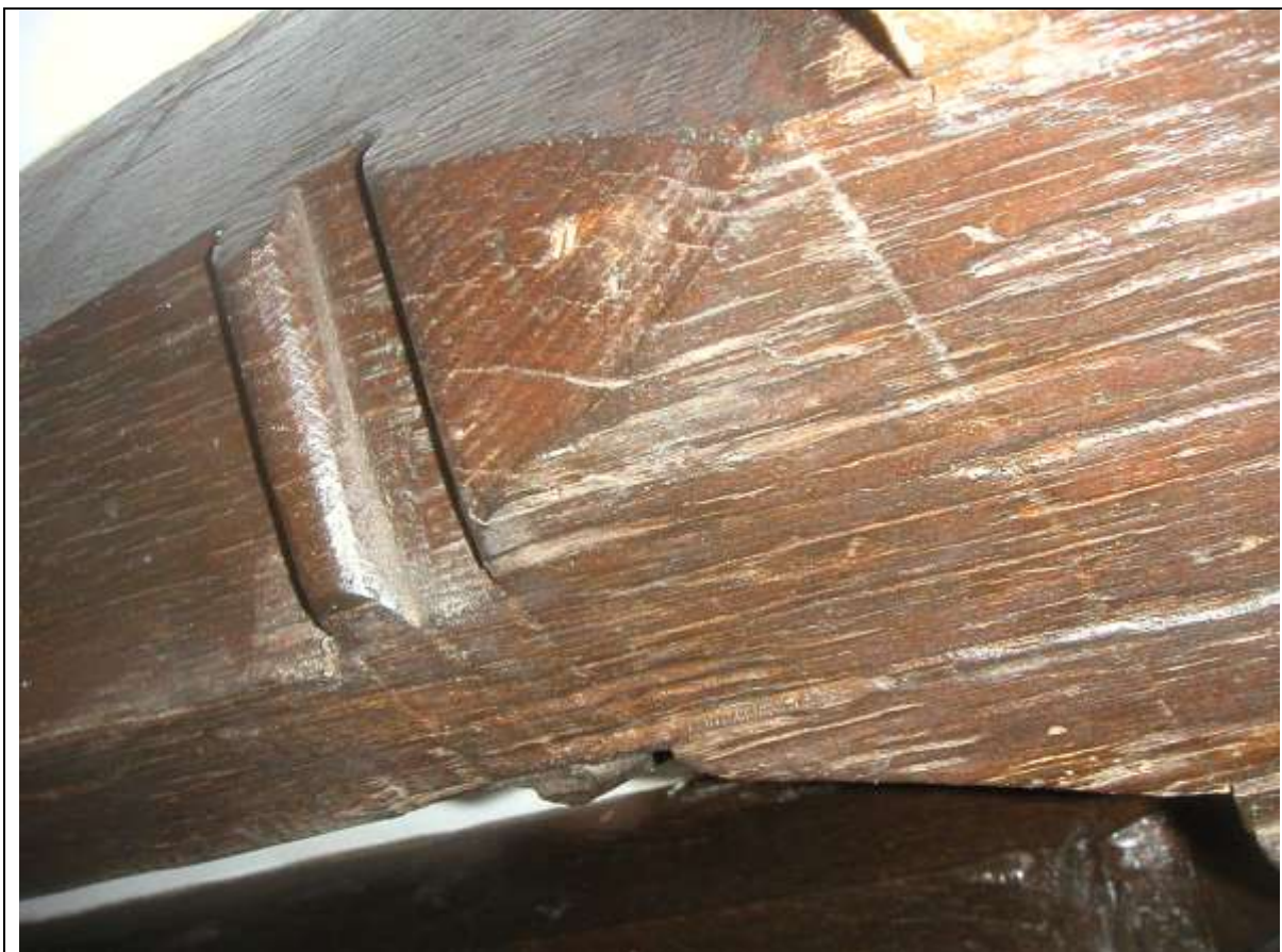
Plate 5 Detail of stop on tertiary beam
