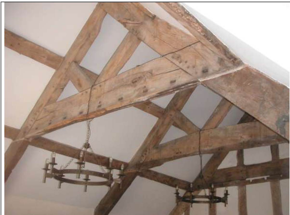
Plate 7 Truss 1 in foreground (from E)
