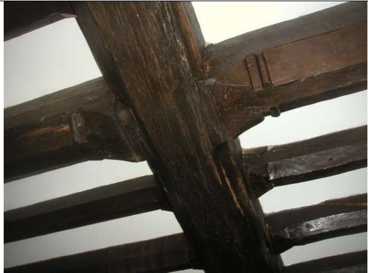
Plate 3 Ceiling to main hall (secondary and tertiary beams)
