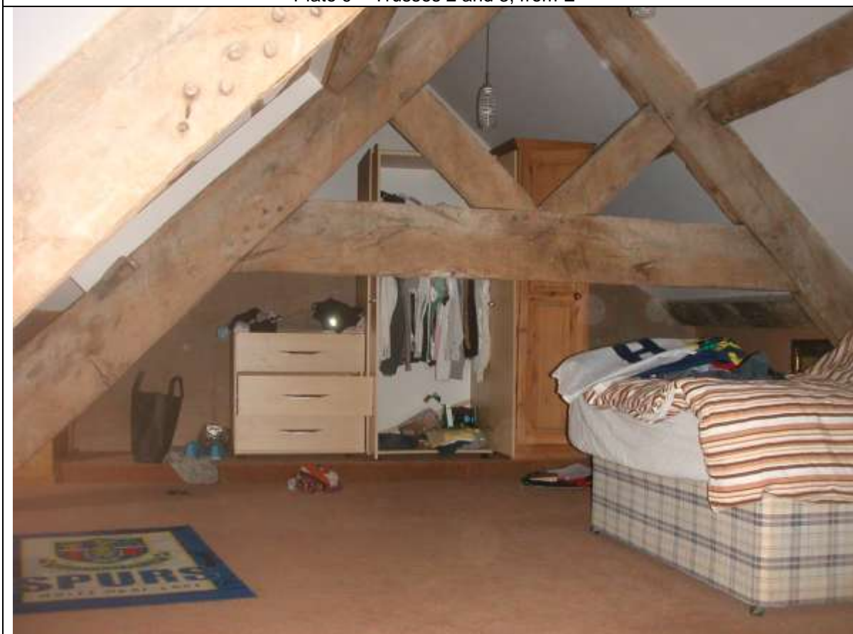
Plate 10 Truss 5 (attic in rear part of house)
