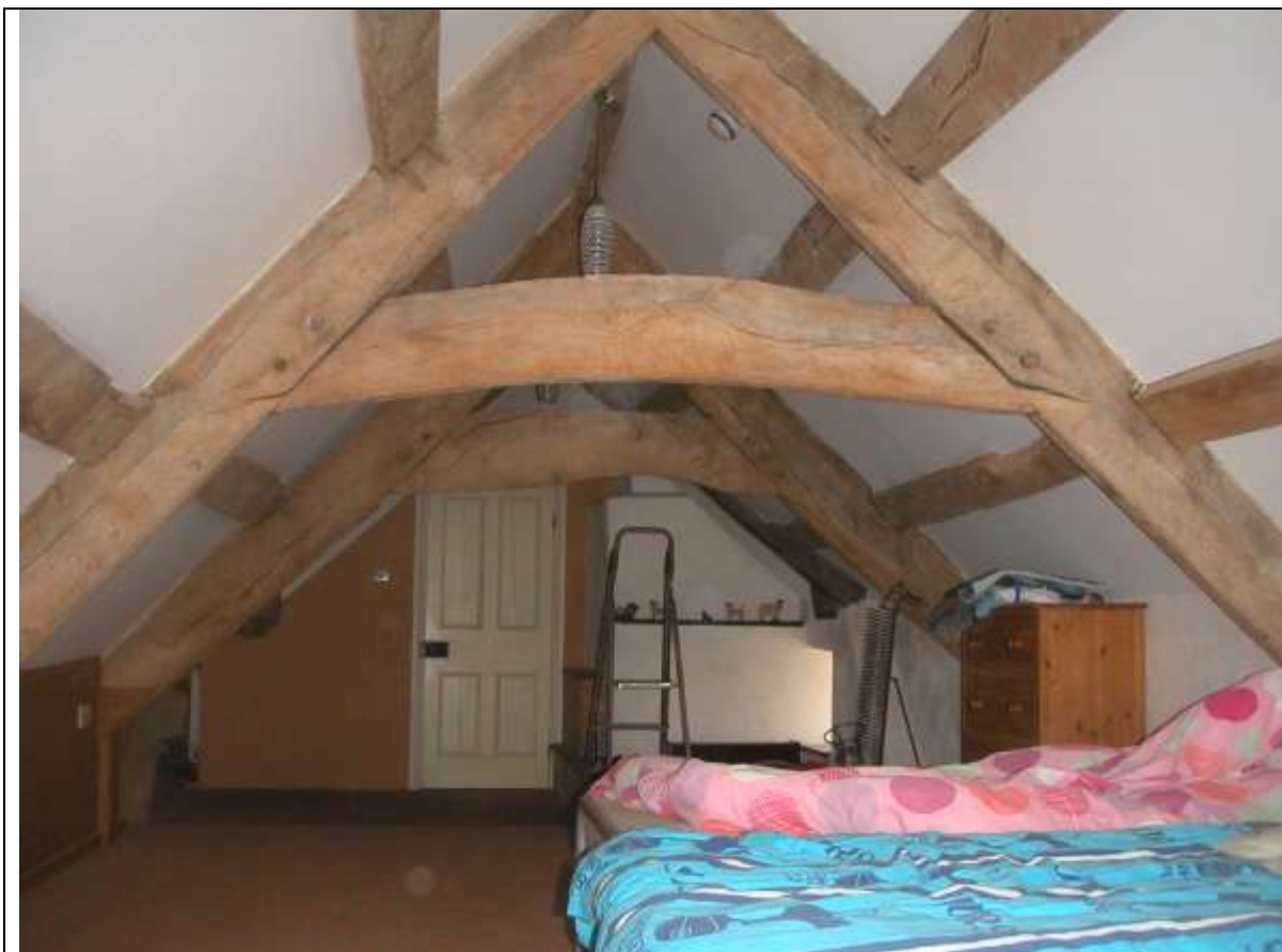
Plate 11 Trusses 7 & 8, from W
