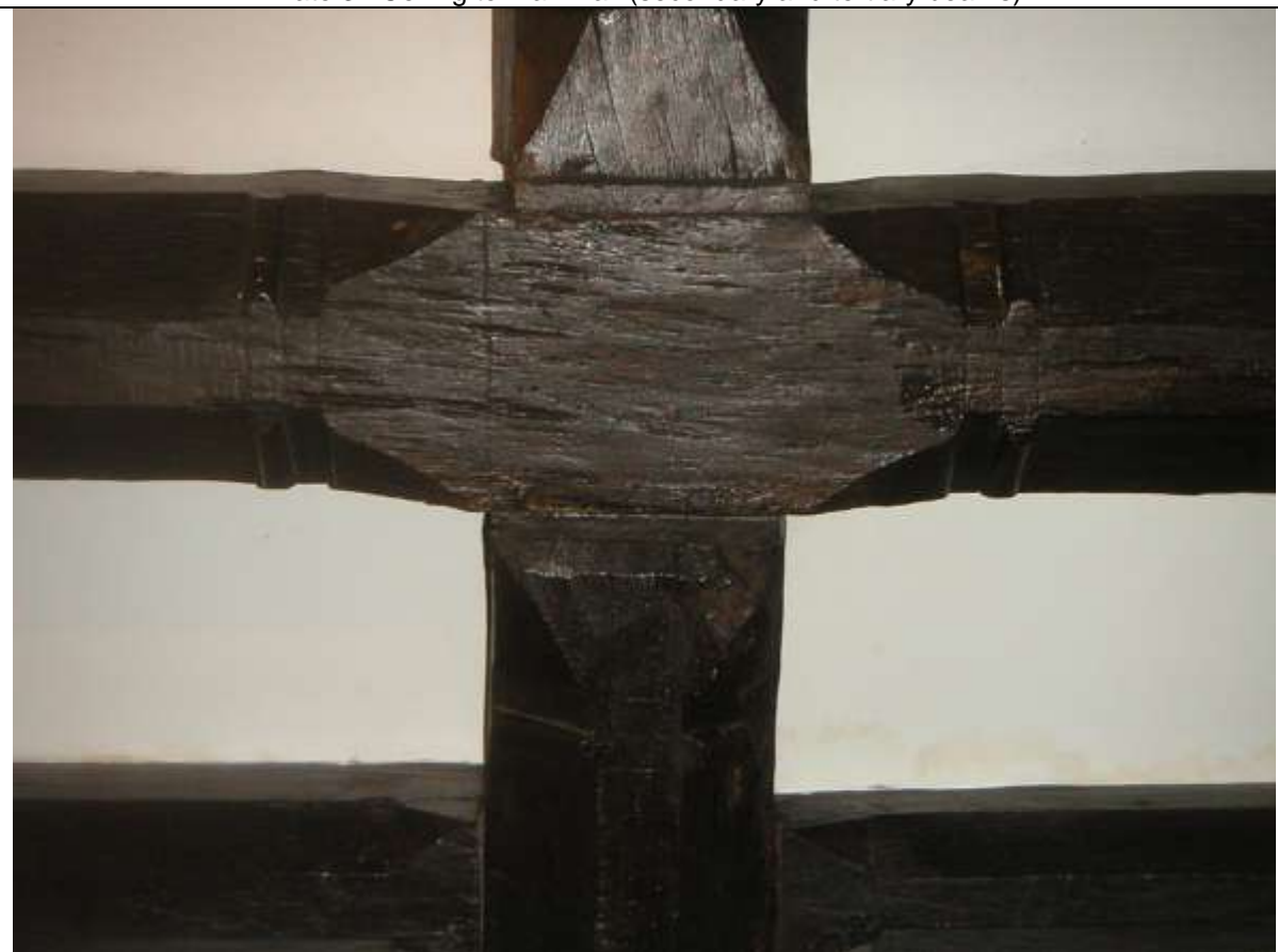
Plate 4 Ceiling to main hall (tertiary beams)
