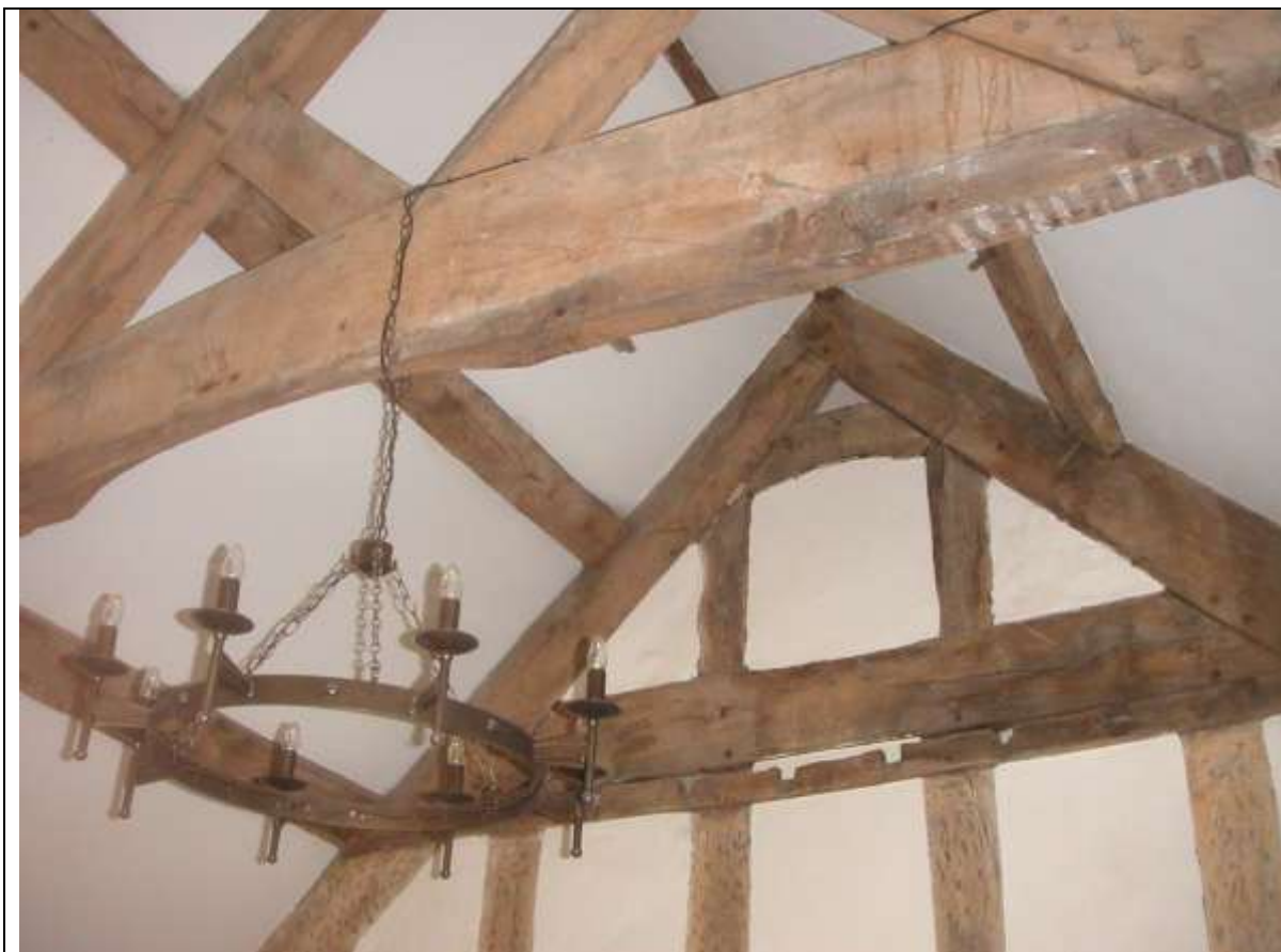
Plate 9 Trusses 2 and 3, from E
