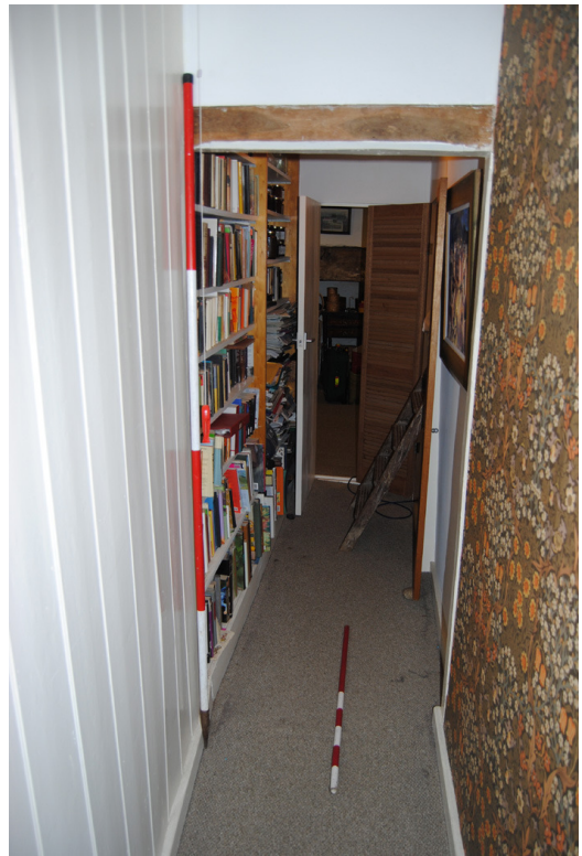
Plate 25: Central passage [1F01] including primary doorframe beneath T2.
