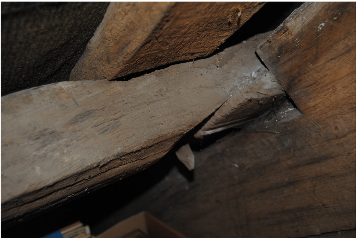
Plate 38: Detail of splayed scarf at T2 (W).
