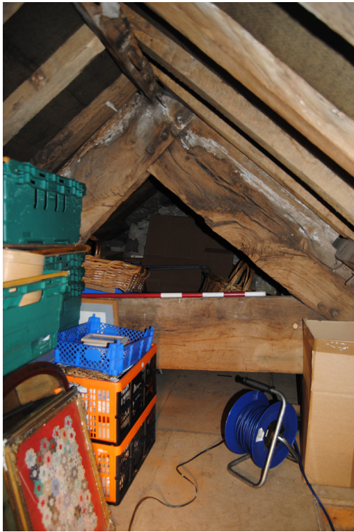
Plate 33: Apex of truss T1 looking south.
