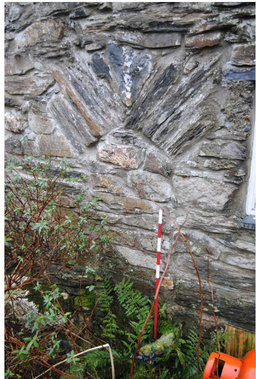
Plate 7: Blocked primary door to west elevation.
