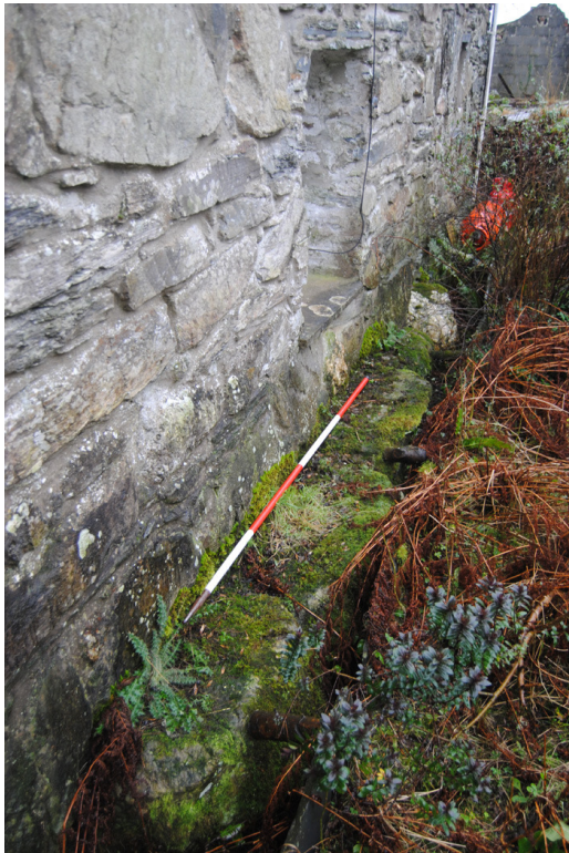
Plate 6: Offset boulder footing to west elevation.
