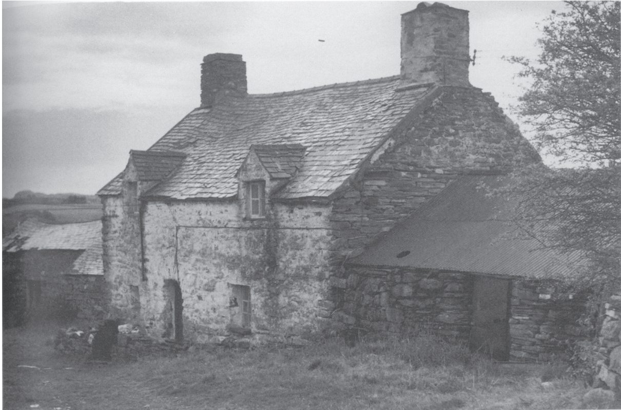
(a) Photograph from north-east, from Peter Smith's Houses of the Welsh Countryside 2nd Edition (1988), plate 39.
