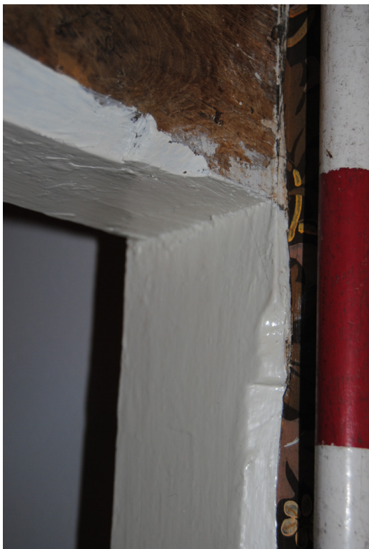
Plate 26: Ogee-stopped door jamb and head below T2.
