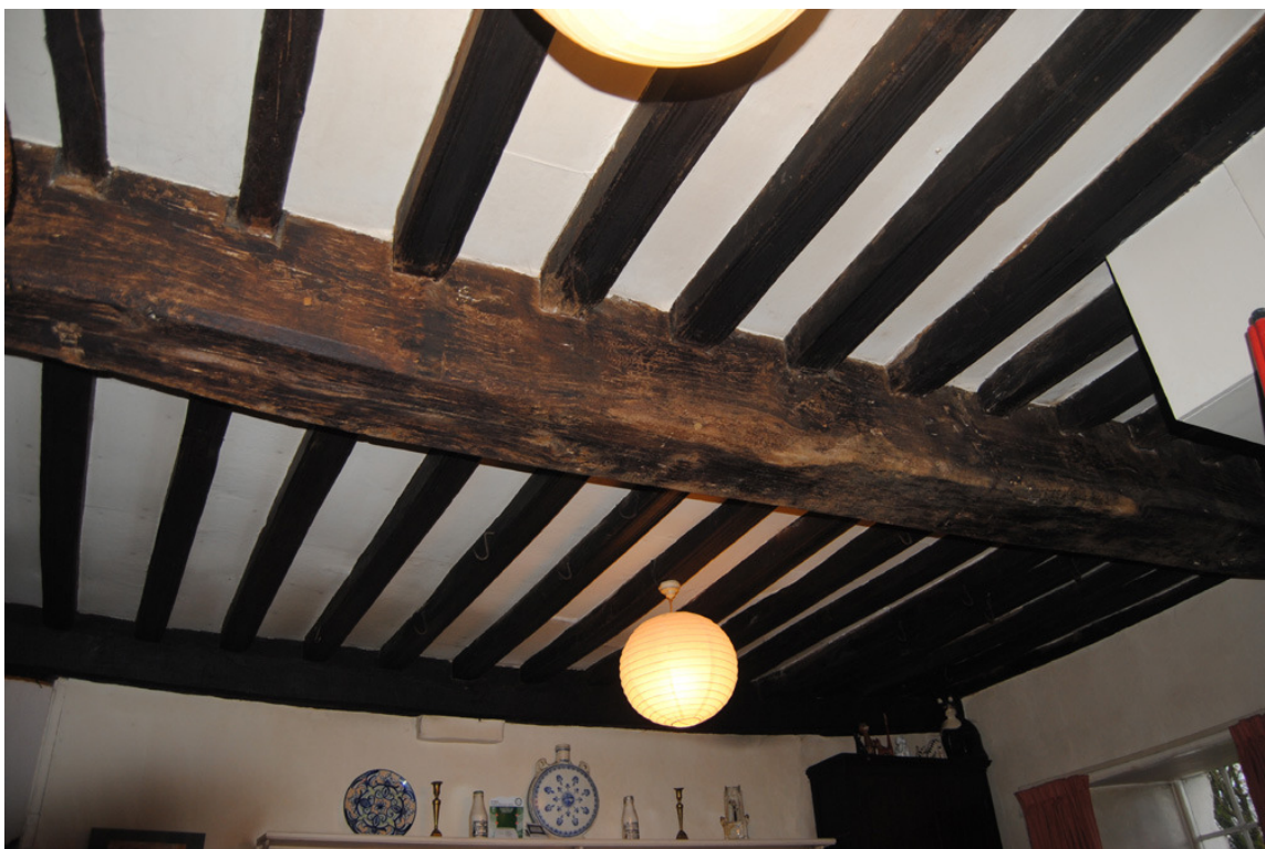
Plate 17: Ceiling structure over [GF02].
