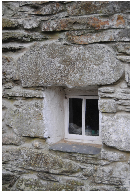
Plate 4: Primary window with monolithic head.
