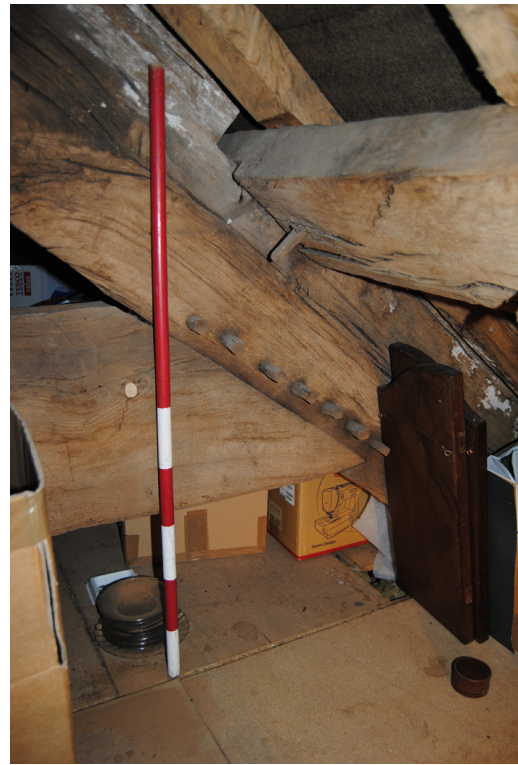
Plate 34: Truss T1, multi-pegged collar joint.
