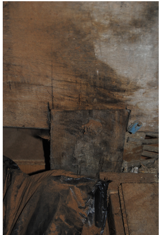
Plate 37: Truss T2, halved and lapped stud.
