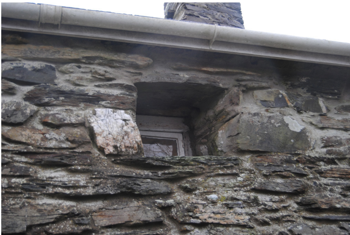
Plate 8: Primary window to west elevation, first floor (south).
