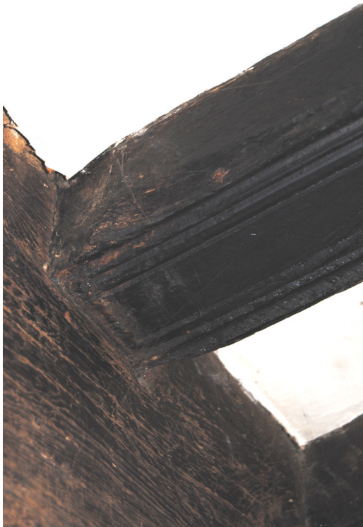
Plate 18: Detail of moulded common joist, [GF02].
