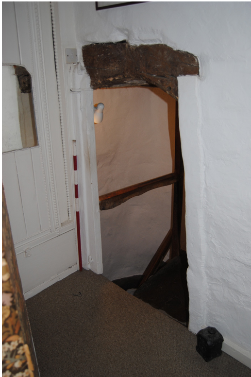
Plate 24: Head of winder stair.
