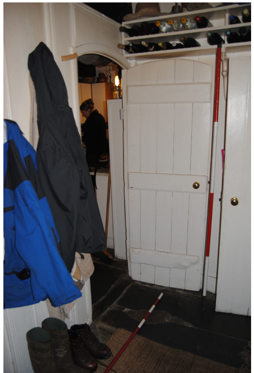
Plate 12: [GF01]; primary door with raised head (see also Plates 22-3).
