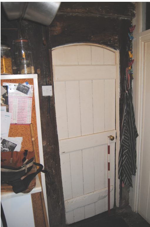
Plate 22: Door to [GF03] with raised head.
