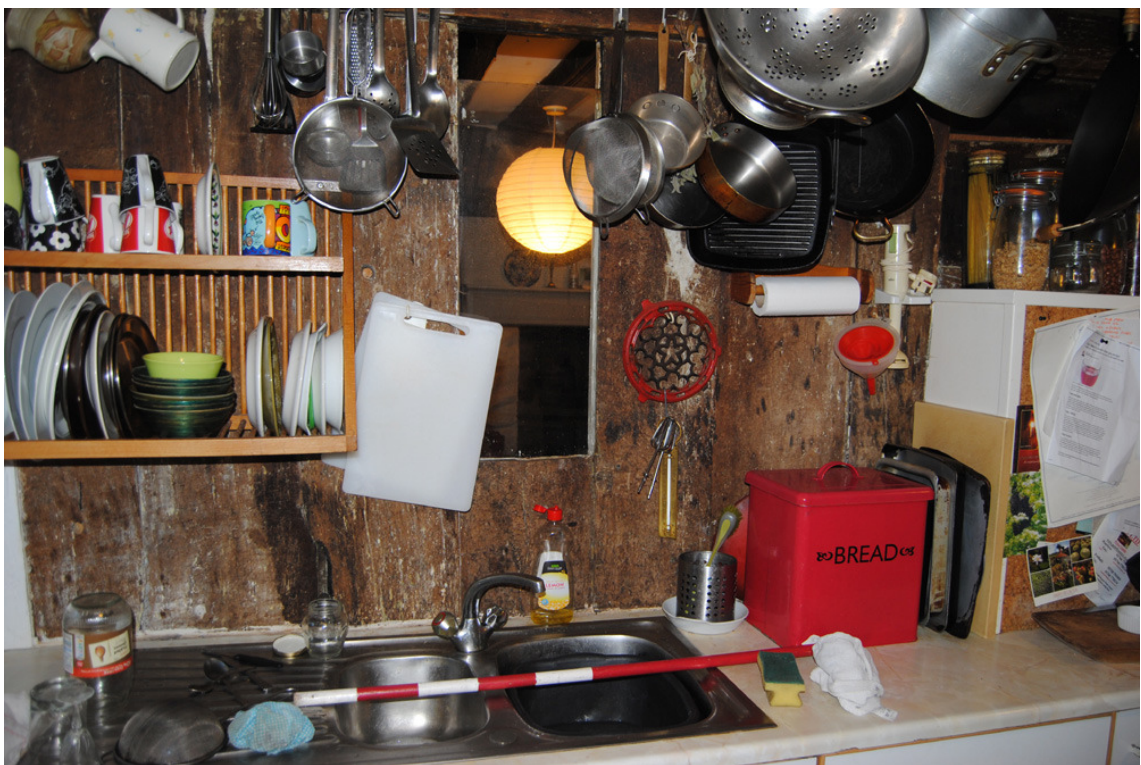
Plate 20: Rear of post and panel partition visible within [GF03].
