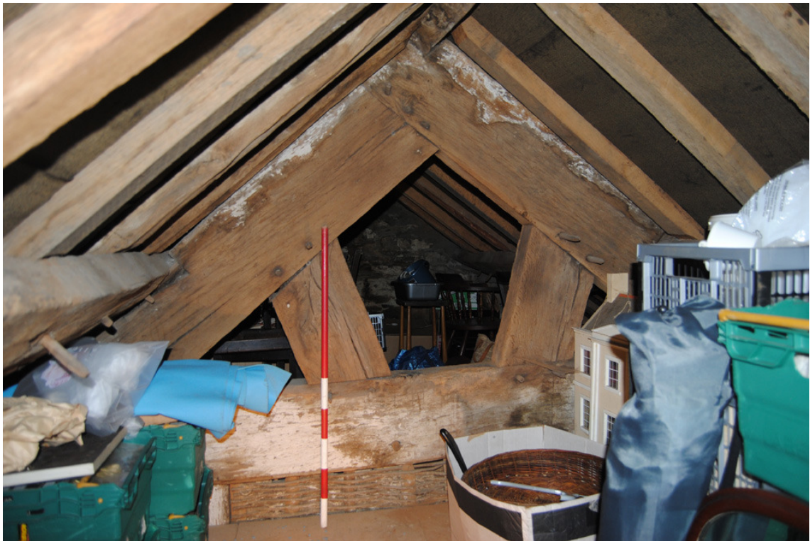
Plate 35: Apex of truss T2 looking north.
