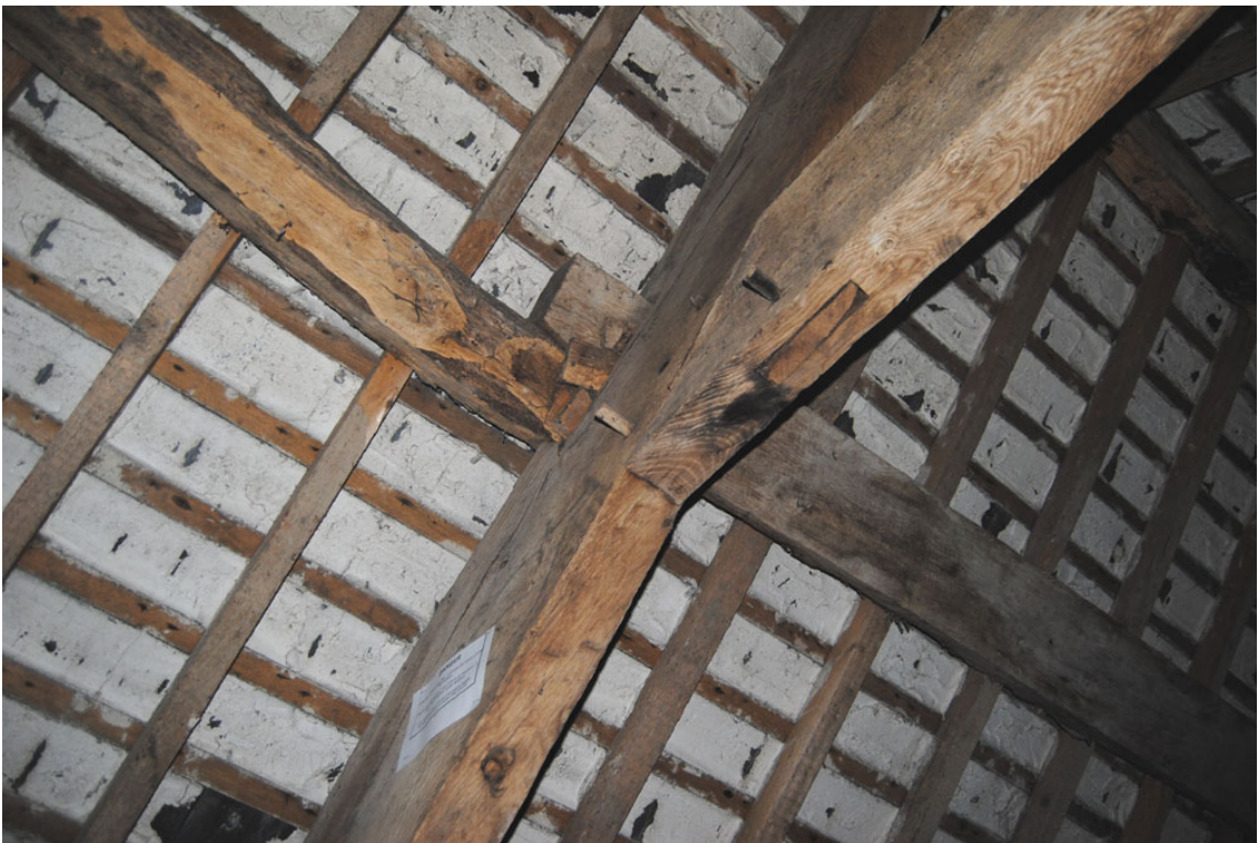
Plate 43: Roof over north-west range, T3 with queen-struts cut off flush with soffit of collar.
