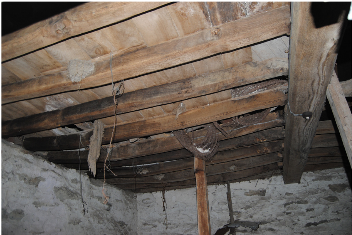
Plate 18: Ceiling structure of [1F01], northern section looking east.
