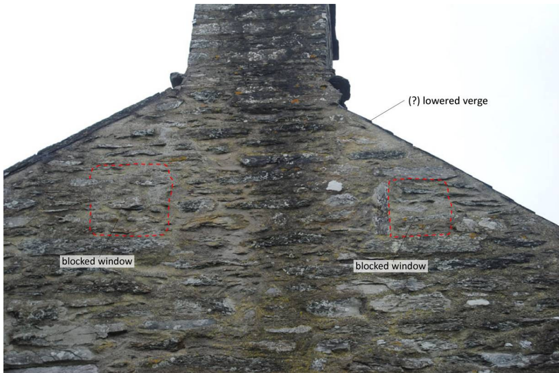
Plate 30: North-west range, east elevation; blocked windows at attic level.
