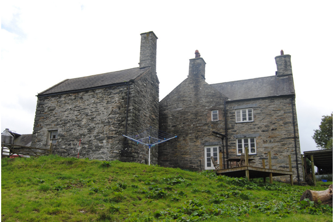
Plate 2: General view of farmhouse from north with kitchen extension to right.
