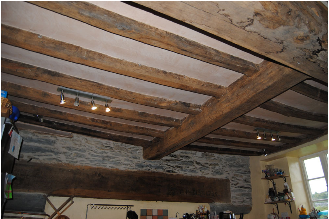
Plate 52: Ceiling structure to [GF04].
