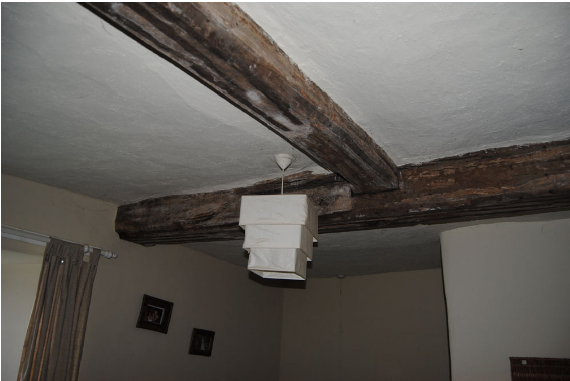
Plate 39: Western transverse beam and southern secondary, longitudinal beam, [1F02].
