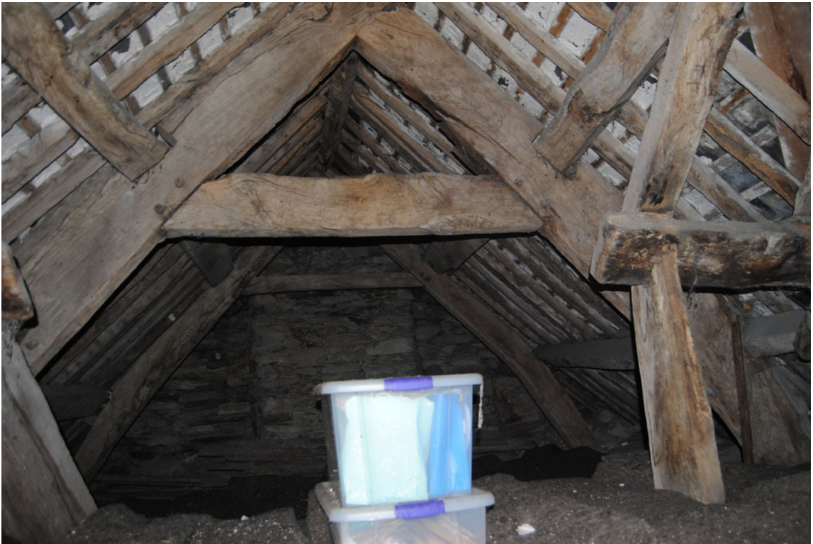
Plate 61: Roof structure over kitchen extension looking north from [1F04].
