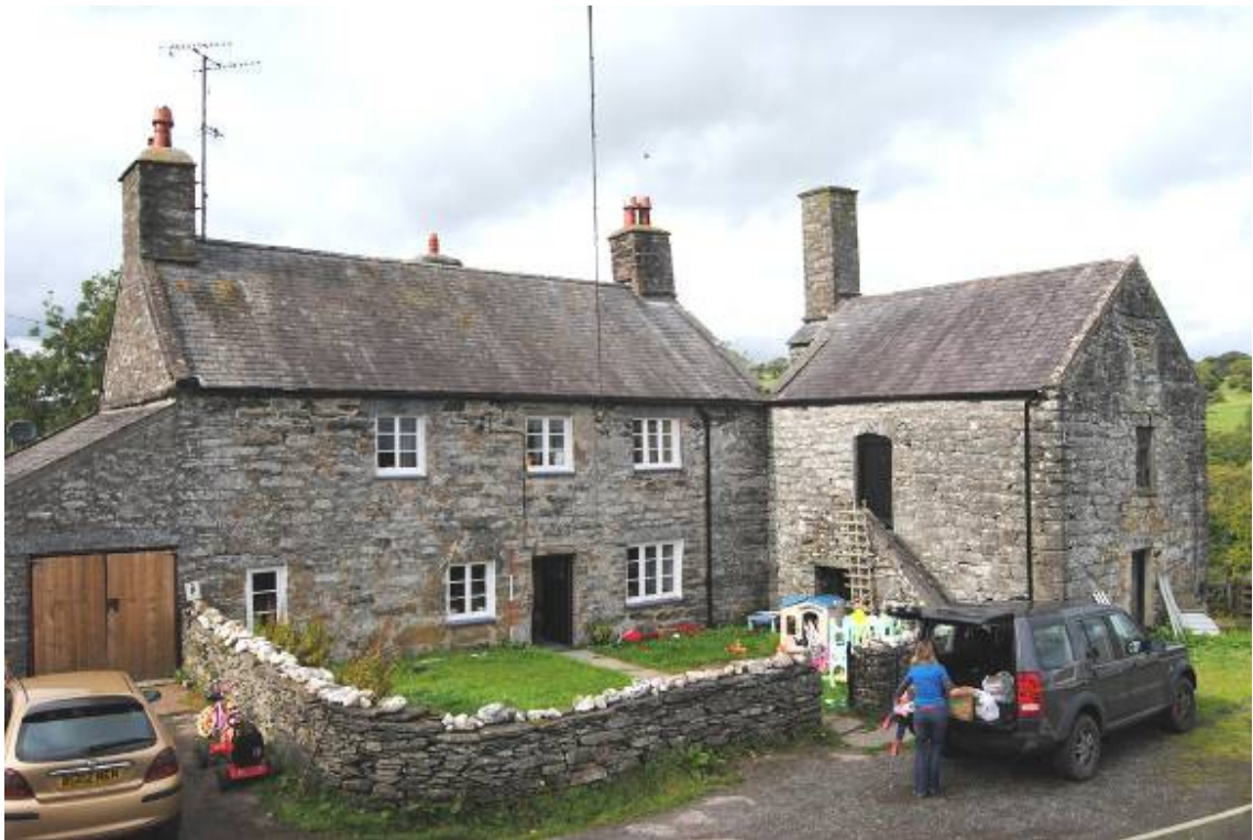
Plate 1: General view of farmhouse from south; early south-east range to right and north-west range to left.
