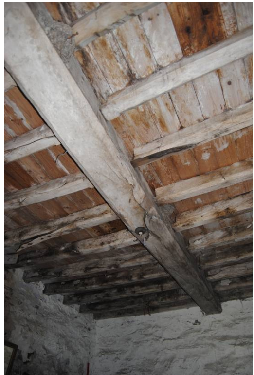
Plate 14: Primary ceiling within [GF01].
