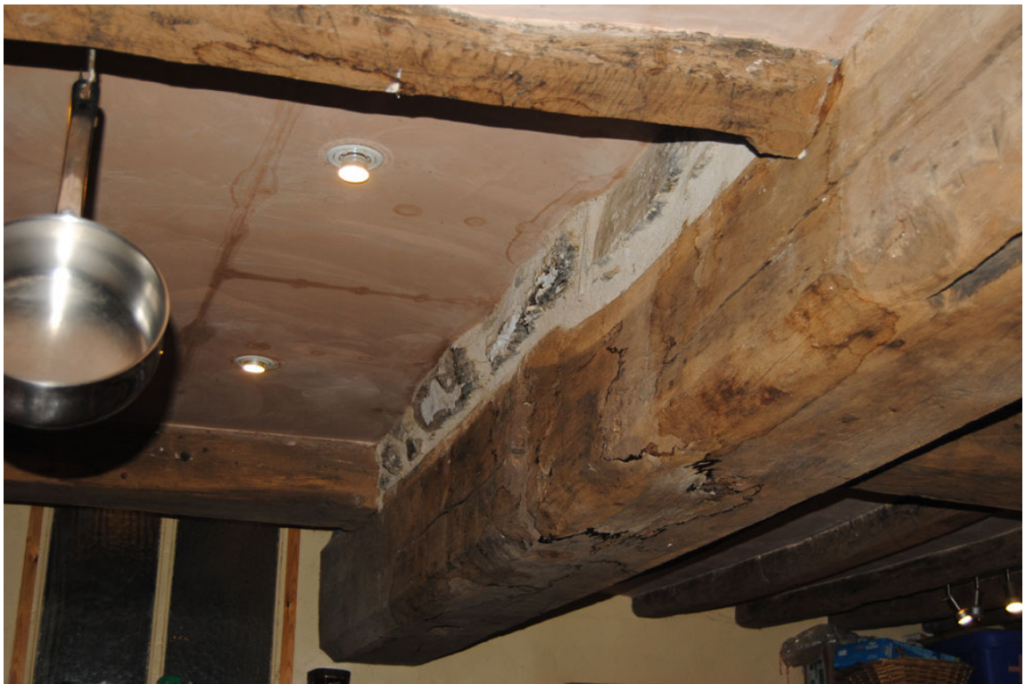
Plate 51: Southern transverse beam of [GF04], note stonework above.
