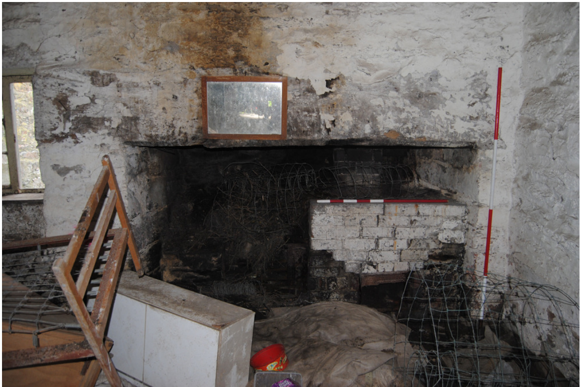
Plate 12: Wide fireplace opening within north wall of [GF01] with inserted copper setting (r.) and range (l.).
