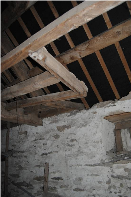
Plate 19: Trimmers at SE corner denote location of former stair.
