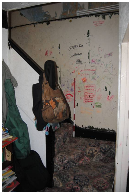
Plate 32: Main stair, [GF02].
