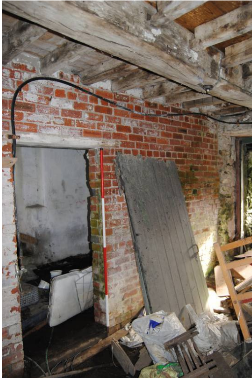
Plate 16: Inserted brick partition.
