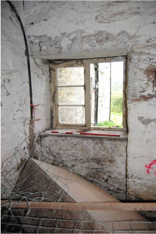
Plate 13: Primary doorway to west of stack.
