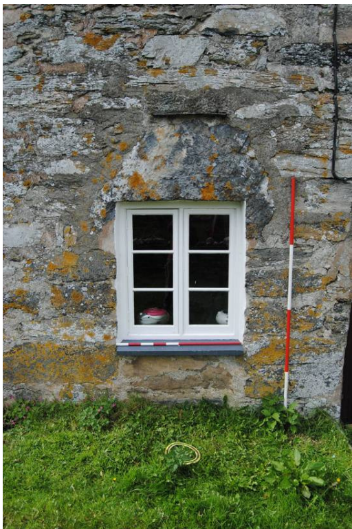
Plate 25: Primary doorway converted to window. NB: massive stone lintel.
