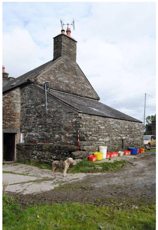
Plate 66: Phase IV Carthouse looking south-east
