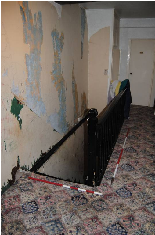
Plate 37: Head of main stair, [1F01].
