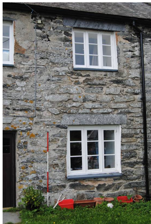
Plate 26: Superimposed windows to [GF03] and [1F04], both reduced in width.
