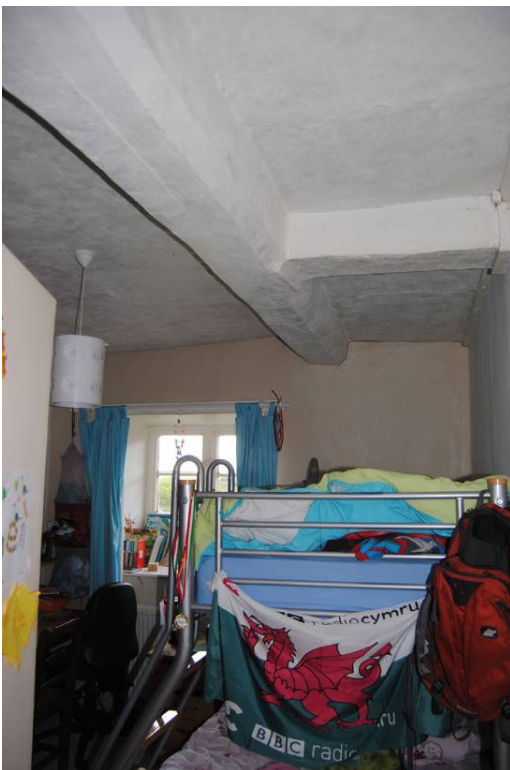
Plate 40: Room [1F03]; transverse and longitudinal ceiling beams
