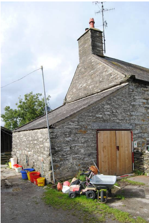
Plate 65: Phase IV Carthouse looking north-east.
