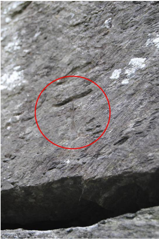
Plate 6: Mason's mark 'T' on quoin of SW angle.
