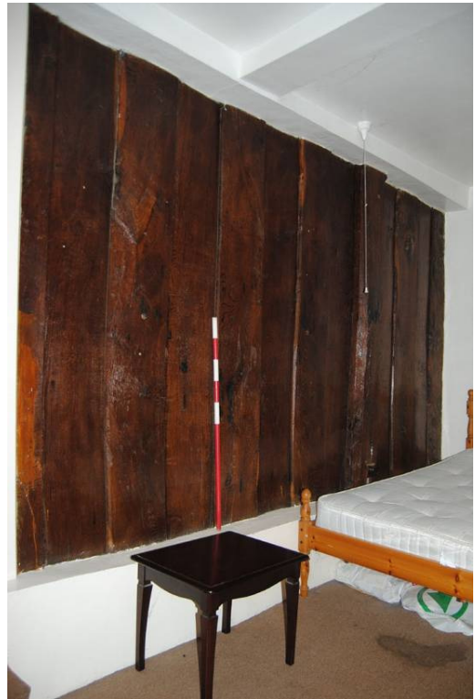
Plate 59: Plank and muntin partition, [1F06].
