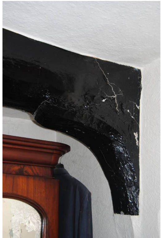
Plate 38: Bracket to western transverse beam.
