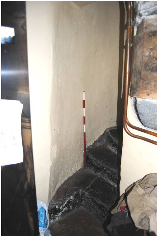
Plate 58: Stone winder stair to east of fireplace, serving [1F06] (see also Plate 59).
