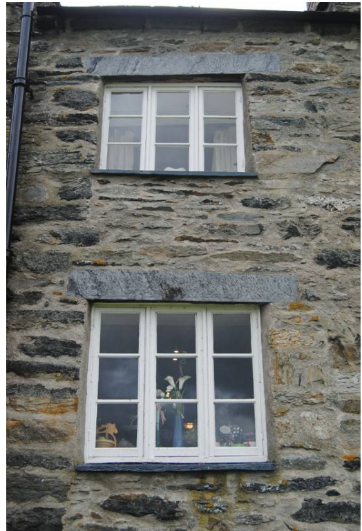
Plate 45: Detail of windows.
