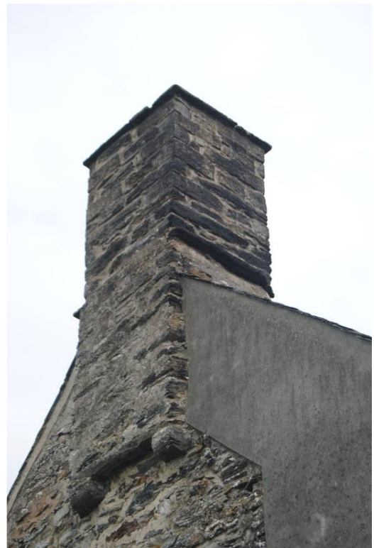
Plate 47: Corbelled stack at attic level.
