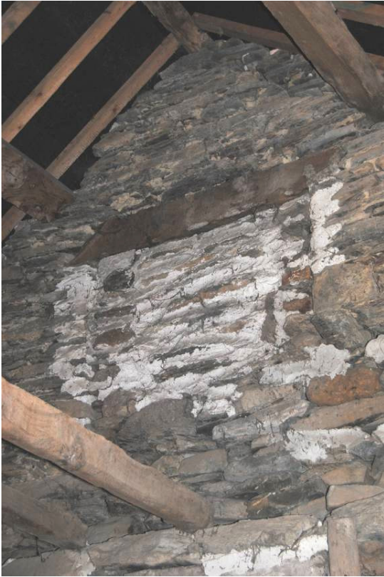
Plate 22: Blocked window in south gable.
