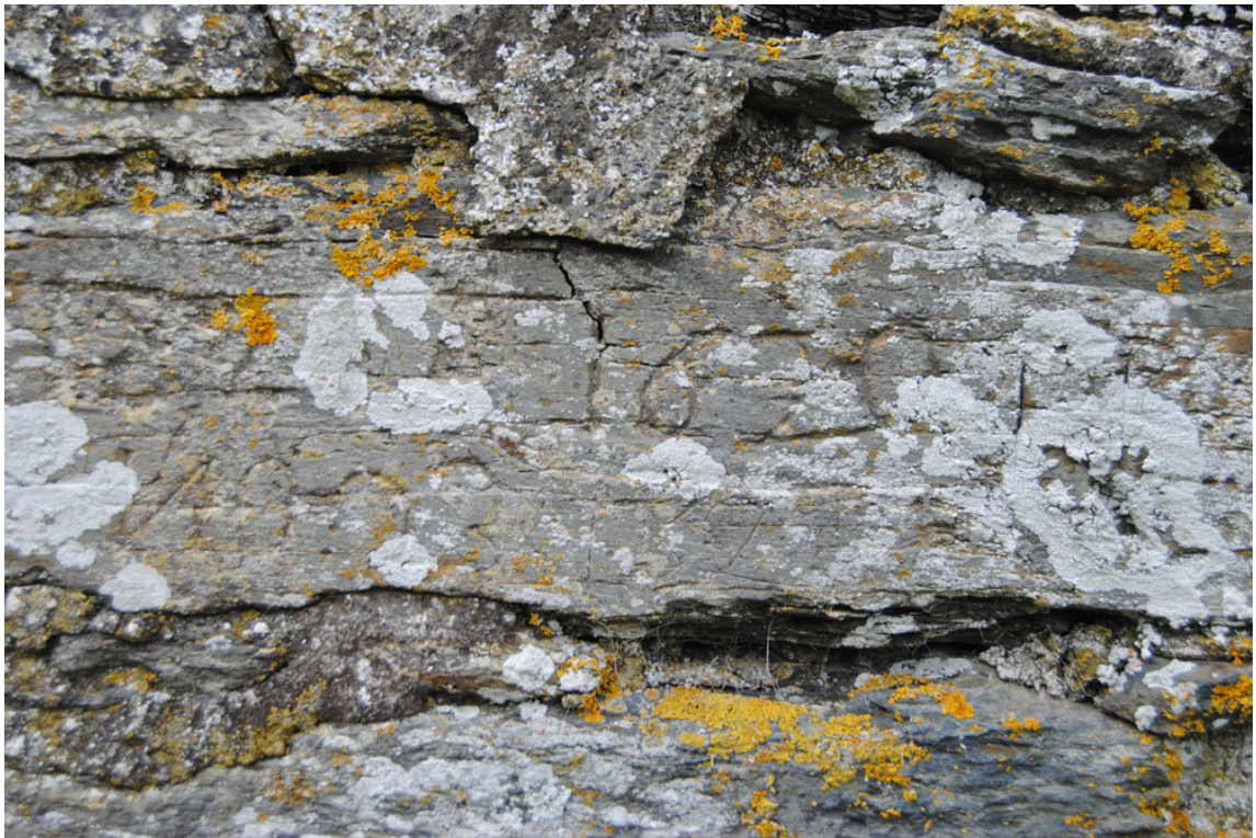
Plate 27: Date inscription ('1620') to west of GF window serving [GF01] (see Figure 9).
