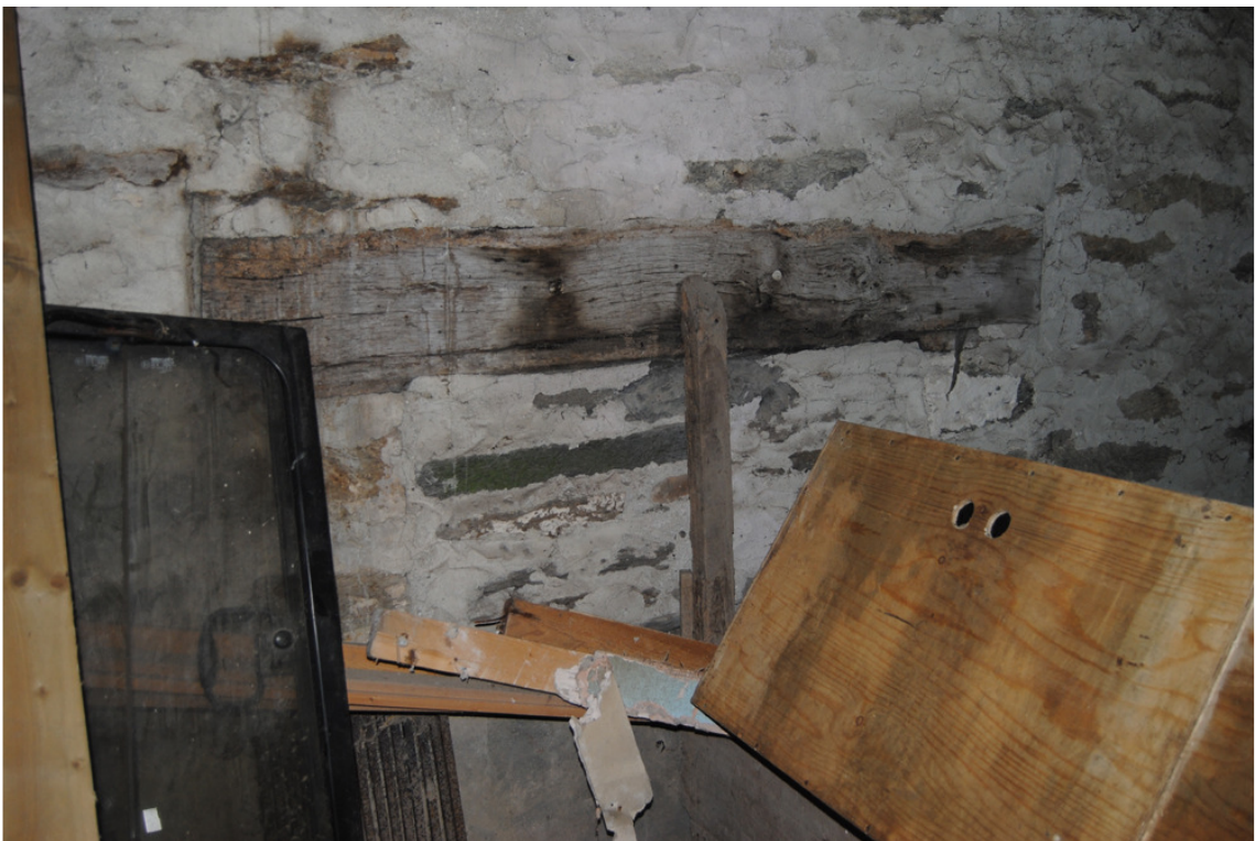
Plate 21: Blocked fireplace with stop-chamfered lintel in north wall of [1F01].
