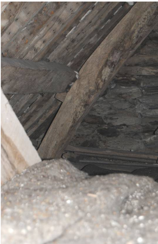
Plate 62: Truss T5, cruck-like west principal, note SJ of blocked window in gable wall beyond.
