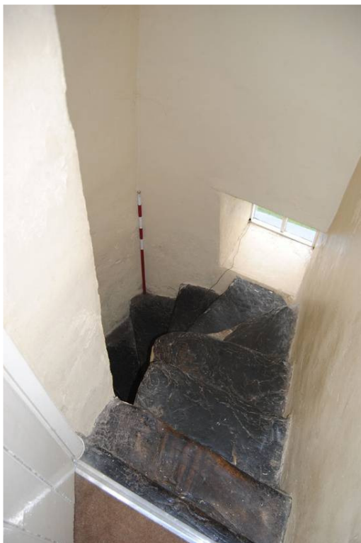
Plate 60: Stone winder stair descends to [GF04].
