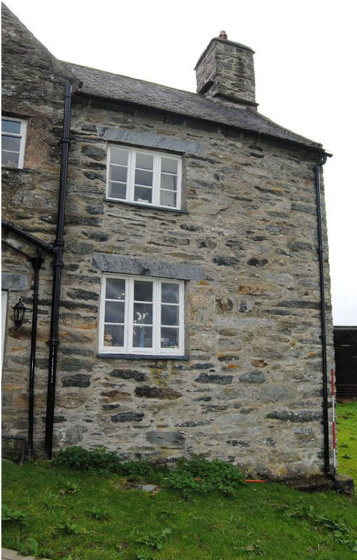
Plate 44: Kitchen extension, east elevation.
