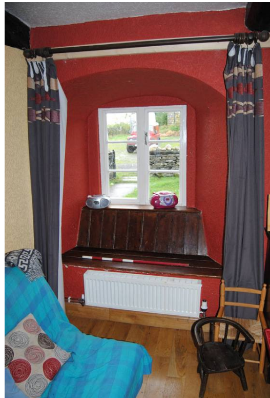
Plate 35: Primary doorway converted to window.
