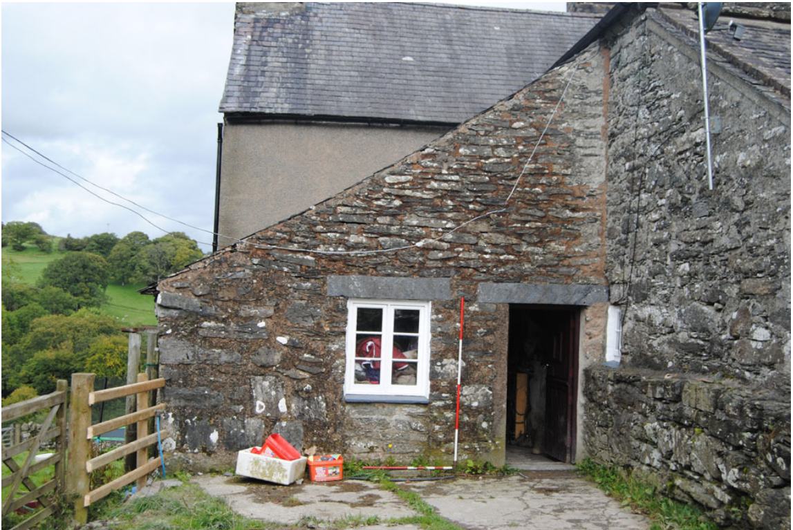
Plate 64: Phase IV (?) dairy (19 th century). NB: straight joints below window evidence former door.
