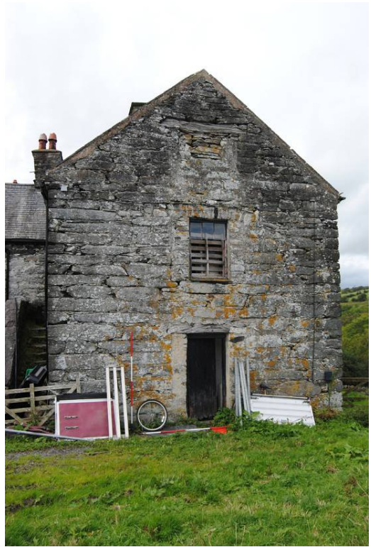
Plate 7: SE range; south elevation. NB: openings to GF/1F/attic (blocked)
