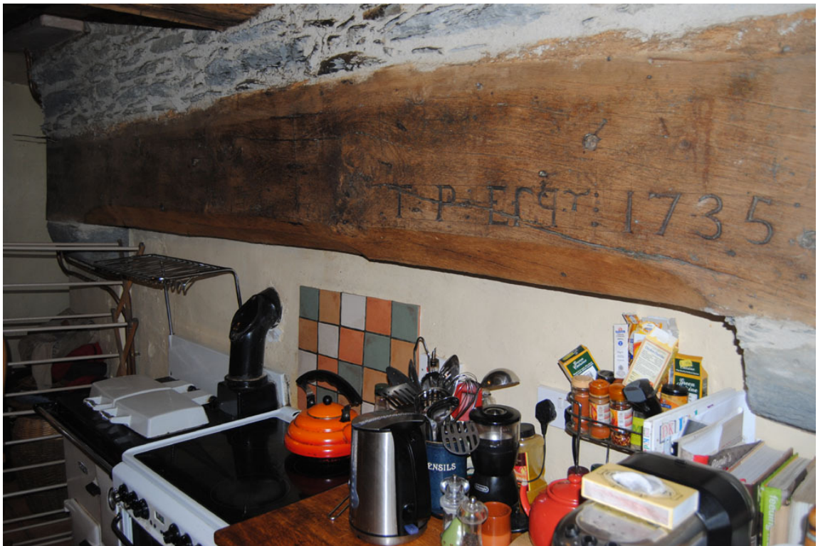
Plate 53: Massive timber mantle beam to fireplace within north wall of [GF04] (note stone corbels).
