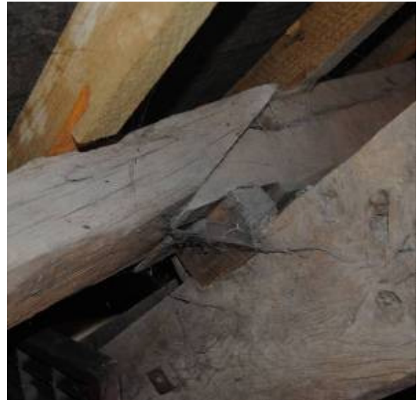
Plate 33: Purlin scarf detail (T3, west).
