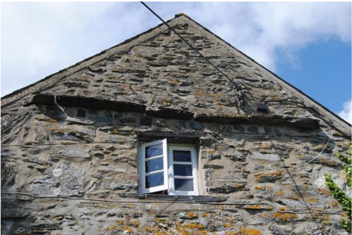
Plate 7: Reduced window opening within east gable.
