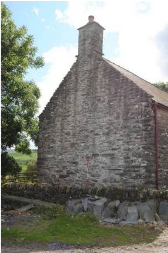
Plate 20: North range, north gable.
