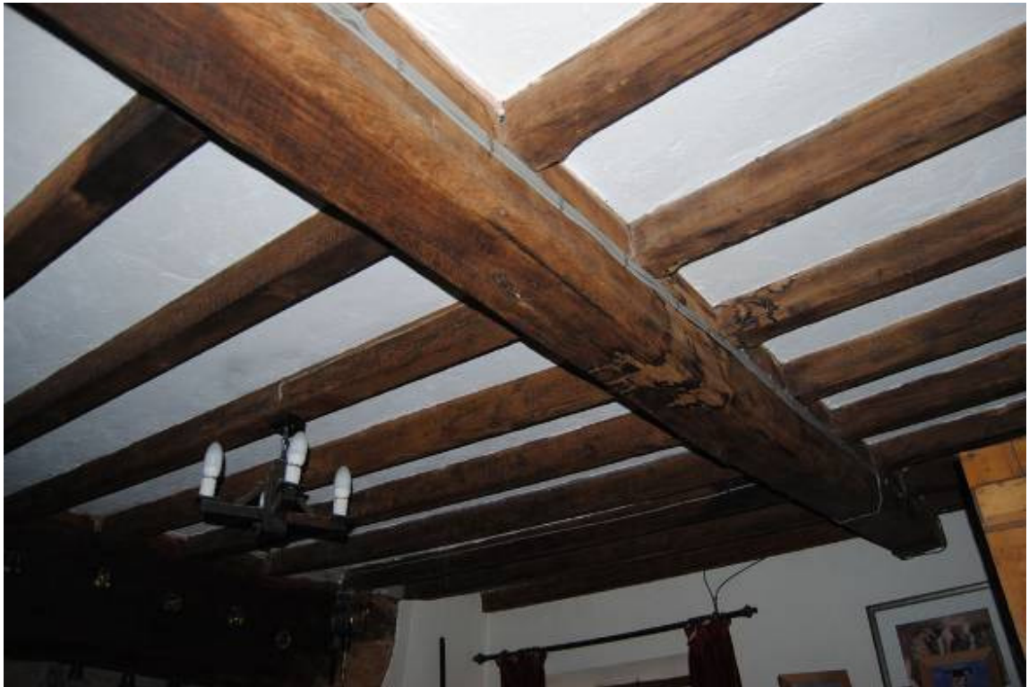
Plate 24: Room [GF04] ceiling.
