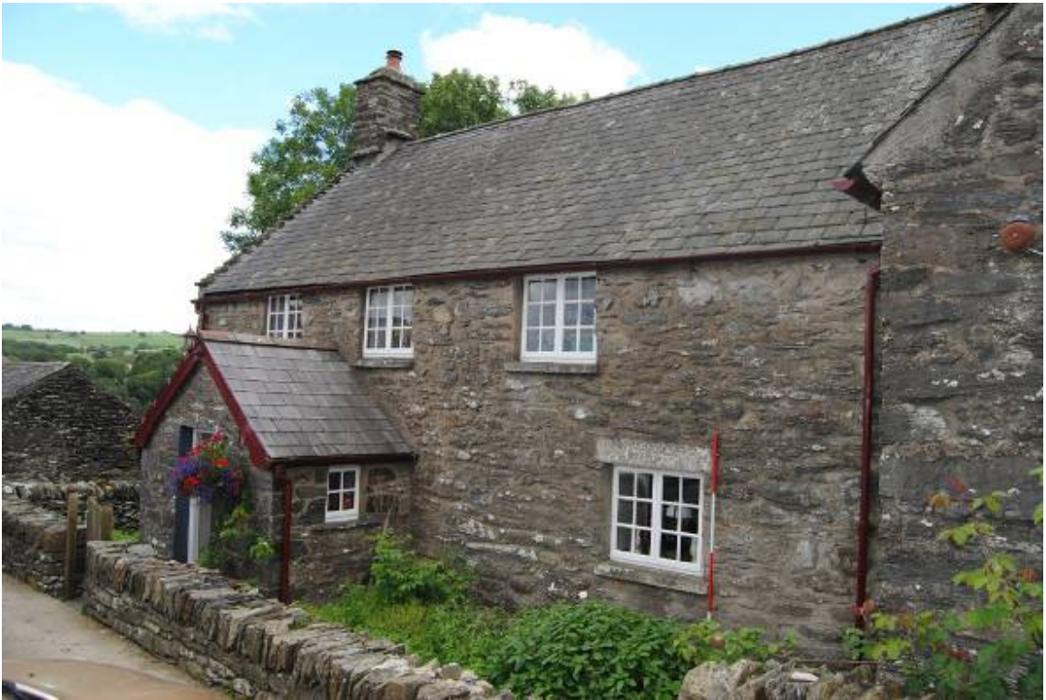
Plate 18: North range, west elevation oblique, looking north-east.
