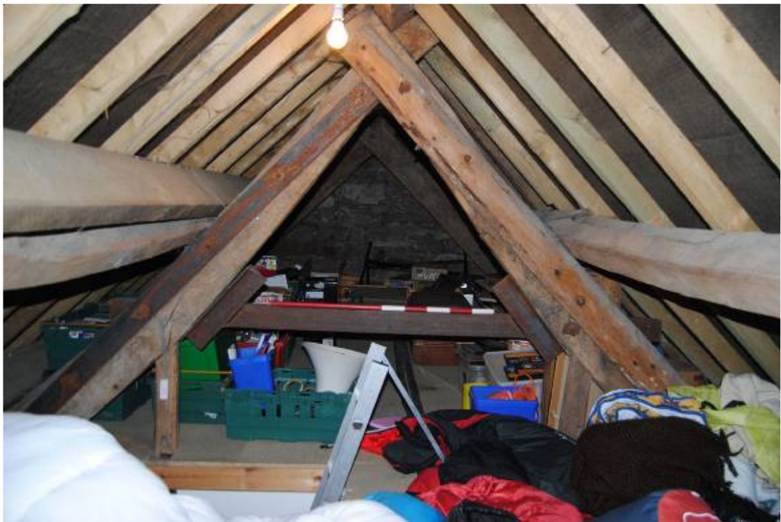
Plate 31: North range, T3 looking north, note vertical struts.
