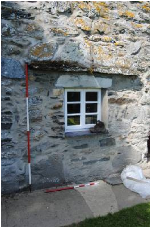
Plate 6: Former door converted to window at centre of south elevation.
