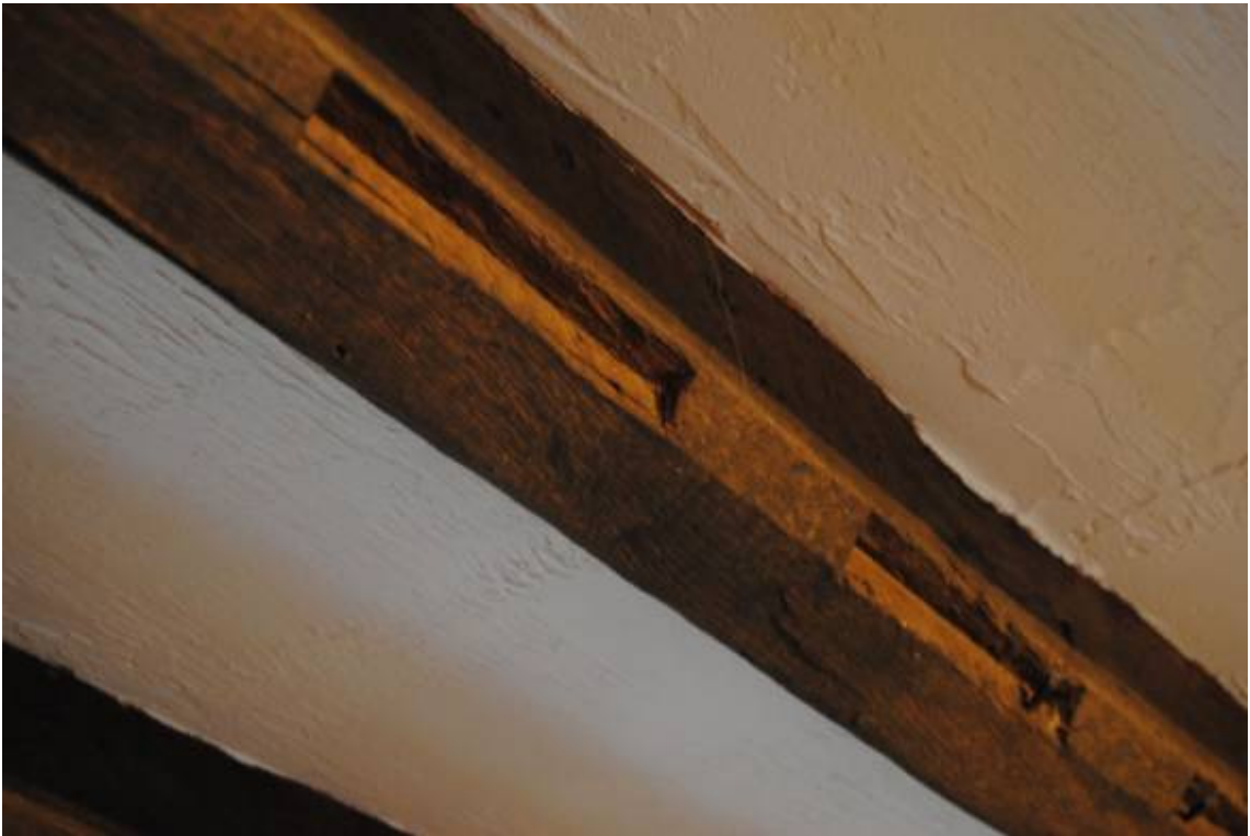
Plate 27: Room [GF06]; evidence for former partition.
