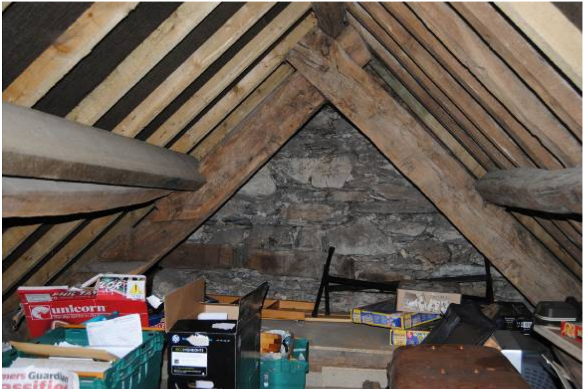
Plate 30: North range, Truss T2 looking north.
