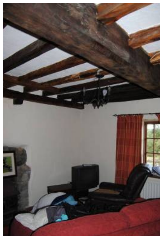
Plate 26: Room [GF06] looking north-east.
