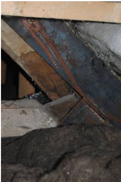
Plate 17: Detail of collar/principal (north), T1.
