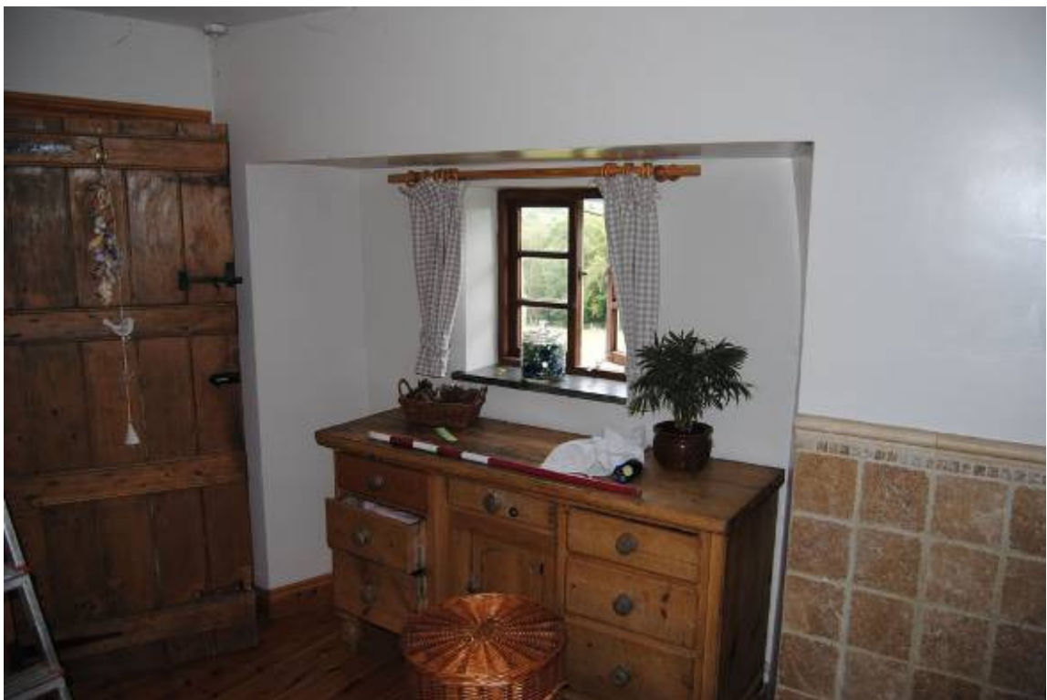
Plate 12: South range, Room [1F02], reduced window opening of east gable (see Plate 7).
