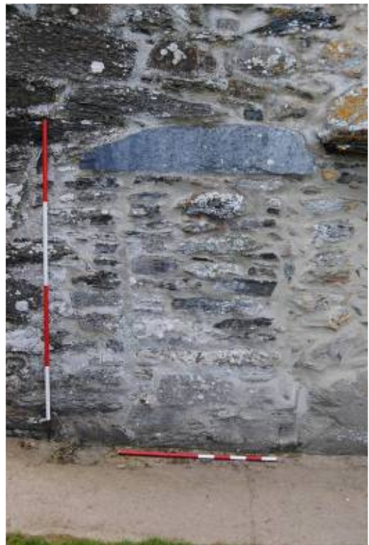
Plate 5: Blocked door at south end, east elevation.
