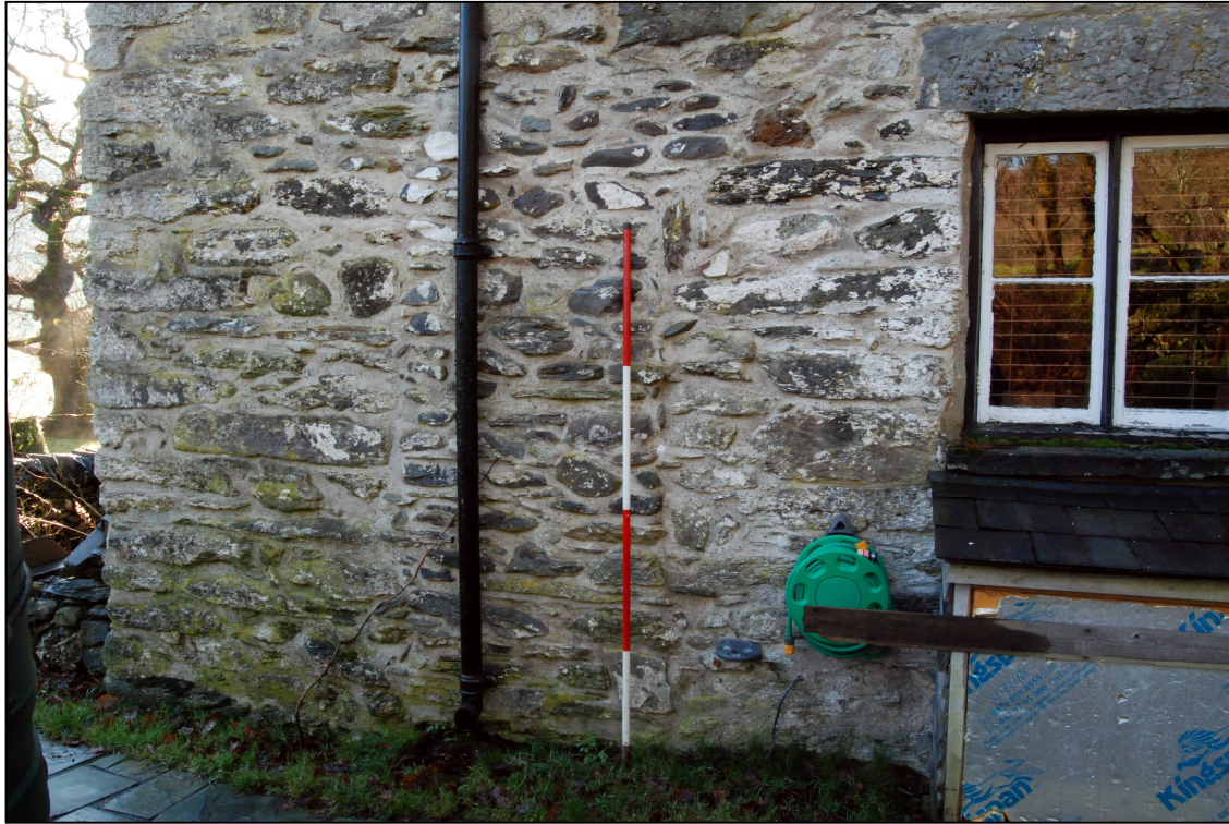
Plate 5: Blocked doorway towards the southern end of the eastern elevation
