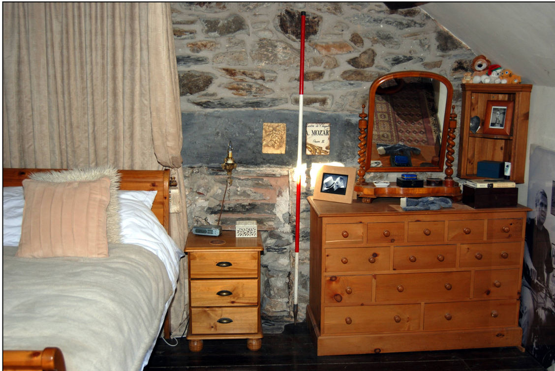
Plate 29: Blocked fireplace in the bedroom in the northern range
