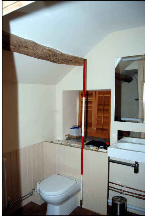
Plate 23: Exposed purlin in the ancillary range
