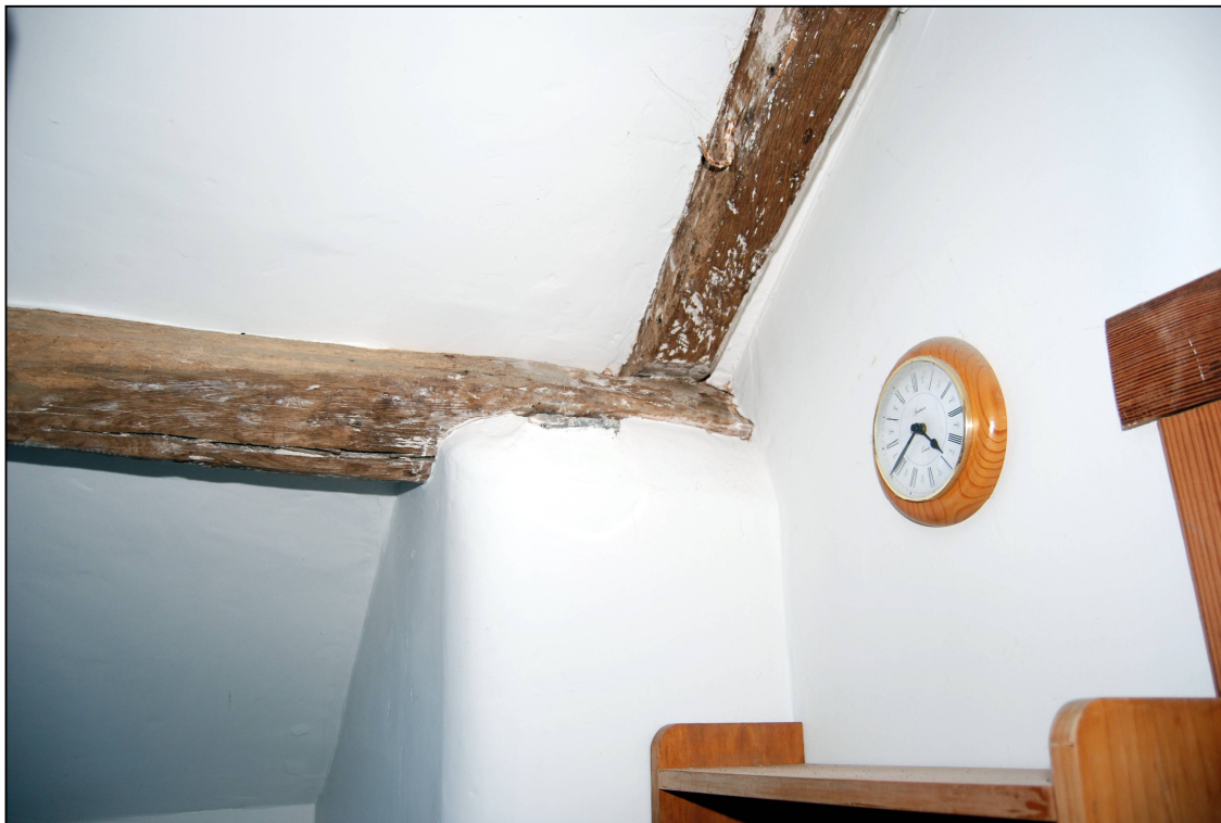
Plate 24: Exposed purlin in the ancillary range
