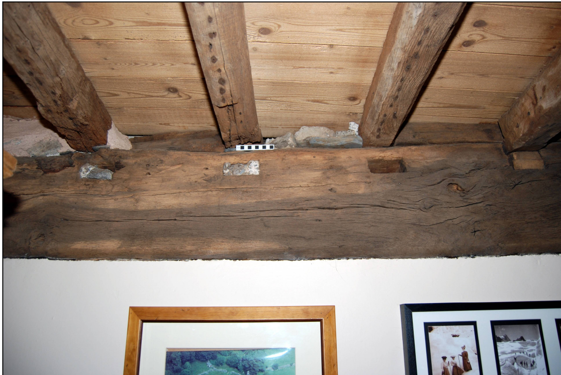
Plate 15: Raised floor on southern side of the “best kitchen”
