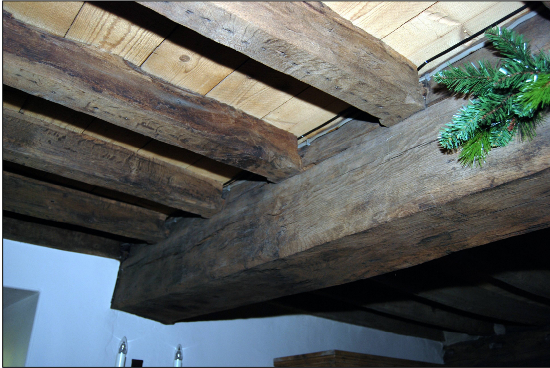
Plate 13: Ceiling beam and joists in the “best kitchen”
