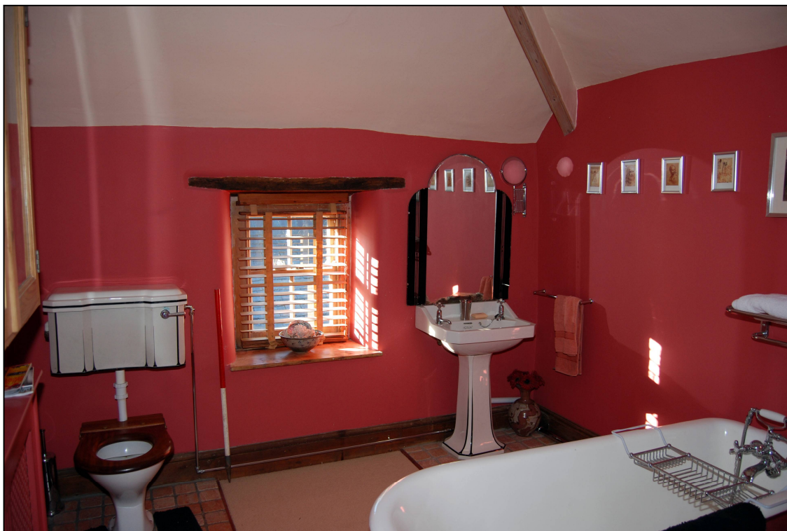
Plate 26: Wooden lintel in the bathroom
