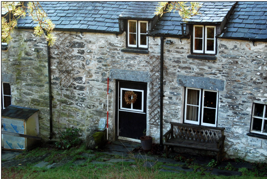
Plate 4: Door way and change of stonework in the eastern elevation
