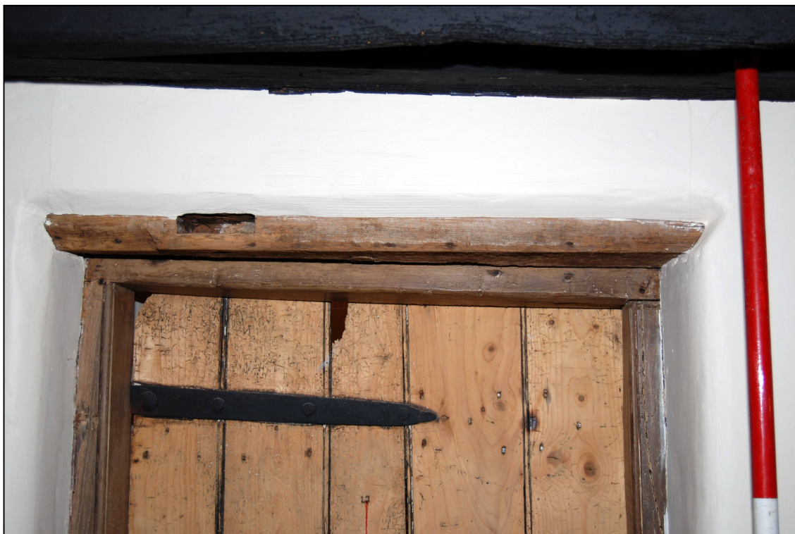
Plate 22: Mortise in the lintel above the door to the ancillary range.
