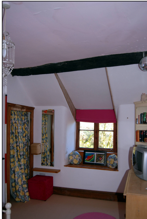
Plate 25: Exposed purlin in the north eastern bedroom of the southern range
