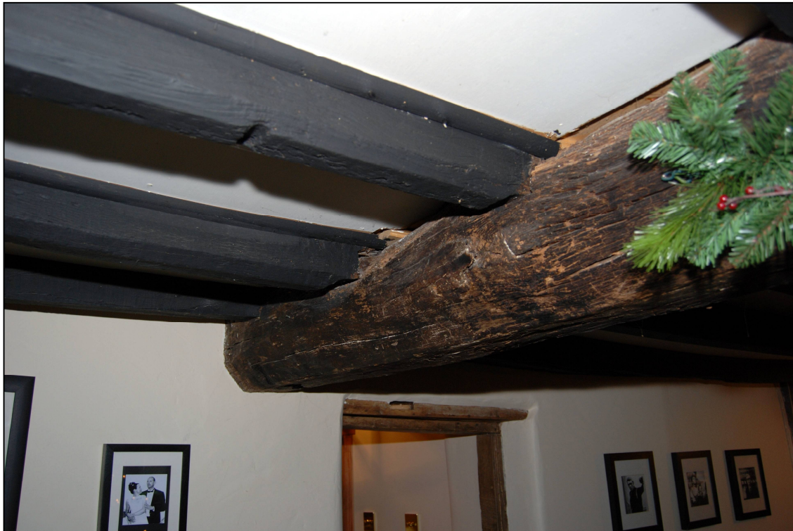
Plate 21: Ceiling beam in the “rear kitchen”
