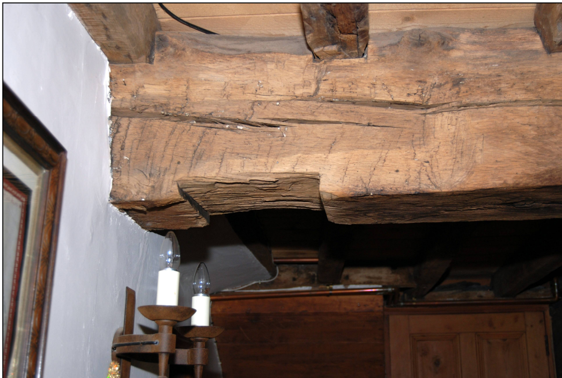
Plate 14: Cut away section of the ceiling beam in the “best kitchen”
