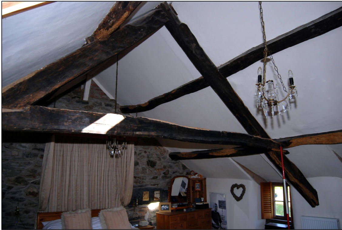
Plate 27: Truss in the northern range
