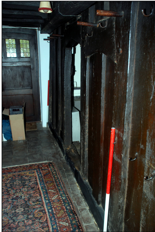
Plate 11: The partition between the pantry and the cross passage
