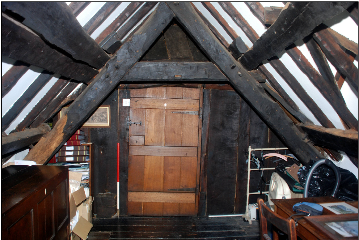
Plate 22: The partition between the first floor hall room and the staircase
