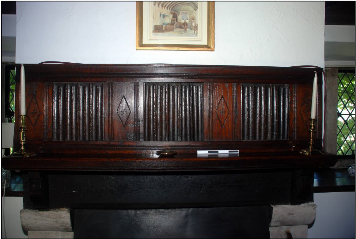
Plate 19: Re-used linen fold panelling above the fireplace in the cross wing
