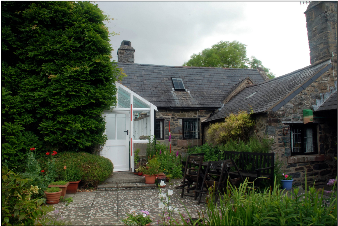
Plate 3: Southern elevation of the hall
