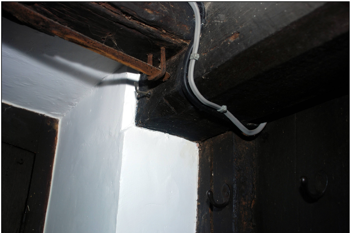
Plate 16: Chamfer and stop on the beam in the cross passage
