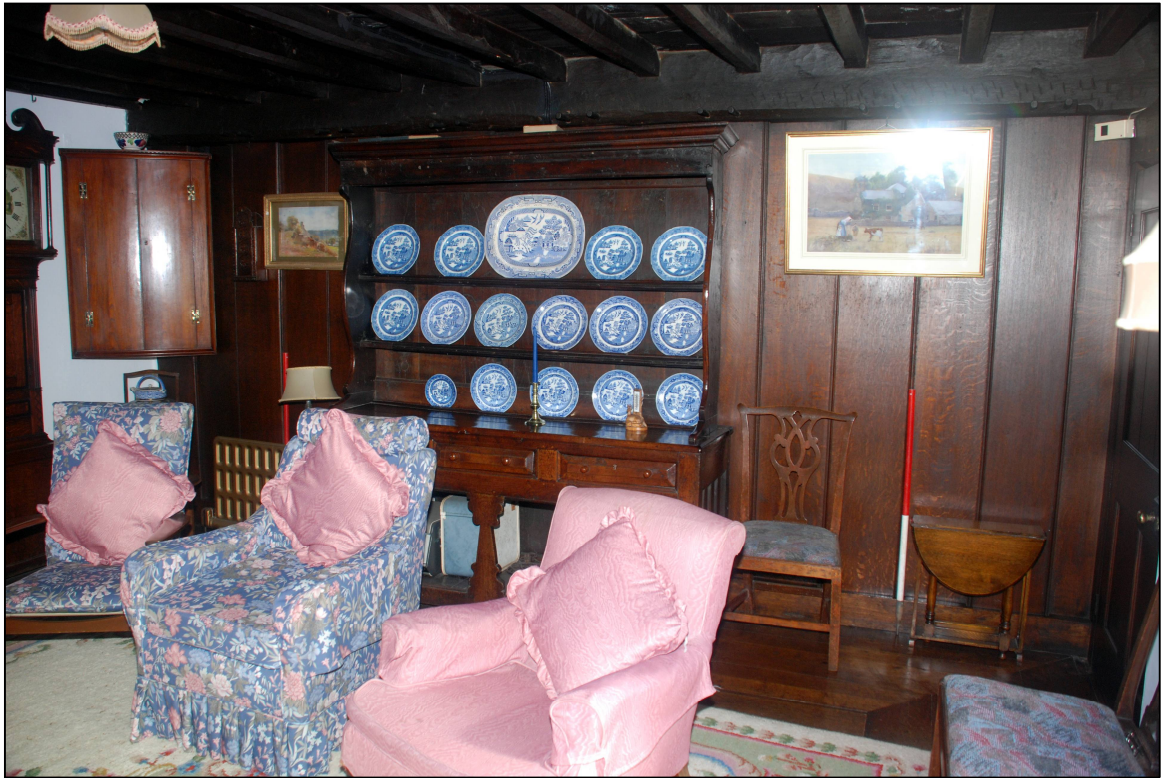
Plate 31: The partition between the two ground floor rooms in the cross wing
