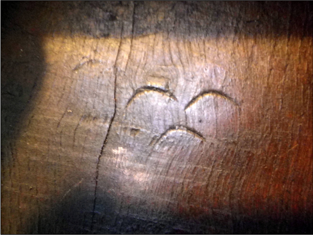
Plate 25: Carpenters marks on the stair partition
