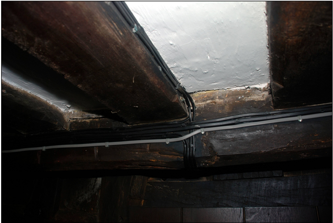
Plate 17: Chamfer and stops on the joists in the cross passage
