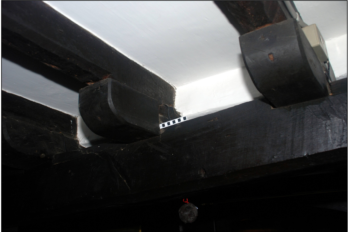
Plate 15: Two level of joists in the hall
