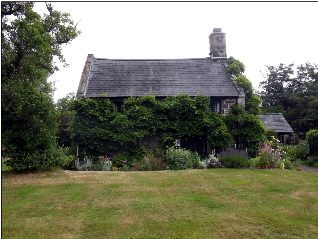
Plate 6: Western elevation of the cross wing
