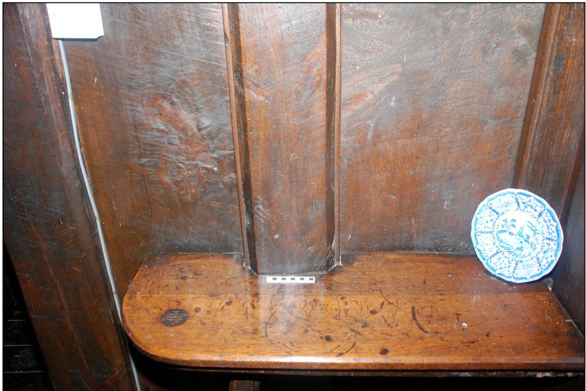
Plate 24: Detail of the form of the posts of the staircase partition
