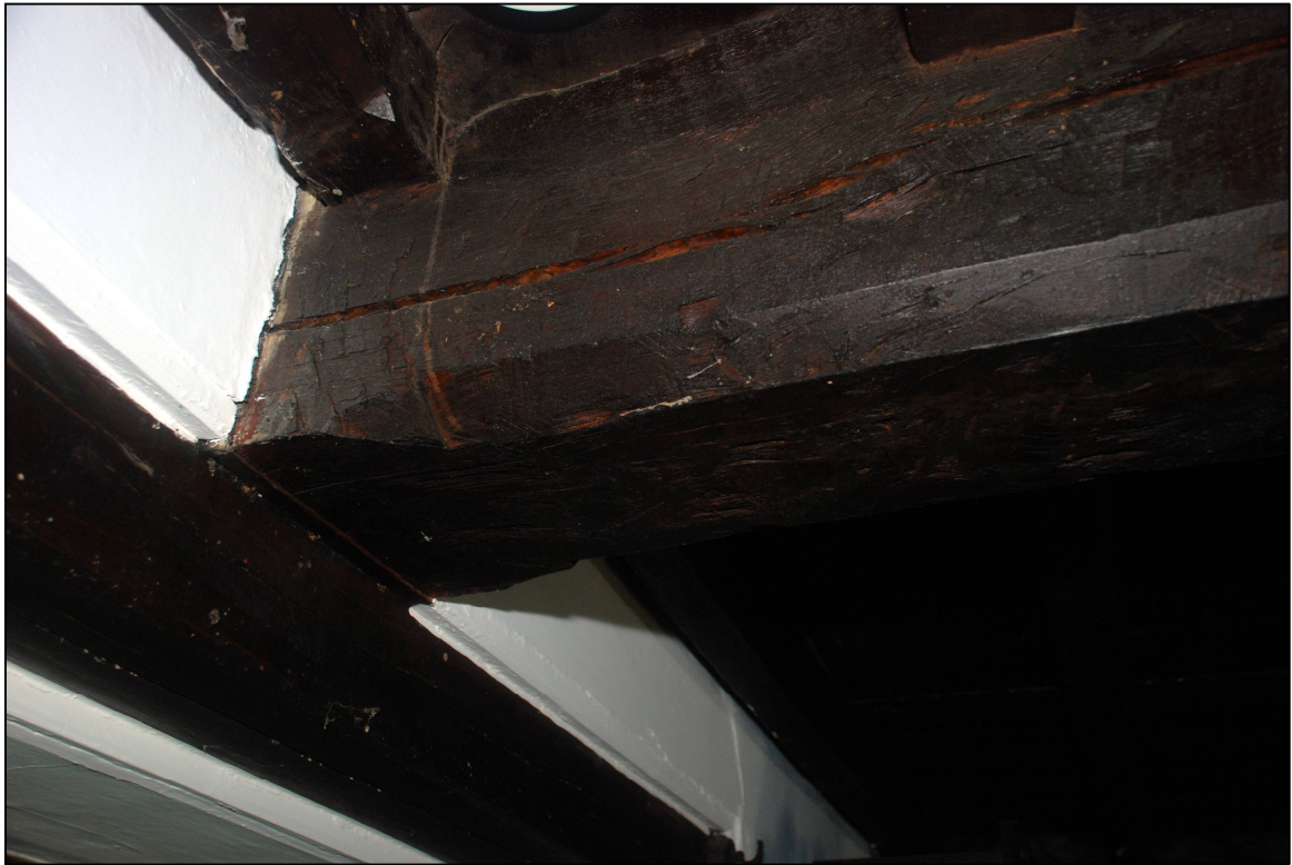
Plate29: Step stop on ceiling beam in cross wing
