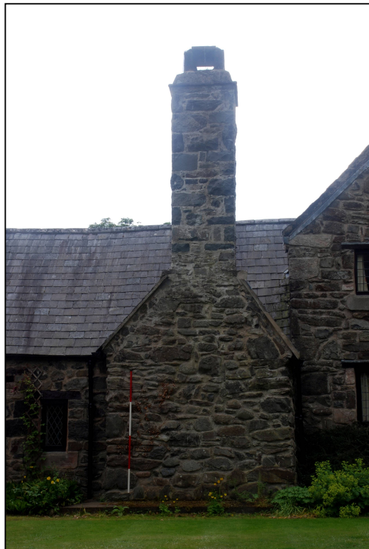
Plate 2: The lateral chimney
