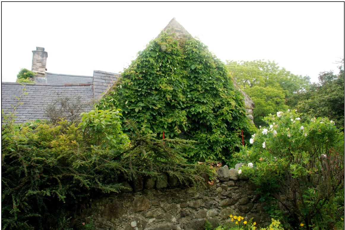
Plate 4: Eastern gable end
