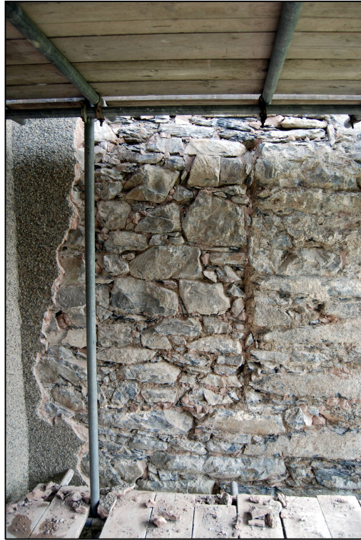
Plate 3: Blocked doorway in the northern elevation of the southern range
