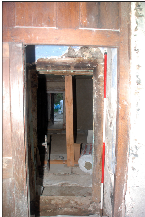
Plate 20: Original doorway between the kitchen and the hall
