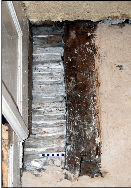
Plate 46: Timber framing in the stair tower
