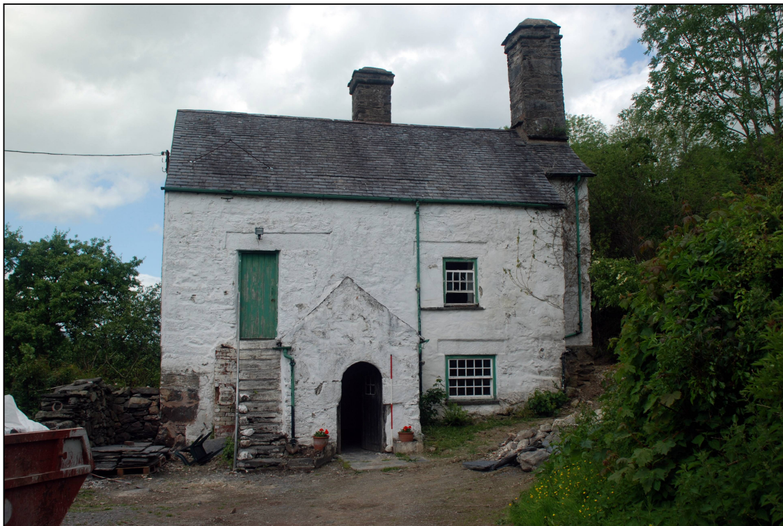
Plate 5: The southern elevation
