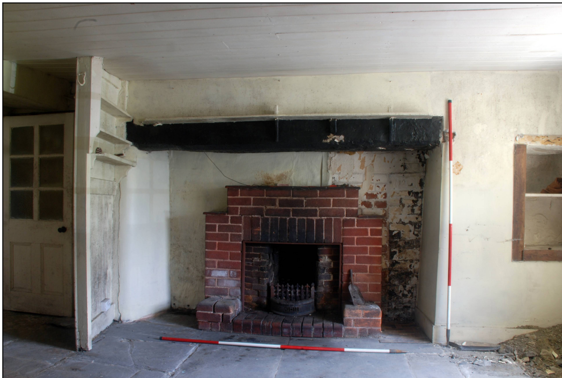
Plate 14: The kitchen fireplace before restoration
