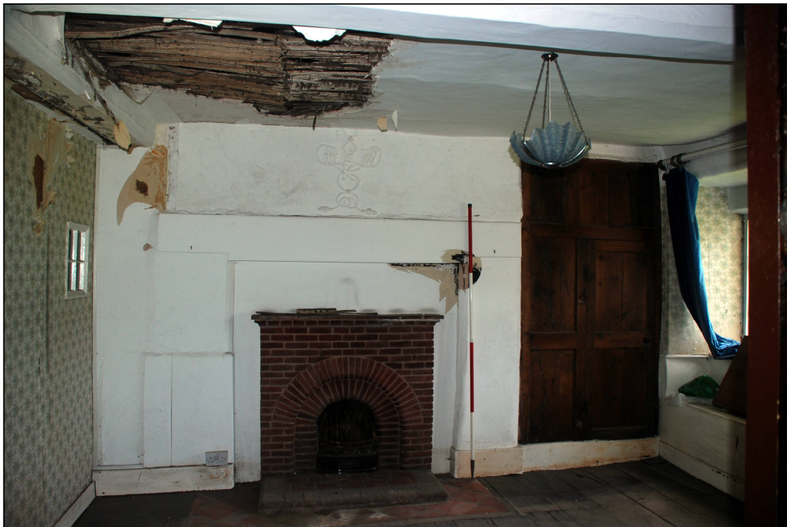
Plate 22: The hall fireplace before restoration
