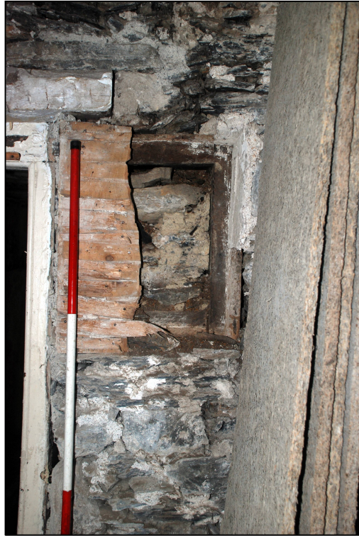
Plate 19: Remains of a cupboard cut by the doorway between the kitchen and the hall
