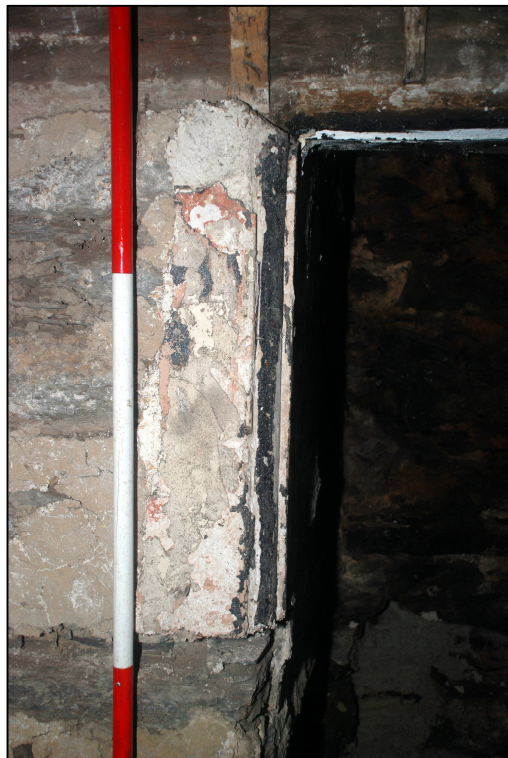
Plate 24: Remains of the plaster moulding around the ground floor hall fireplace
