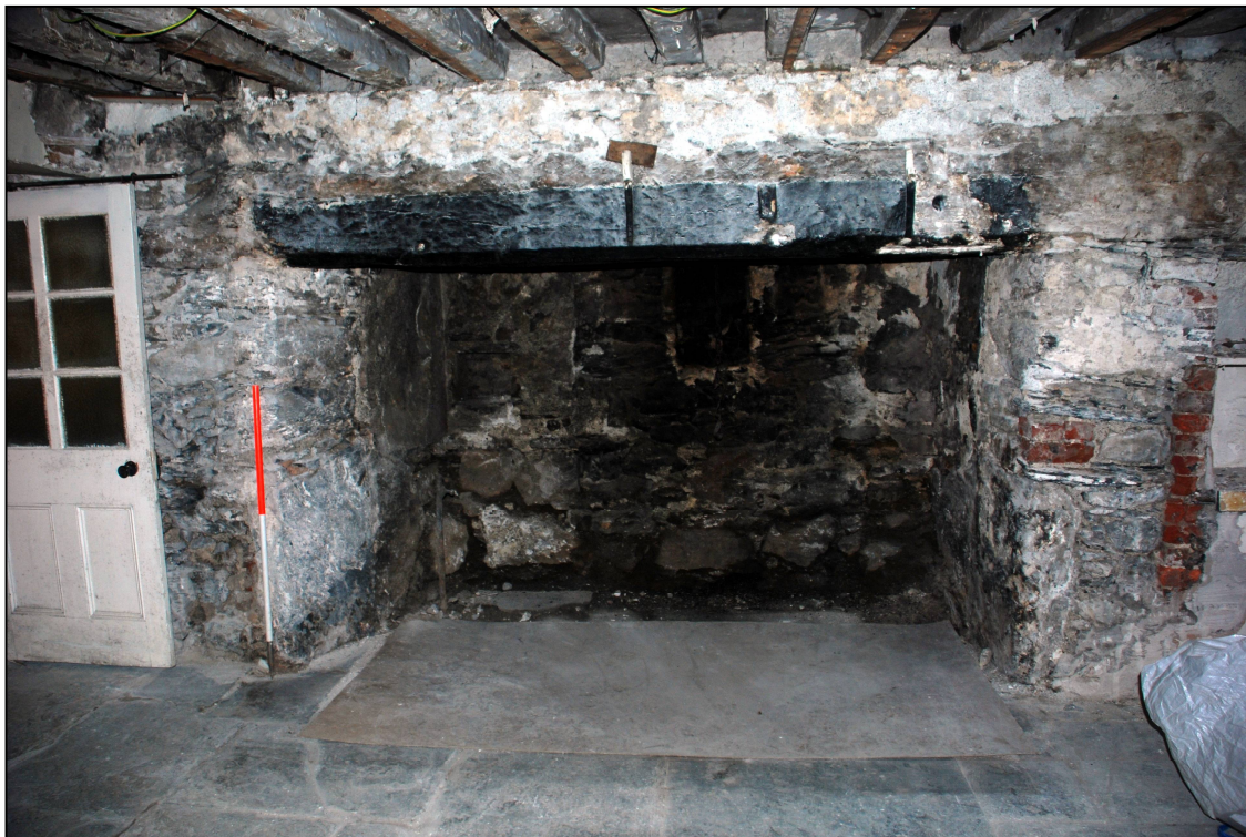
Plate 15: The kitchen fireplace after the removal of the later structures
