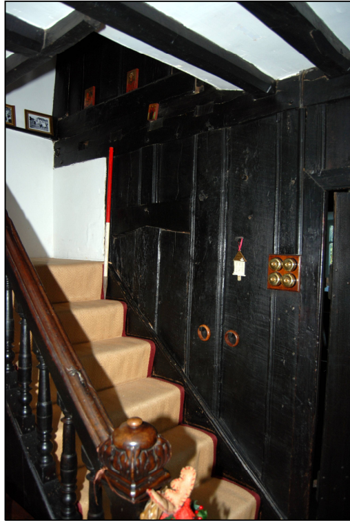
Plate 15: Doorway blocked by the staircase
