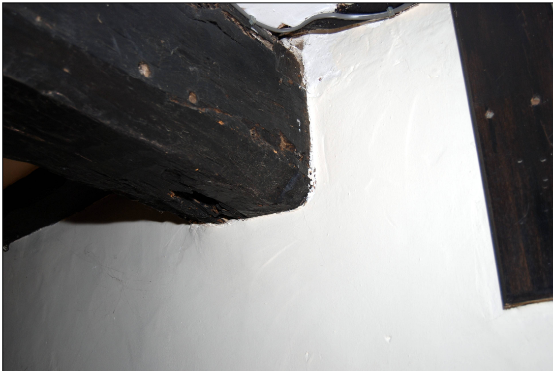
Plate 11: Stop on the beam in the ground floor hall
