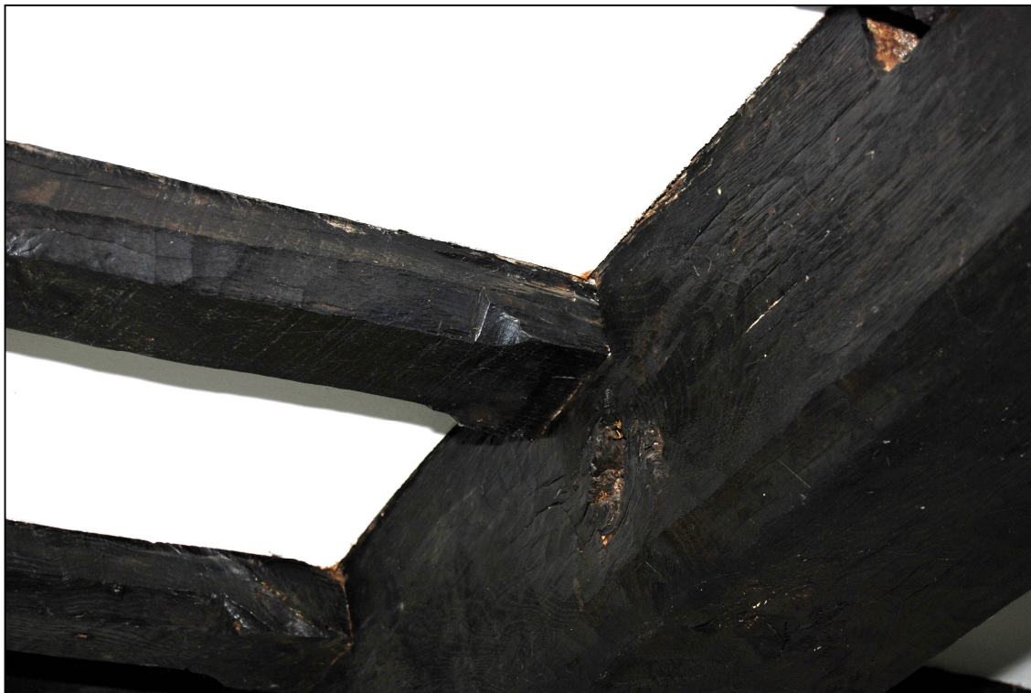
Plate 28: The joists in the bathroom
