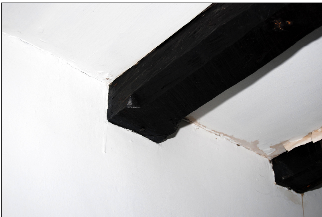
Plate 32: Detail of joist in the south eastern bedroom
