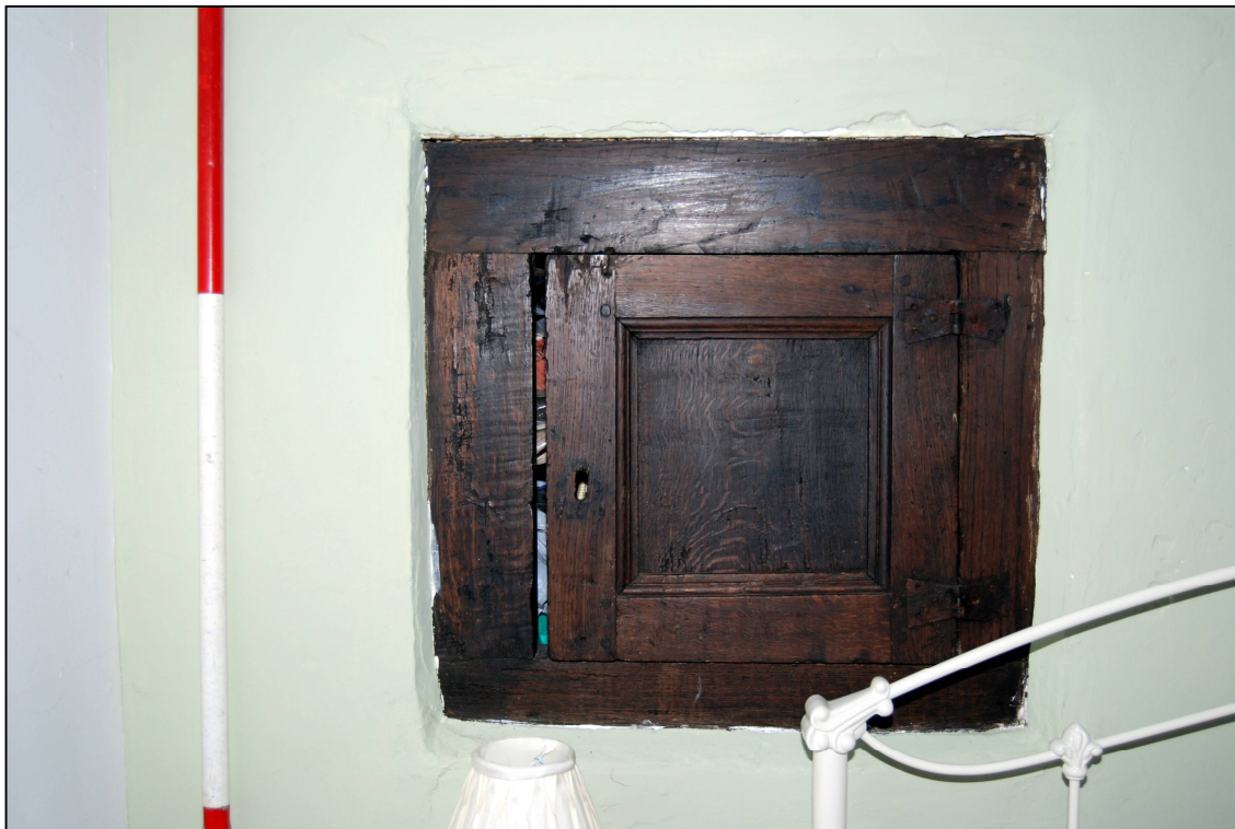
Plate 34: Detail of the cupboard in the north eastern bedroom
