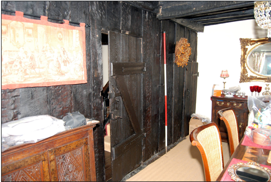
Plate 21: The partition in the parlour looking SW
