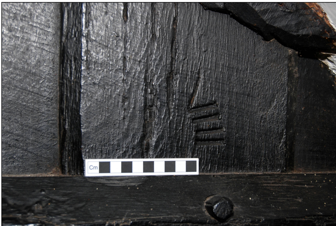
Plate 18: Carpenter's mark on the ground floor partition
