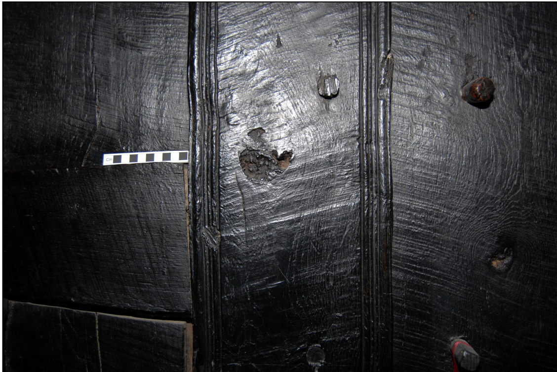
Plate 17: Moulding on the posts of the ground floor partition
