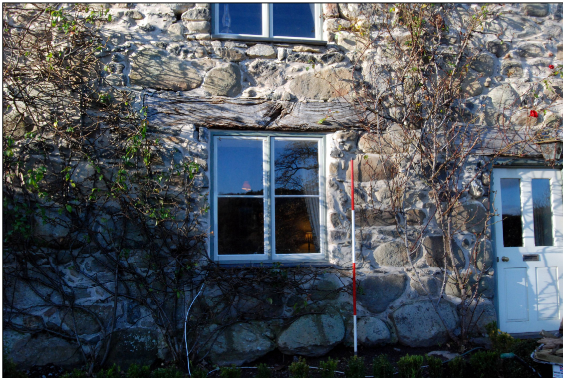
Plate 4: The southern, ground floor window
