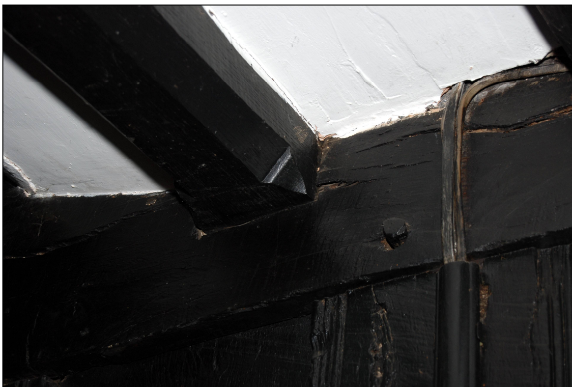
Plate 12: Stop on a joist in the ground floor hall
