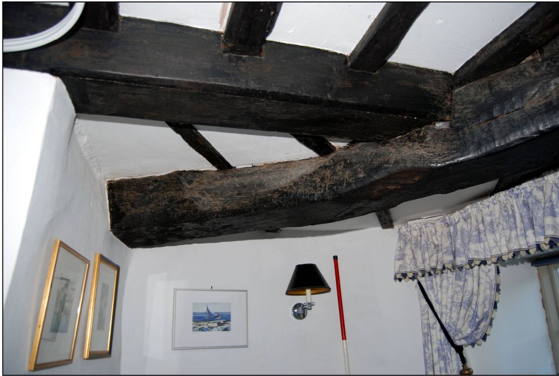
Plate 27: Arrangement of the beams in the bathroom
