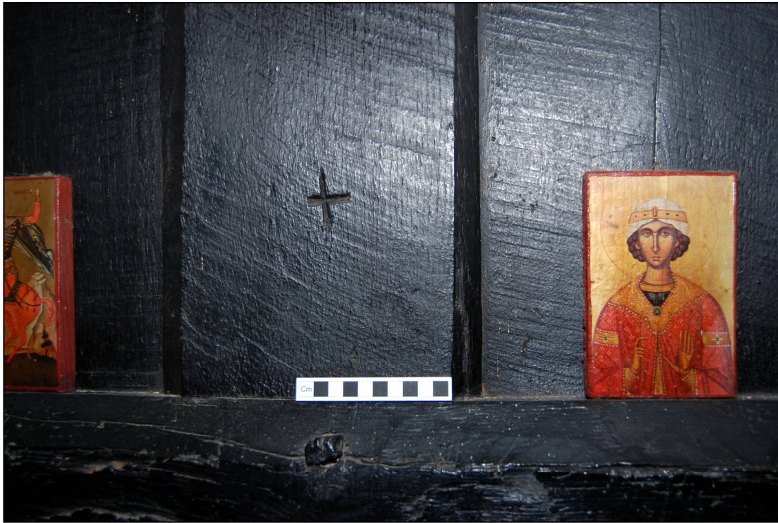
Plate 19: Carpenter's mark on the ground floor partition
