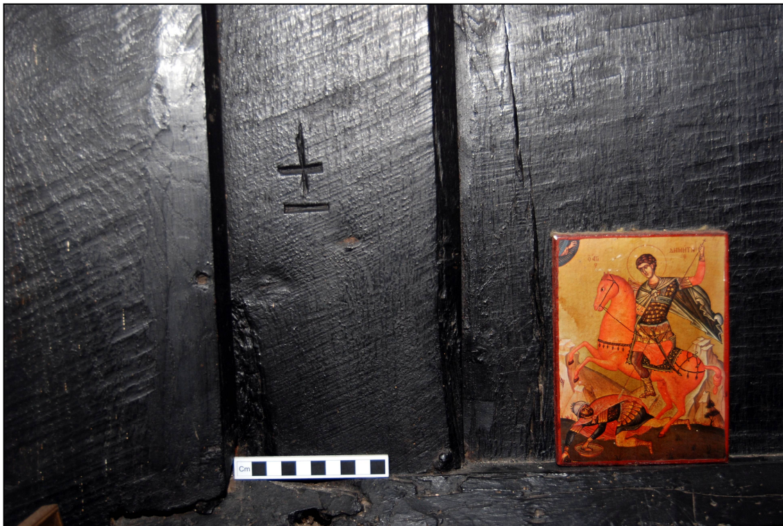
Plate 20: Carpenter's mark on the ground floor partition
