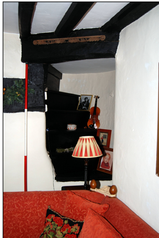
Plate 10: Partially blocked staircase in the ground floor hall
