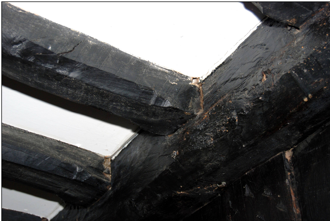
Plate 25: The joists in the parlour
