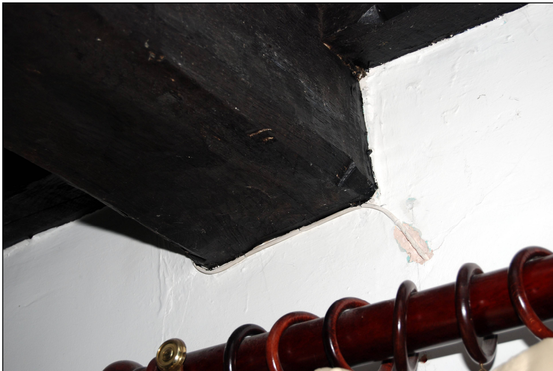
Plate 31: Ceiling beam in the south eastern bedroom
