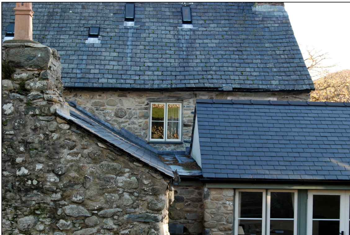
Plate 8: Window in the rear elevation
