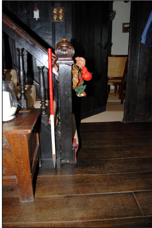
Plate 13: The ground floor section of the staircase
