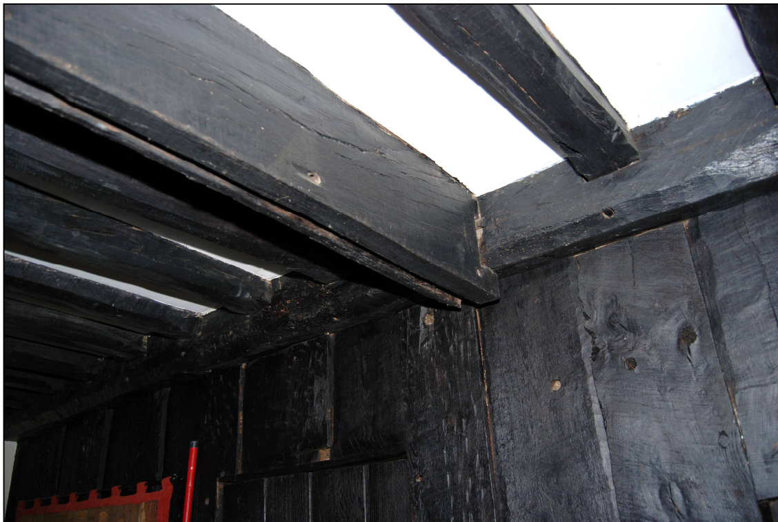
Plate 24: Slot below a joist in the parlour
