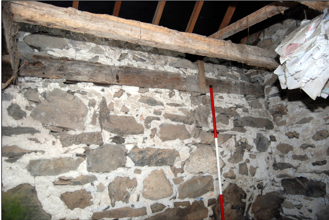
Plate 18: Rail in north wall
