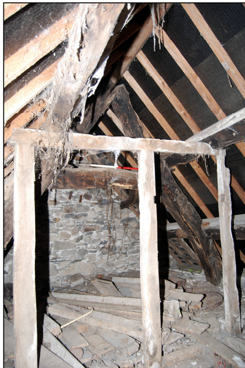
Plate 21: Joints in top of lateral beam
