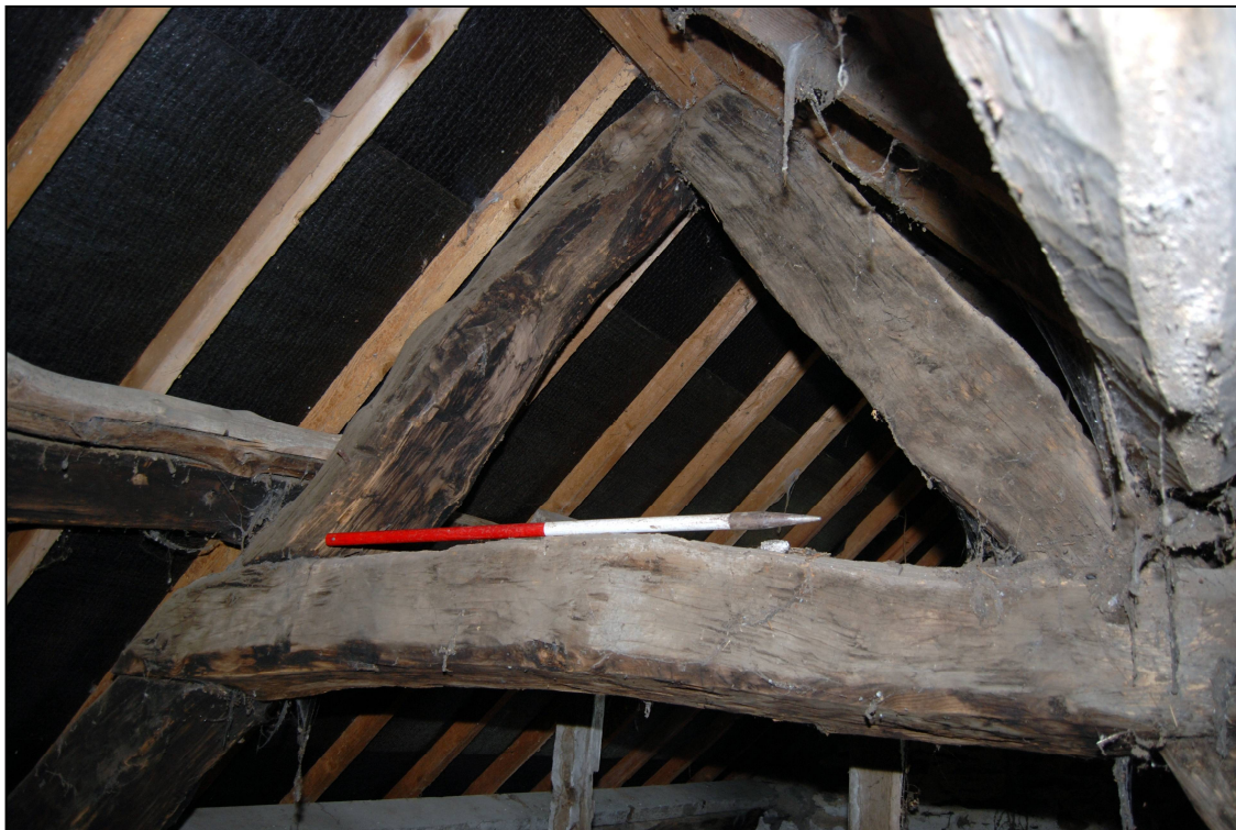
Plate 23: Apex of Truss 1, looking NE
