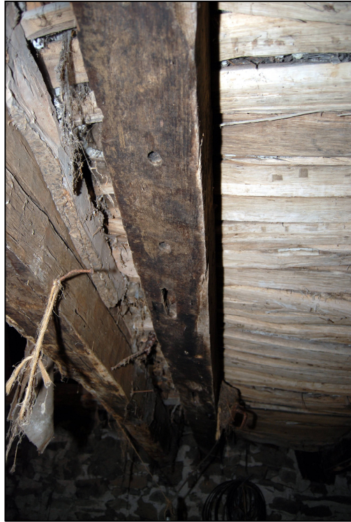
Plate 17: Evidence for the partition below Beam 4
