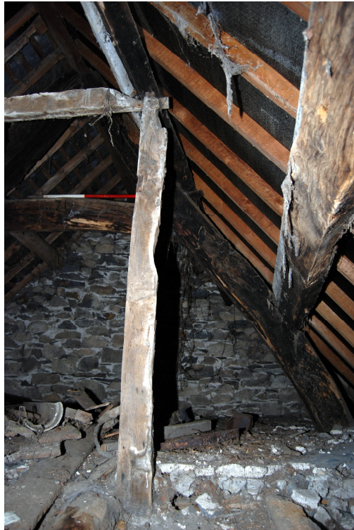
Plate 25: Detail of northern blade of Truss 1
