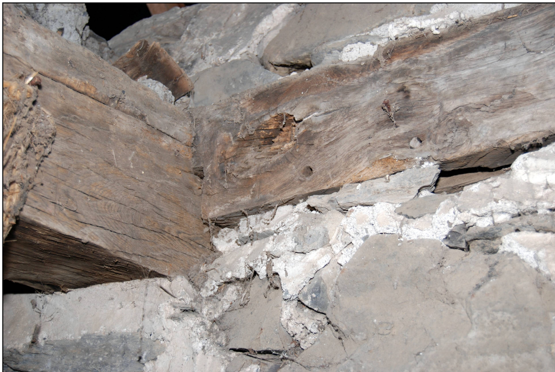
Plate 19: Joint between the rail and the platform
