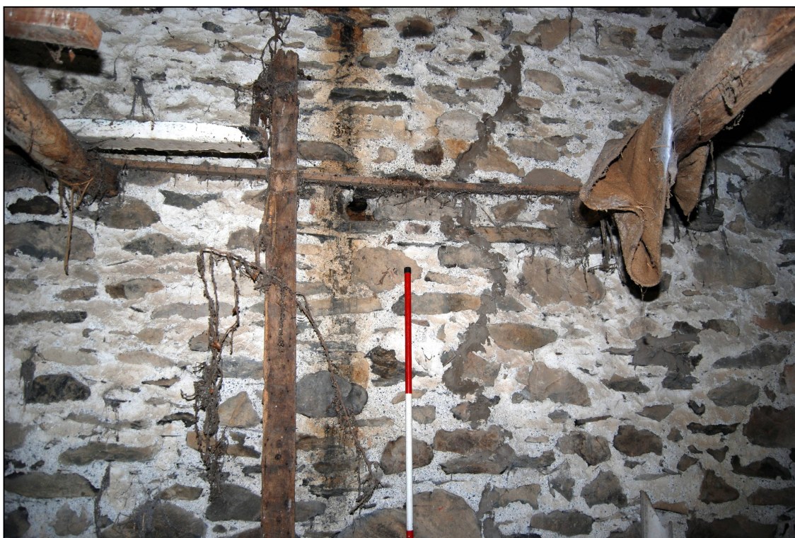
Plate 20: Lateral beams and socket for missing support
