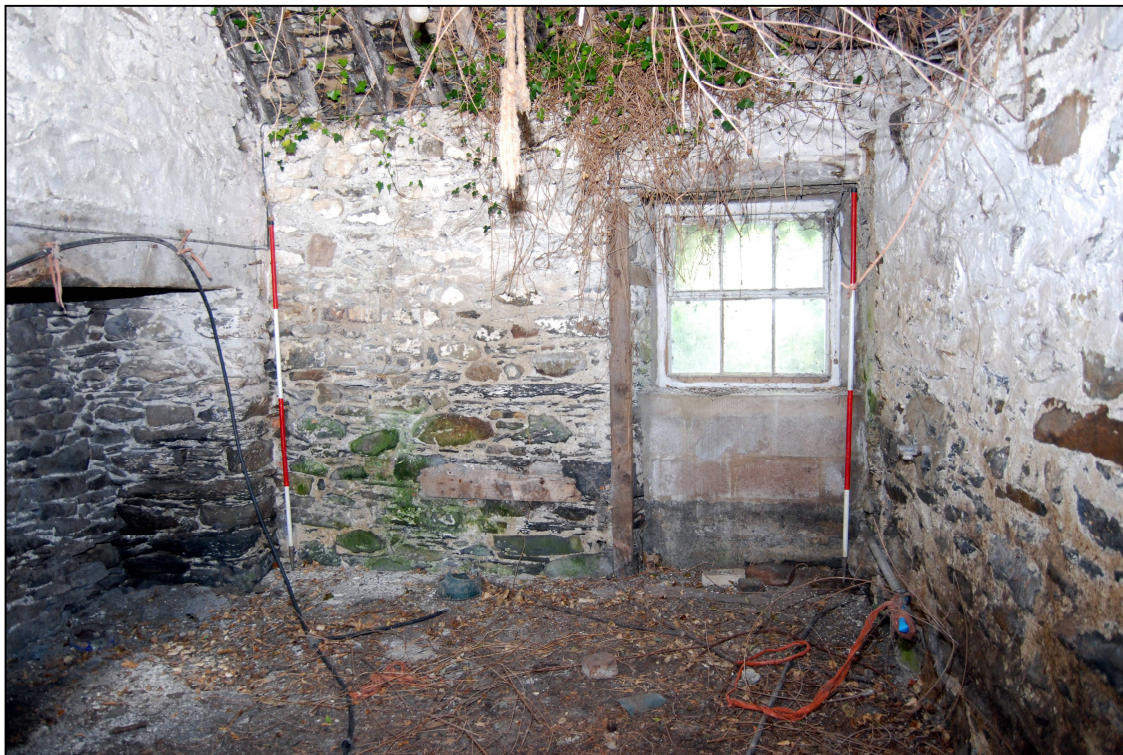
Plate 7: Window in north eastern corner of the building.
