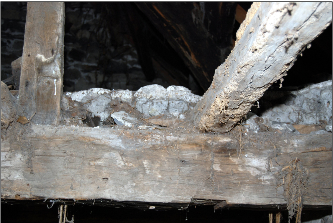
Plate 16: Plaster surface of the platform
