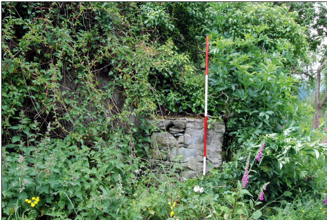
Plate 6: Stub wall on north eastern end of building
