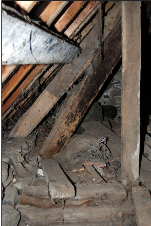
Plate 26: Detail of southern blade of Truss 1
