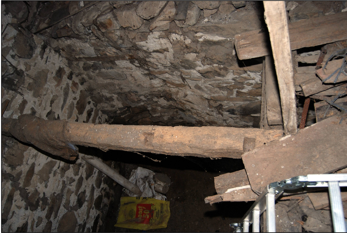
Plate 21: Joints in top of lateral beam
