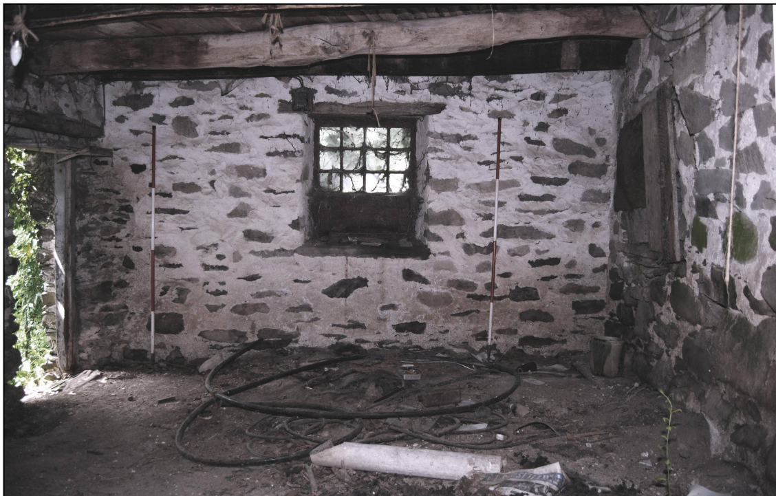
Plate 10: Western room looking west
