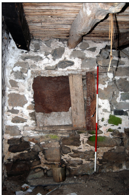
Plate 12: Blocked opening in western room, looking north
