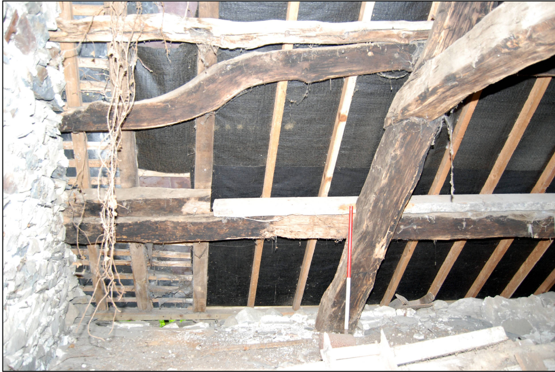
Plate 27: The western end of the northern purlins
