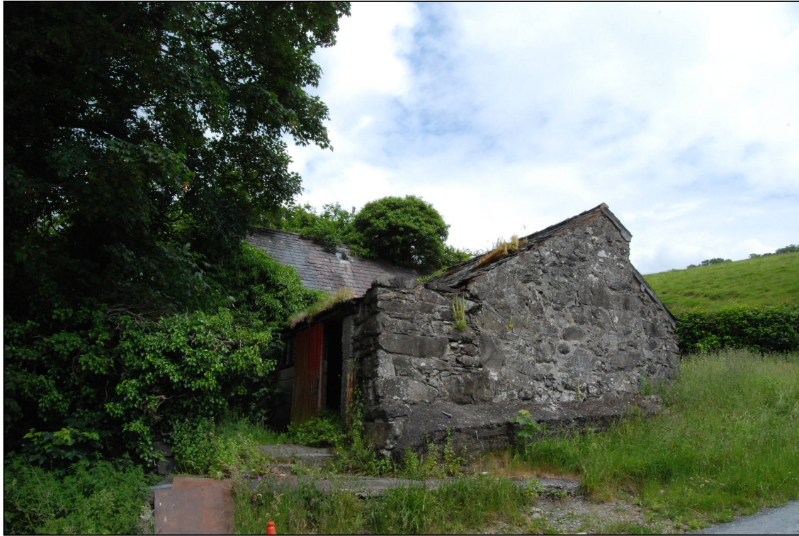
Plate 5: Old house looking NE showing, later, attached agricultural buildings
