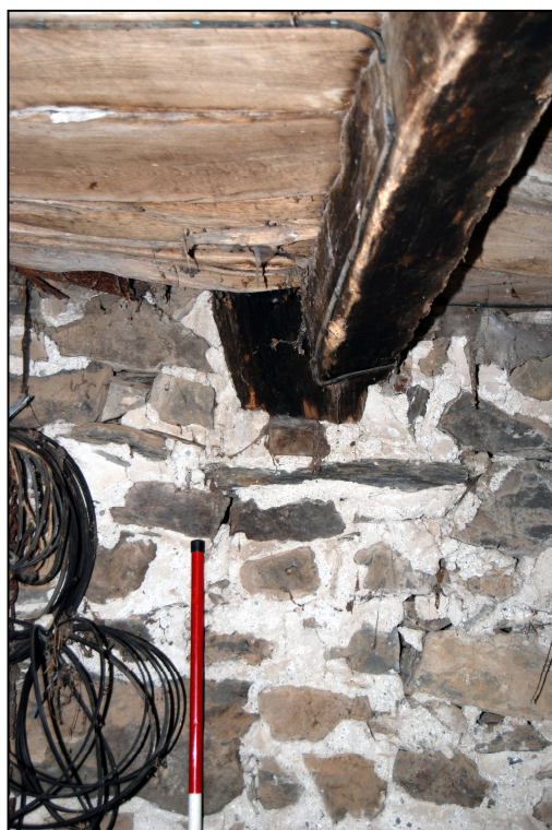
Plate 24: Foot of Truss 1 in southern wall of building
