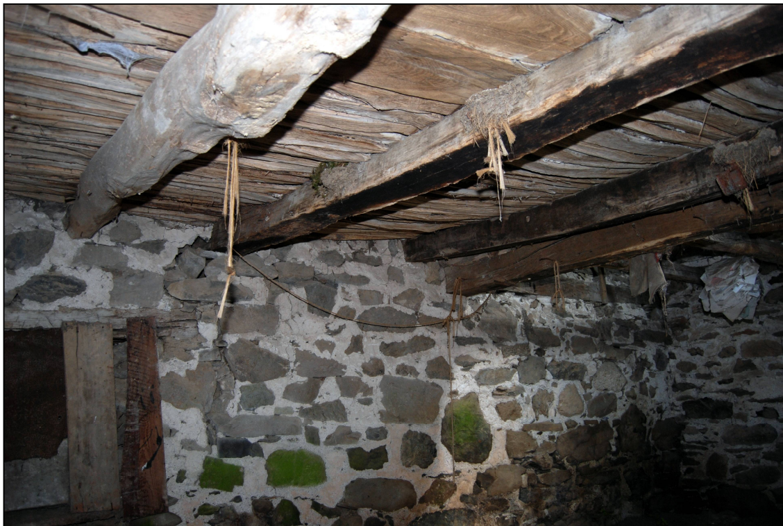
Plate 14: Beams supporting the platform, Beam 2 in the foreground
