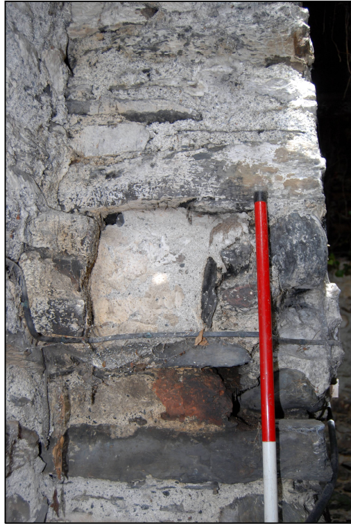
Plate 29: Blocked opening on the southern side of the chimney breast
