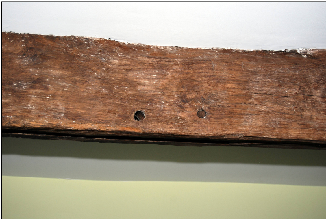
Plate 20: Peg hole in the beam in the parlour
