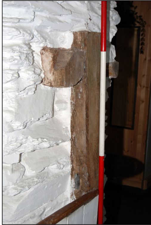
Plate 29: Timbers embedded in the northern wall of the landing
