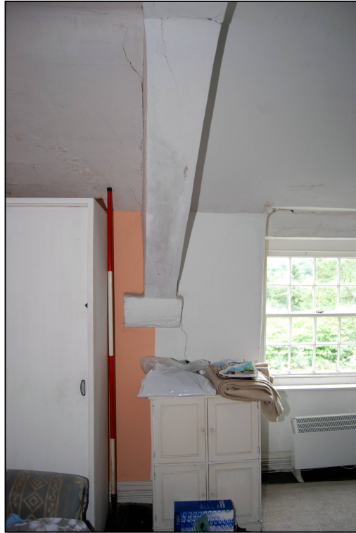
Plate 31: The eastern foot of Truss 1
