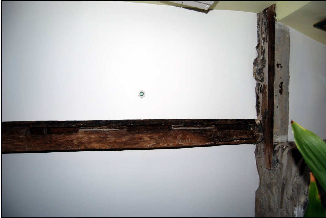
Plate 19: The sockets for the plank and muntin partition below the beam in the parlour
