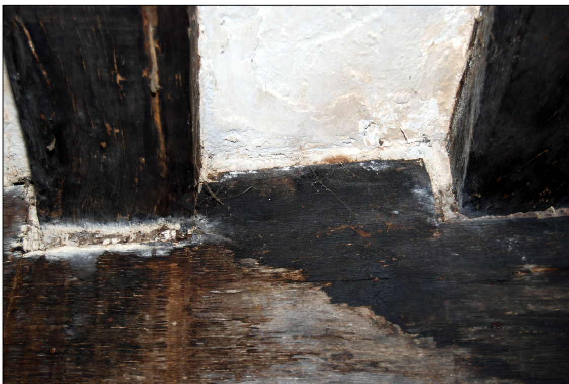
Plate 24: The chamfer and stop on the joists in the hall
