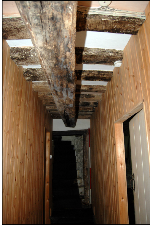
Plate 15: Beam in the cross passage looking west
