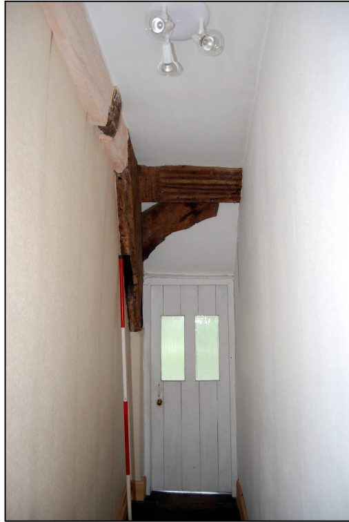
Plate 35: Eastern base of Truss 2
