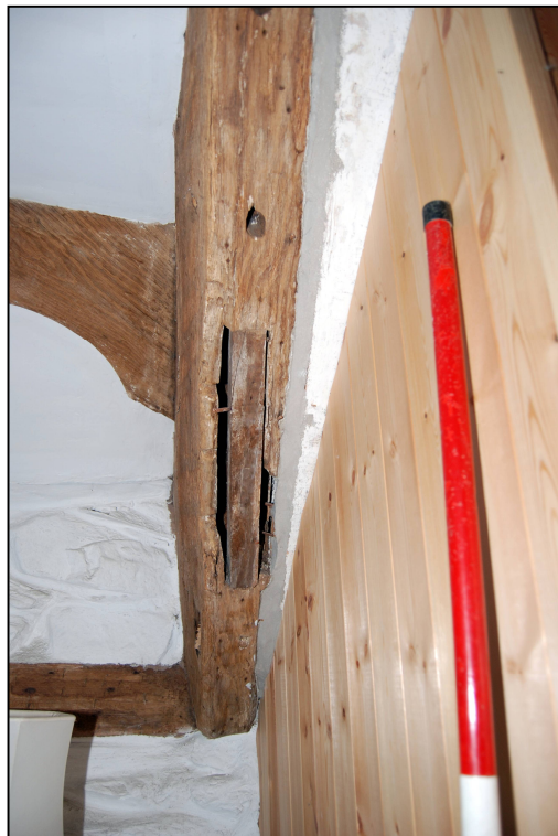
Plate 34: Socket for the tie beam at the western end of Truss 2
