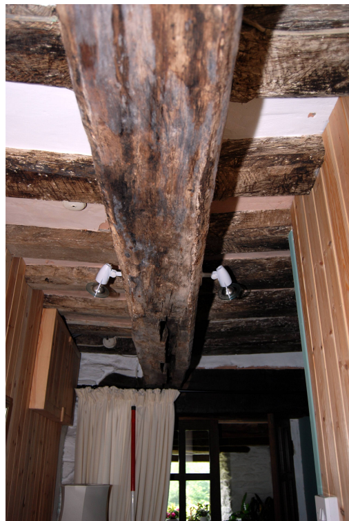
Plate 16: Beam in the cross passage looking east
