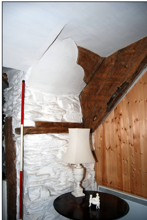
Plate 32: Western end of Truss 2 on the landing
