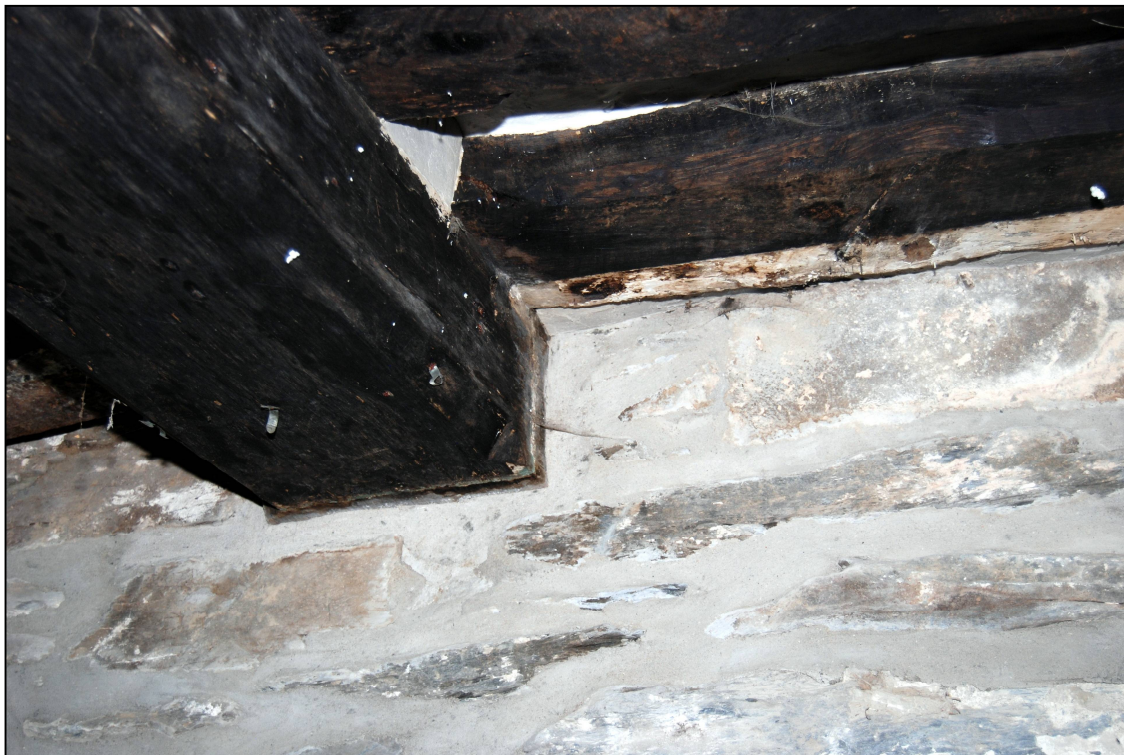
Plate 23: The chamfer and stop on the cross beam in the hall
