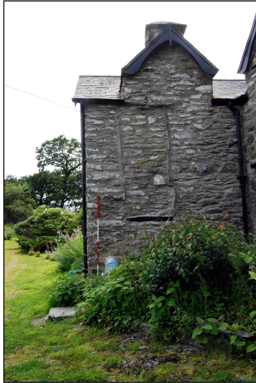
Plate 5: Northern elevation of the porch
