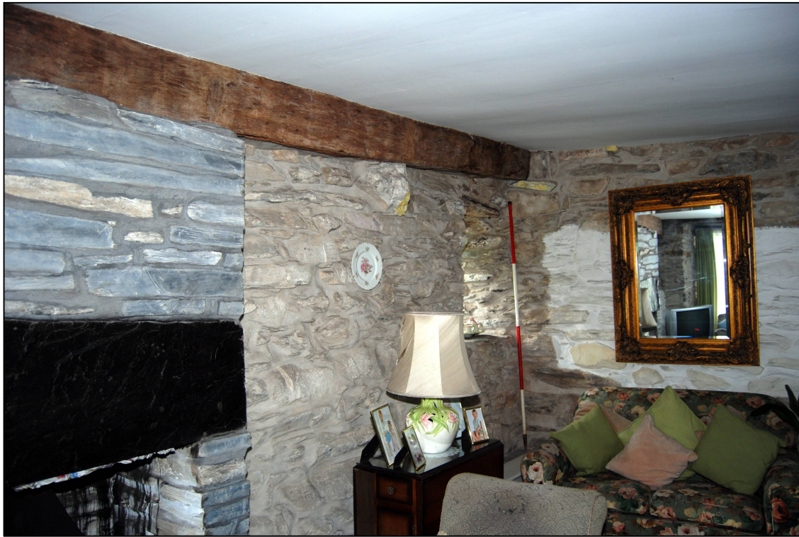
Plate 21: Beam along the southern wall of the parlour
