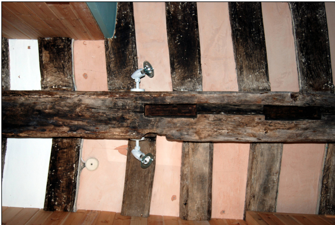
Plate 17: Socket for the plank and muntin partition in the cross passage
