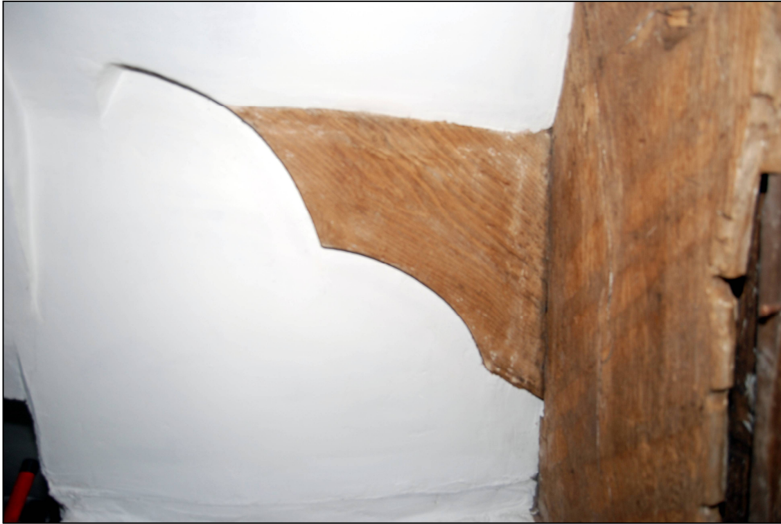
Plate 33: Cusped windbrace at western end of Truss 2 on the landing
