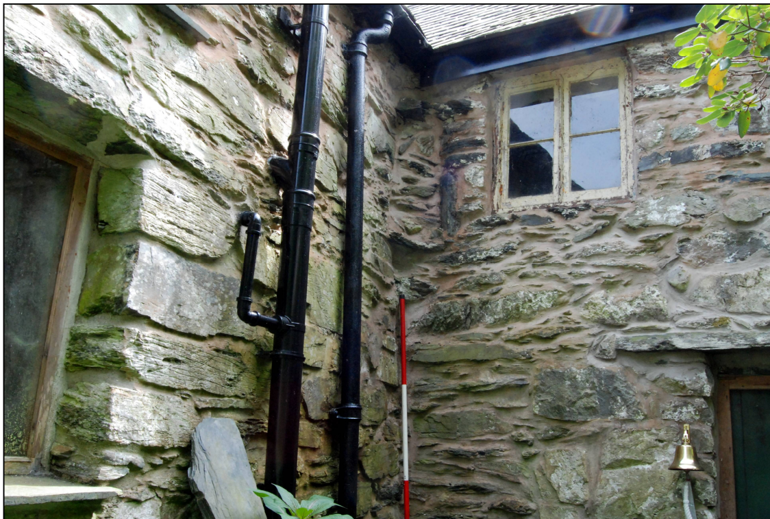
Plate 9: First floor, blocked opening between the kitchen range and the main house
