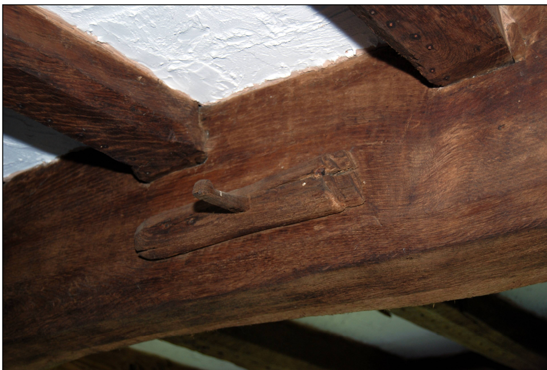
Plate 14: Wooden "hook" attached to the central beam in the porch
