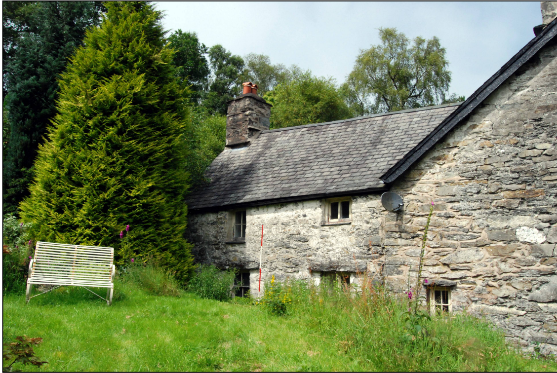
Plate 7: Southern elevation of the kitchen range
