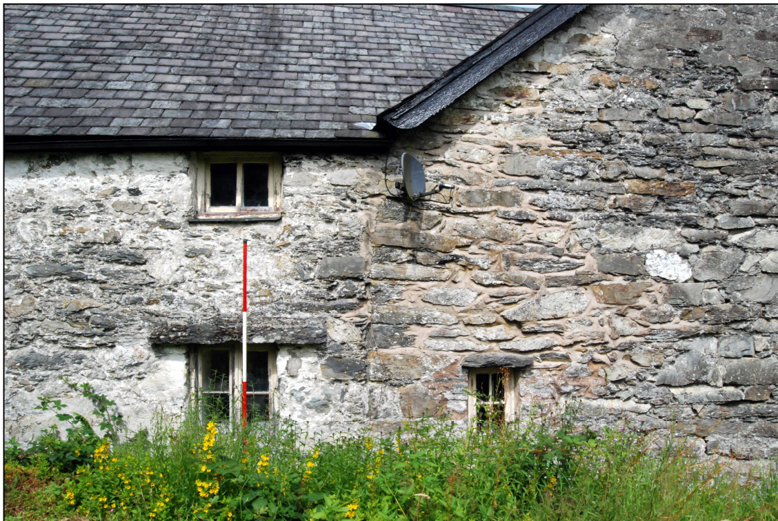
Plate 6: The junction between the main house and the kitchen range on the southern elevation
