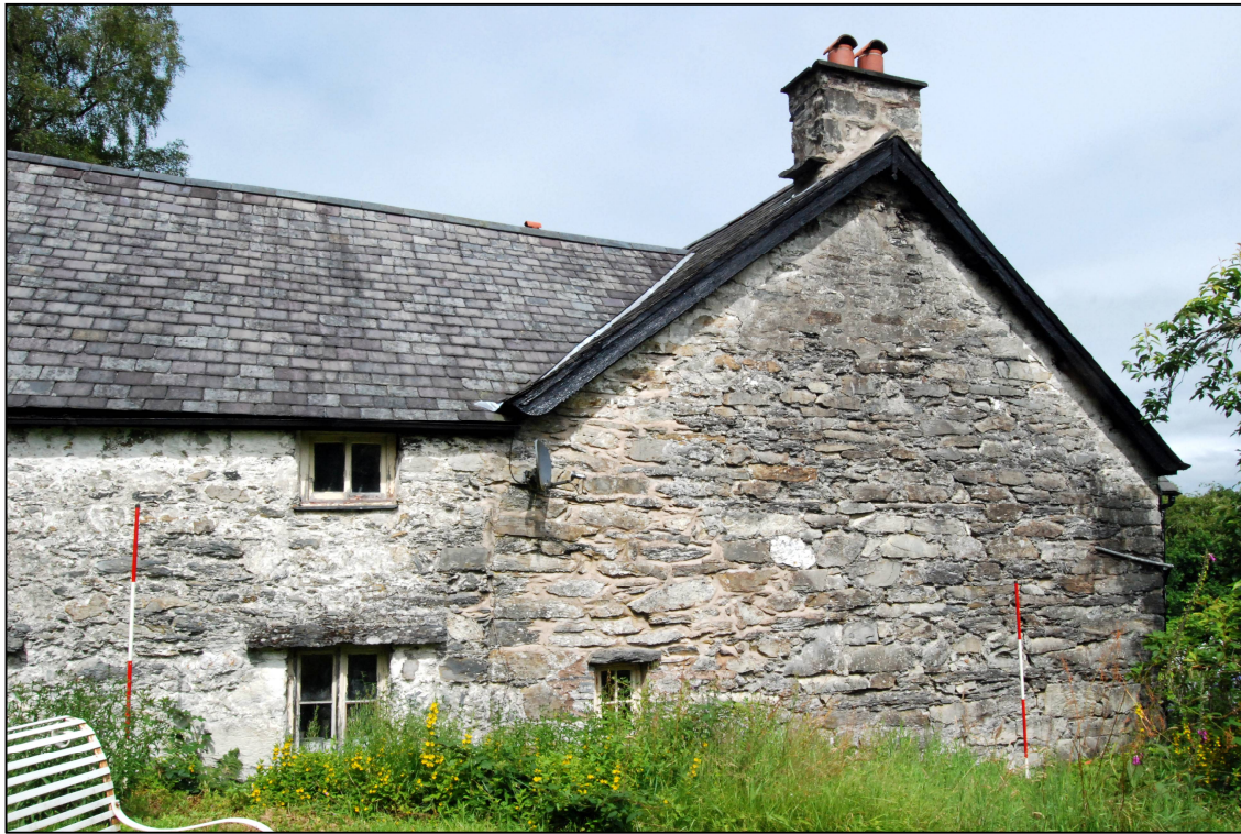
Plate 3: Southern gable end
