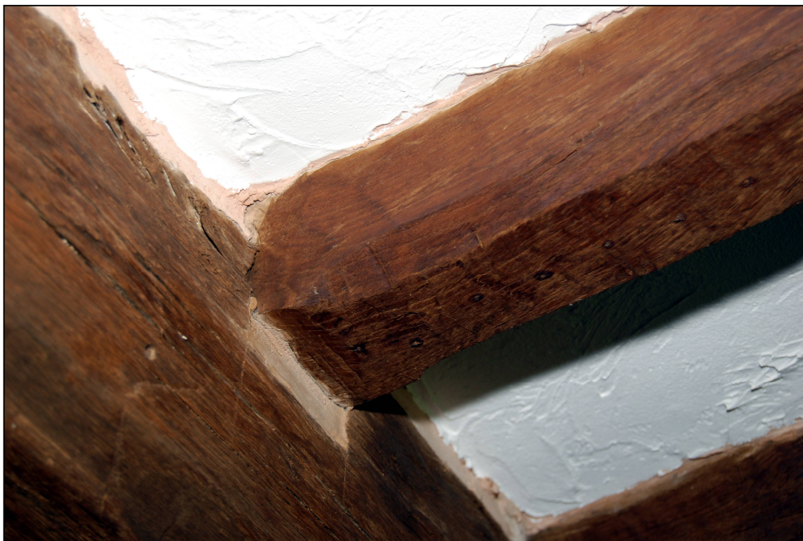
Plate 12: Chamfering and straight cut stop on a joist in the porch
