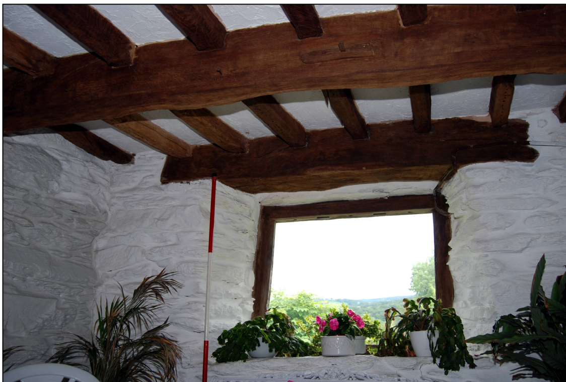
Plate 10: Ground floor of the porch, looking east
