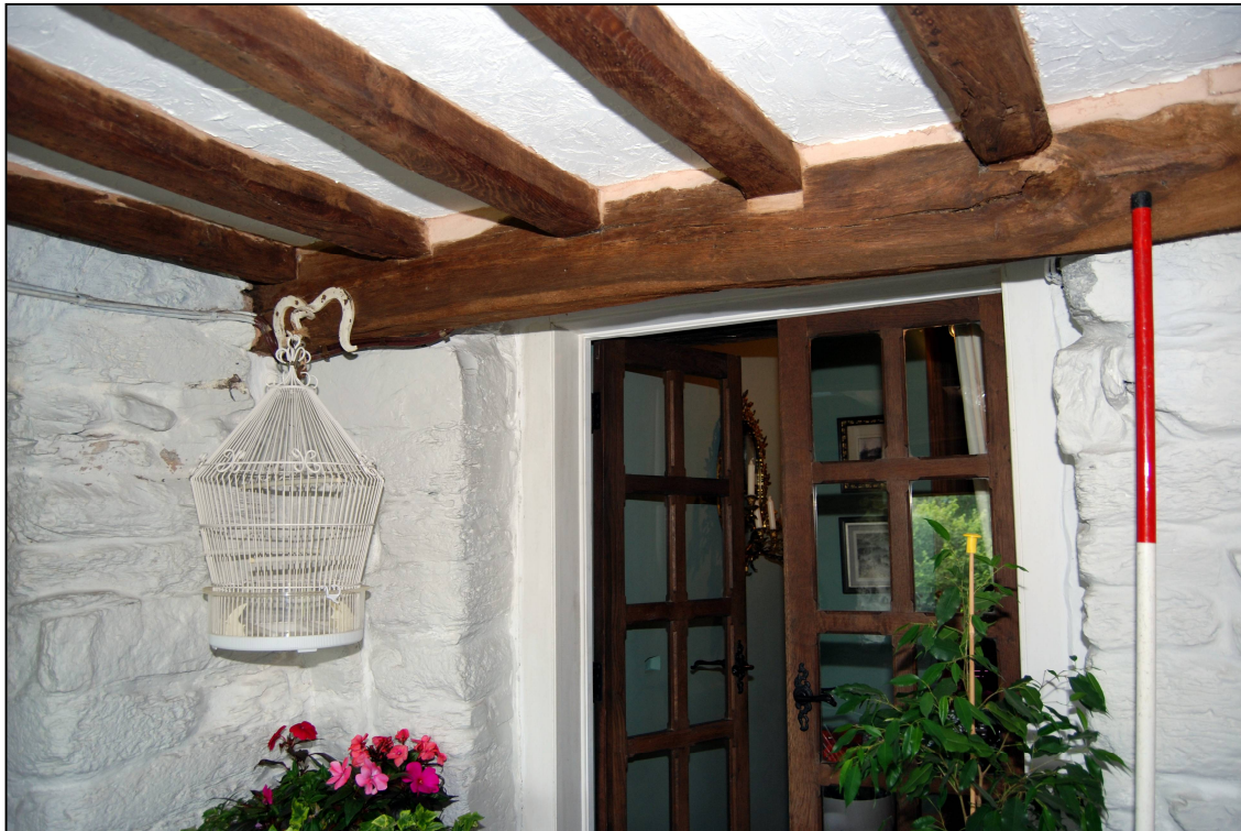
Plate 11: Ground floor of the porch looking west
