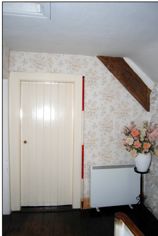
Plate 28: Base of Truss 5, exposed on the landing
