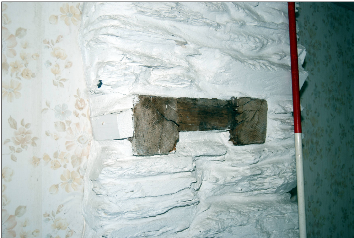
Plate 30: Timbers embedded in the southern wall of the landing
