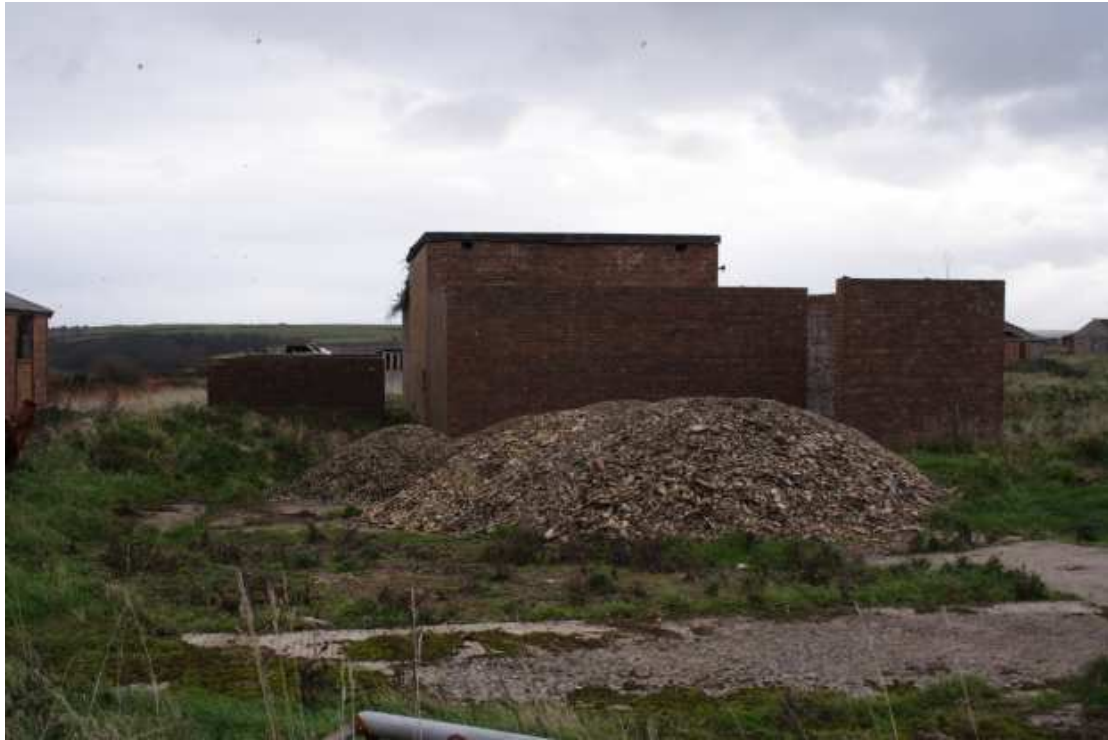
Photo 21 (685). Generator House 29581. View E
