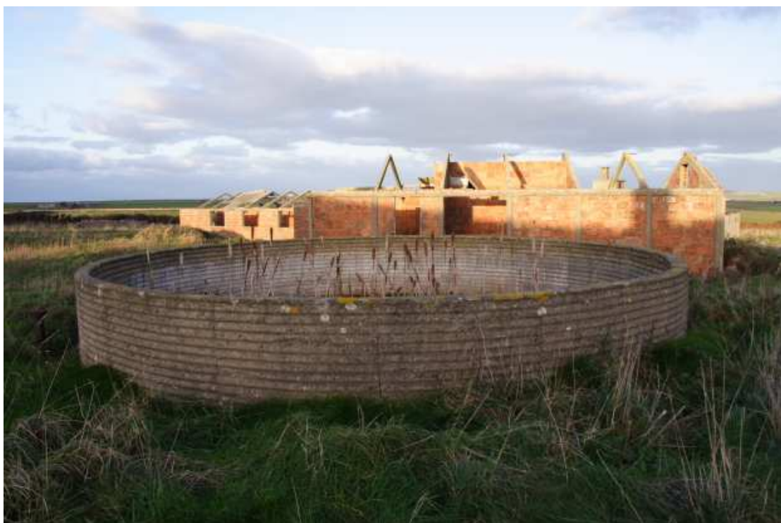
Photo 20 (668). Water Tank 28580. View NE
