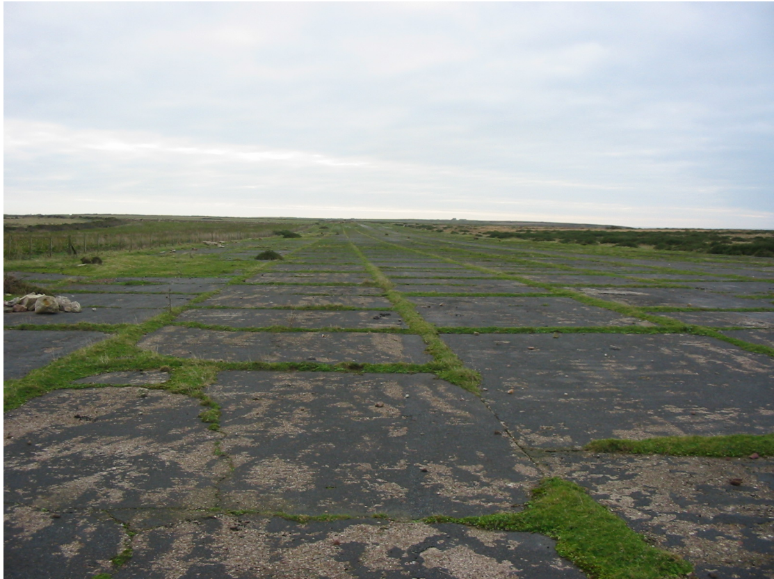
Photo 43 (2351) Runway from main cross over. View SSE
