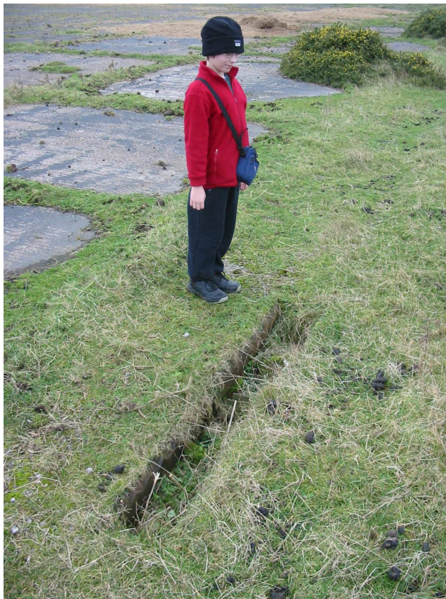
Photo 44 (2355). Example of main runway drains.
