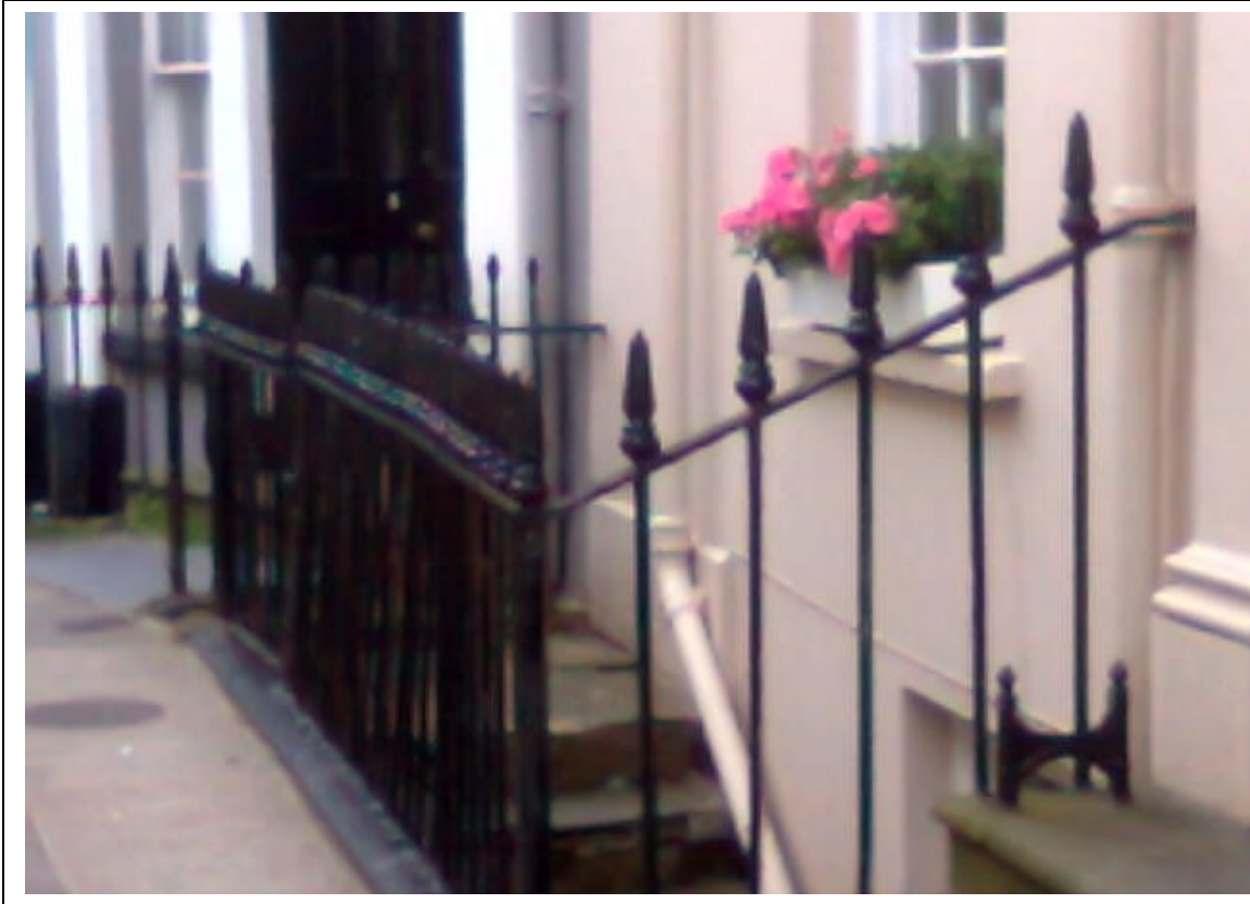
1,2 and 3 Rock House, St Julian Street
