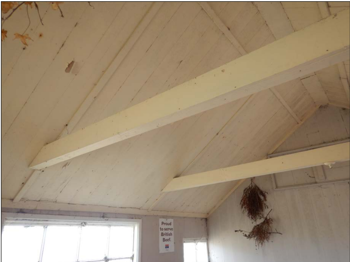
25. Detail of roof trusses.
