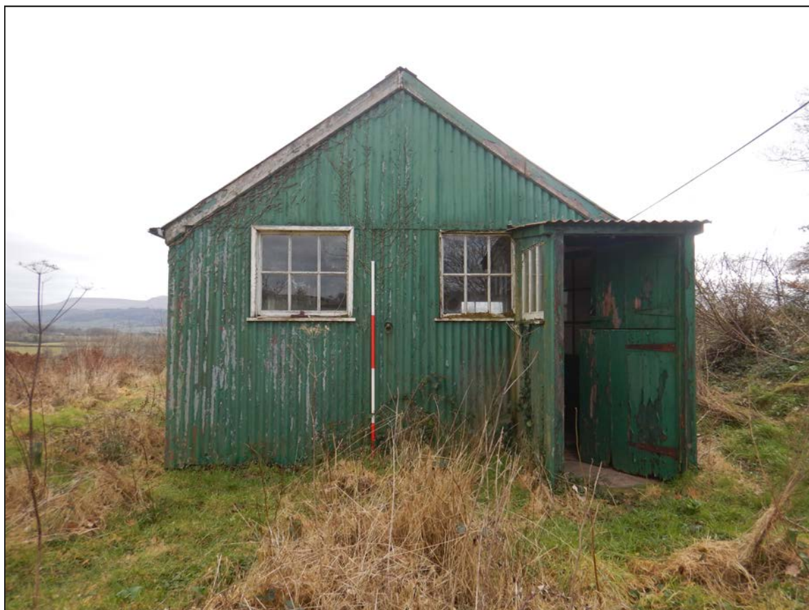
8. View of W facing elevation, looking E.
