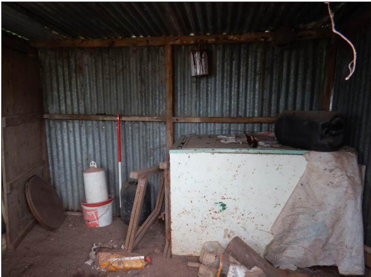
31. View into shed looking S.
