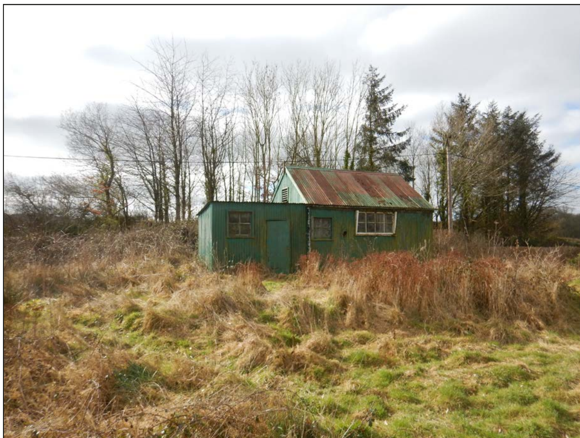
14. View of W facing elevation. looking E.
