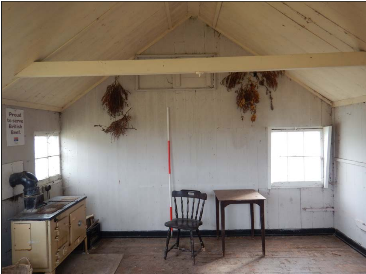
18. View of interior looking E.
