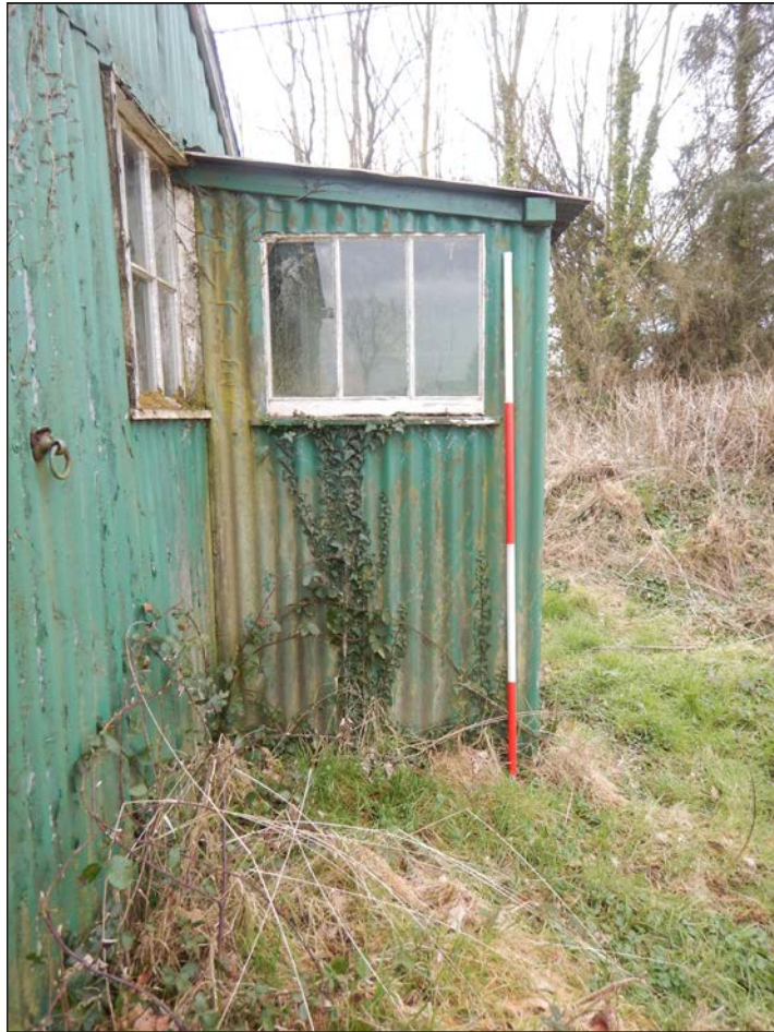
3. Porch S facing elevation, looking N.
