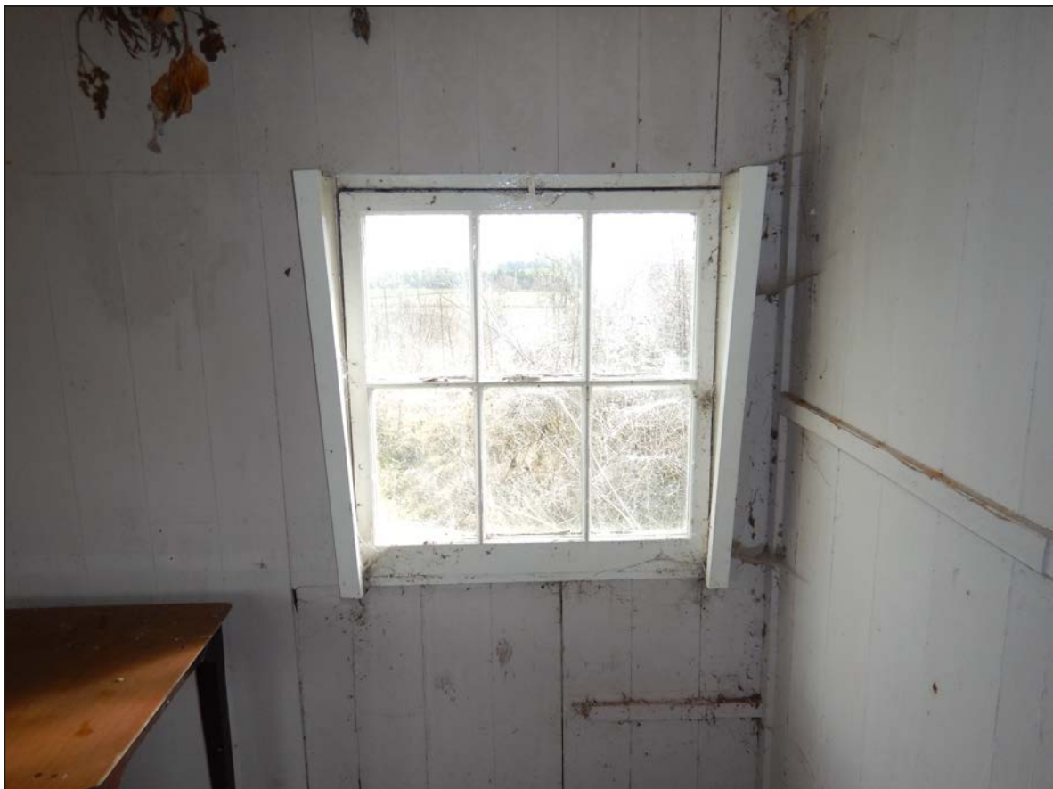
19. Close-up, interior looking E.
