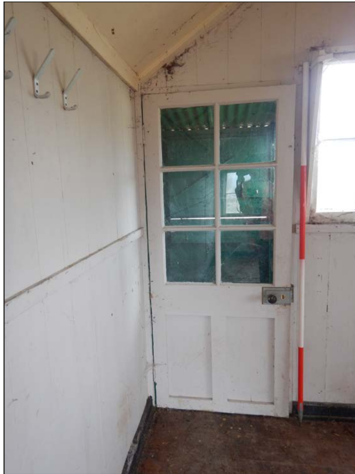
22. Door detail, E elevation looking W.
