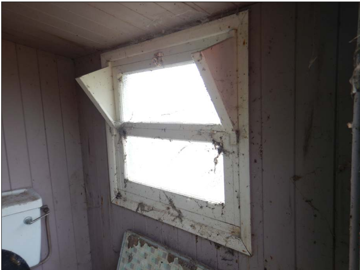
29. View of window, toilet block looking W.
