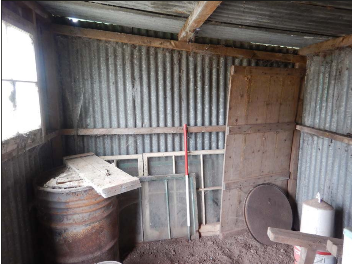
30. View into shed looking E.
