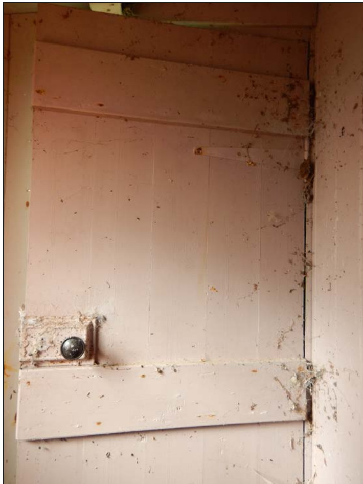
28. View of toilet block door - looking SE.
