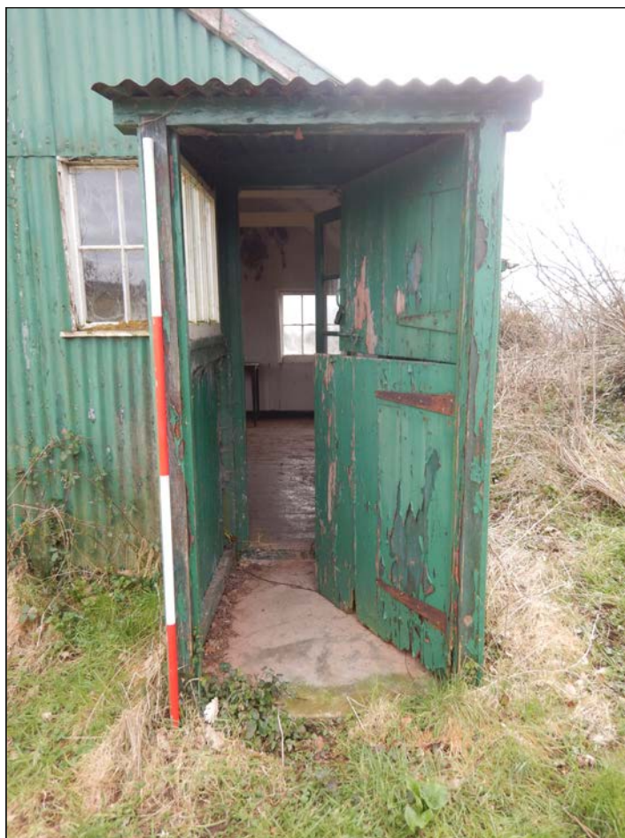
7. Detail of entrance, W facing elevation looking E.
