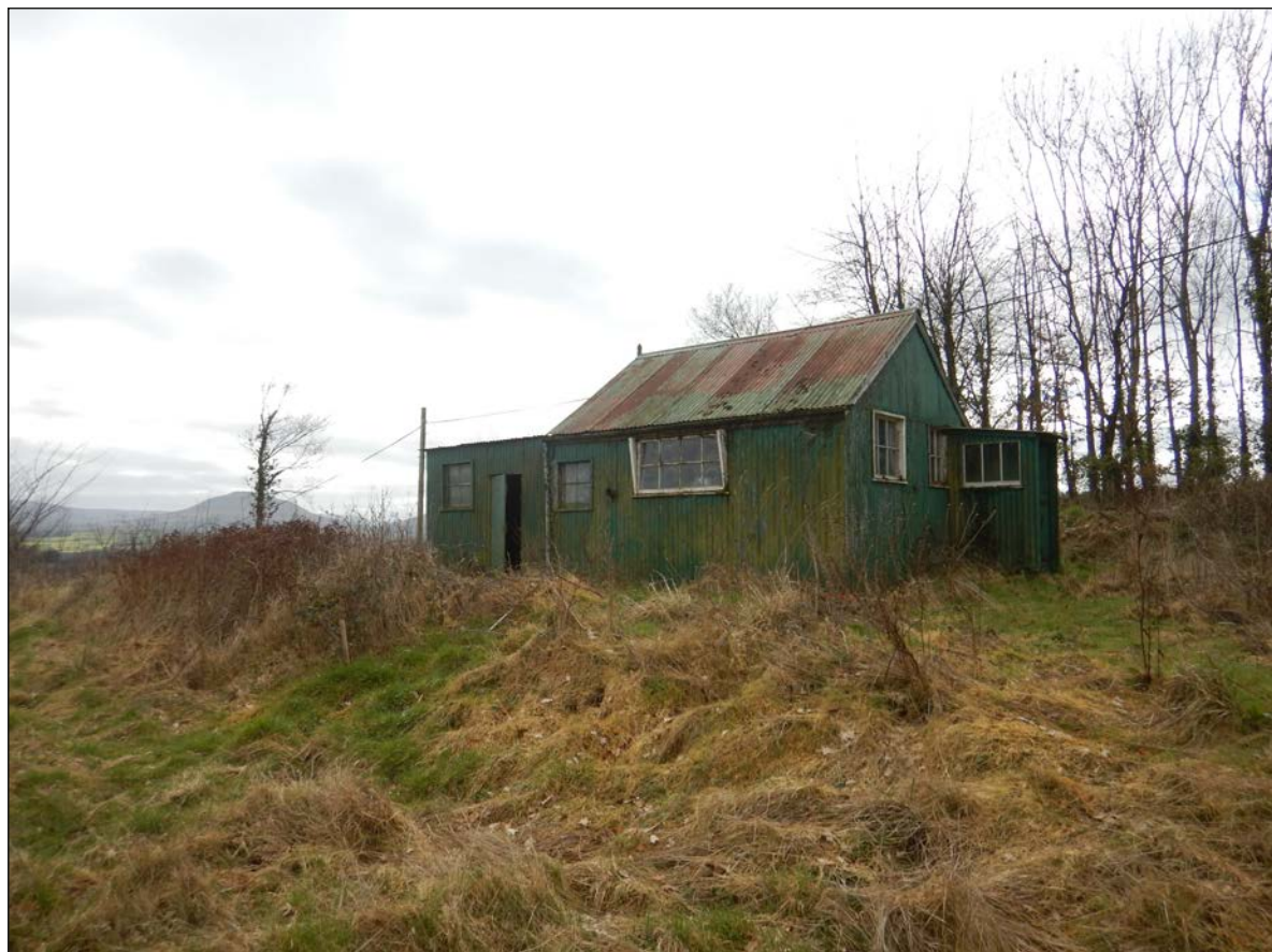
2. View of N elevation, oblique.
