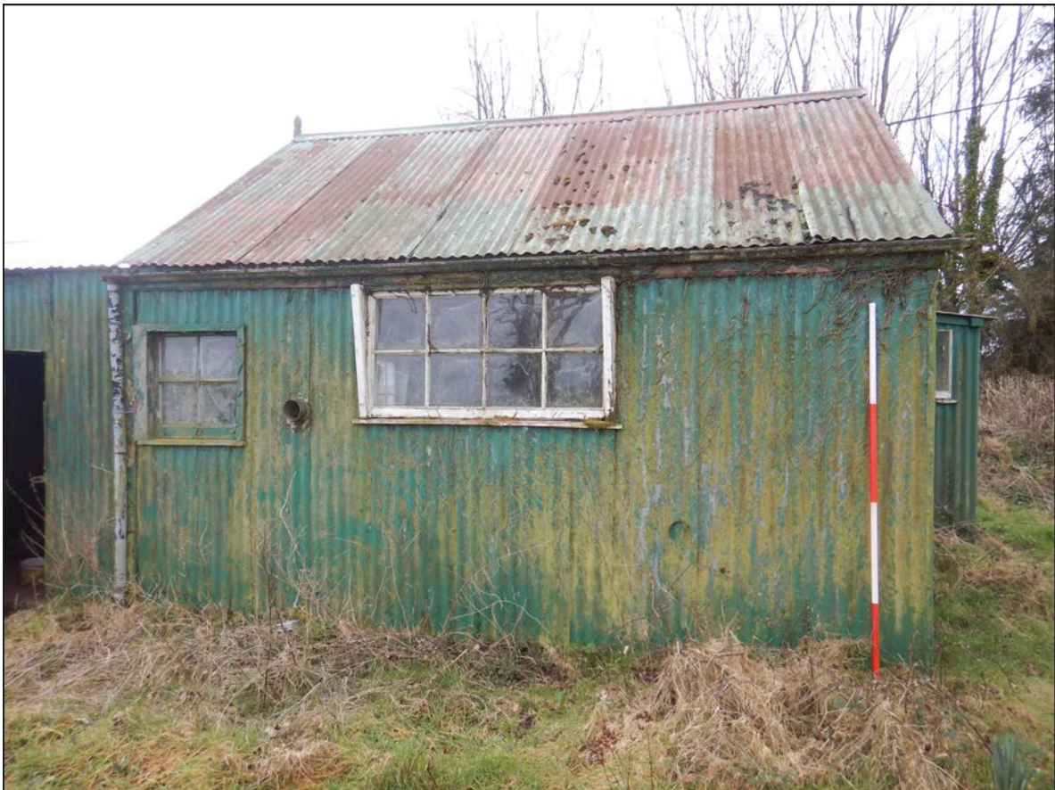
4. Close-up view of S facing elevation, looking N.
