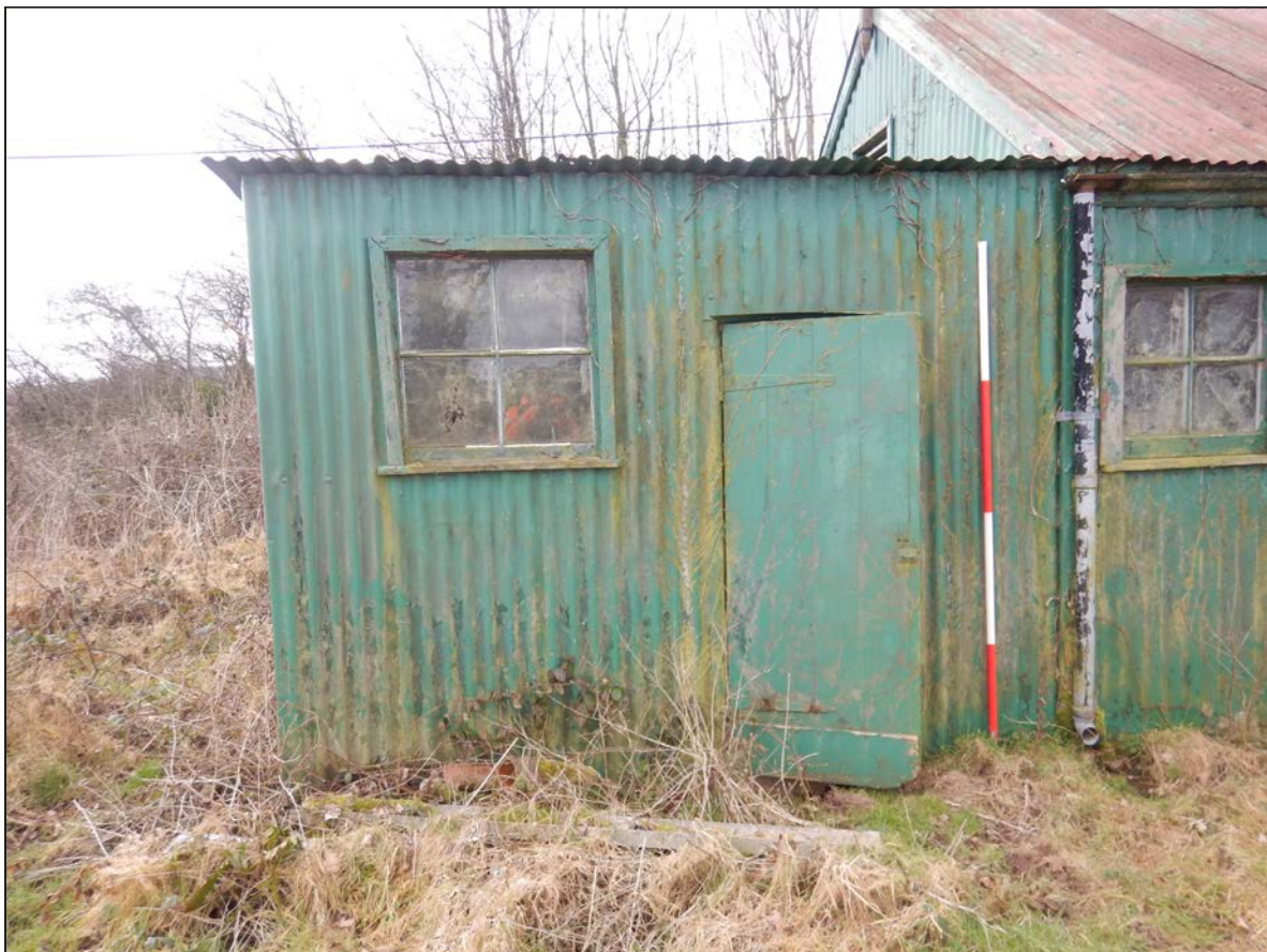
6. View of E extension, looking S.
