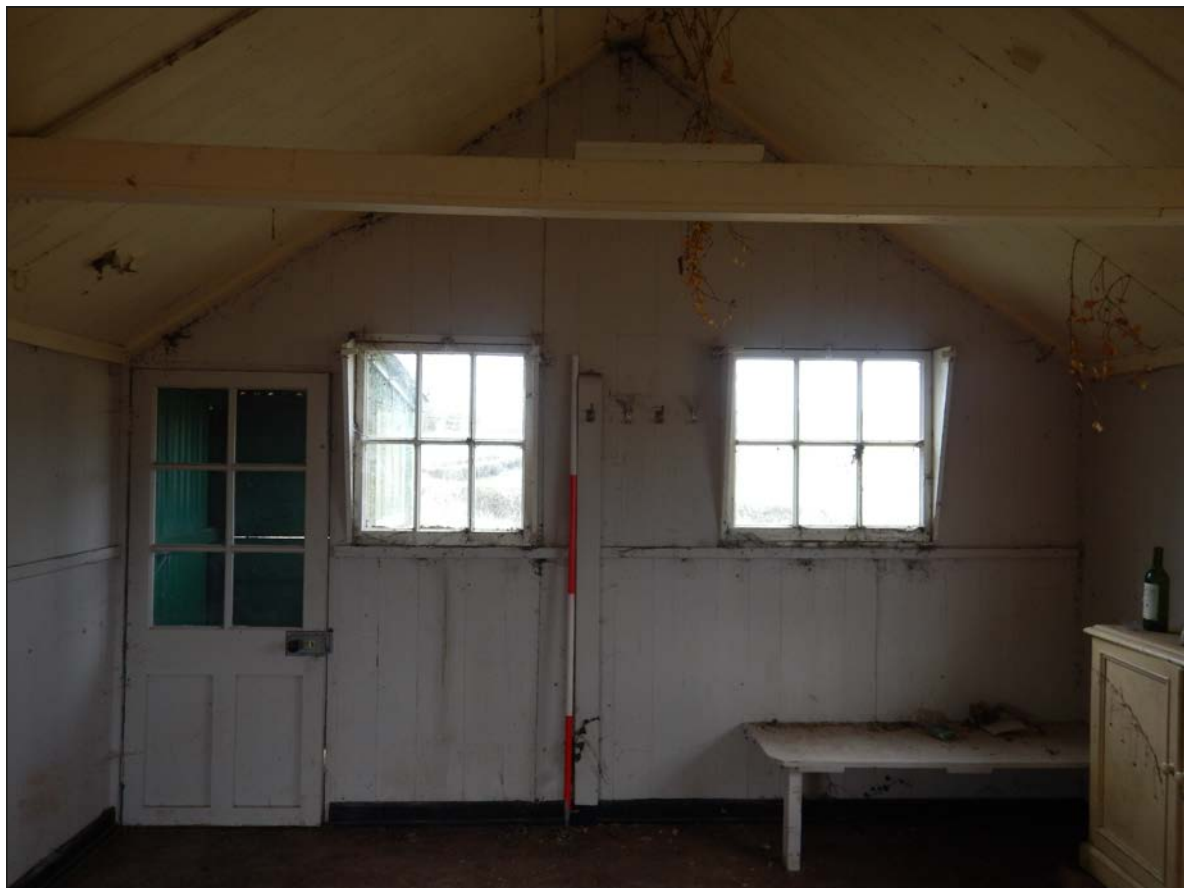
23. View of E facing elevation looking W.
