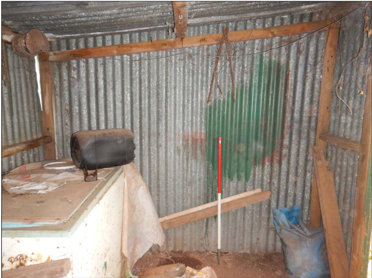
32. View into shed looking W.
