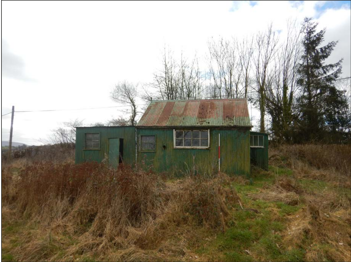
1. View of N facing elevation, looking S.
