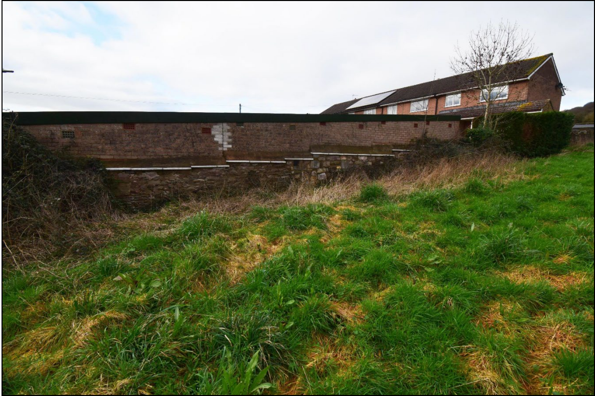
Plate 23 - TRW2024_023: A view of the rear of the Tudor Road garages along the west boundary of the proposed development site. The stone wall contains some fragments of the Tudor House garden wall (ID number 18). The garage will be removed for the development. Looking west-northwest.
