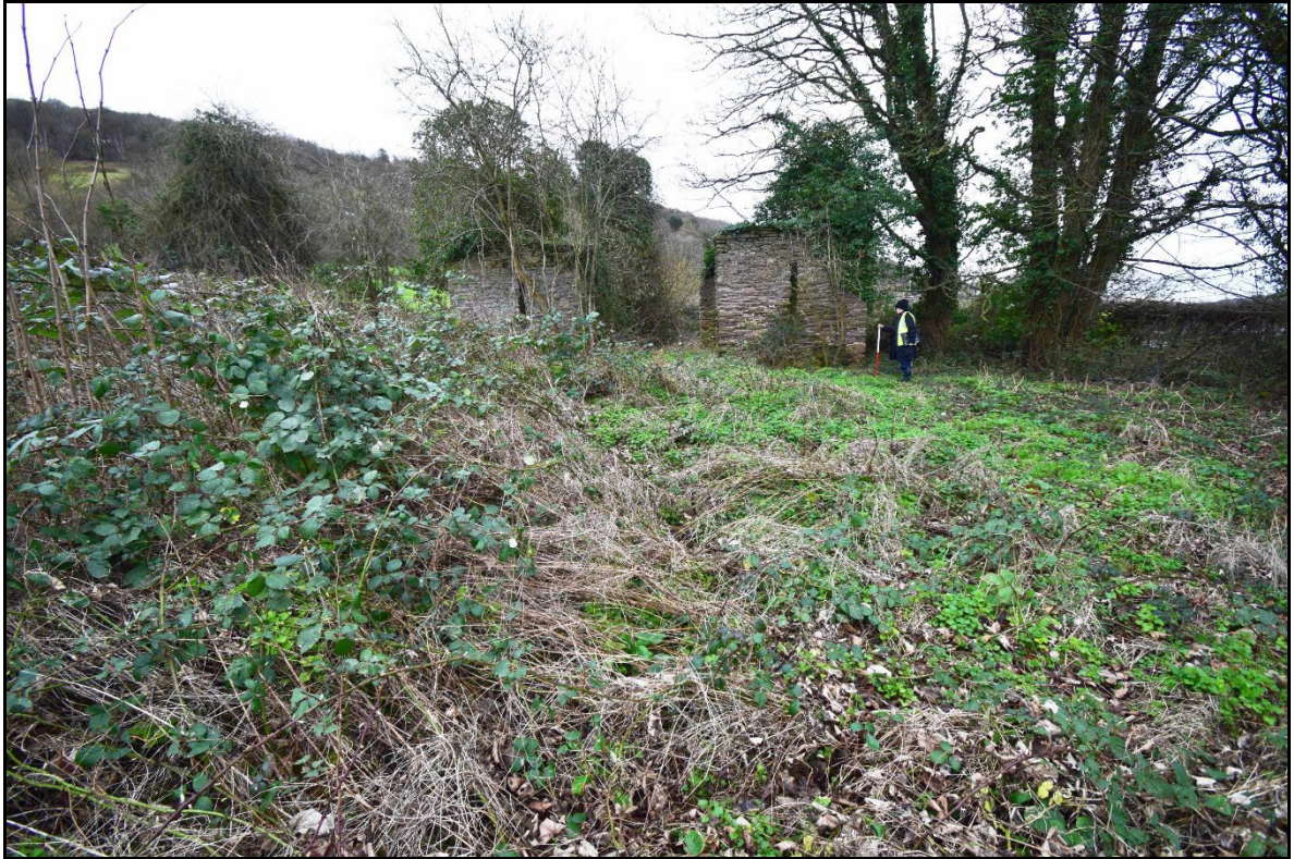
Plate 6 - TRW2024_006: A view of the now derelict barn (ID number 22) which once belonged to Tudor House. Mature deciduous trees are still present close to the building, on the south boundary of the proposed development site. Looking east.
