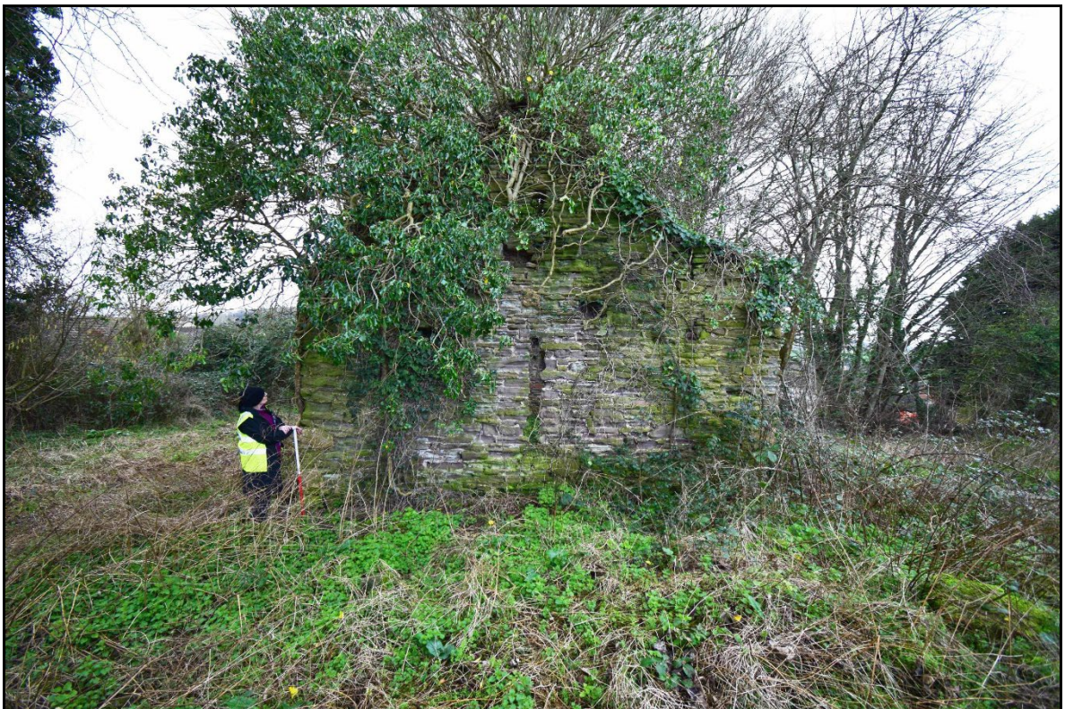
Plate 12 - TRW2024_012: A view of the northern gable wall of the now derelict barn (ID number 22). Looking south.
