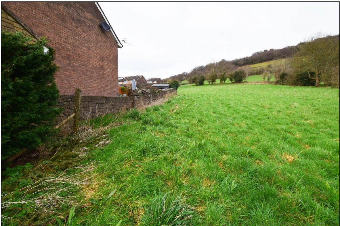
Plate 24 - TRW2024_024: A view along the western side of the proposed development site showing the preserved section of the Tudor House garden wall (ID number 18) left of centre. Looking north.
