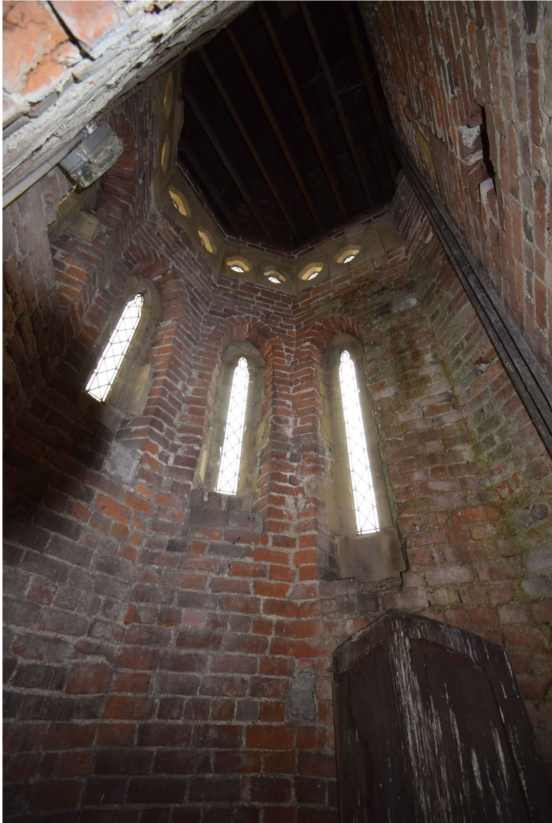
Plate 32: PSC2023_032, A view inside the "tower" at the north corner of the chapel. It seems that only the base was built initially, and the upper part of the tower was never added. Looking southeast.
