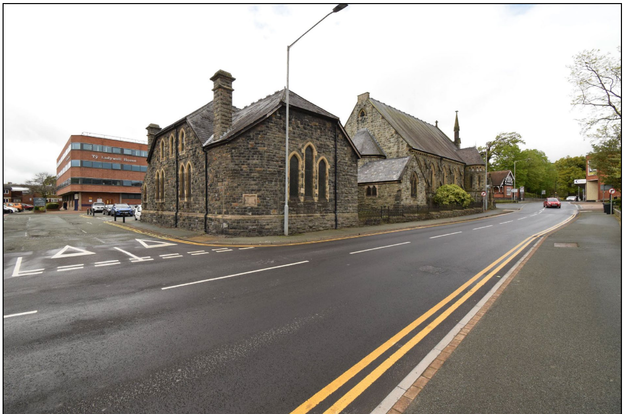
Plate 9: PSC2023_009, A view of the chapel and schoolroom from New Church Street. Looking west-northwest.
