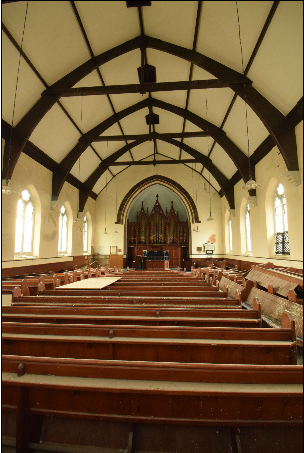
Plate 27: PSC2023_027, A view inside Park Street United Reform Chapel, looking towards the pulpit and pipe organ. Looking southeast.
