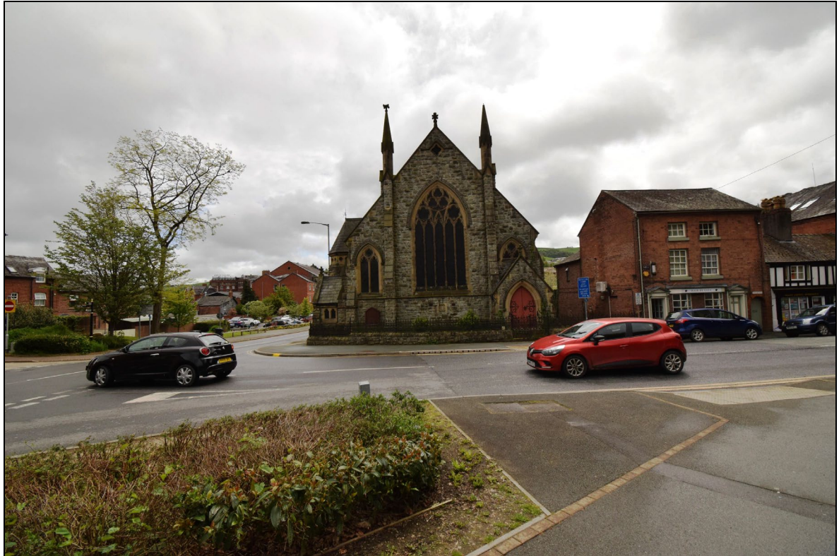
Plate 22: PCS2023_022, A view of Park Street United Reform Chapel, viewed from Park Street. Looking southeast.
