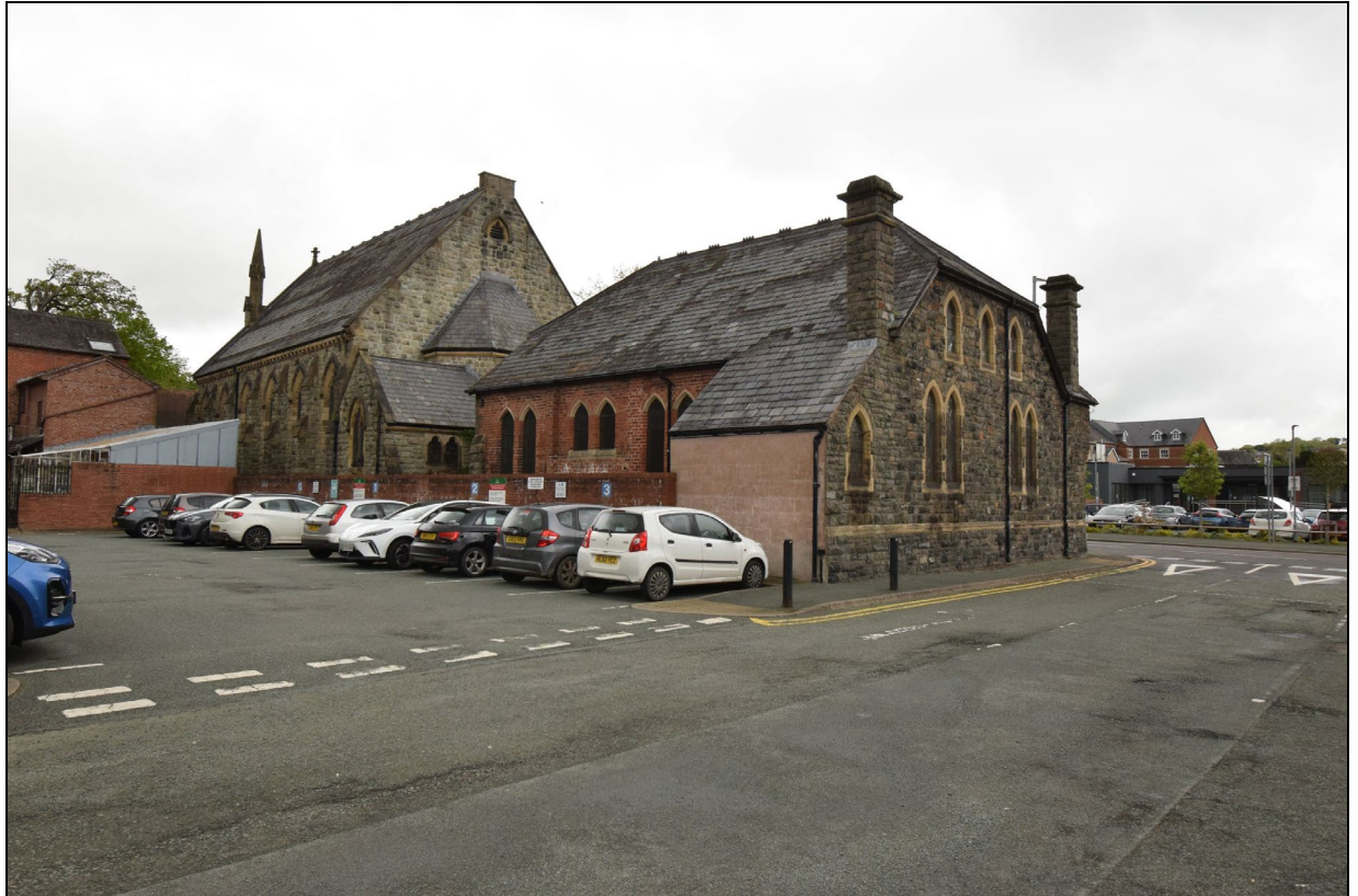
Plate 1: PSC2023_001, A view of Park Street Chapel (left) and its schoolroom (centre), viewed from New Road. Looking north.
