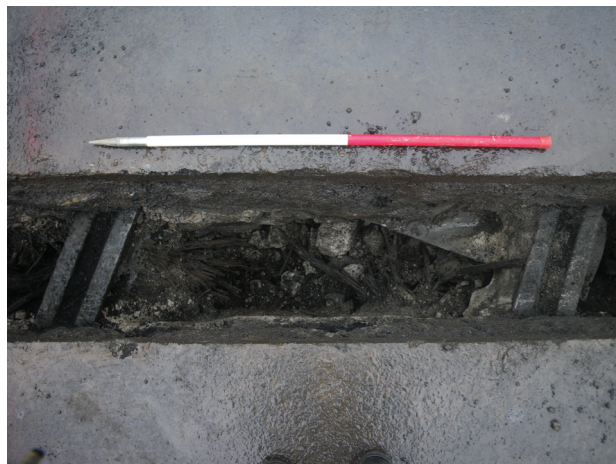
Rail track 4014, looking north-east
