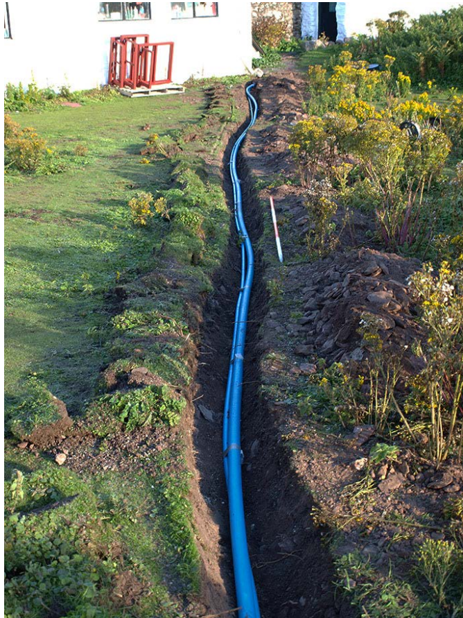
Pipe trench excavated to the west of the building complex
