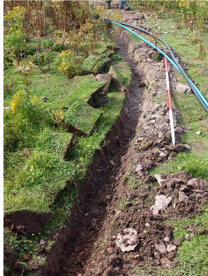
Pipe trench excavated to the east of the building complex
