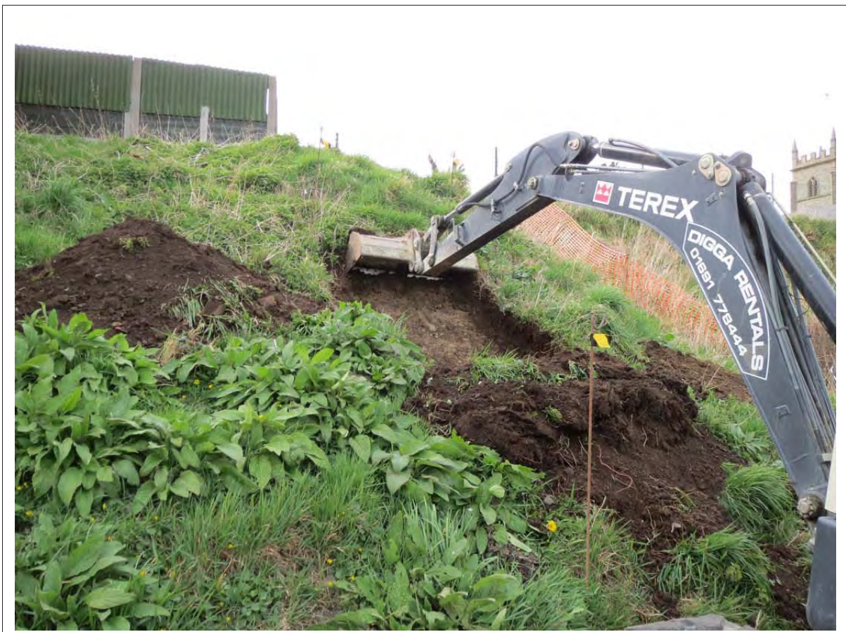
Plate 4: Working shot of excavation of trench 1. Looking west north west
