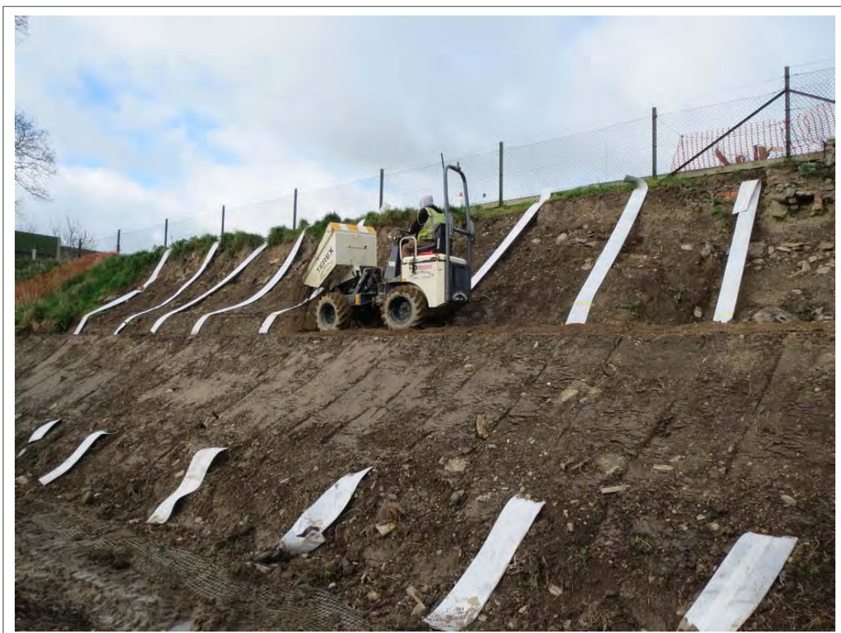
Plate 26. Working shot of the restoration work showing soil infill (over geo-textile strips pinned to the truncated bank). Looking South-South-West.
