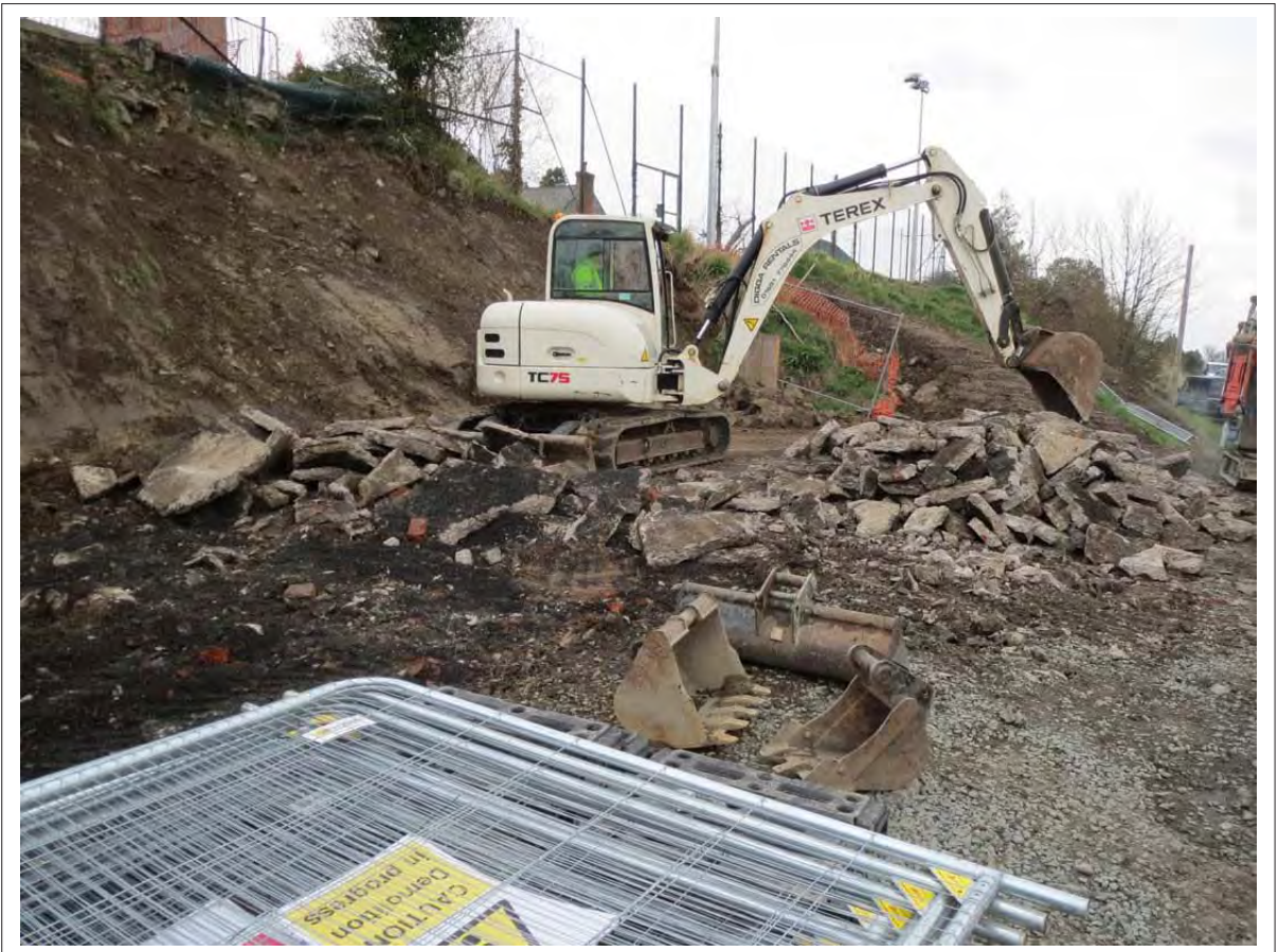
Plate 10. Removal of concrete slab at location of former garages. Looking North-North-West.
