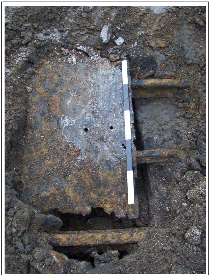
Plate 14: View of steel repairs to surface of culvert [105] Scale 1x1m
