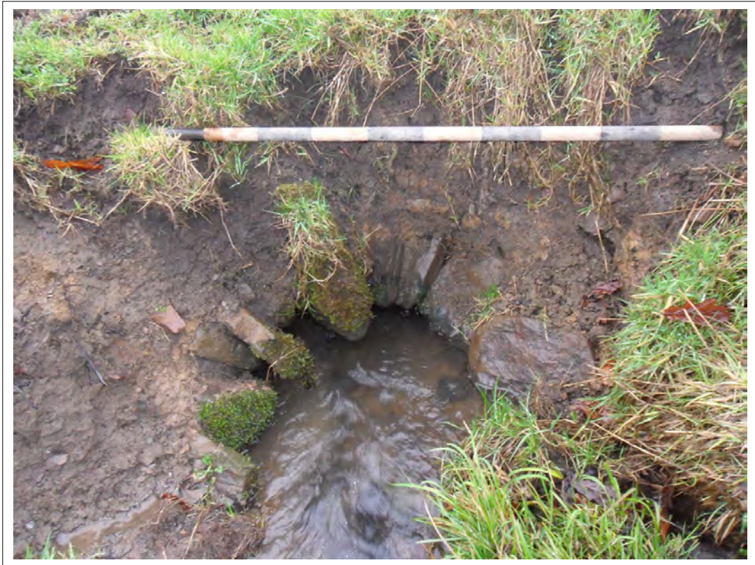
Plate 9: View of entrance to culvert [105], Looking north, Scale 1x1m
