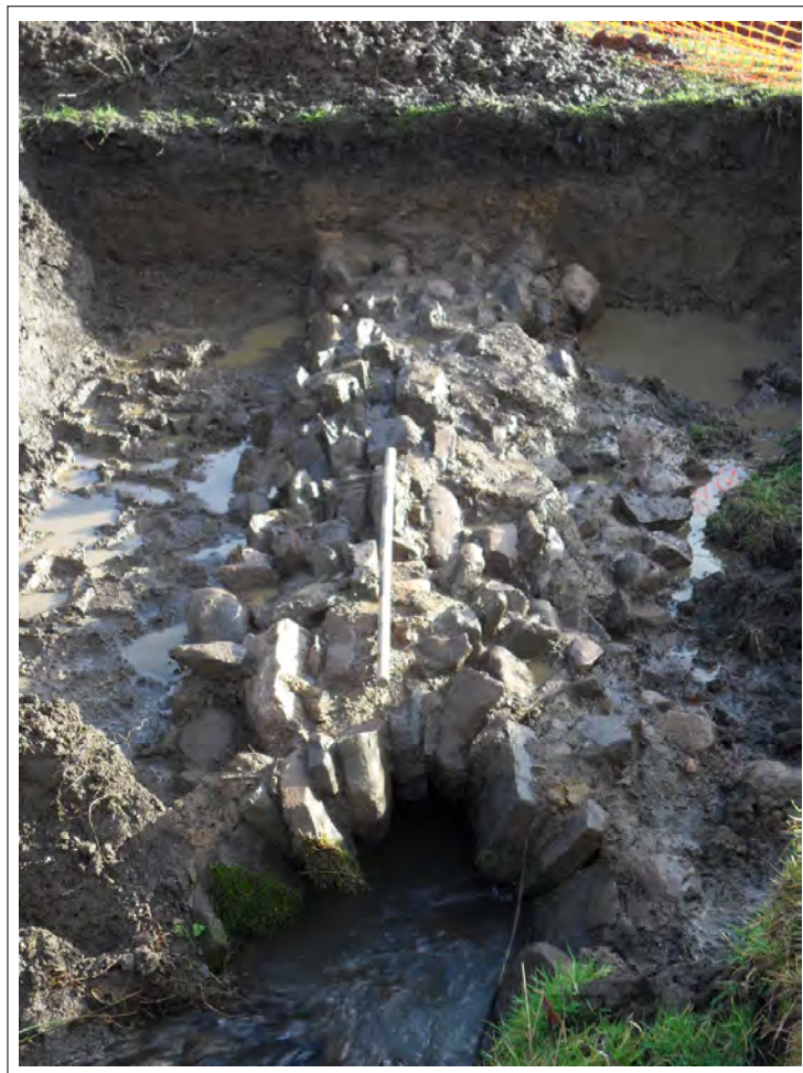
Plate 10: View of culvert [105] structure Looking north, Scale 1x1m
