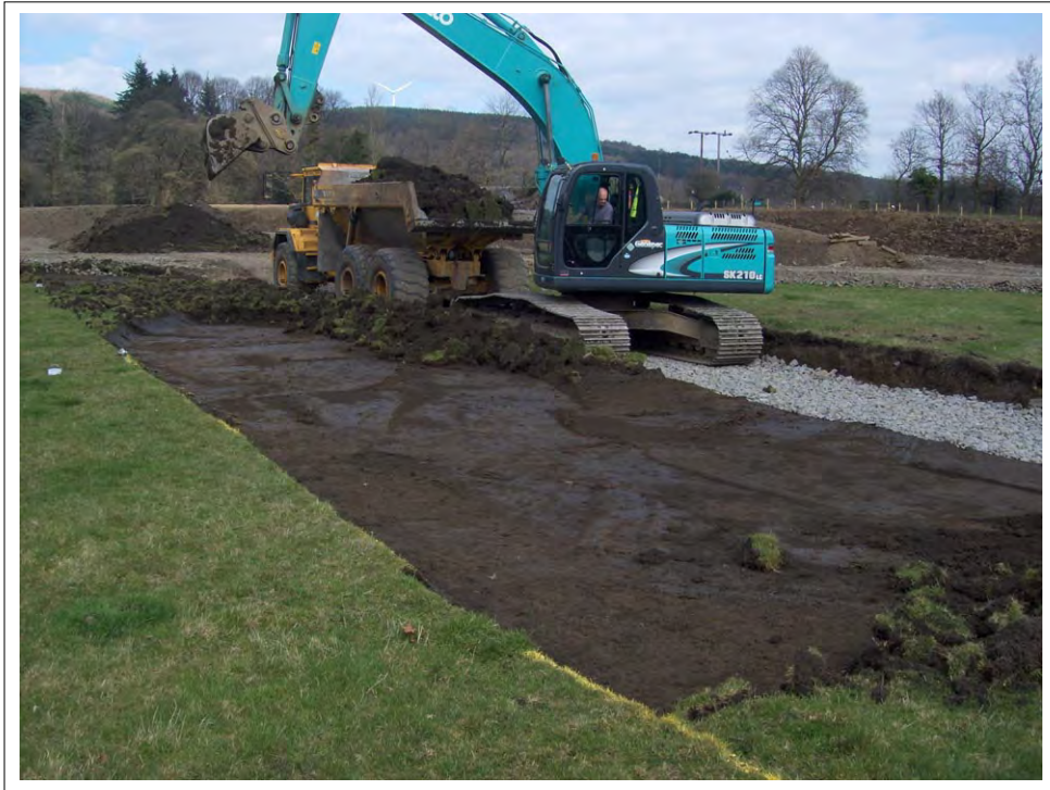
Plate 3: Area 2 under excavation
