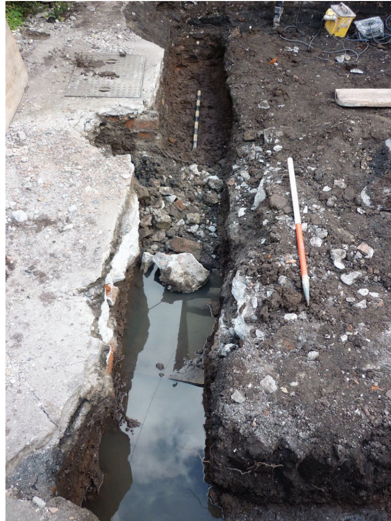
North-eastern trench - brick in centre of trench acting as a dam
