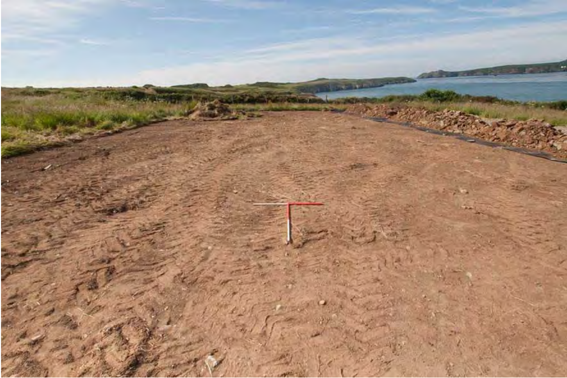
Photo 13: South facing view across the stripped area in the westernmost field, showing deposit 103. 1m scales.
