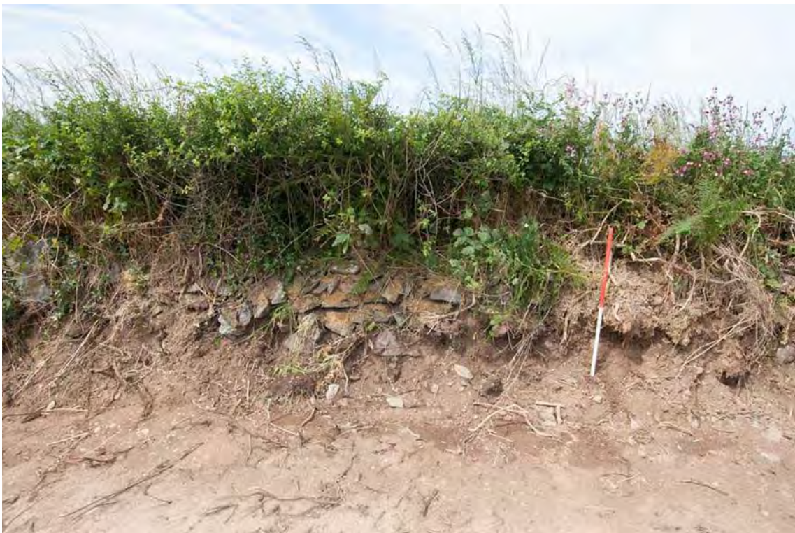
Photo 10: East facing shot of the field boundary between the two fields within the development area. 1m scale.
