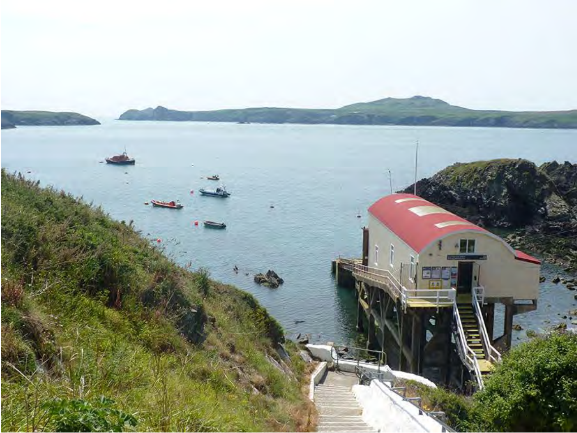
Photo 1: The existing St David's Lifeboat station.
