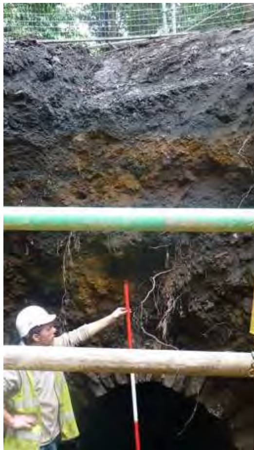
Photo 22: Backfill deposits above the culvert, also showing the dark layer of modern disturbance and overburden at the top. The partial scale shown is a 2m scale, divided into 0.5m segments.
