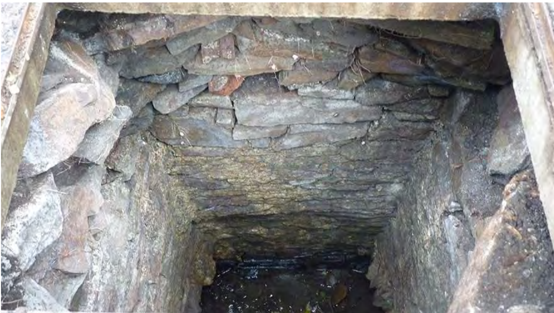
Photo 26: East facing shot of the manhole opening, showing the line of the culvert at the base running left to right and the mortared wall of the shaft topped by unmortared slightly corbelled stonework now carrying the modern concrete and metal manhole cover.
