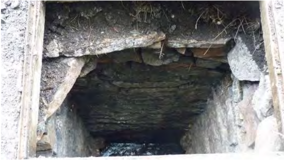
Photo 27: West facing shot showing the opposing side of the manhole shaft.
