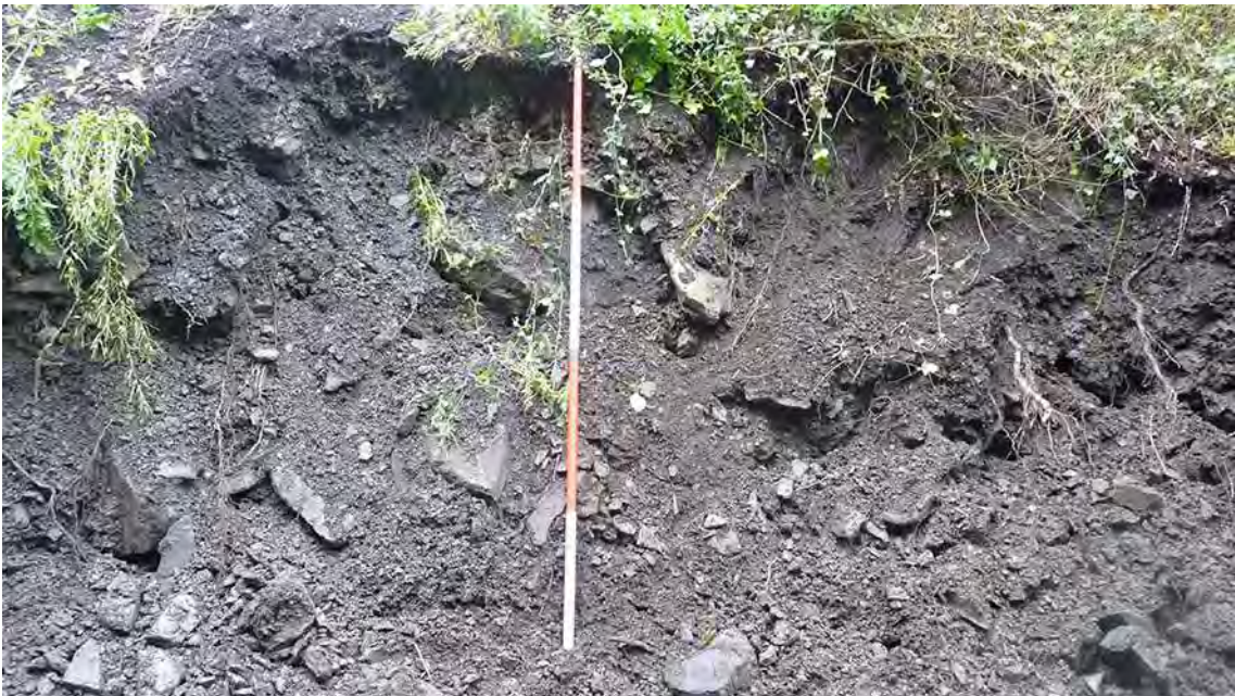
Photo 6: West facing shot of the edge of the scoured area at the base of the valley. Showing the current profile of the western side of the valley is made up of loose modern material. 2m scale.
