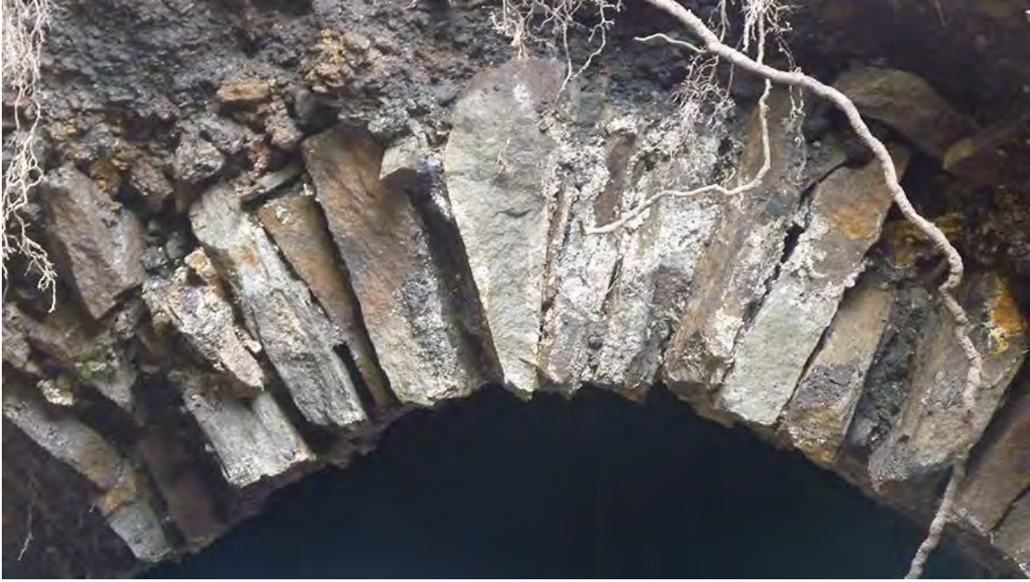
Photo 15: Detail of arched roof of culvert.
