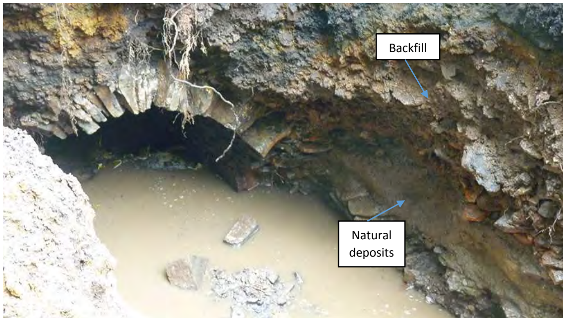
Photo 20: Southwest facing shot showing original natural stone and clay deposits into which the culvert is cut, with backfill deposits above.
