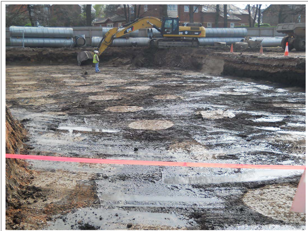
Plate 6: General view of Area 3 under excavation
