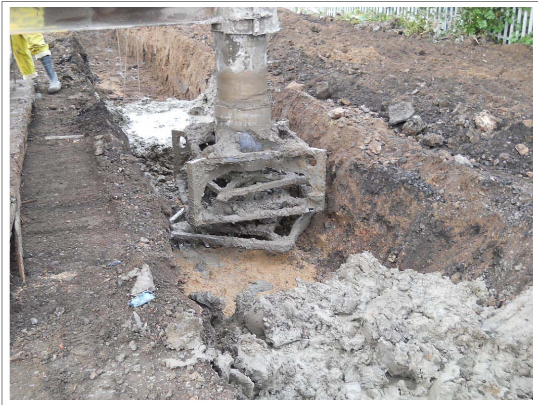
Plate 11:View of soil mixing within Area 3.
