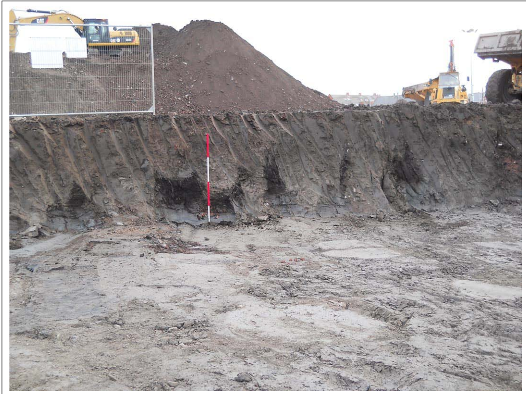
Plate 3: View of section edge within Area 1 showing intermittent peat deposits Scale 1x2m
