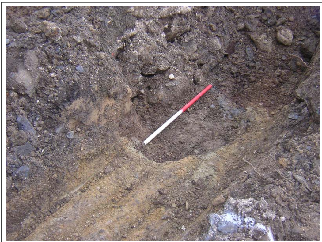
Plate 4: View of foundation cut for modern building demolished prior to excavation Scale 1x1m
