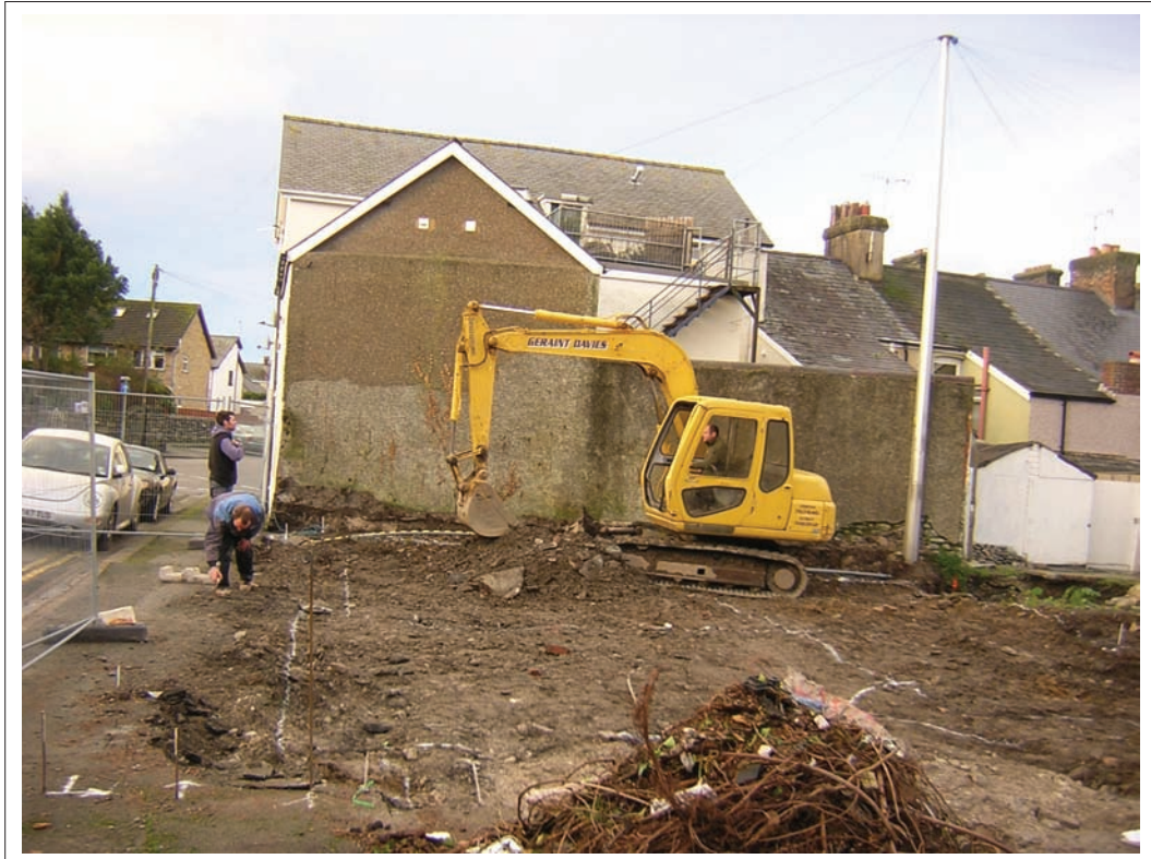
Plate 1: View west along street frontage during cutting of foundations
