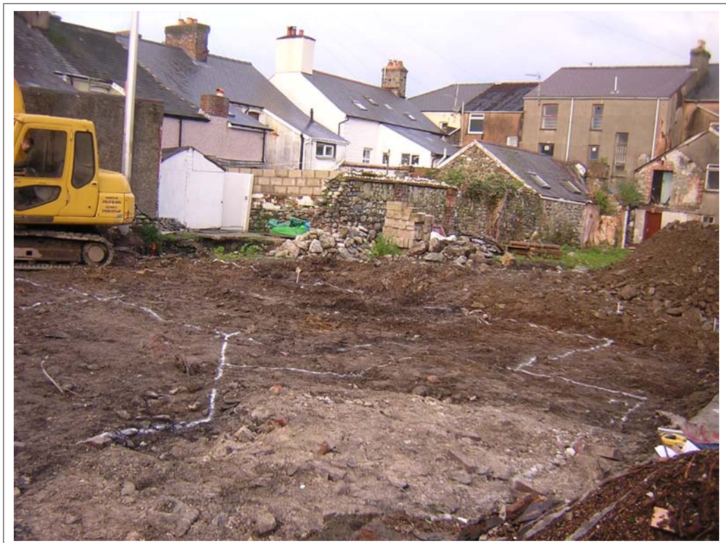
Plate 2: View north west across plot showing sprayed locations of foundation trenches
