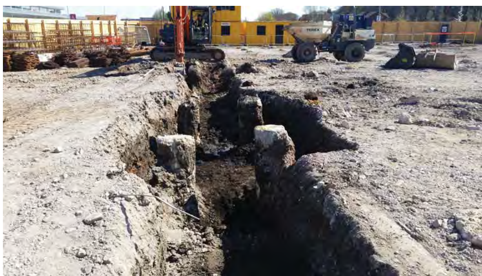
Plate 4 Foundation trench with peat revealed, viewed from the west
