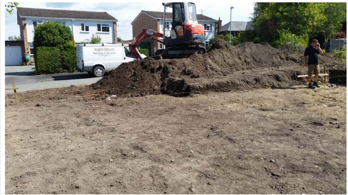
Plate 3: View north east across assessment area after levelling of ground
