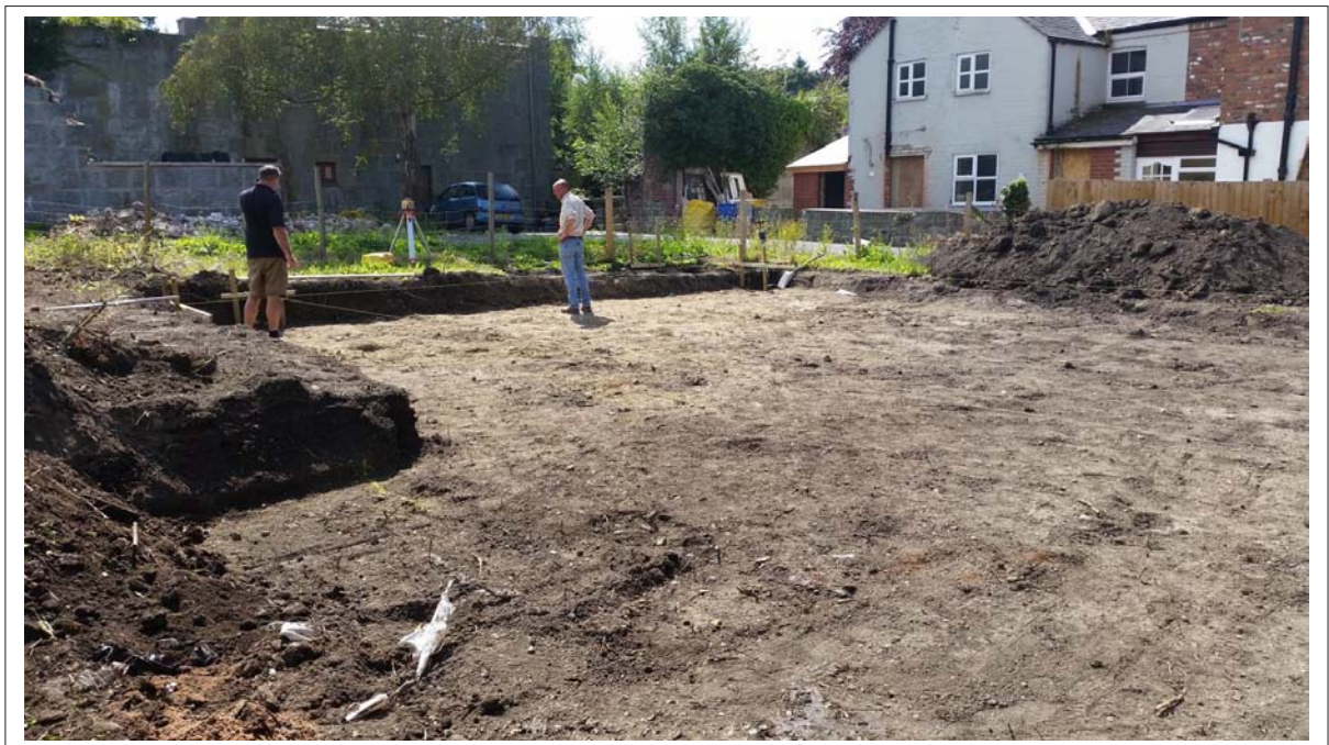
Plate 2: View south east across assessment area after levelling of ground
