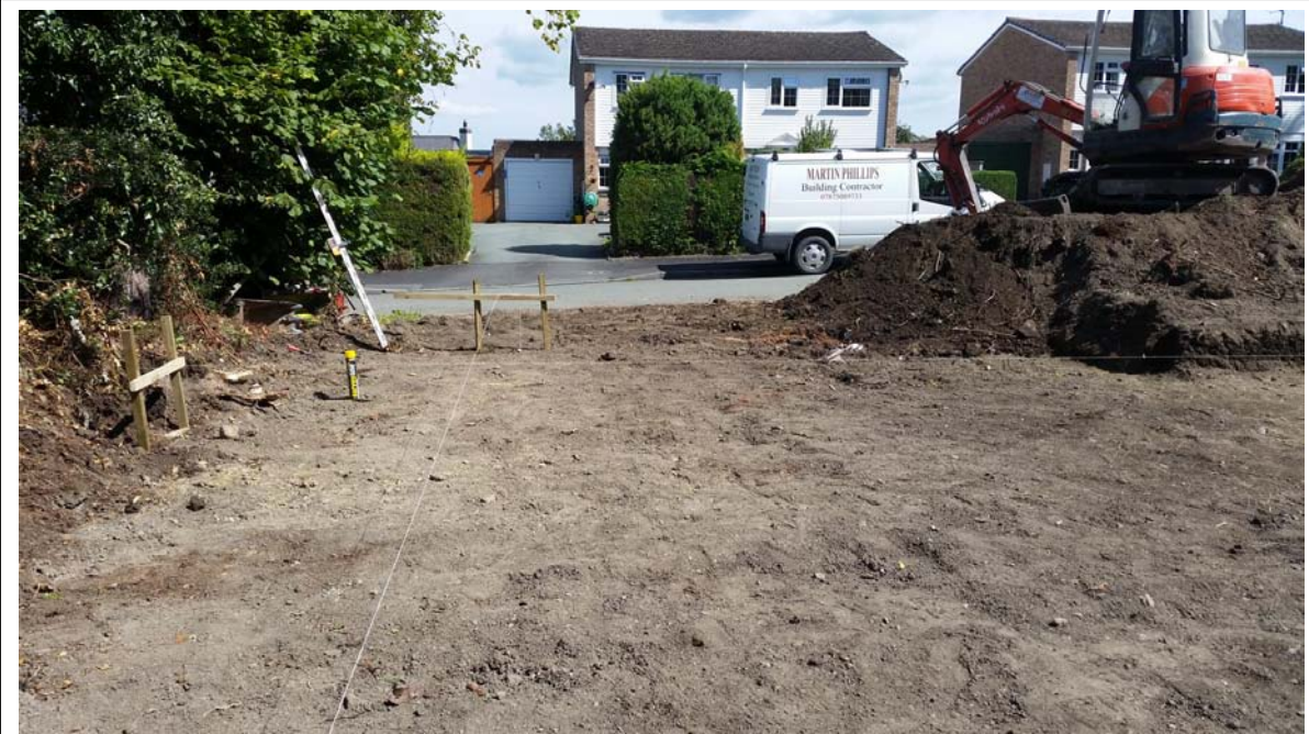
Plate 4: View north across assessment area after levelling of ground
