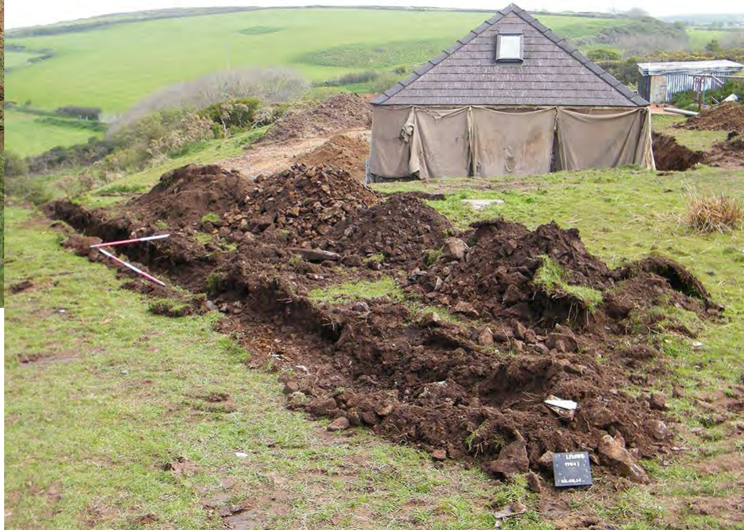
Fig. 14 Service trenches around the structure
