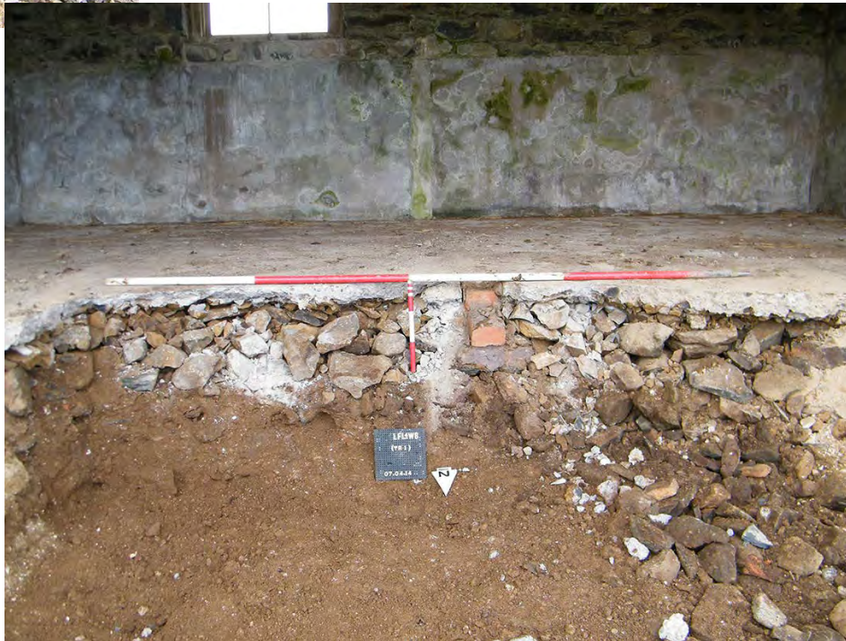
b. Section through concrete floor and underlying rubble deposit
