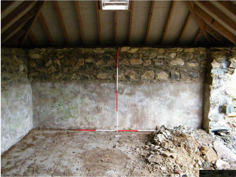
a. Intact concrete floor and wall covering
