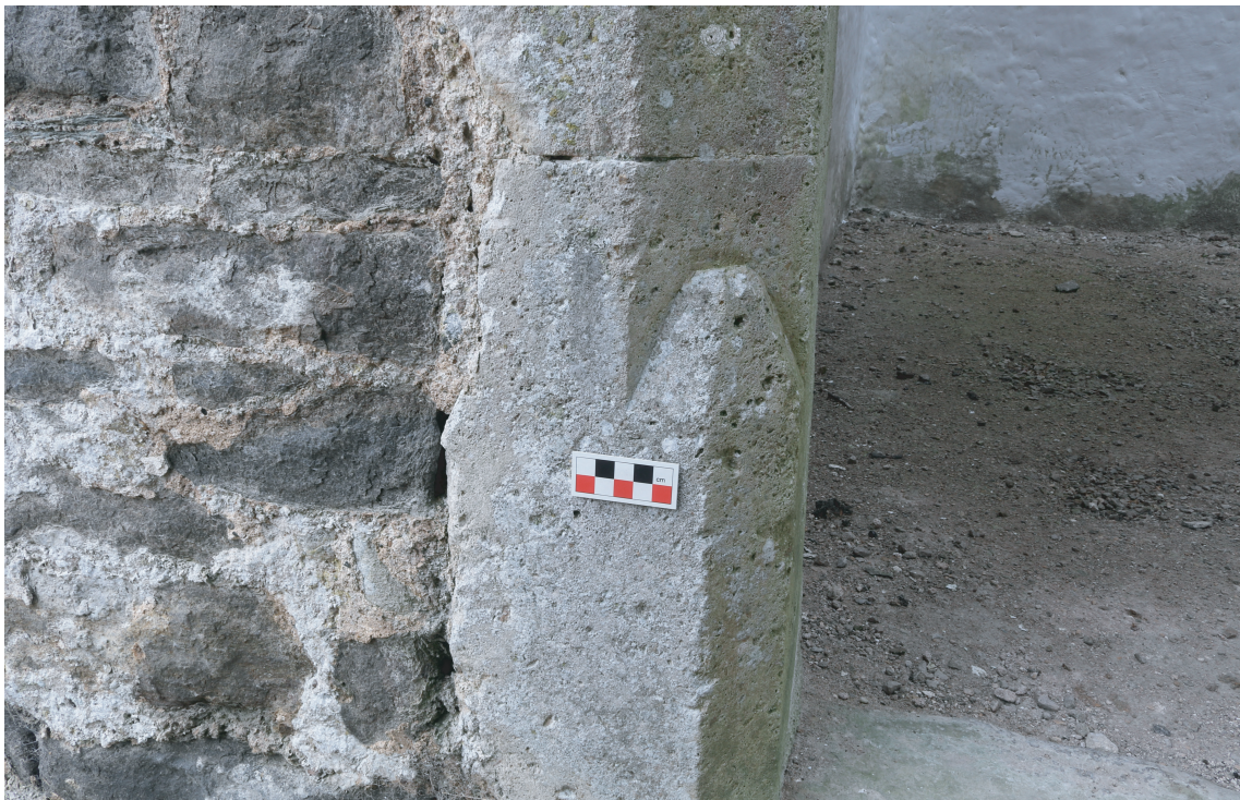
Plate 11. Old Beaupre - View of stop end in doorway into western room of Gatehouse. Looking W.
