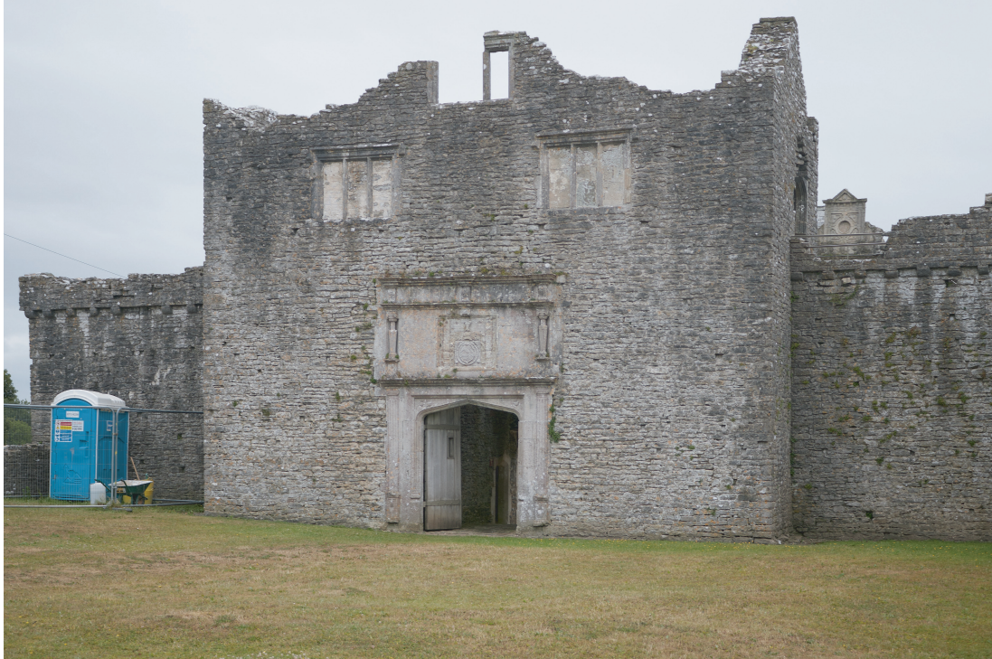
Plate 01. Old Beaupre - View of front elevation of Outer Gatehouse. Looking southeast.
